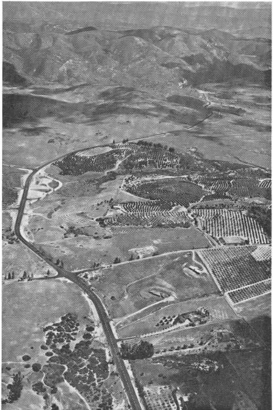
Improvement of the Del Dios Highway (shown here) was a co-operative federal-state-San Diego County project. This aerial view looking northeastward was taken near the west end of the project and shows the Rancho Santa Fe area in the foreground and the Lake Hodges Dam in the background.
