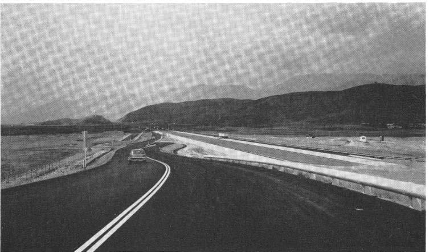
Two photos of recent construction of the San Bernardino Freeway show (upper) the new freeway looking south from the San Bernardino city limits and (lower) looking north from the vicinity of Highland Avenue.
