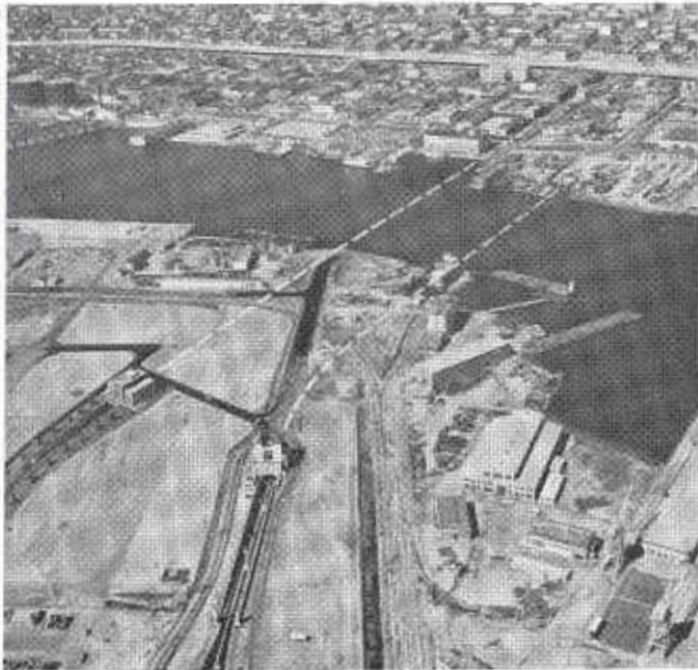
Location of the existing Posey Tube in the photo above is shown by the dotted white line on the right; the dotted line on the left indicates the location of the future Webster Street tunnel.
