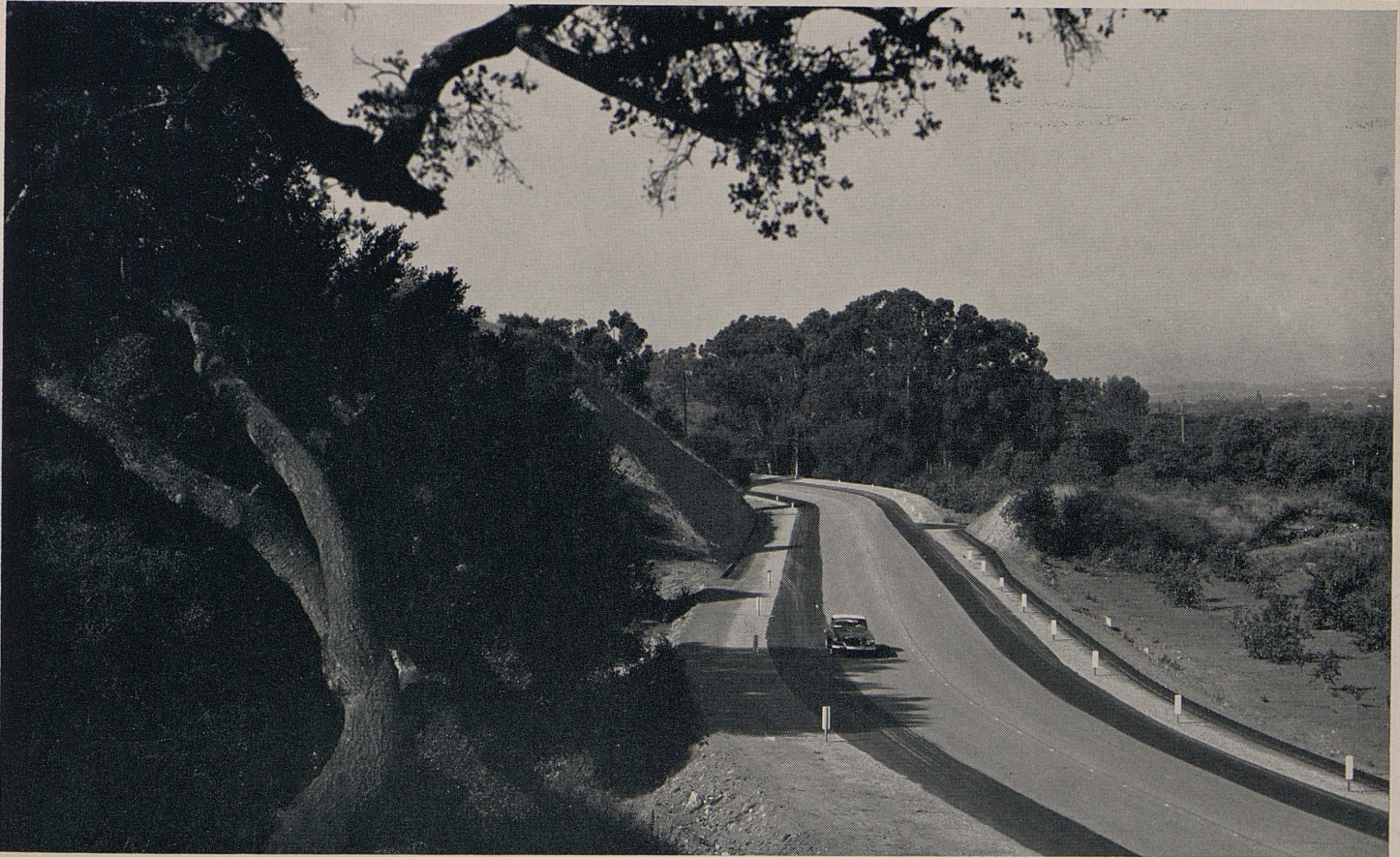
UPPER LEFT—A reconstructed section of Sign Route 41 in northern San Luis Obispo County. UPPER RIGHT—An aerial of the new section of US 101 freeway west of Santa Barbara near Elwood. LOWER—An improved section of Turnpike Road north of US 101 near Santa Barbara.
