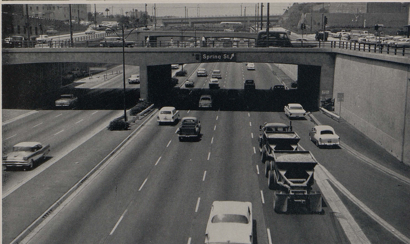
UPPER—This eastward view of the Santa Ana Freeway, taken from Los Angeles Street, shows the added lane for westbound traffic (extreme right). LOWER—A westward view of the Santa Ana Freeway at the Los Angeles Street on-ramp showing the added traffic lane occupied by the truck and trailer (right foreground).
