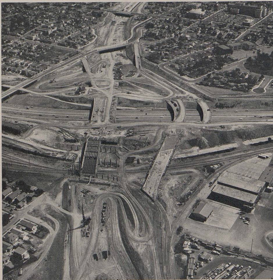
A southward view along the Golden State Freeway construction and the future interchange with the San Bernardino Freeway.
