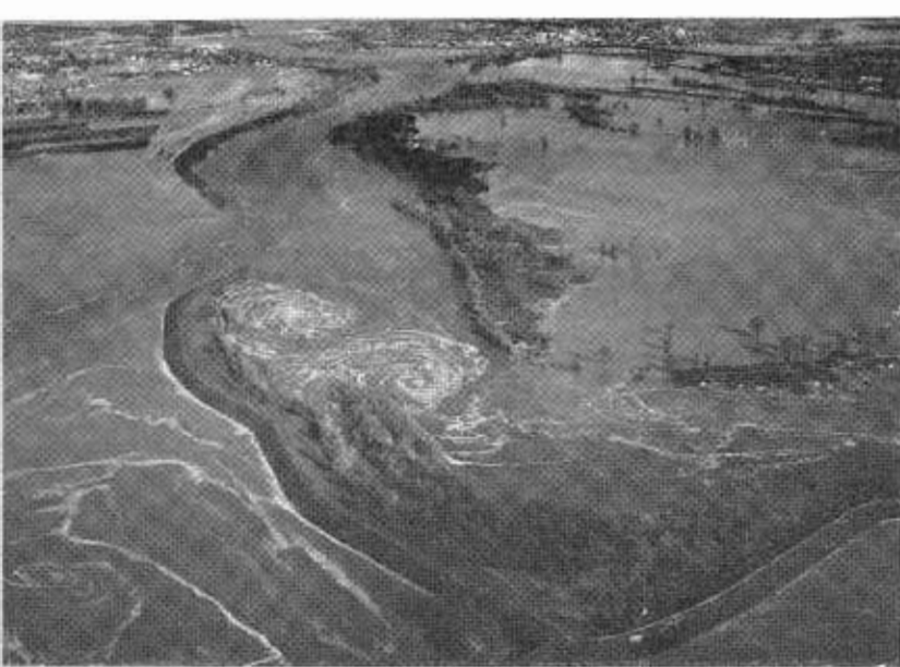
The Feather River levee which broke at Yuba City in the disastrous 1955 floods. State highway damage alone was more than $10,000,000.
