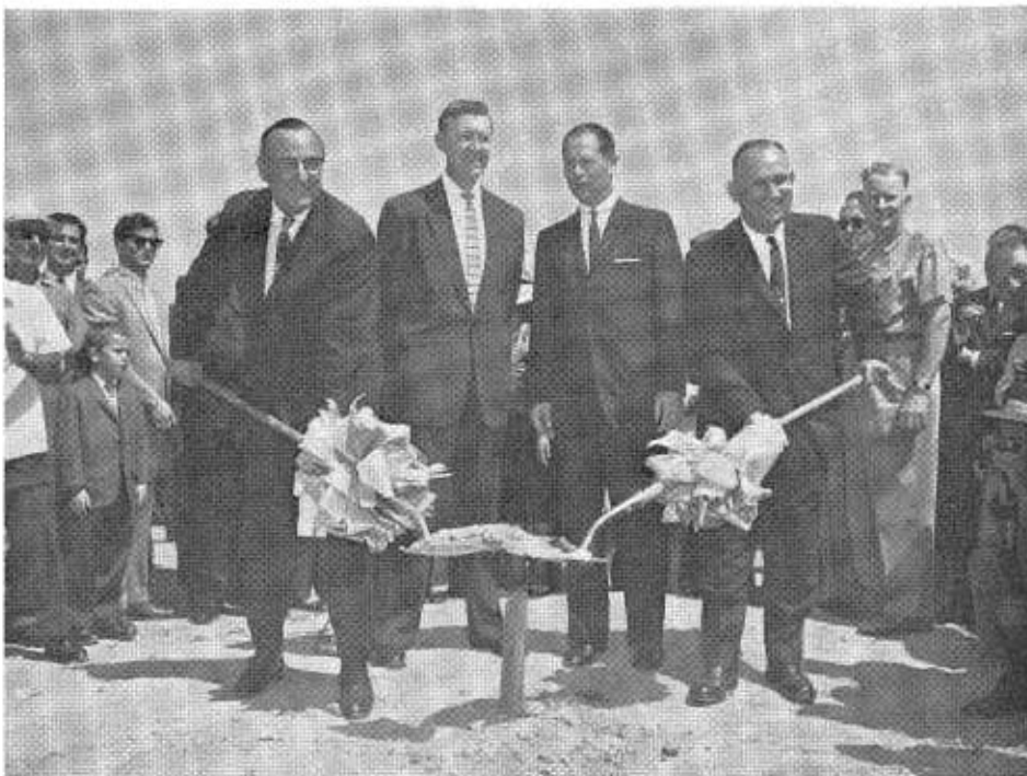
Signalling the start of actual work on the San Pedro-Terminal Island Toll Bridge project, Governor Edmund G. Brown (left) and Assemblyman Vincent Thomas of San Pedro wield the traditional ornated shovels at the project site on May 28. The two closest observers are (left to right) State Senator Richard Richards of Los Angeles County and Lieutenant Governor Glenn M. Anderson, who also took part in the open-air ceremonies attended by several hundred spectators.
