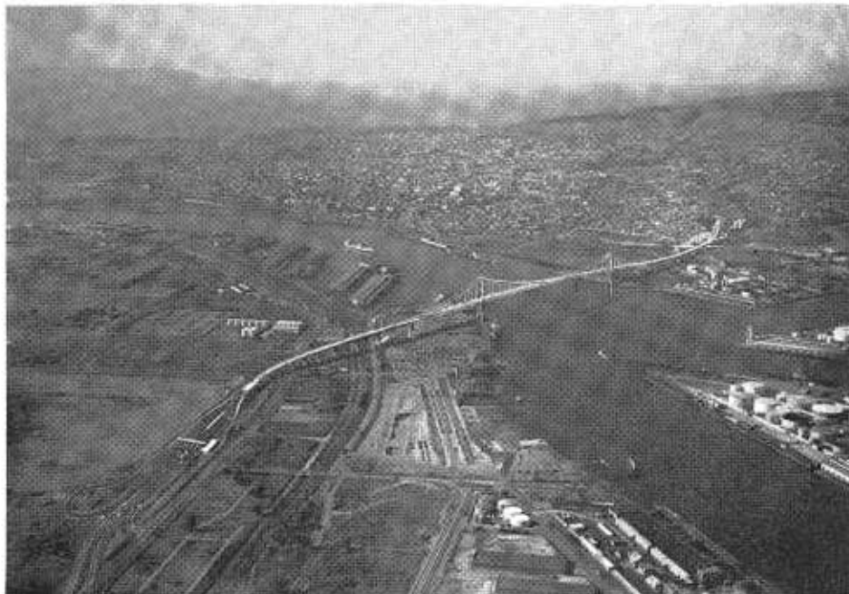
This drawing superimposed on an aerial photo by a Division of Highways artist shows how the new San Pedro-Terminal Bridge will appear after completion.
