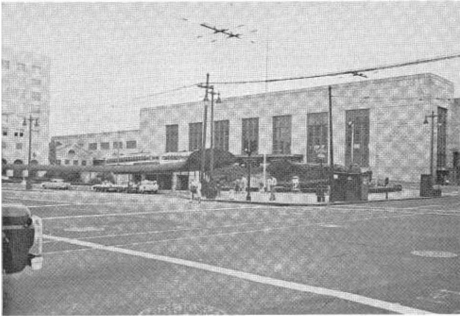
A ground view of the front of the Transbay Transit Terminal.
