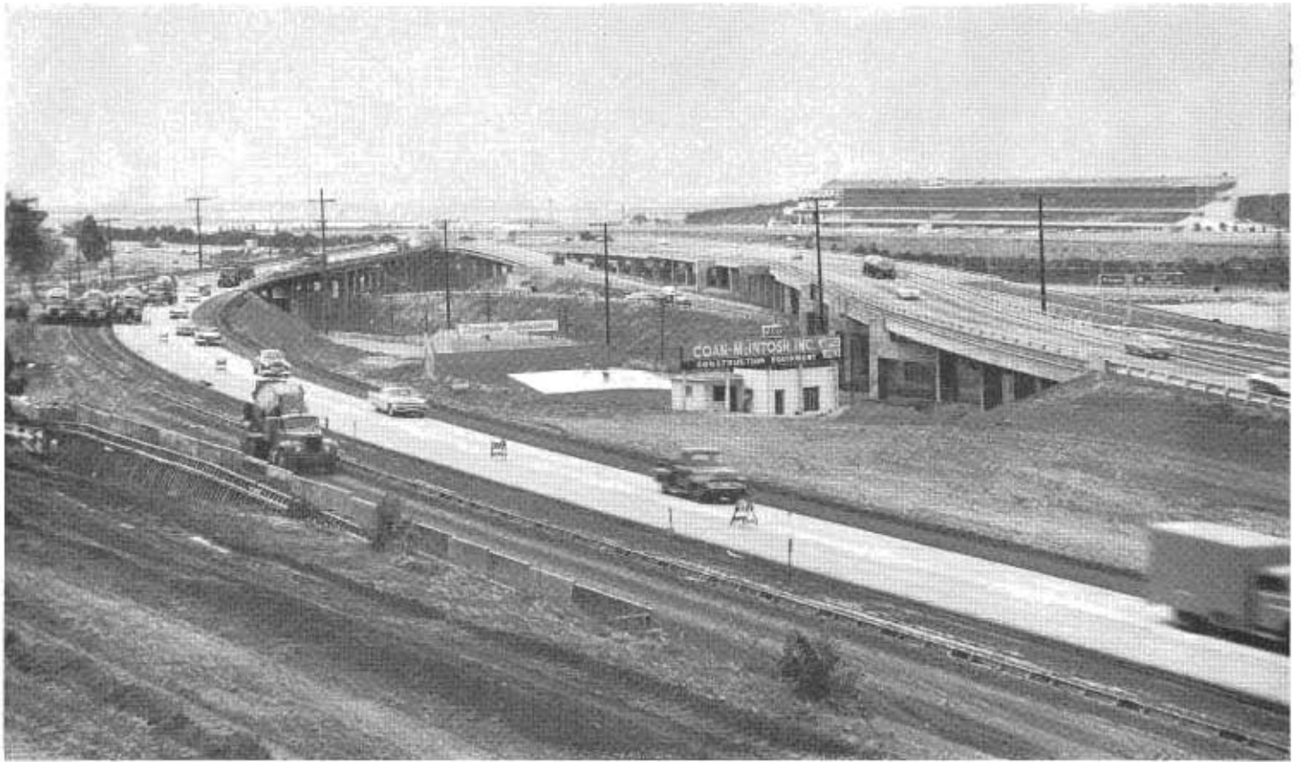
Provision was made to handle Eastshore Freeway traffic while construction on the El Cerrito overhead was underway. The view is southwest.
