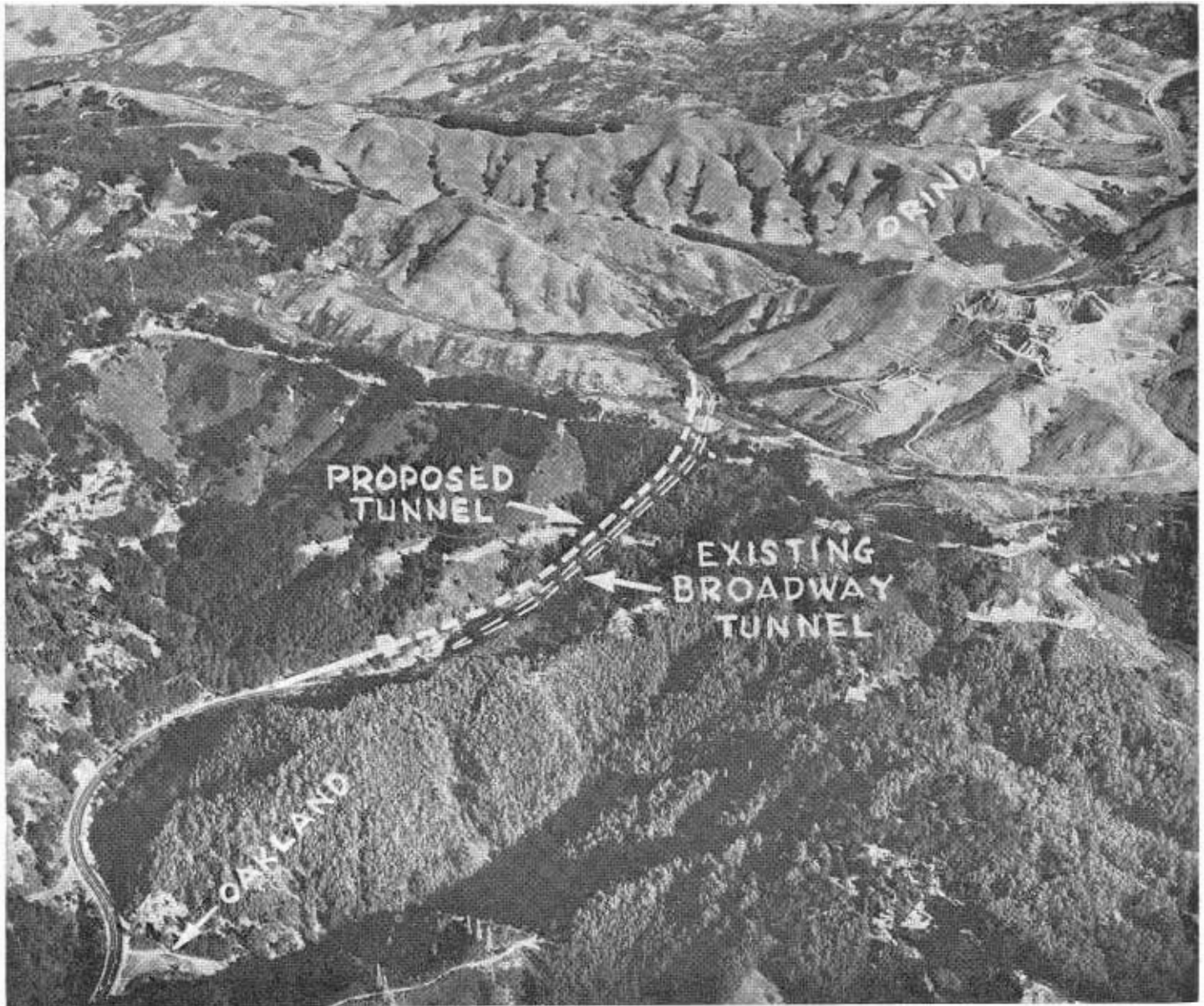
An aerial of the Berkeley Hills looking from eastward showing the location of the existing and proposed tunnels.
