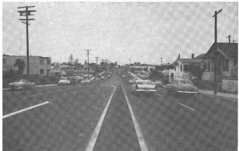
A view of Washington Street in San Diego after completion of a widening project.
