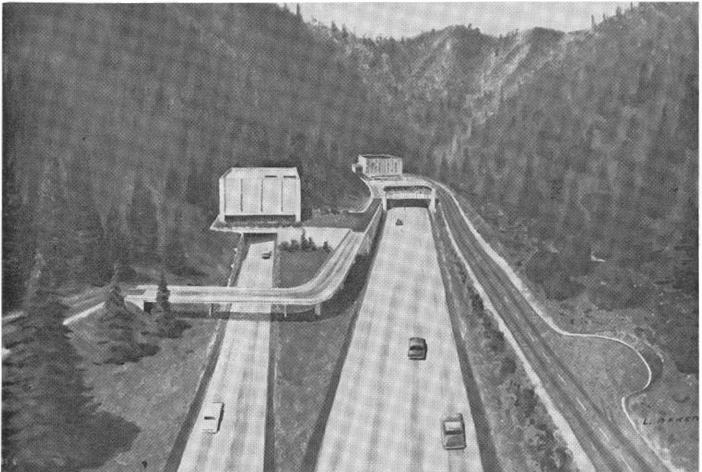
This artist's sketch shows how the Oakland approach to the Broadway Tunnel will look after completion of the new bore. The view is eastward, with the existing bores at the right and the new one at the left. The new portal building above the new tunnel will house the controls for all three bores, and will be reached by the new service roads shown in the sketch.
