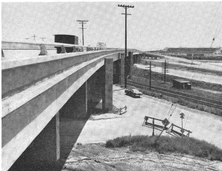
A side view of the same tee-beam bridge shown in the photo above.
