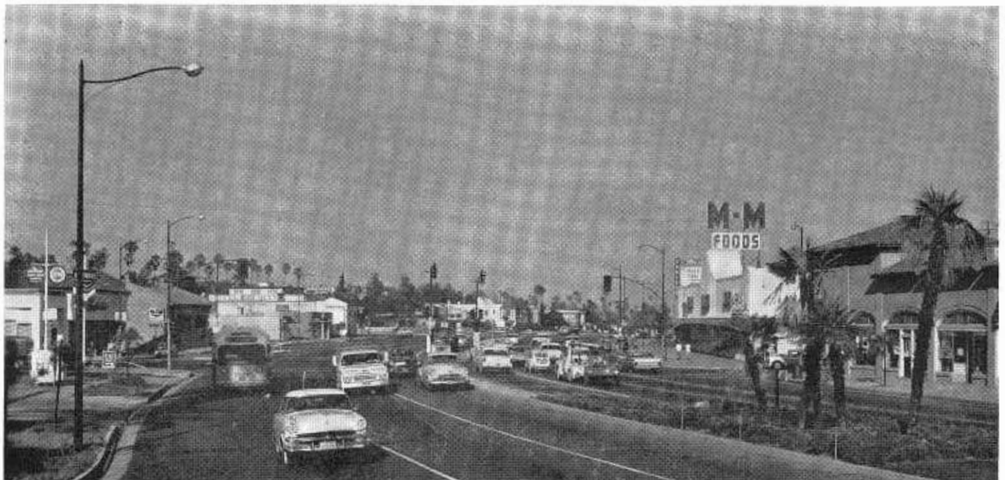
A photo of Huntington Drive in South Pasadena after it was widened to six traffic lanes, two parking lanes and an 18-foot median strip.
