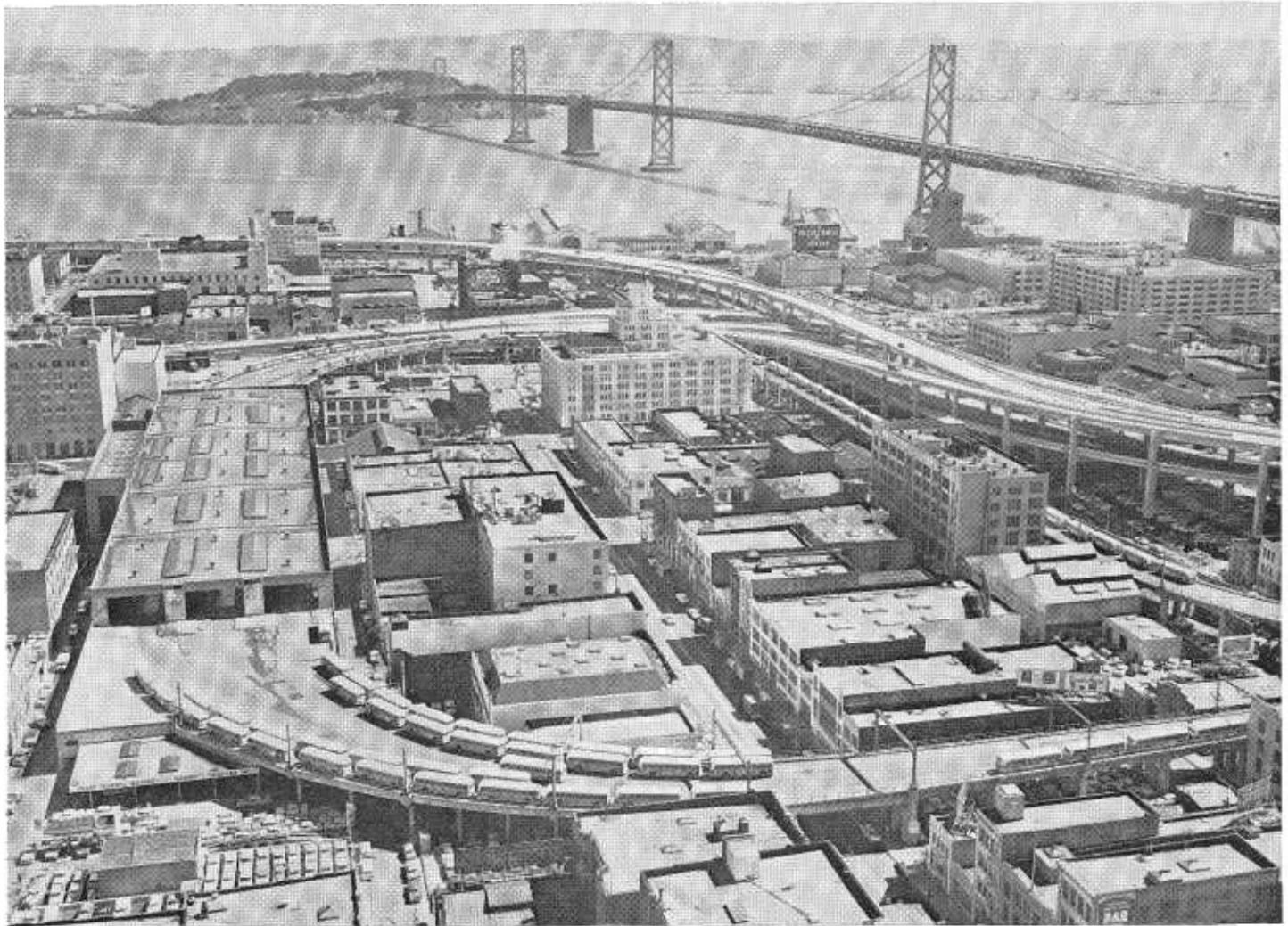
A view of the Transbay Transit Terminal and connecting loop viaduct looking eastward with the Bay Bridge in the background.
