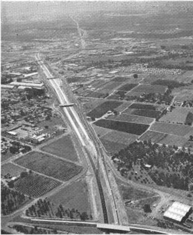
Looking westward on US 101 (Bayshore Freeway) toward the new interchange with the Nimitz Freeway (left background).
