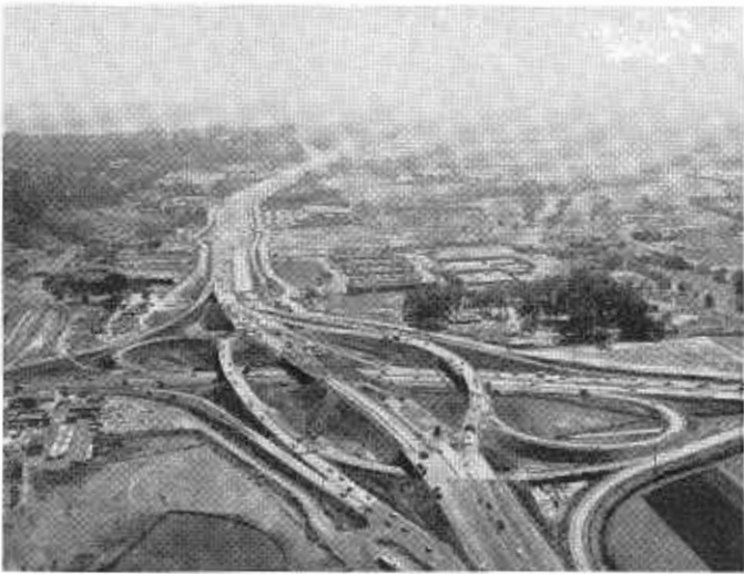
A photo showing typical traffic density during the construction of the US 80-395 Interchange.
