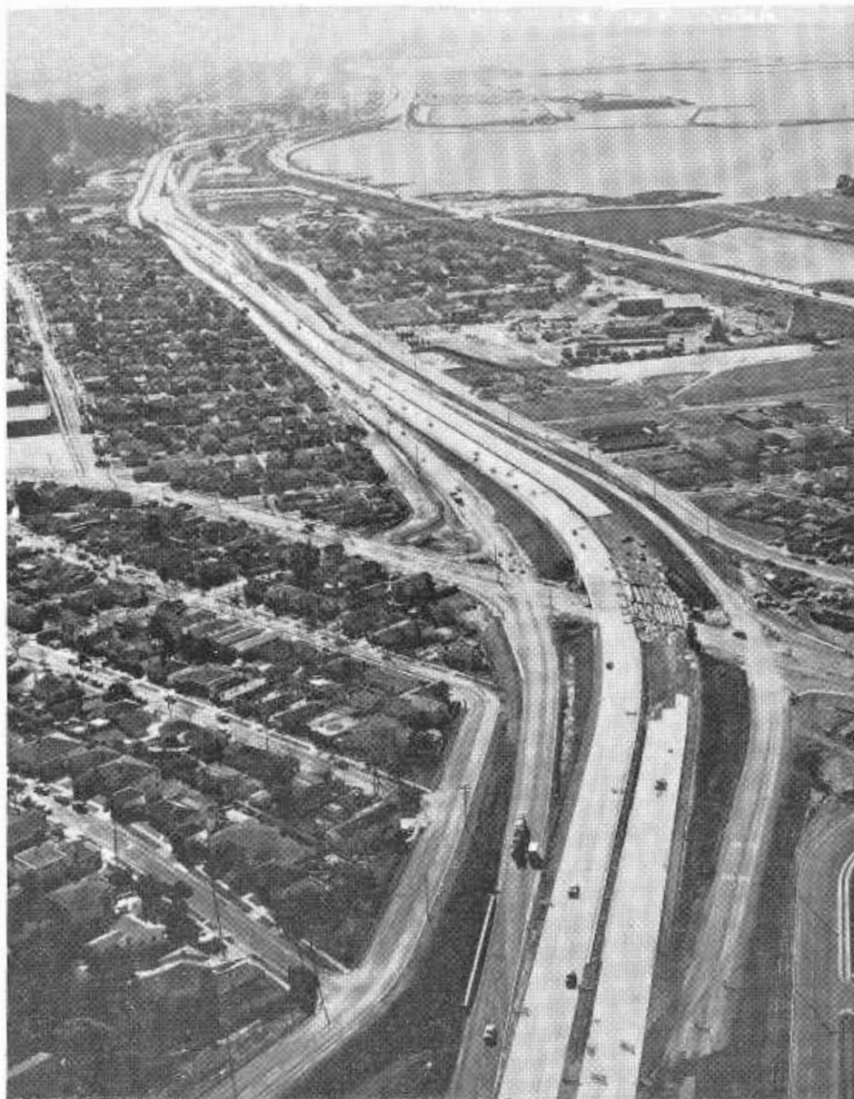
An aerial looking southward along the new section of US 40 in Richmond toward the Eastshore Freeway. The Carlson Avenue interchange is in the foreground.
