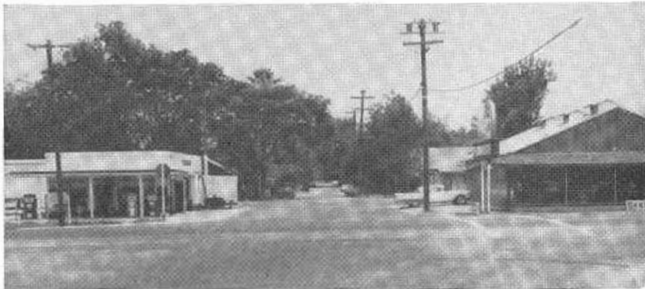
This photo shows a portion of 15th Street in Live Oak, Sutter County, after it was improved.
