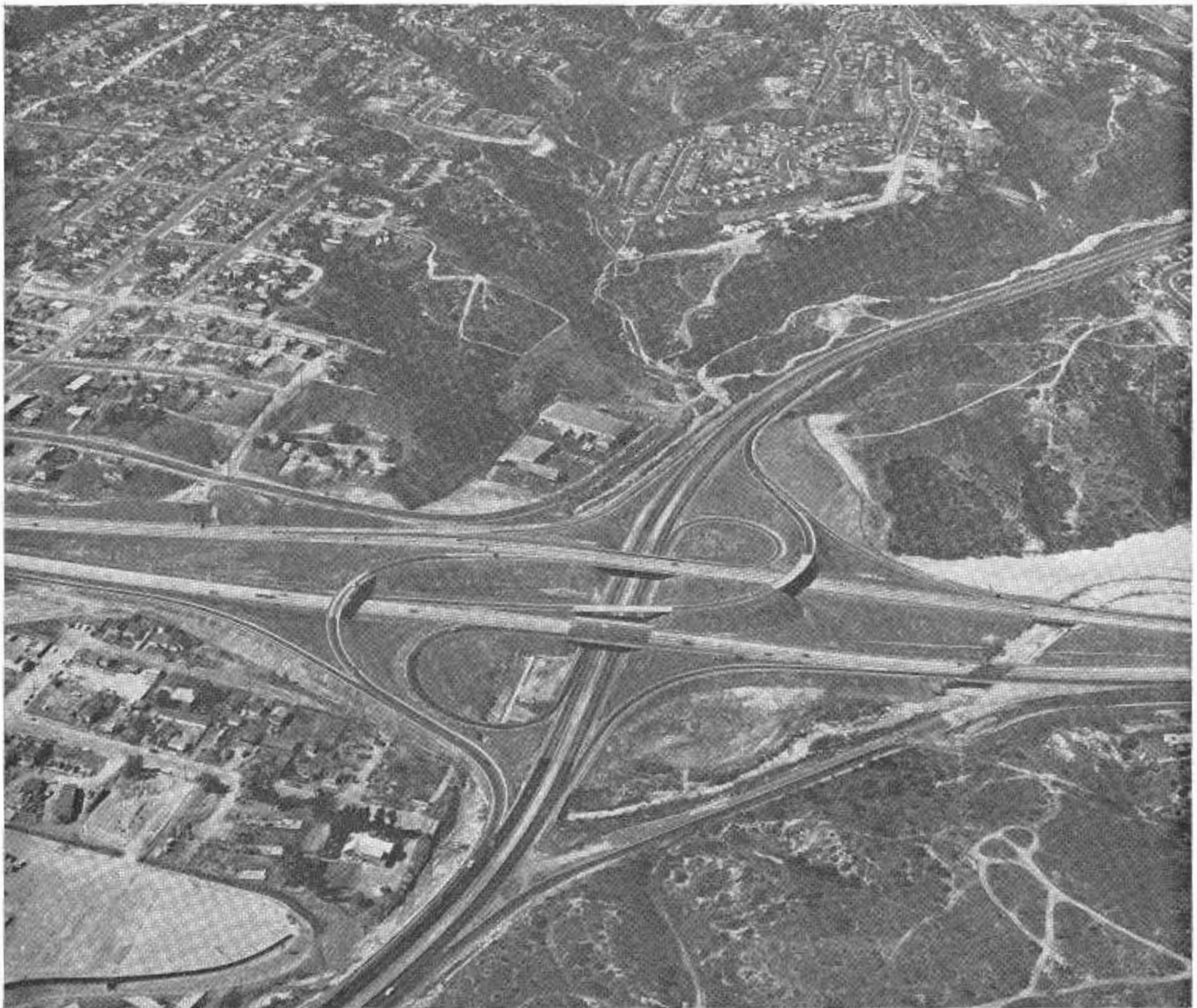
The photo looking north along Wabash Boulevard, shows the new Sign Route 94 Interchange. The original interchange built by the city included the eastbound bridge on Sign Route 94 (dark surfaced structure near center of photo) and a portion of the cloverleaf and right-turn ramps. State construction of Sign Route 94 as an eight-lane freeway necessitated expansion of the interchange as shown in this photo.
