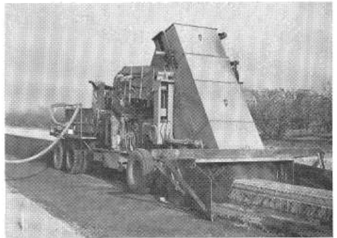
The "monster" achieved a production rate on cement-treated subgrade of 6.4 cubic yards a minute.
