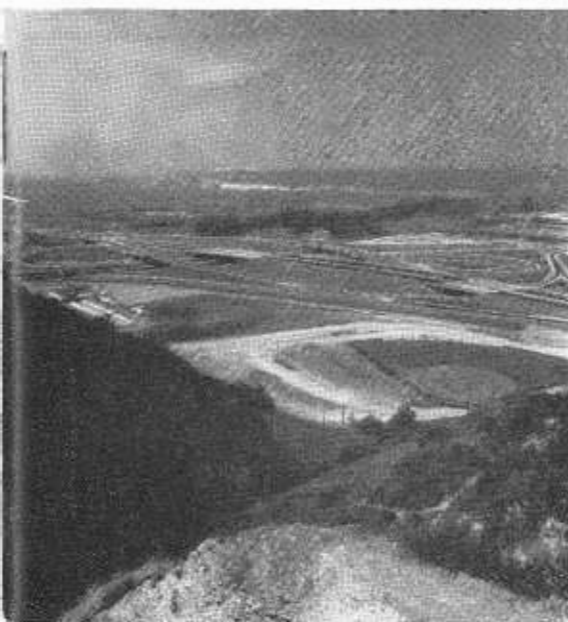
BACK COVER—A photo of the reconstructed Mission Valley interchange which connects US 80 (upper level) with US 395 (lower level) in San Diego. The view, taken from the high ground south of the interchange, is northwestward. (See the article "US 80-395" in this issue.) Photo by Bill Ruland
