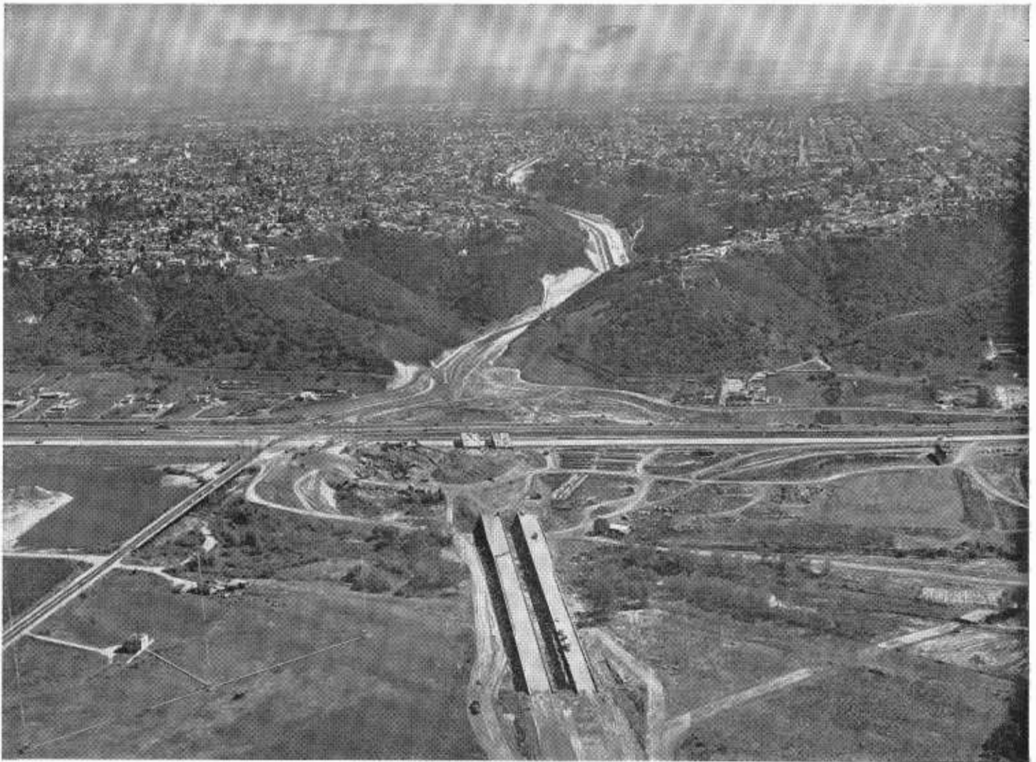
The above photo is looking south along Murphy Canyon Road and Ward Road, with US 80 running horizontally through the center of the picture. New bridges over the San Diego River are in the foreground. Construction on Ward Road is a city-county financed project.
