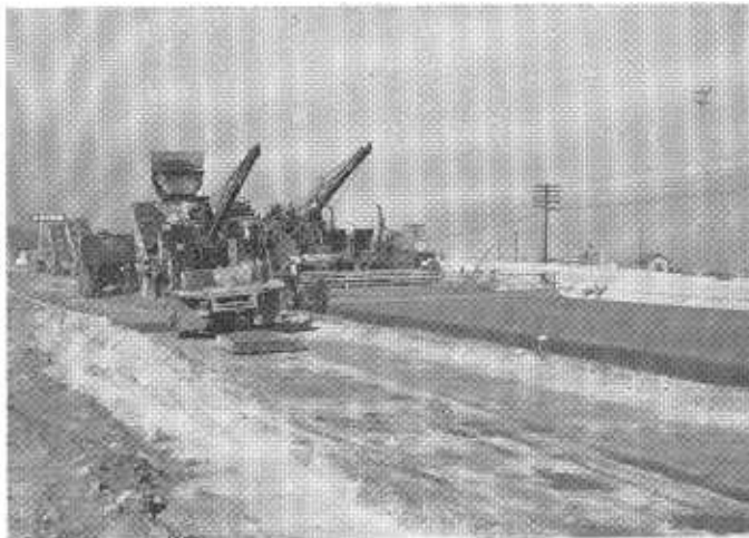
The electronically controlled and guided slip form paver in action.
