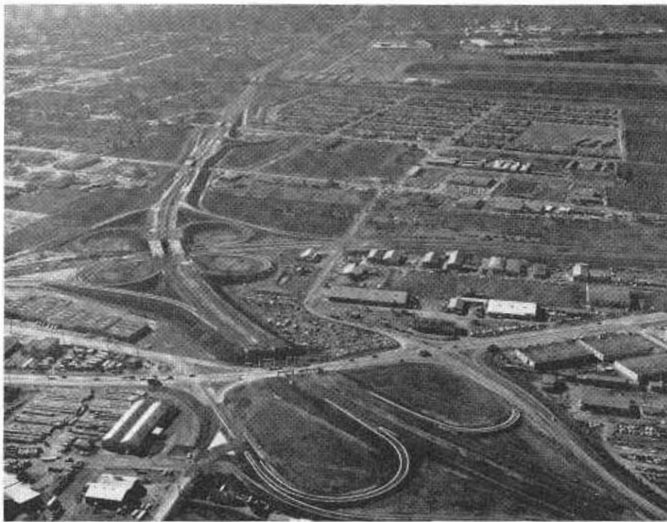
Looking southerly at the site of construction for interchange facilities between Sign Route 17 and US 101 Bypass (Bayshore) near San Jose. Old Bayshore Highway Intersection in foreground, new Nimitz-Bayshore Interchange in center.
