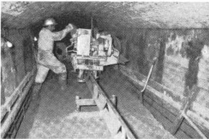
Pouring the floor slab with a monorail unit.
