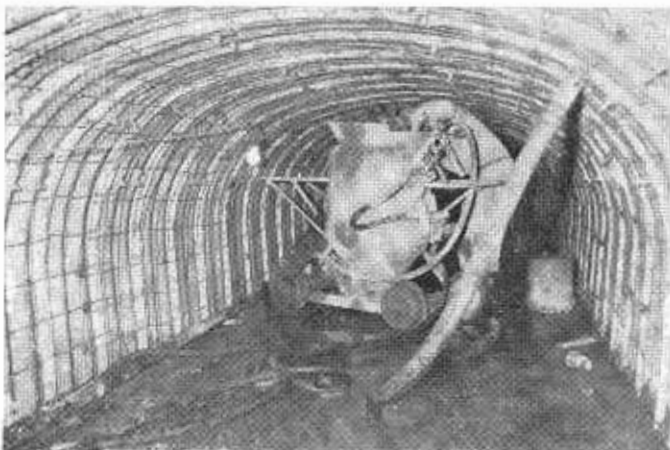
Forcing grout between the new and old tunnel lining.
