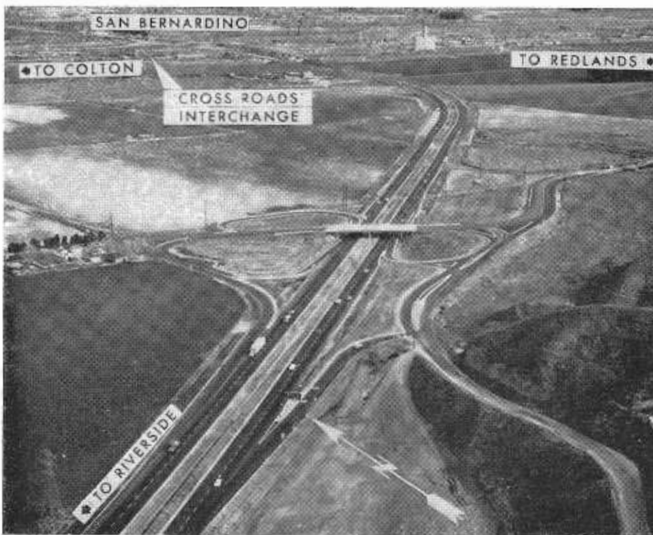
The north portion of the newly completed section of the Riverside Freeway.
