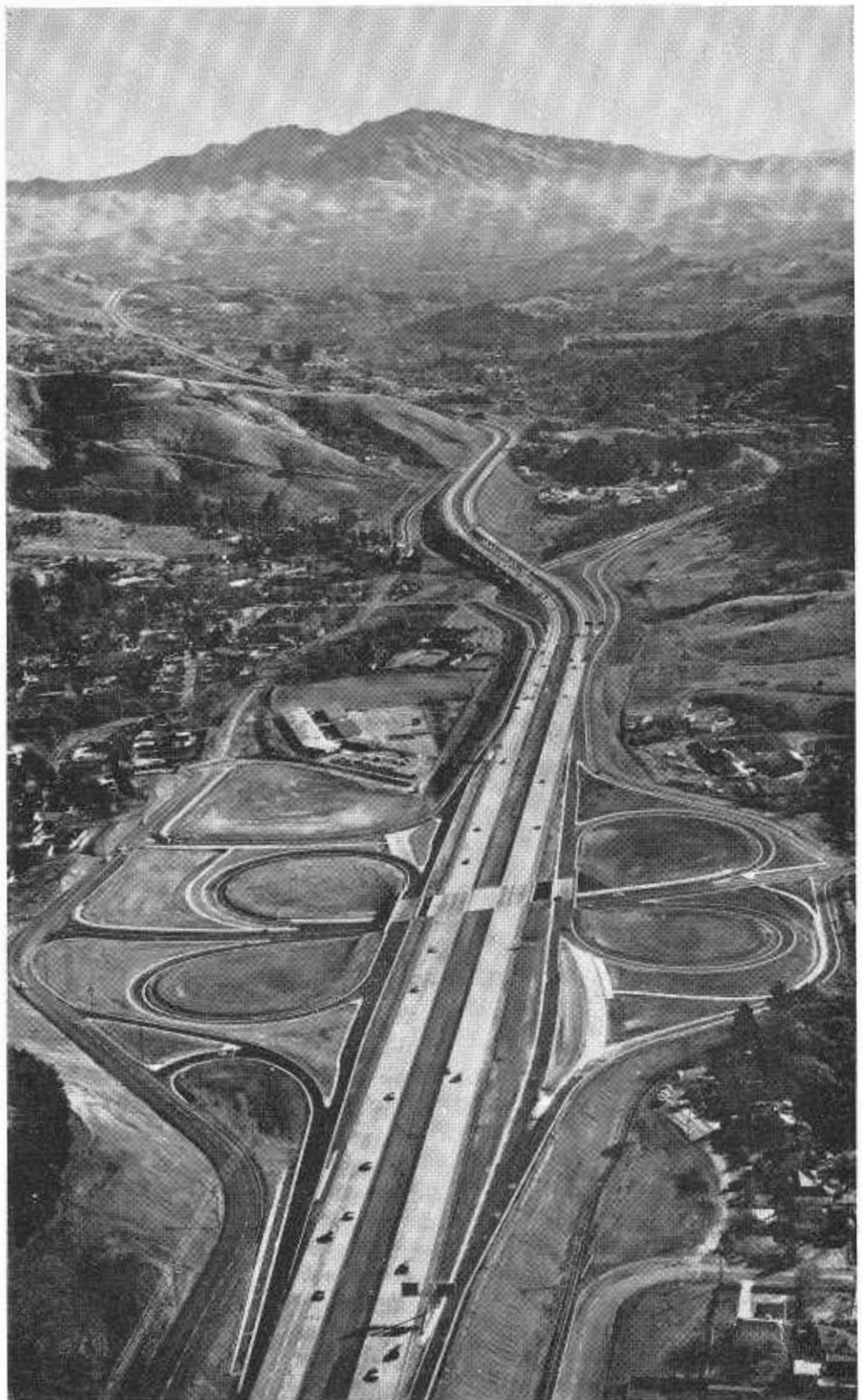
Looking east along Sign Route 24 toward Mt. Diablo with Acalanes Valley Road Interchange in foreground.
