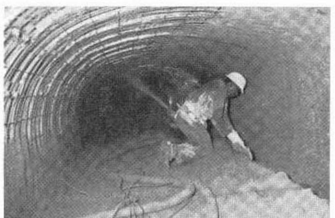
Applying air-blown mortar to the inside of the new tunnel lining.
