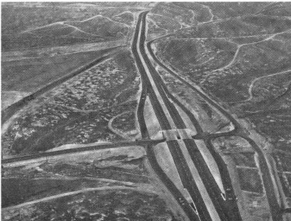
A "diamond" interchange on the Alfred Harrell Highway between Bakersfield and Hart Memorial Park.
