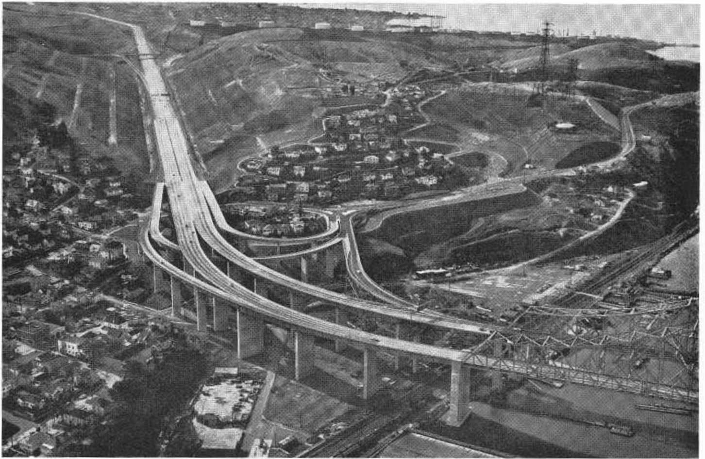
Looking southwest over the Crockett Interchange from the Carquinez Bridge, through the "big cut."
