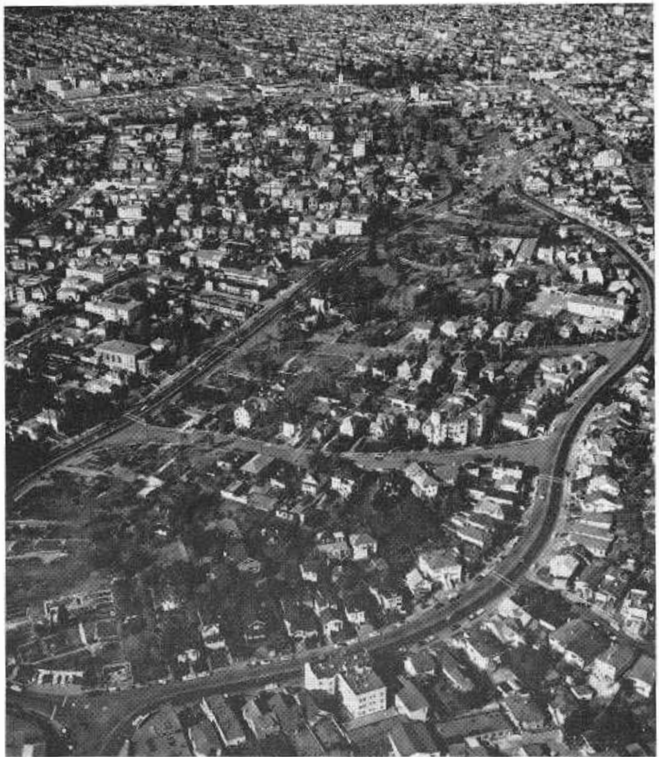
Looking westerly across Oakland residential area from vicinity of Grand Avenue, showing right of way clearance for proposed MacArthur Freeway.
