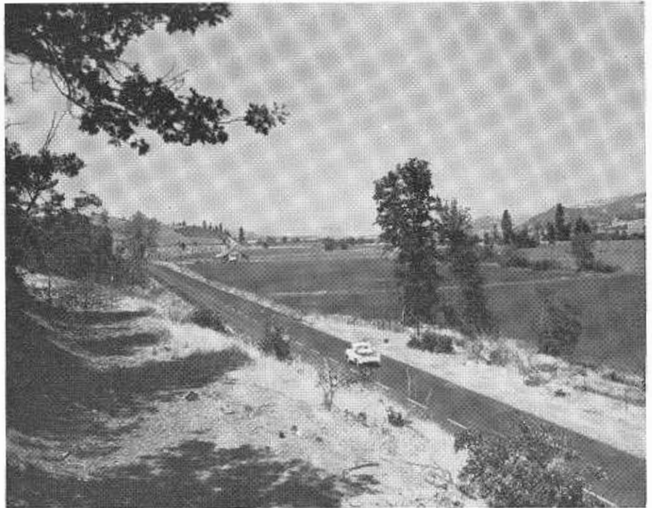
A recently improved section on FAS 1089 at the south end of Scott Valley in Siskiyou County.
