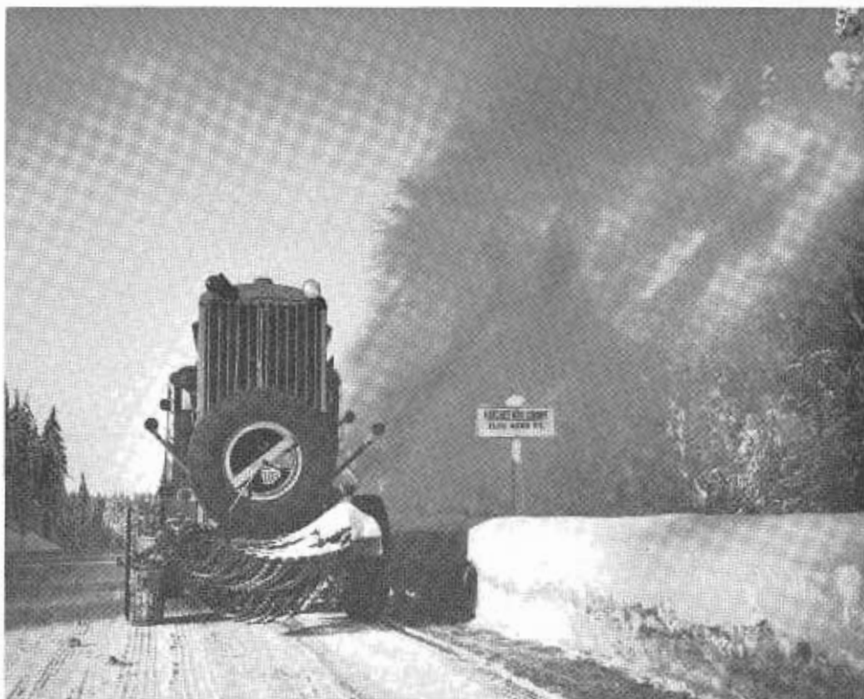
Snow removal operations at the summit.
