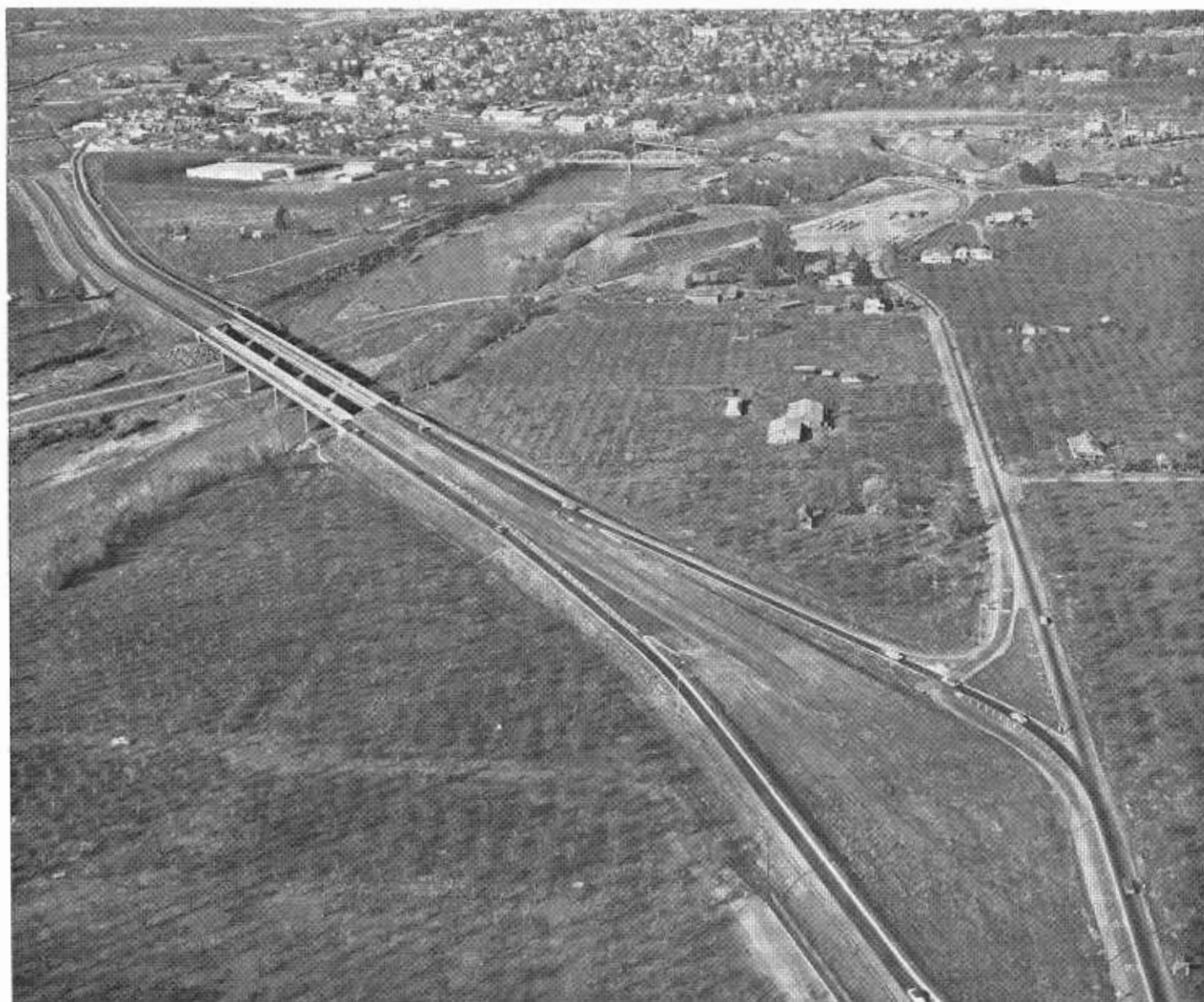
Healdsburg Bypass, looking east from intersection of new construction with existing highway at Grant. City of Healdsburg in background. Russian River in center with bridge crossings (left to right) at freeway, old highway and NWP Railroad.
