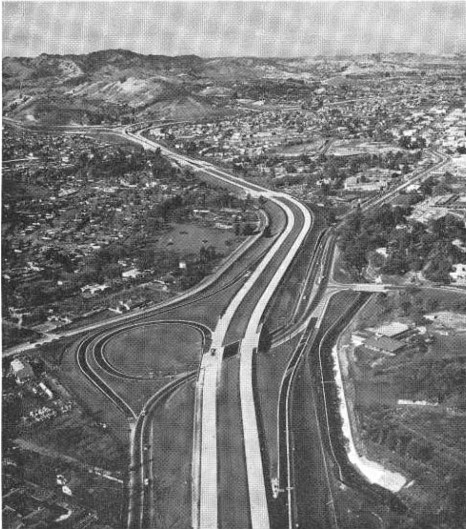
South Main Street Interchange on SSR 24 in Walnut Creek, with new Walnut Creek "Y" Interchange in upper left.
