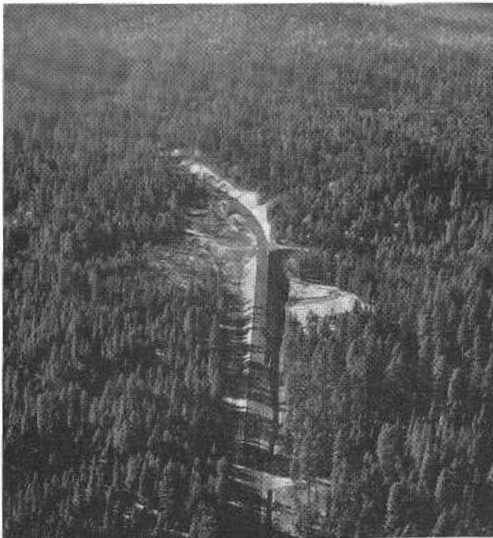
West from Burney Valley showing nearly completed expressway.
