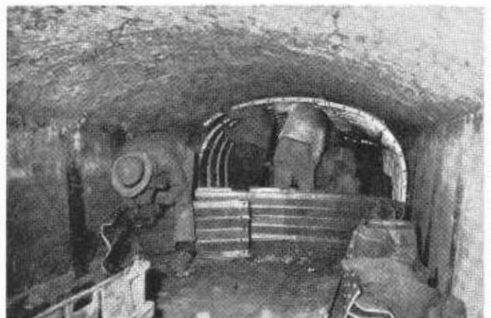
A crew placing the tunnel liner.
