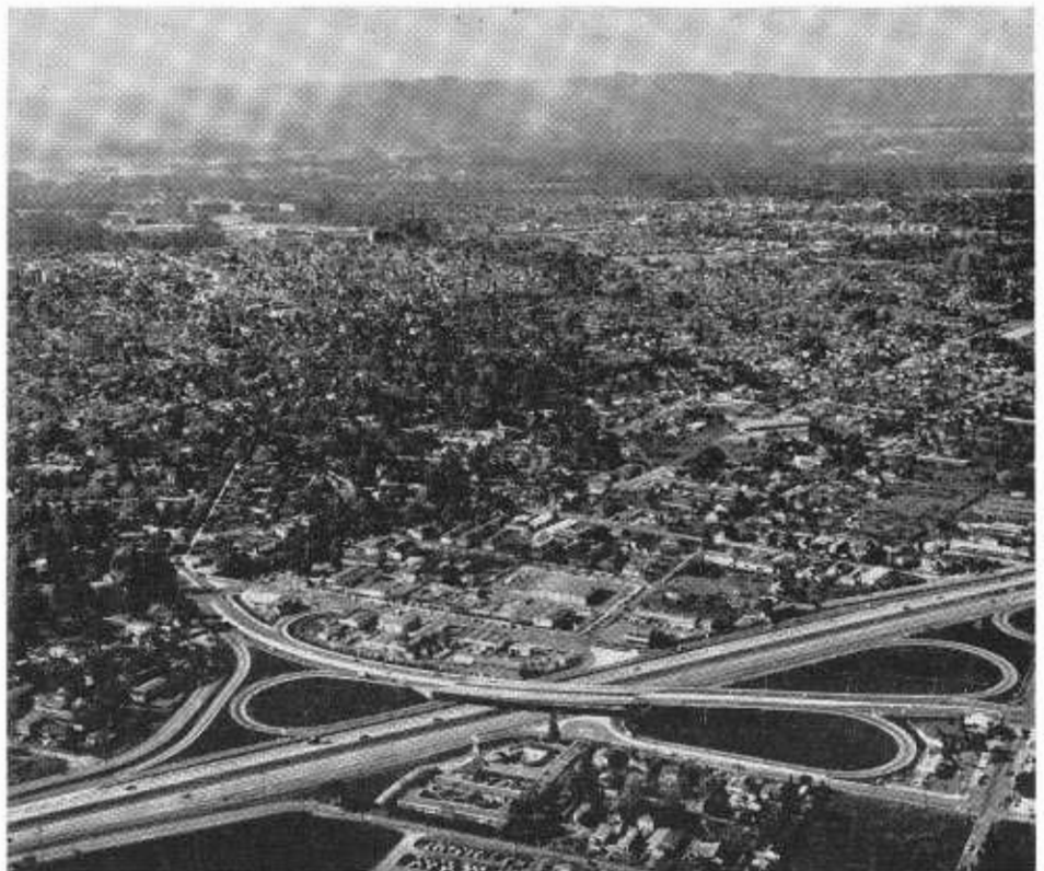
Looking westerly across the University Avenue Interchange on Bayshore Freeway in the City of Palo Alto.
