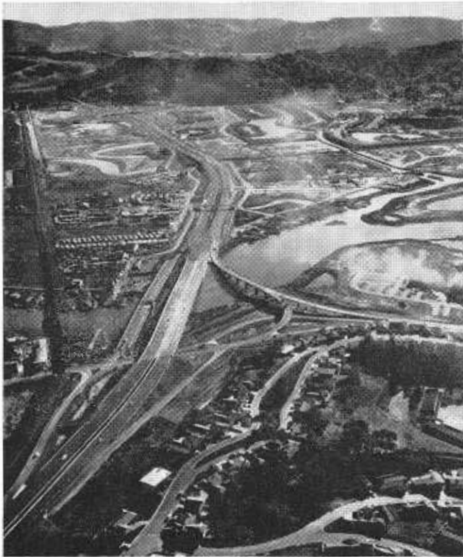
Greenbrea Interchange in Marin County on US 101 at Corte Madera Creek, looking south. Corte Madera Interchange structure in upper left background.
