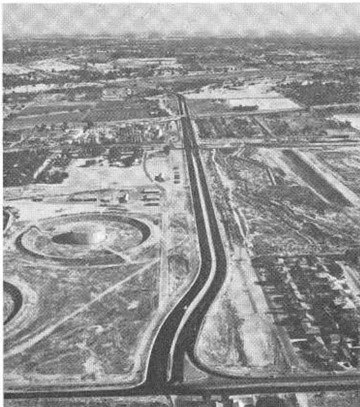
Looking south at expressway portion of FAS Route 887 on Manor Street in Oildale, Kern County.
