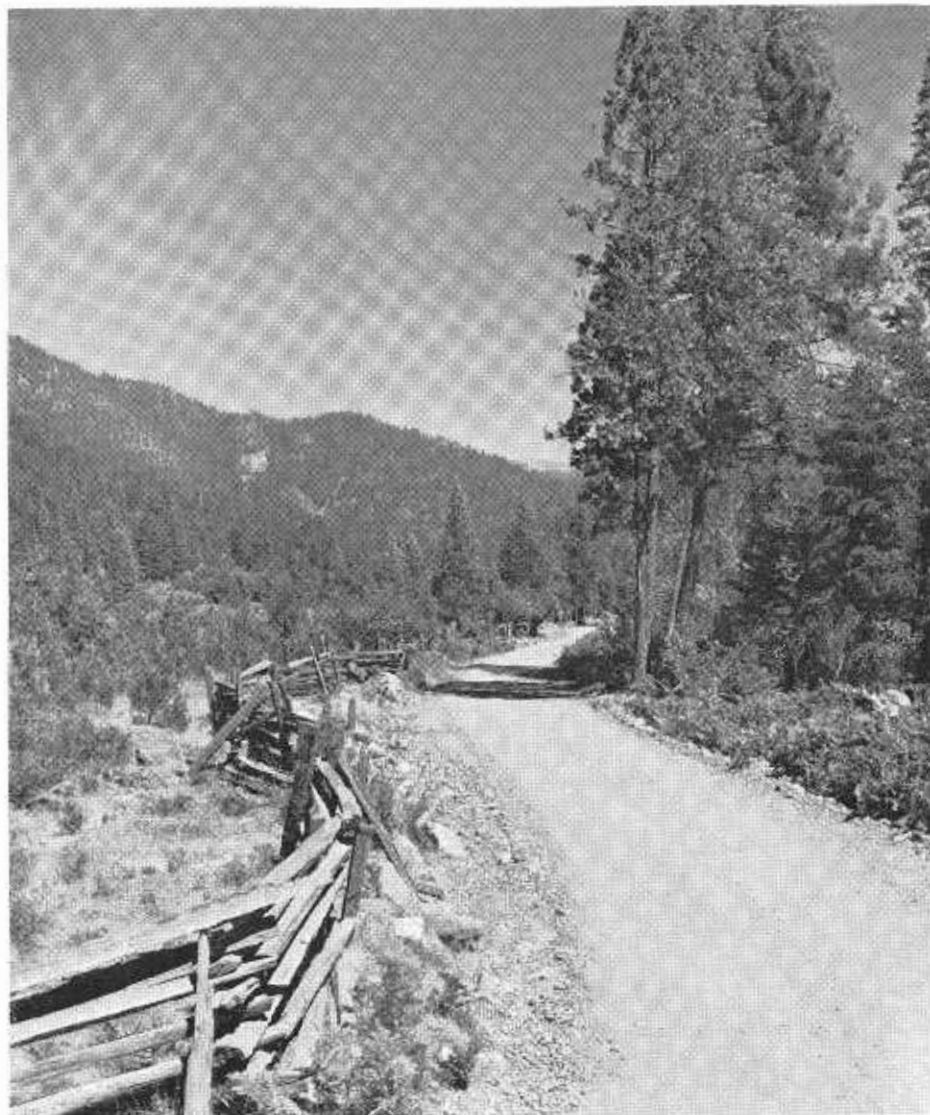
This view of FAS 1089 south of Carrville in Trinity County is typical of the unimproved sections of the road which are being replaced by modern two-lane highway.
