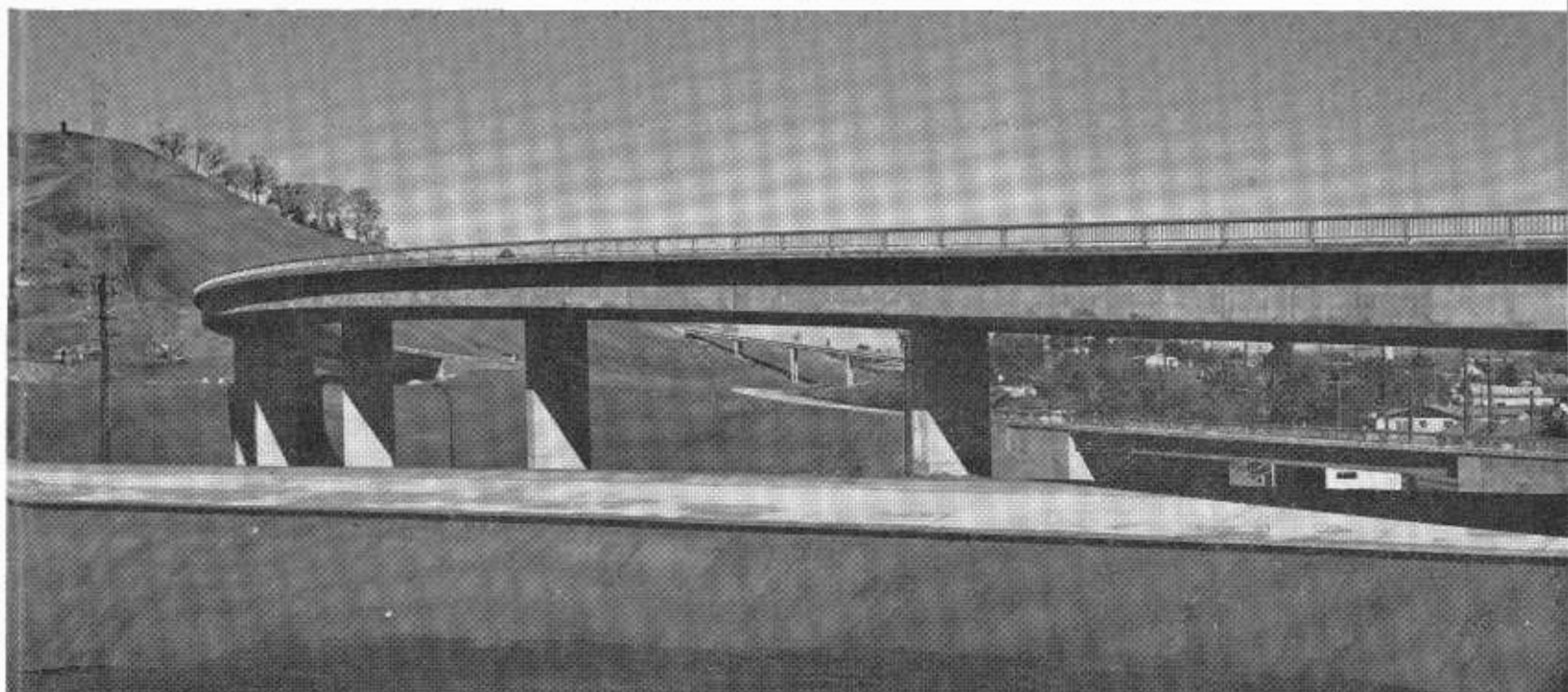
Photo below—Ground view of the Walnut Creek "Y" Interchange. Branch connection structure from SSR 24 to SSR 21 in immediate foreground.
