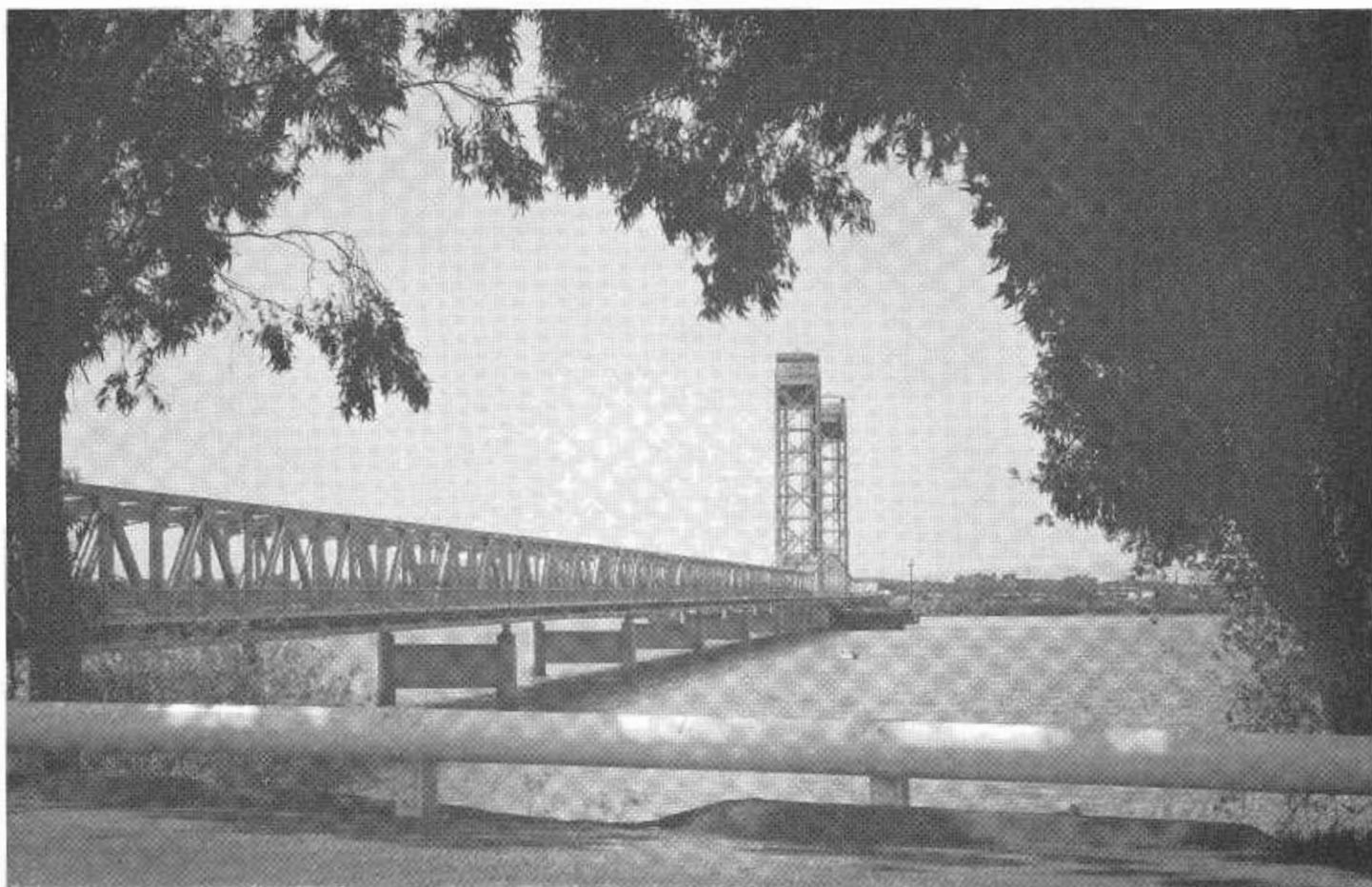
Looking west toward Rio Vista along the upstream side of the completed structure.
