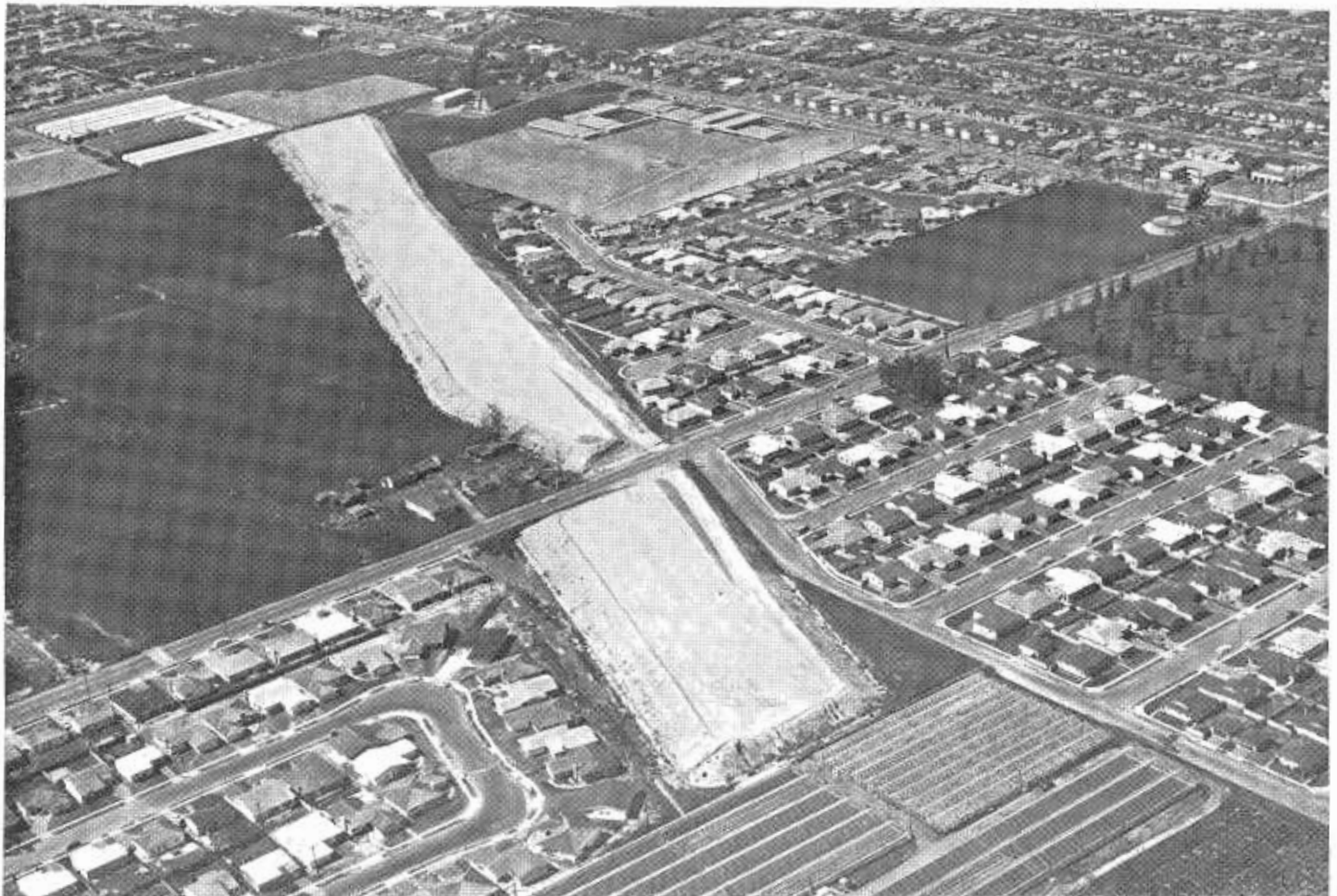
Compacted embankment for San Diego Freeway in City of Torrance placed by State's contractor from excess excavation on Harbor Freeway. This 226,000-cubic-yard fill is in addition to the 1,080,000-cubic-yard 1959 disposal program, as detailed in the accompanying article.
