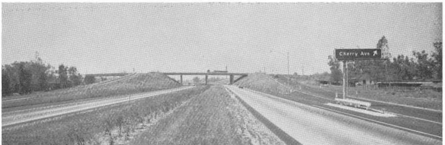
Cherry Avenue overcrossing is in the center of the picture; Cherry Avenue railroad overhead is to the left of it. These structures and approaches replace the former grade crossing at this location.
