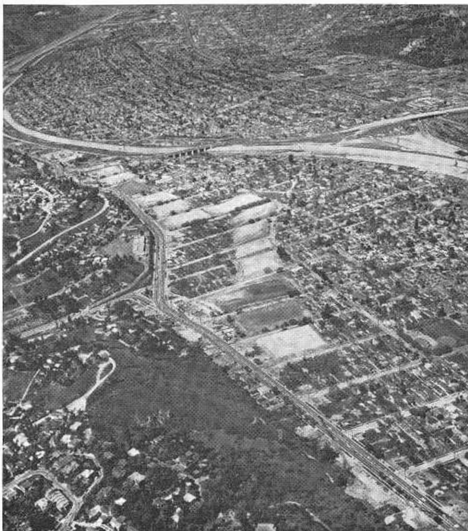
A view of the future Golden State Freeway alignment in the vicinity of the Glendale Freeway Interchange. In the foreground are 14 disposal sites with compacted embankments, a total of approximately 400,000 cubic yards of material. Los Angeles River in background.
