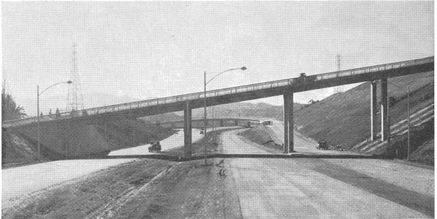
Oakvale Road Overcrossing on Sign Route 24, looking south. Slope stabilization through tie-down process, described in article, shows at extreme right.
