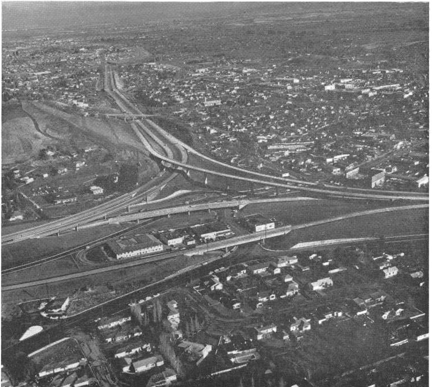
View of "Y" interchange in Walnut Creek. Looking northerly on Sign Route 24 to Oakvale Road Overcrossing with North Main Street interchange in background.
