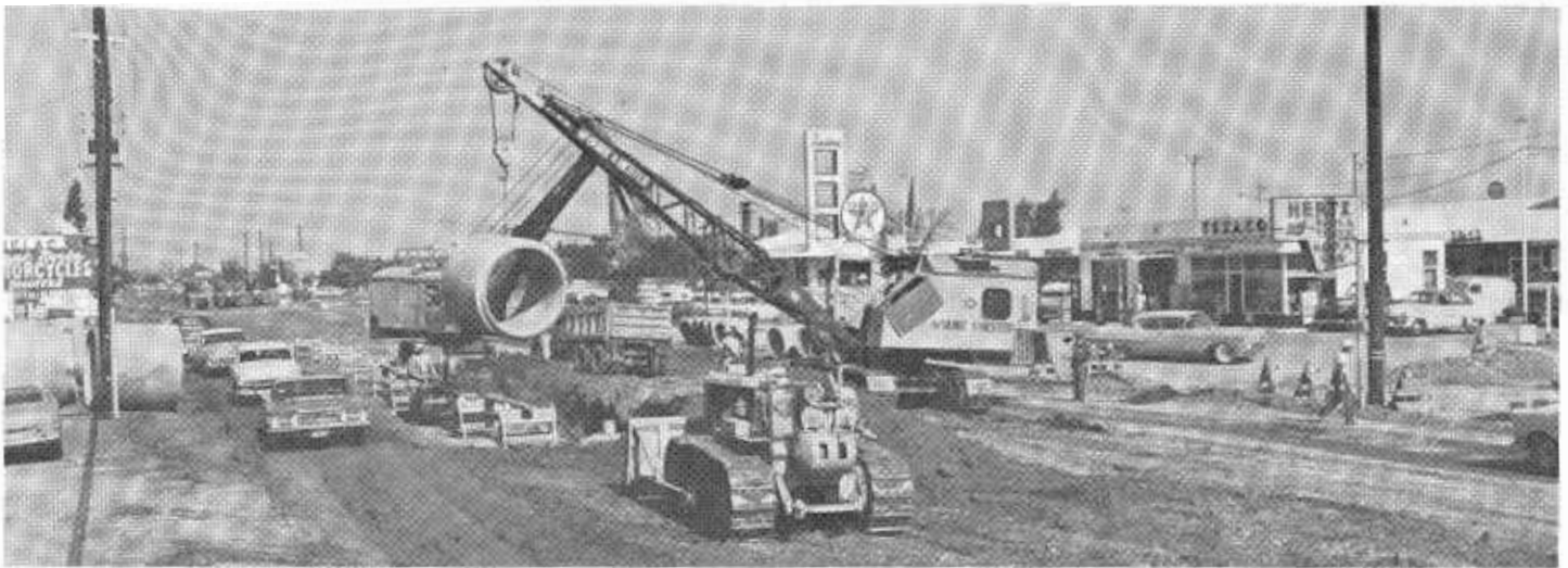
McHenry Avenue, October 1959, while construction operations were under way.
