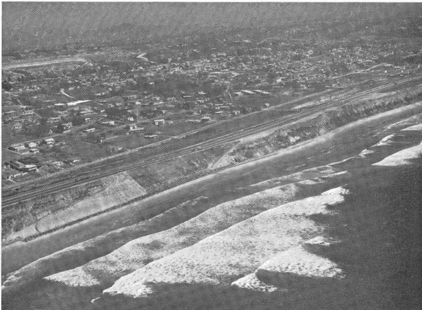
Looking southeasterly at US 101 showing limits of bank protection work. Dark area in center shows full rock riprap section at toe of completed embankment. Light area to north shows partial rock riprap section and stockpiled talus. The next contract which has been advertised will provide for removal of talus, completion of riprap section and placement of compacted embankment plus additional work to the north. Right center of photograph shows beach access road and parking area formed by excavation of necessary borrow material.
