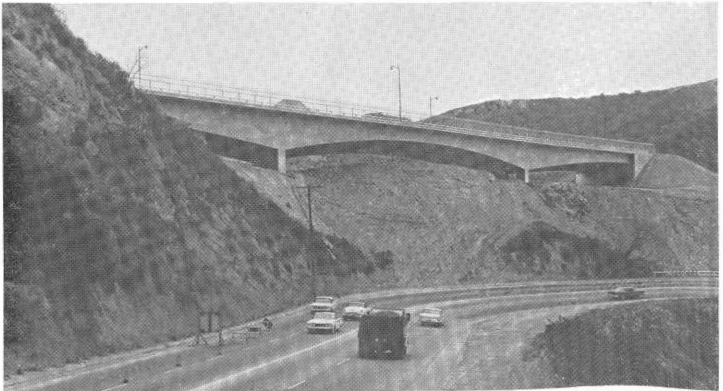
A view of the new Mulholland Drive Bridge spanning the future San Diego Freeway, taken from the old highway (Sepulveda Boulevard).
