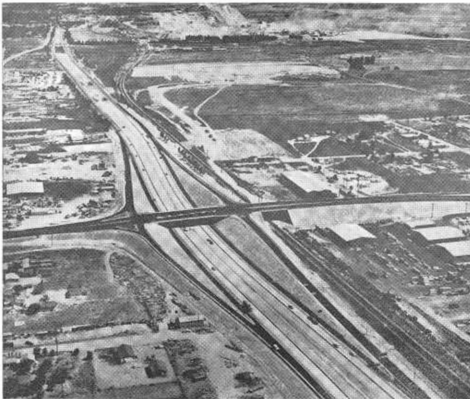
Recently completed Riverside Avenue interchange and freeway on US 70-99. Looking east.
