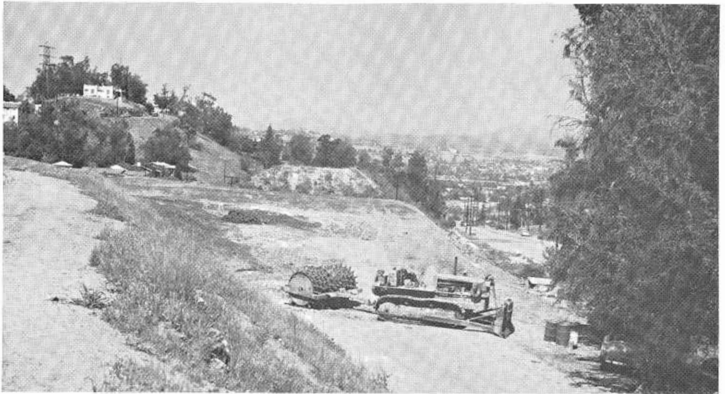
Looking north on the future Glendale Freeway with existing Alessandro Street at the right side of photo. District VII has under permit 100,000 cubic yards of freeway embankment in this vicinity.
