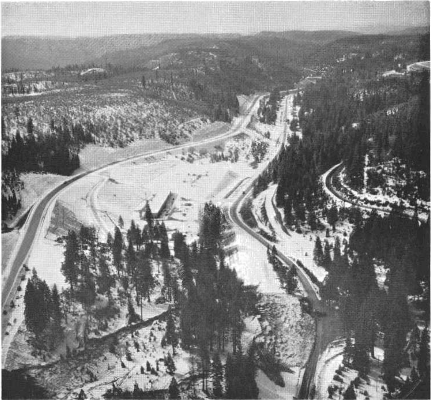
This slide (foreground) threatened to block U.S. Highway 40 near Baxter at a time when heavy traffic was expected for the 1960 Winter Olympics at Squaw Valley. Four lanes had been in operation on a temporary basis with the partly completed freeway carrying eastbound traffic (left) and the old highway handling westbound vehicles. The slide was successfully cleared from the old highway and a detour was constructed around the danger area on the east-bound lanes. The freeway has now been completed on this section.
