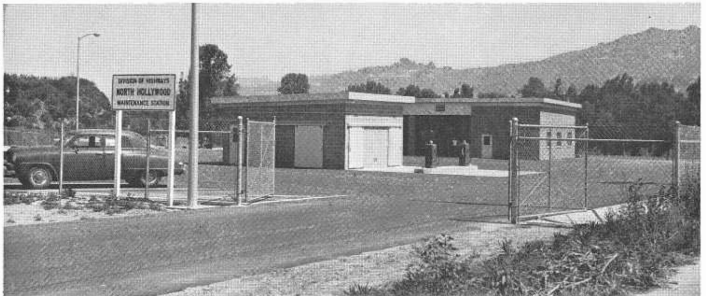
California's highways are kept in safe and serviceable condition by some 3,600 maintenance employees of the Division of Highways. Maintenance equipment is located at some 270 major road maintenance stations throughout the State, including this new North Hollywood station near the Ventura Freeway.
