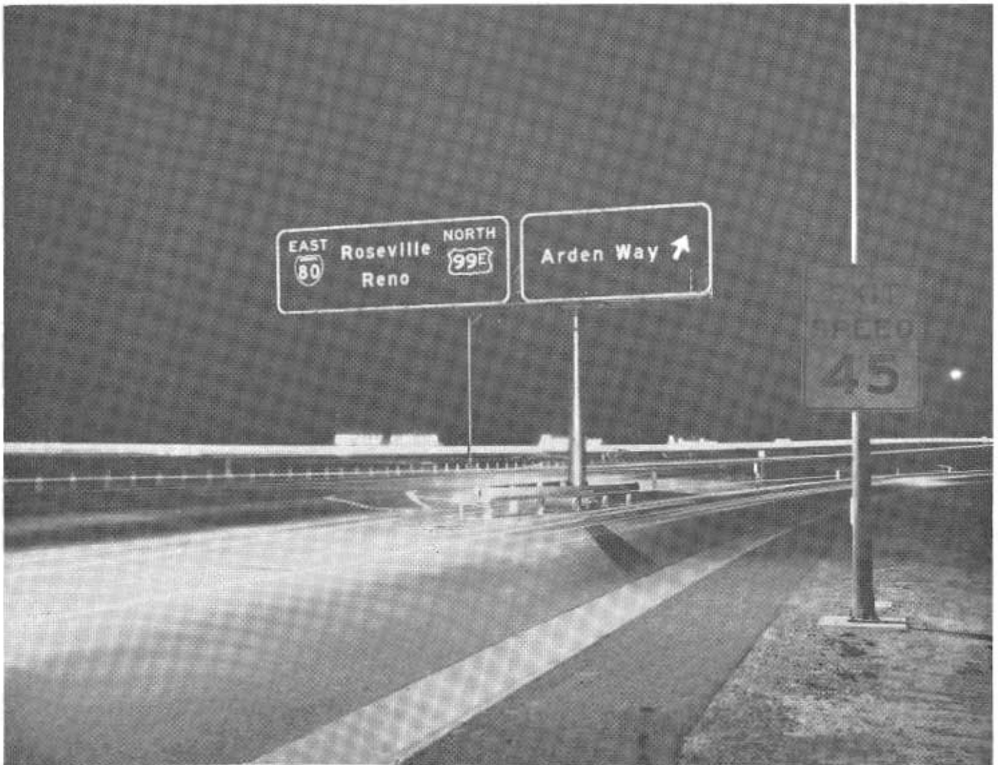
This experimental electro-luminescent overhead sign is being tested on U.S. Highway 99E just northeast of Sacramento. New equipment of this type is tried to determine its suitability for highway use under actual operating conditions.
