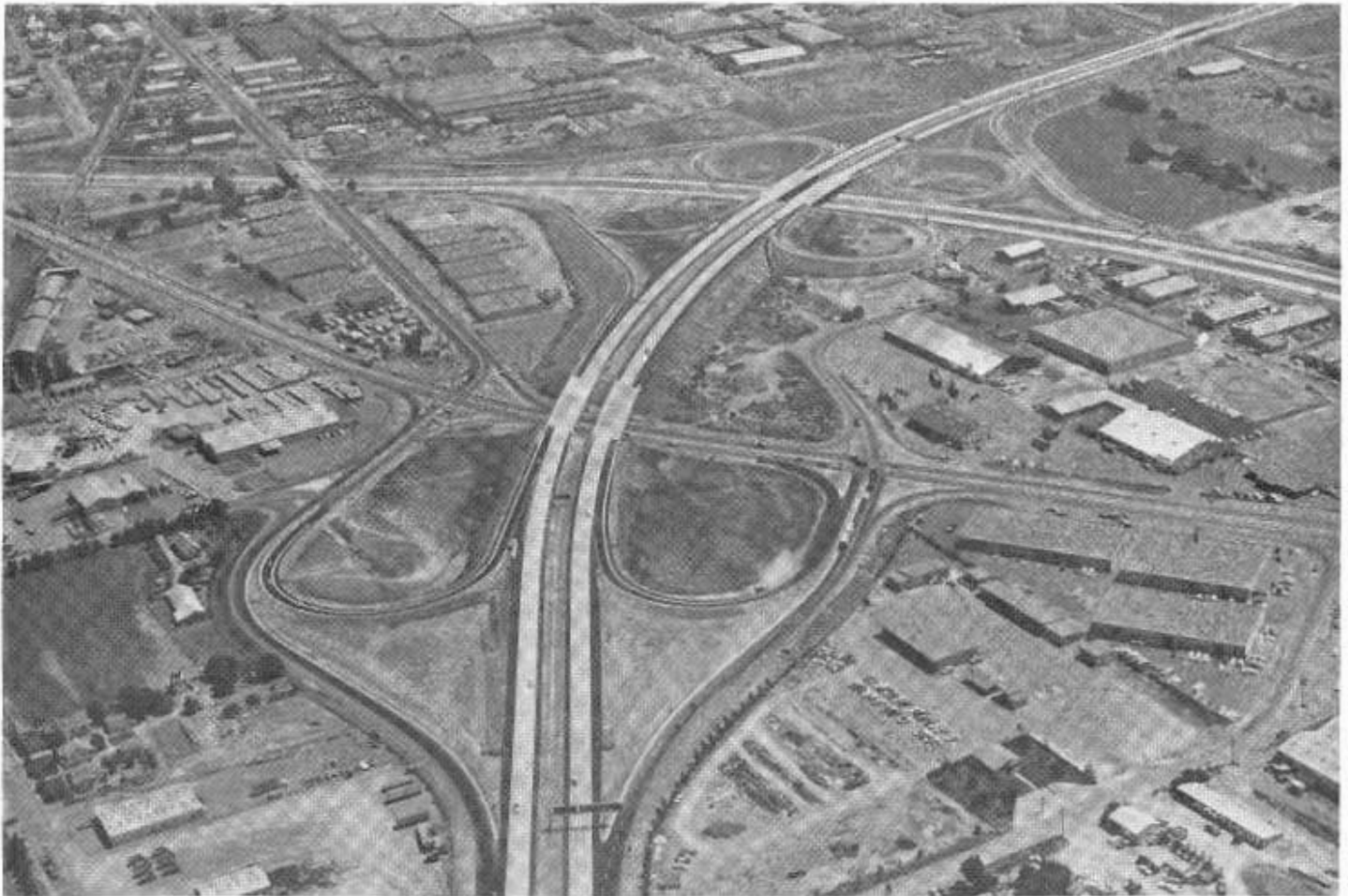
This new section of freeway eliminated the final gap in continuous freeway on Sign Route 17 through San Jose. Photo shows traffic separation structures which take the Nimitz Freeway over the former Bayshore Highway (center) and the new Bayshore Freeway lanes.
