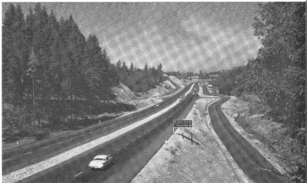
EXPRESSWAY (Above) —Four-lane divided highway with most full freeway features, but cross traffic may be permitted at some intersections as shown above.
