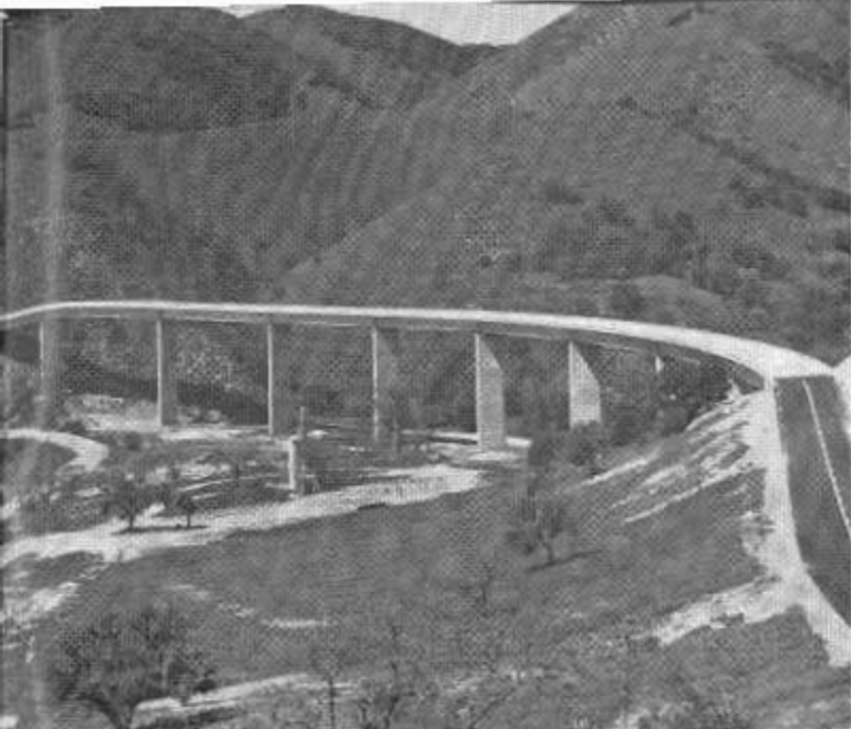
The Huasna River Bridge on Sign Route 166 some 10 miles northeast of Santa Maria received first prize in Class II which includes bridges with fixed spans costing more than $500,000.
