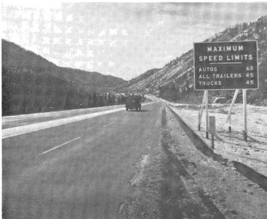
New speed limit signs were installed near state boundaries to inform motorists of maximum limits on California highways. This sign is on U.S. Highway 40 near the Nevada border.
