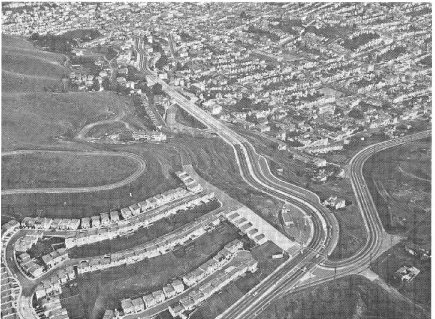
The \frac{3}{8} -cent gas tax funds were used to finance a large scale improvement on Market Street (above) in southwest San Francisco. The major city street project involved realignment, widening and construction of bridges.
