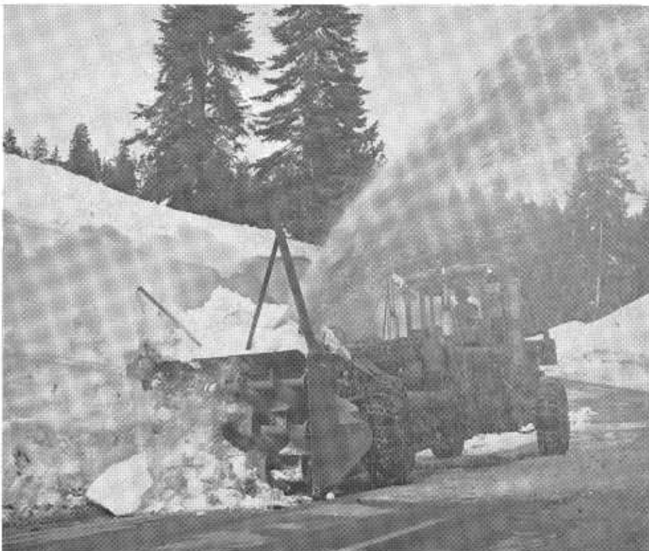
Rotary snowplows go into action each winter to clear California's mountain pass highways. The Division of Highways operates three new-type heavy-duty rotaries mounted on motor graders (above) and 53 truck-mounted rotary plows.
