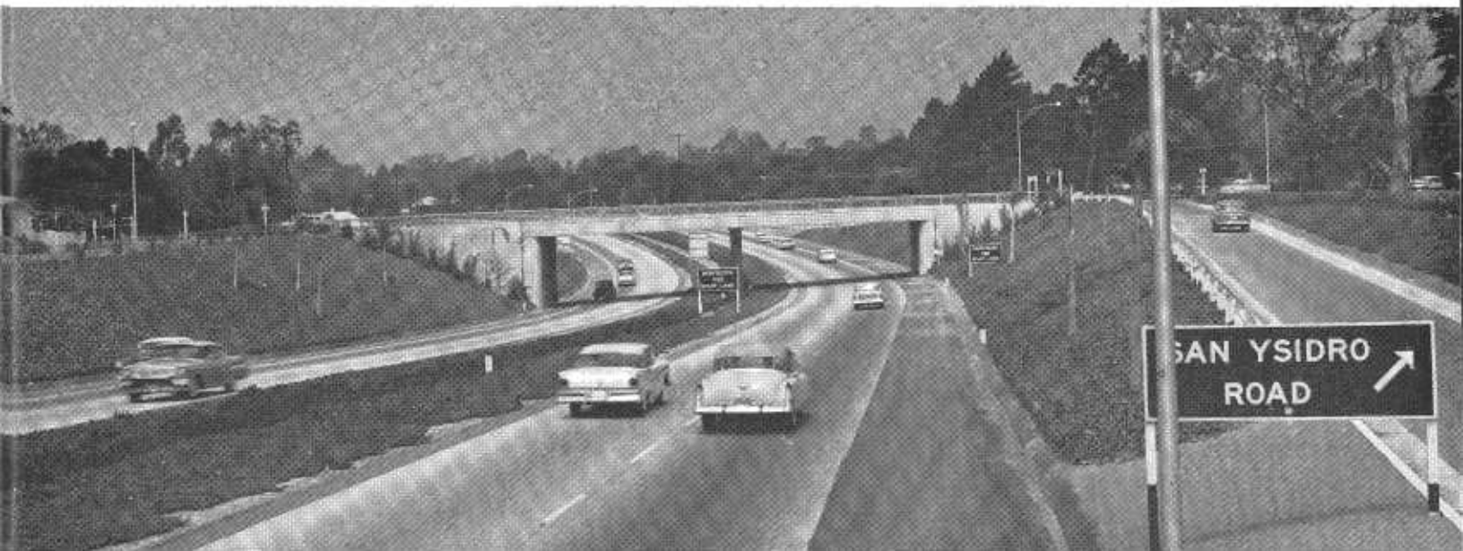
FULL FREEWAY (Below) —Crossing structures, interchanges, and complete access control eliminate traditional traffic conflicts and make full freeways safer and more efficient than any other type of highway.
