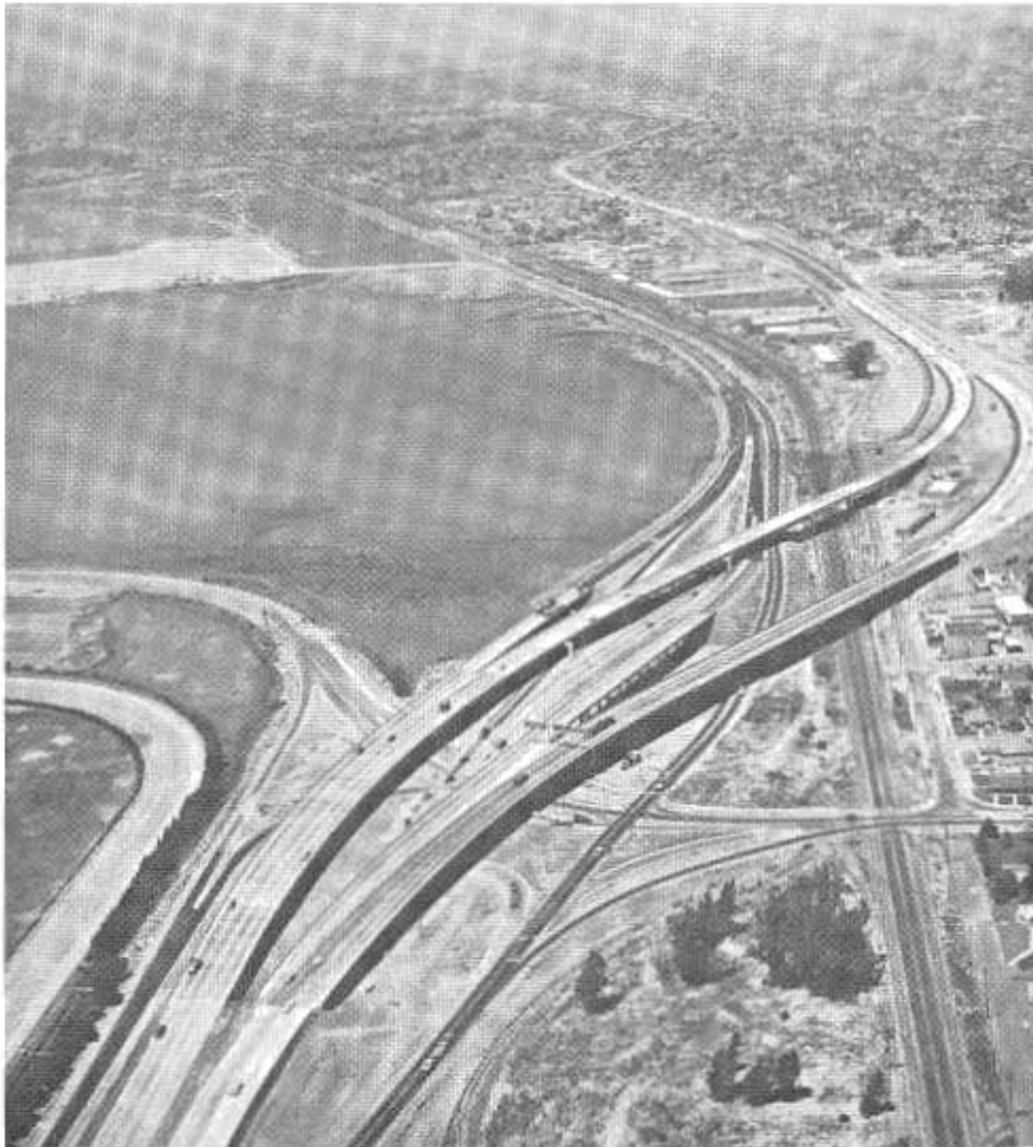
Recently completed six-lane freeway on U.S. Highway 40 in Richmond which eliminated final gap in continuous full freeway between Los Gatos and Vallejo.
