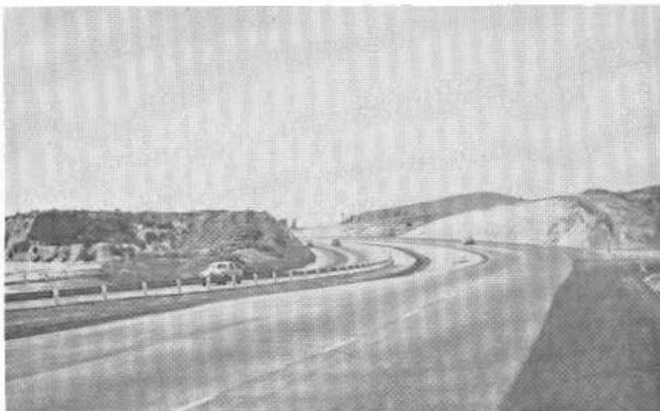
This four-lane expressway on Van Buren Boulevard, a Riverside County Road near Redding, was completed in 1960 under the Federal Aid Secondary County Road Program.
