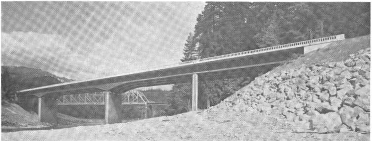
This structure across the South Fork of the Eel River on US 101 (Redwood Highway) in Humboldt County was among bridges judged most beautiful in national competition sponsored by the American Institute of Steel Construction.
