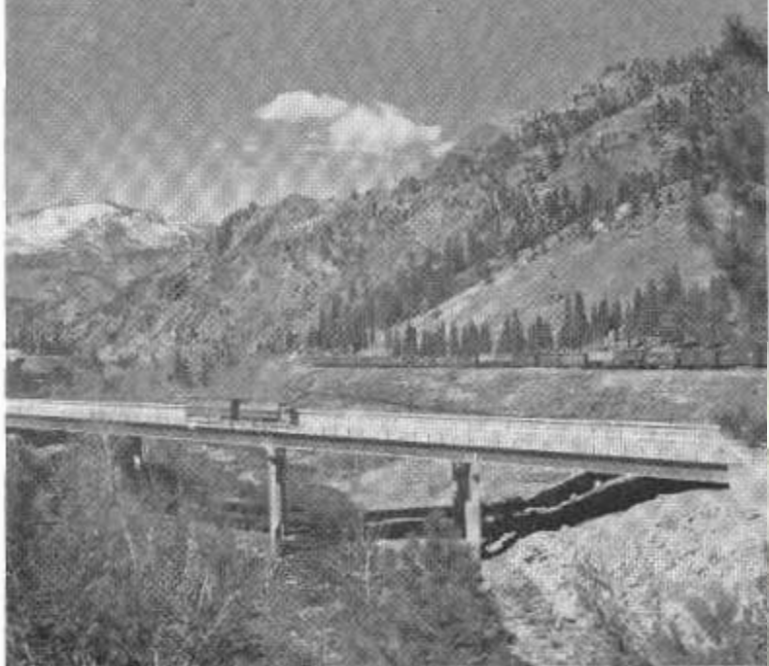
The Truckee River Bridge on US 40 13 miles northeast of Truckee received an honorable mention award in Class III which includes bridges with fixed spans costing less than $500,000.
