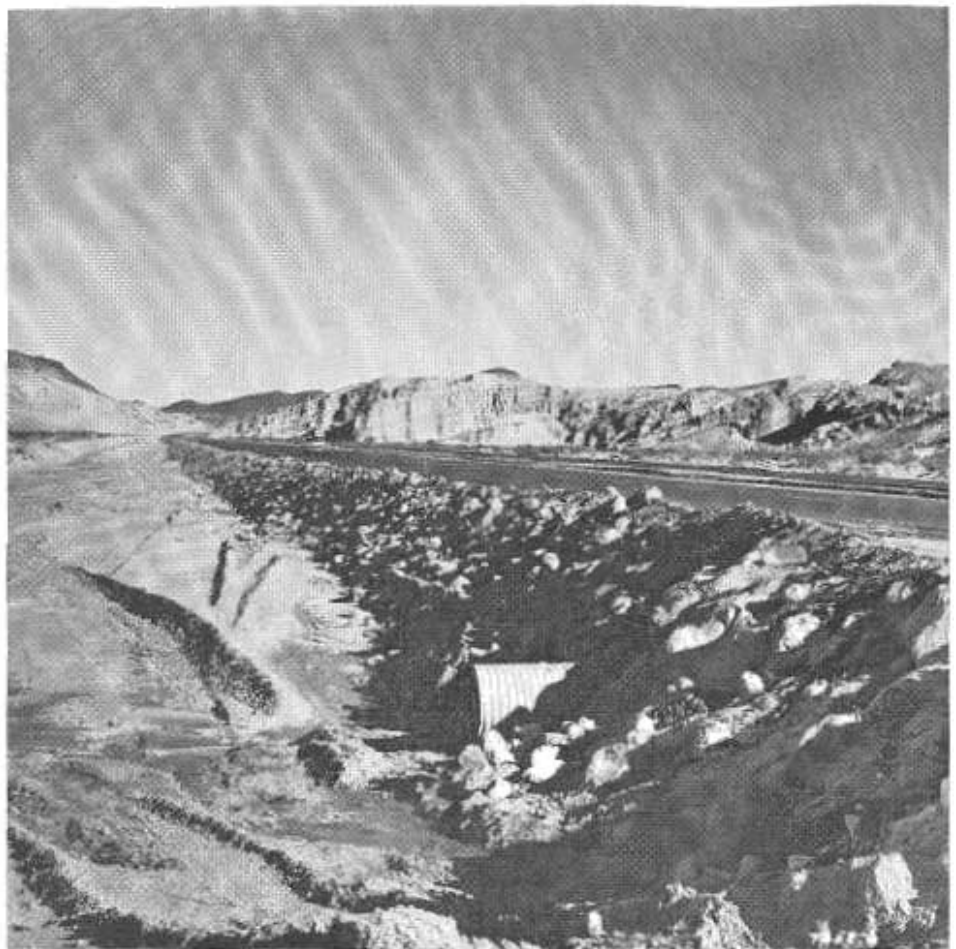
Recently realigned four-lane section climbing out of the main wash of Red Rock Canyon on U.S. Highway 6 about 25 miles north of Mojave, Kern County.
