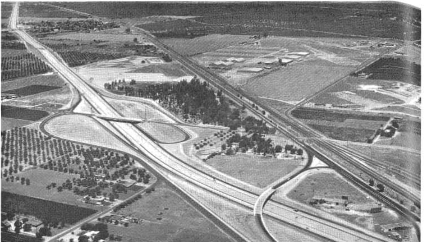
The last section of three-lane highway on US 99 was eliminated in 1960 when this new four-lane freeway was opened north of Fresno. Note old highway parallel to railroad at right.
