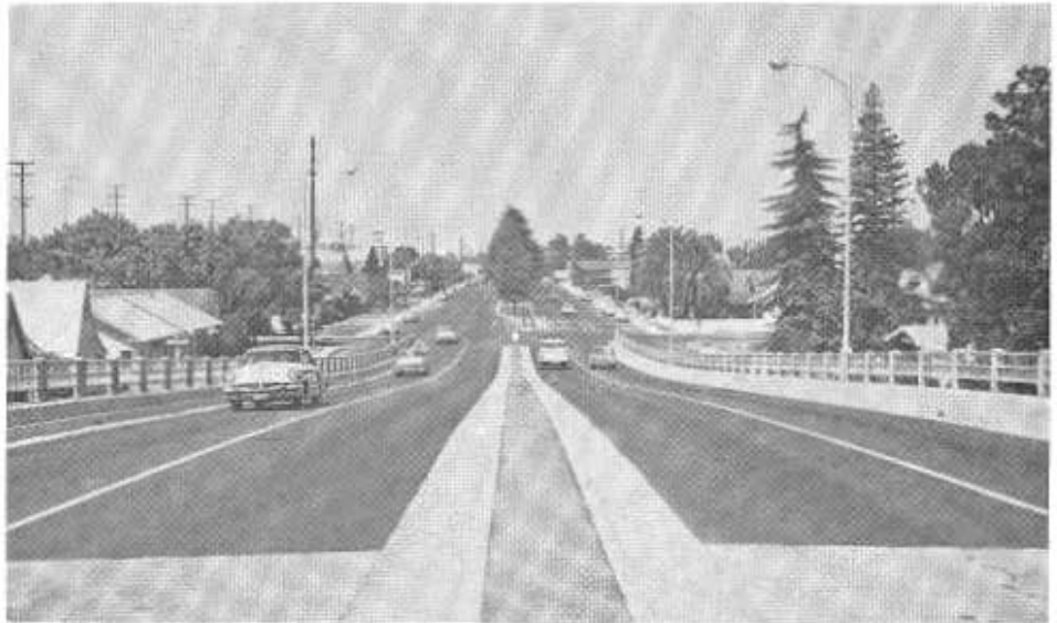
Truxtun Avenue in Bakersfield was completed as a six-lane major city street in May, 1960, at a cost of $156,000 in 5-cent gas tax funds.
