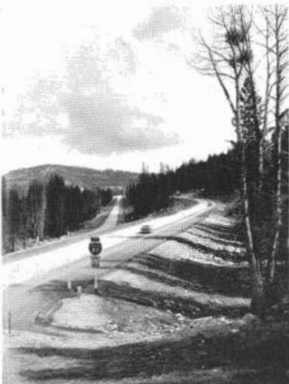
FRONT COVER —Looking east toward Donner Summit on US 40 (Interstate 80) showing a recently completed section of freeway between Hampshire Rocks and Soda Springs. Note the two roadways at different levels, with a stand of trees in the median. Elevation at this location is about 6,000 feet.
