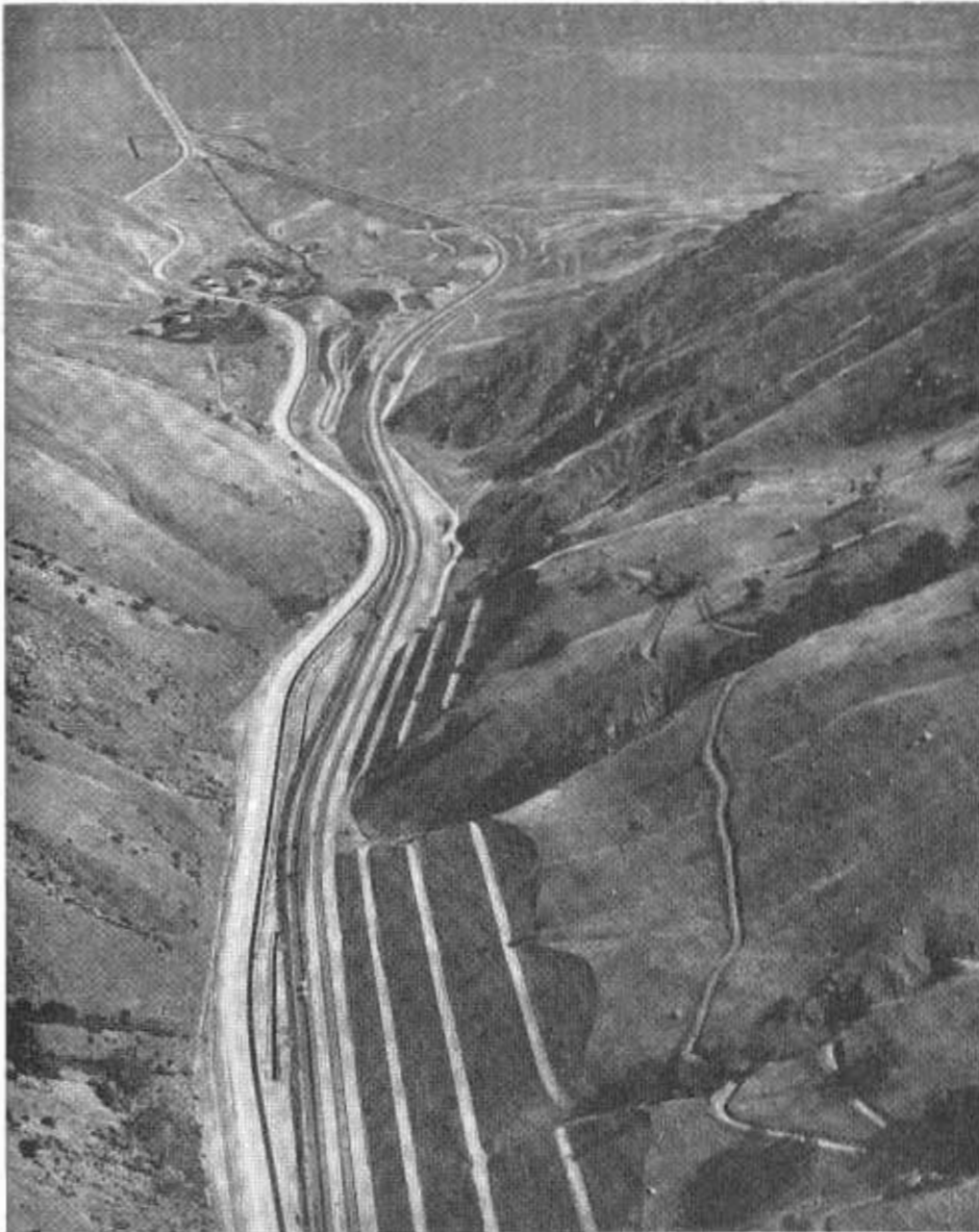
This new section of eight-lane freeway over the Grapevine Grade on US 99 in Kern County was opened June 28, 1960. The photograph shows a northerly view through the canyon toward the San Joaquin Valley.
