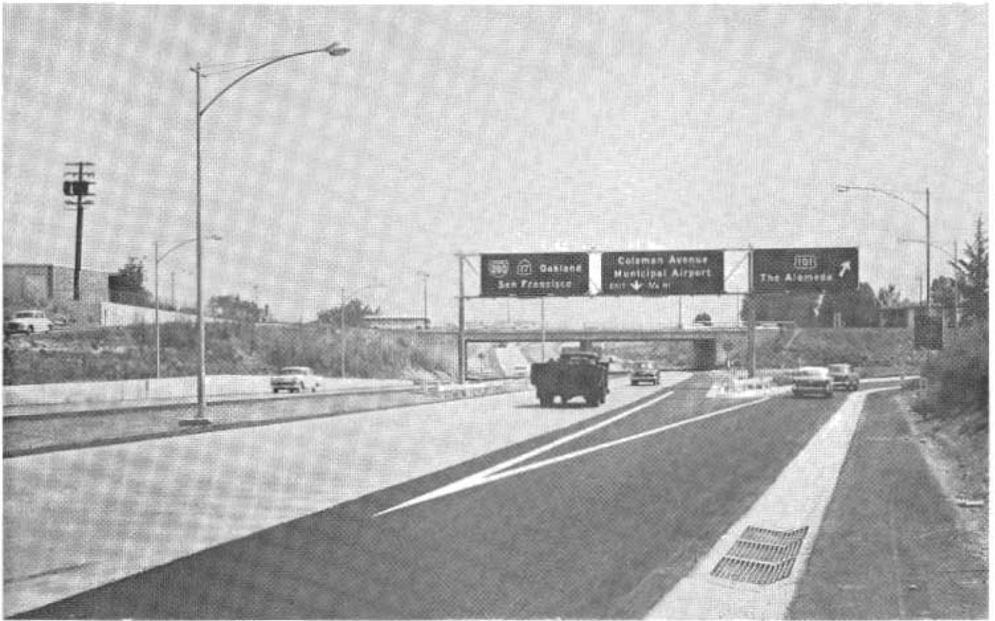
This large overhead sign is typical of those now in use on new freeways throughout the State. Note the "up arrow" to direct movements off the freeway.
