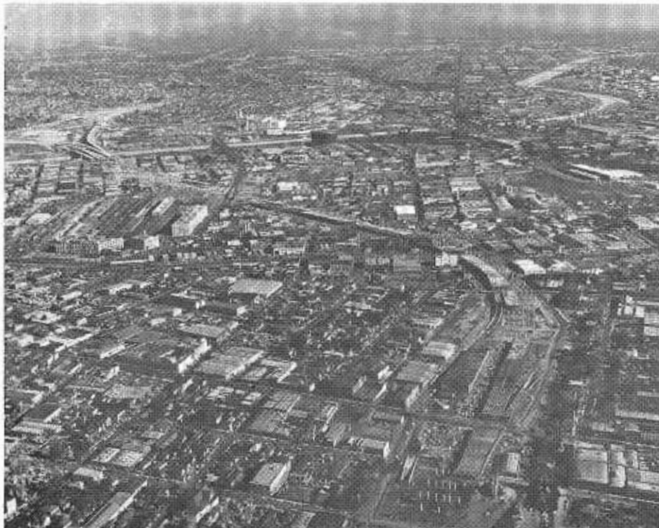
Looking east along the Santa Monica Freeway viaduct construction connecting the Harbor Freeway and the East Los Angeles interchange (upper left) at the Santa Ana Freeway. Structure (top left) is the bridge across the Los Angeles River.
