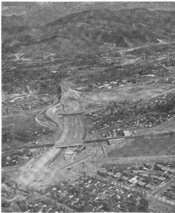
Golden State Freeway construction at Lankershim Boulevard (bridge in foreground).
