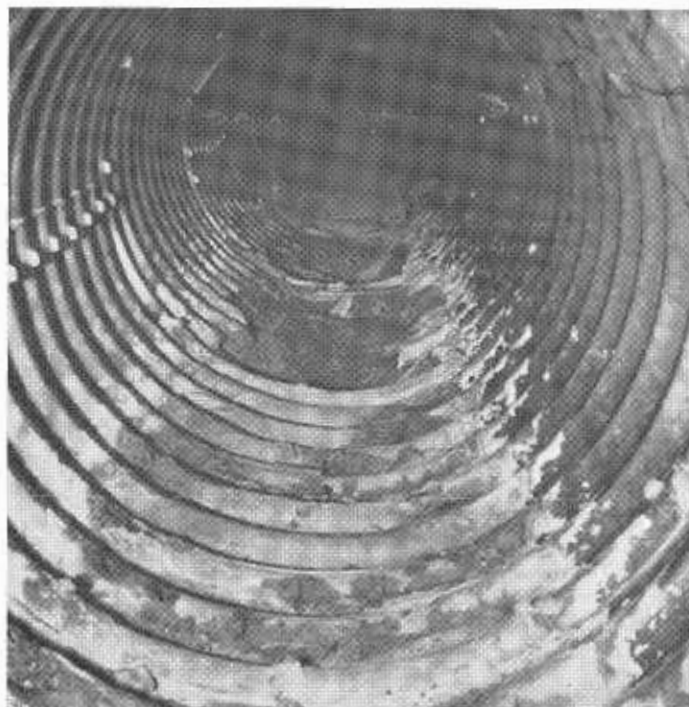
FIGURE 1. Two corrugated metal pipe culverts, each 30 years old but in different locations. The pipe at the left was subject to corrosive flow which has removed the invert. The pipe at the right was installed in an area which is relatively non-corrosive.
