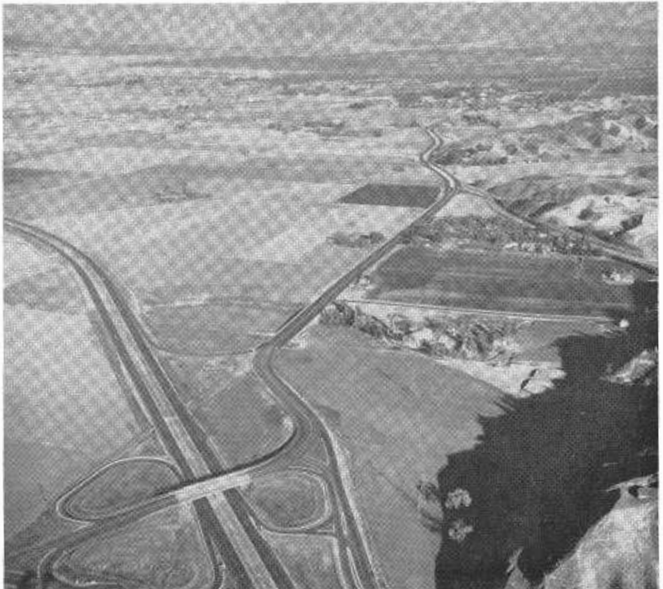
The Washington Street-Barton Road project constructed by San Bernardino County under the F.A.S. Highway Program. The view is northeastward with the Riverside Freeway interchange in the foreground.
