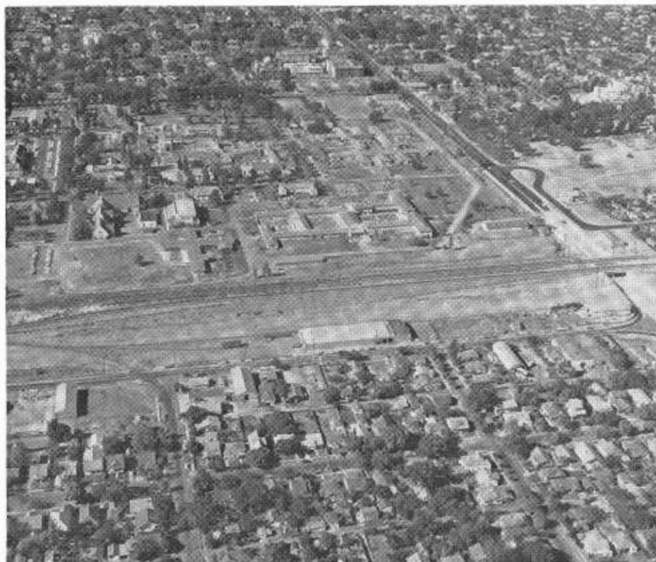
An aerial of the completed Harding Way Underpass (right center). At the center of the photo is the Stockton State Hospital.
