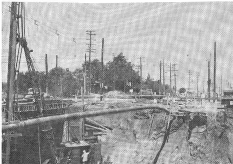
A view of the pile driver in operation between the suspended telephone cables and the west half of the new bridge.
