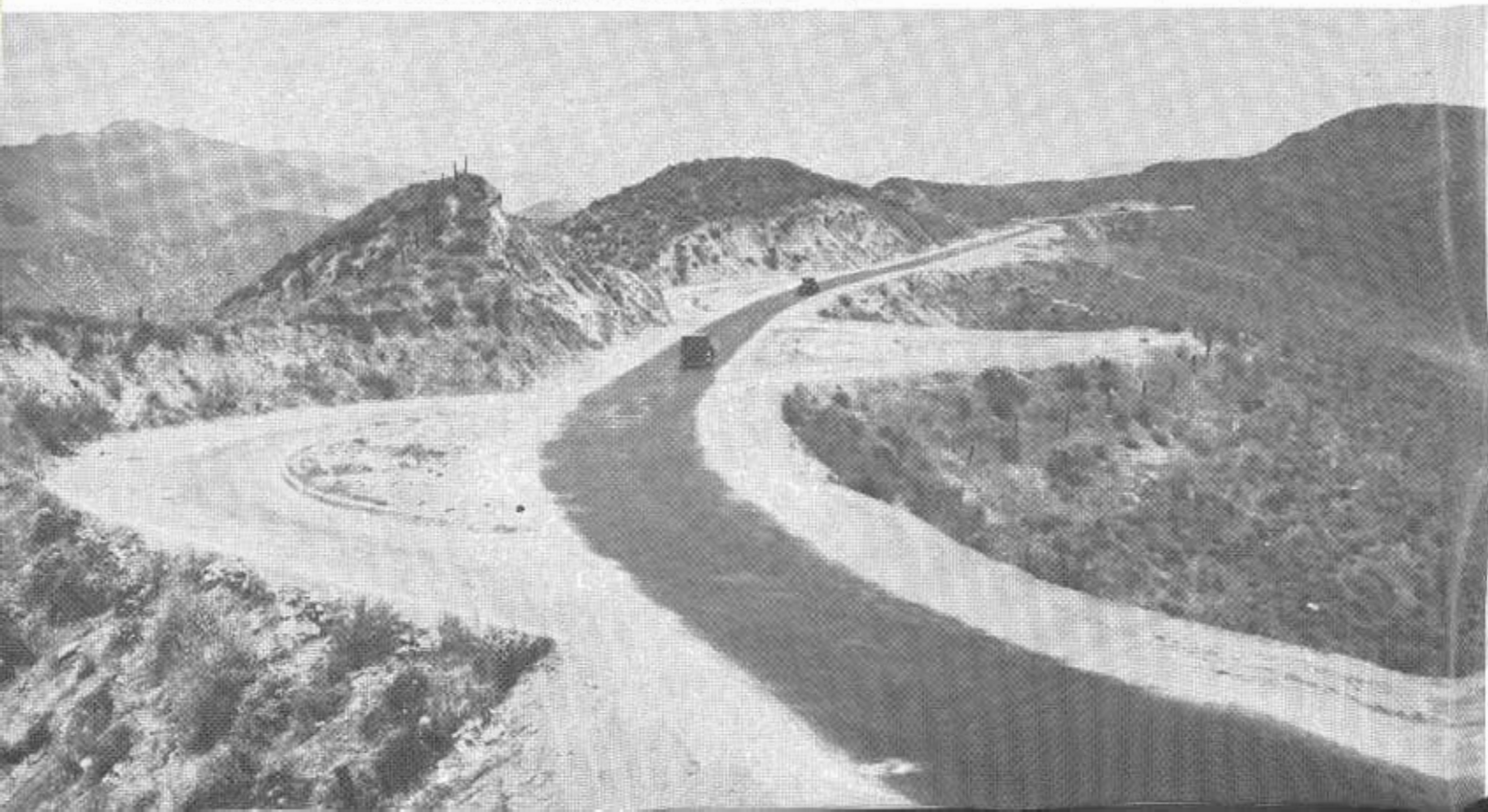
Below: With improved design and increased speed of the motor car, the old short radius curves and contour-following roads developed high accident records, and had to be realigned. This is a section of the Ridge Route on US 99 which was realigned in late 1920's. The old reversing-curve alignment shows clearly.
