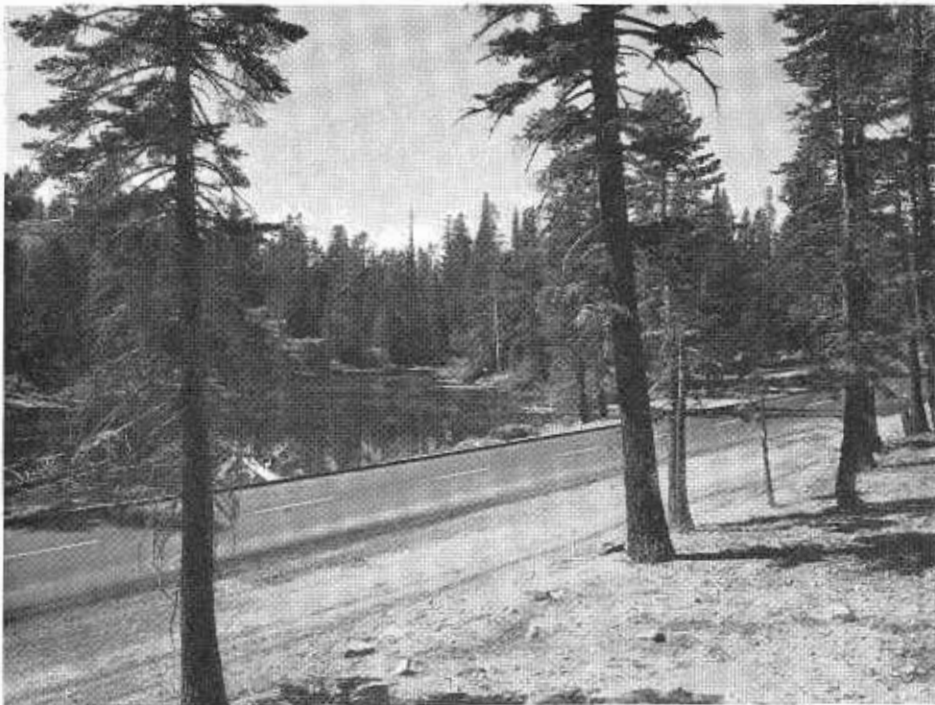
A section of the new reconstructed highway in the vicinity of Carson Spur. Mosquito Lake is on the far side of the road.
