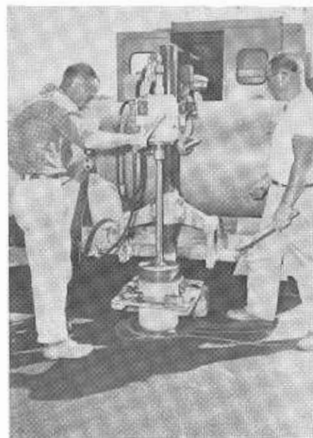
Apparatus used for obtaining cores of completed pavement and bases to measure thickness and test the quality of materials.
