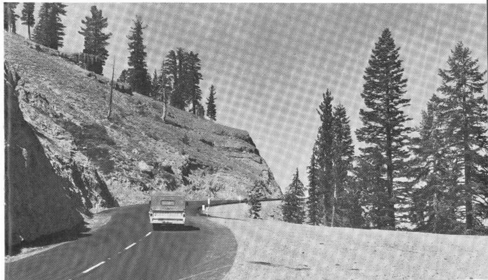
A view of Carson Spur, looking westward, following completion of the widening project.
