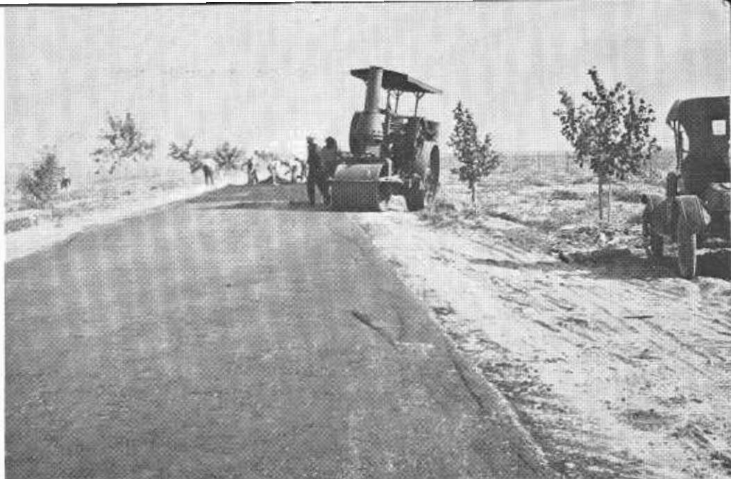
A resurfacing job going forward on another stretch of US 99, near Wheeler Ridge south of Bakersfield, about 1922. Note young roadside trees, planted about 1920. Due to lack of experience of planters, many trees planted in those days were not adapted to climate and soils.
