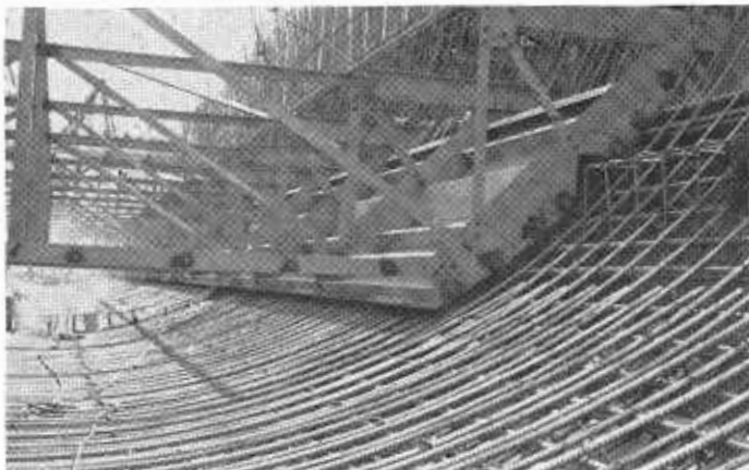
A view of the tube reinforcement and the interior invert form.
