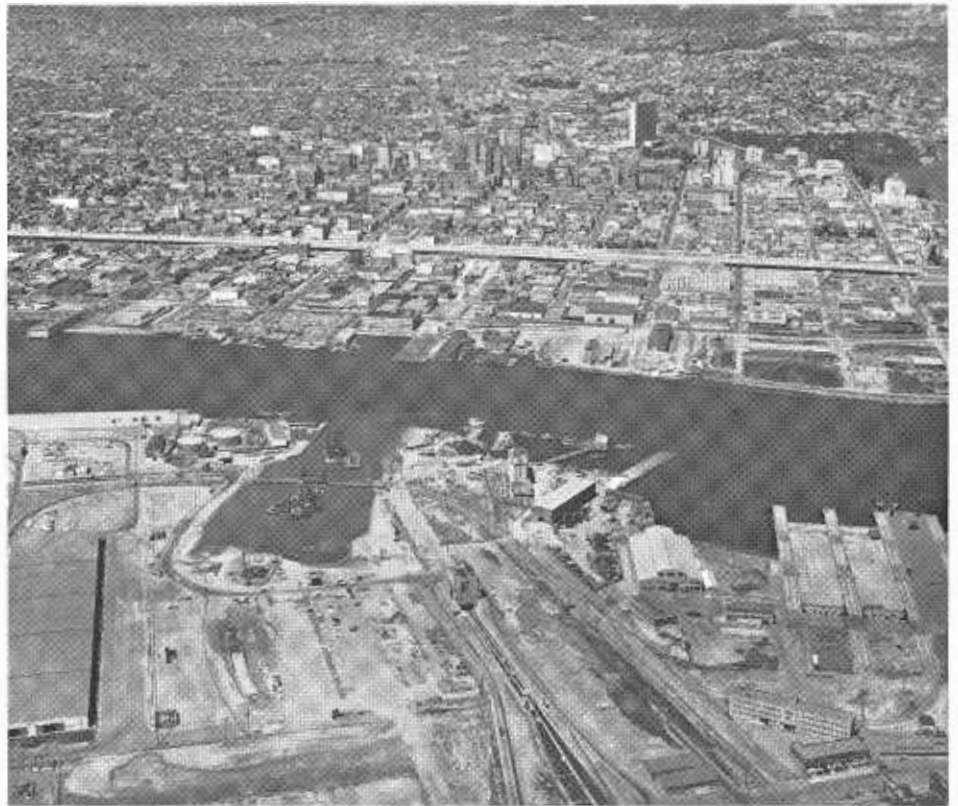
General location of the tube and the project. Note temporary lift bridge on the railroad shoofly. The soft mud is quite unstable and an excavation 450 feet wide is required to provide a stable underwater trench 60 feet deep and 40 feet wide at the bottom.
