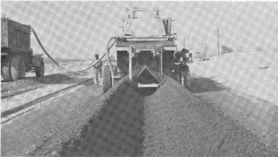
A rear view of the custom-built, cement-treated base mixer shown above.
