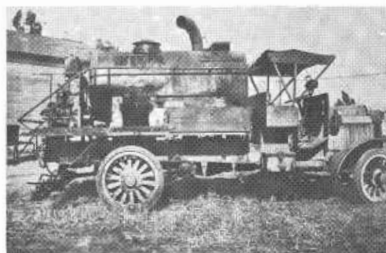
Two early types of road oilers. Horse drawn vehicle (below) used about 1913 was gravity flow, would only work in warm weather. Motorized model (above) had heater and pump. Both required a driver and an operator who rode seat in rear.
