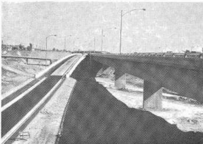
Completed interchange roadways at the East Los Angeles interchange.
