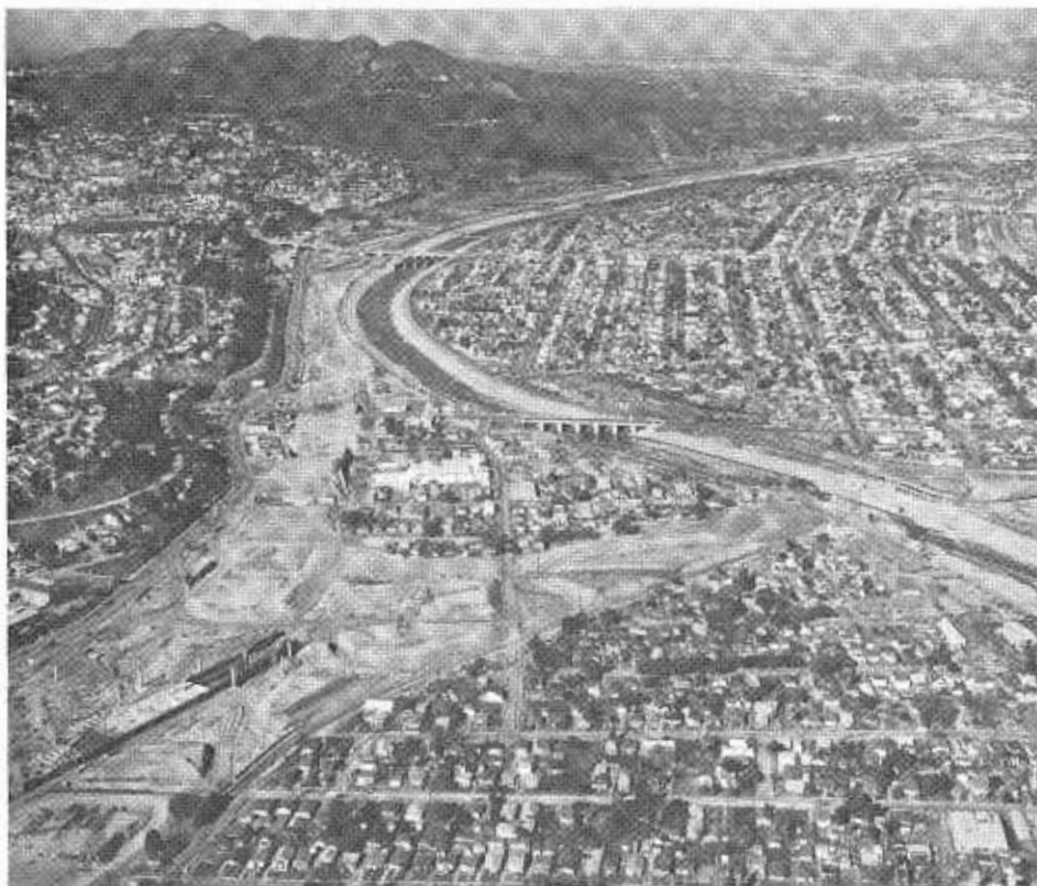
The Golden State Freeway-Glendale Freeway interchange. The Glendale Freeway will enter from the right across the Los Angeles River.
