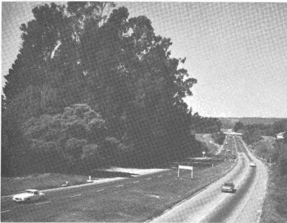
Modern freeway section of State Sign Route 1 south of Santa Cruz. Simple roadside planting treatment here functions well for slope control, also blends roadside attractively into surrounding terrain.
