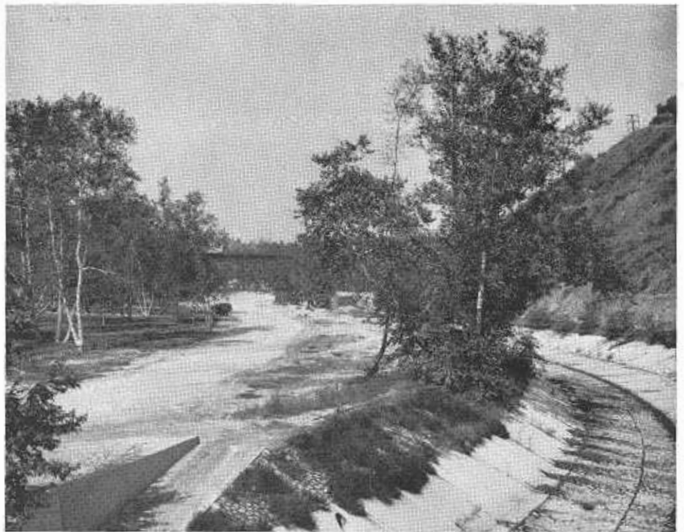
BEFORE. In January, 1940, the Arroyo Seco looking north from Avenue 60 looked like this. The Santa Fe Railroad viaduct is in the background.
