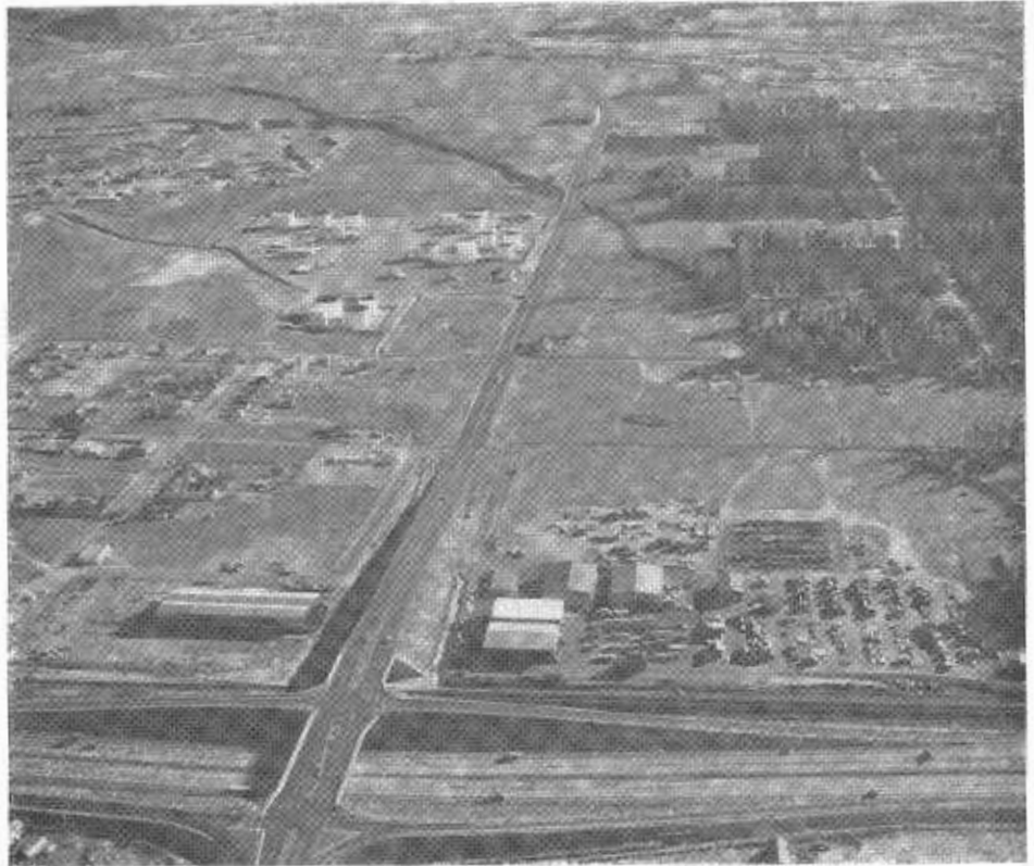
The Riverside Avenue F.A.S. project looking from above the San Bernardino Freeway south toward Riverside.
