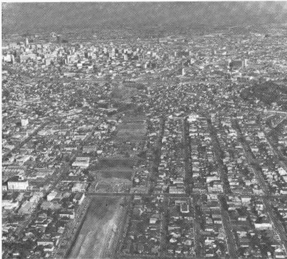
Looking east along the cleared route of the Santa Monica Freeway from Vermont Avenue. The bridge structure (top center) crosses the Harbor Freeway.
