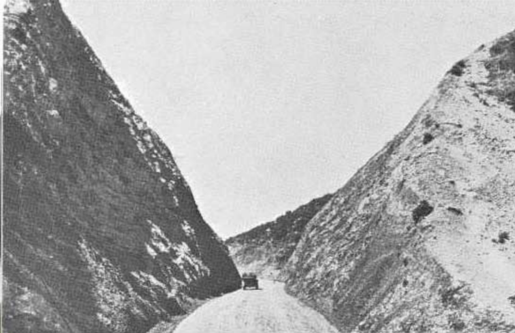
In early days of road expansion, cuts were made steep to save money, but savings were lost when slides became serious problem in wet season. Above is ridge route about 1915.
