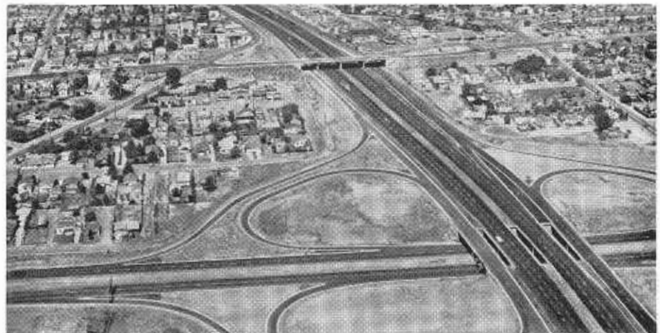
AFTER—An aerial of the State Route 74 Separation (foreground) and Benicia Road Overcrossing (background) following construction of the freeway.
