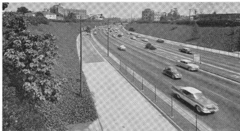
Hollywood Freeway in Los Angeles area. Algerian ivy has proved one of the best vines for this type of slope planting, if sprinkling is provided. Screen at top is Japanese privet. Trees are catalpa and liquidambar, both of which will become much more significant in the overall design as they grow larger.
