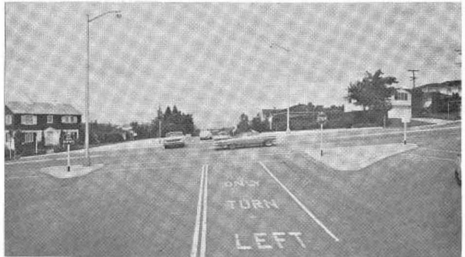
Channelization of the intersection of Parrott Drive and Alameda De Las Pulgas in San Mateo was designed with provision for future traffic signals when needed.
