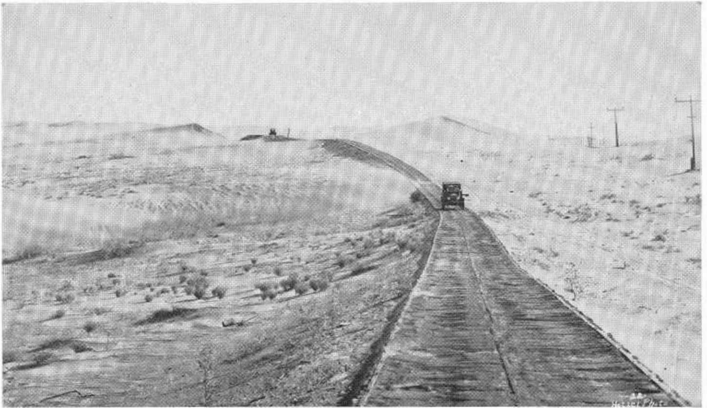
A section of the improved plank road constructed by the California Highway Commission across the Sand Hills in 1916.
