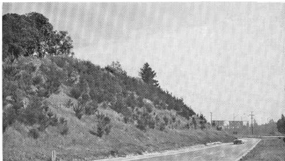
Hillside in the Santa Cruz area planted with native Monterey pines. These fast-growing native trees are ideal for this climate and will quickly bind the slope.
