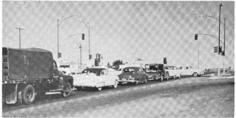
BEFORE—This is a scene from the U.S. 40-Benicia Road intersection in Vallejo prior to construction of the freeway.
