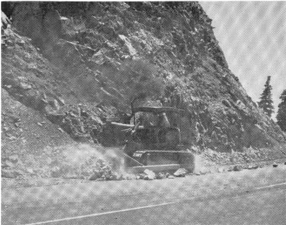
Slide Removal Operations. A bulldozer gathers the loose rock into piles.
