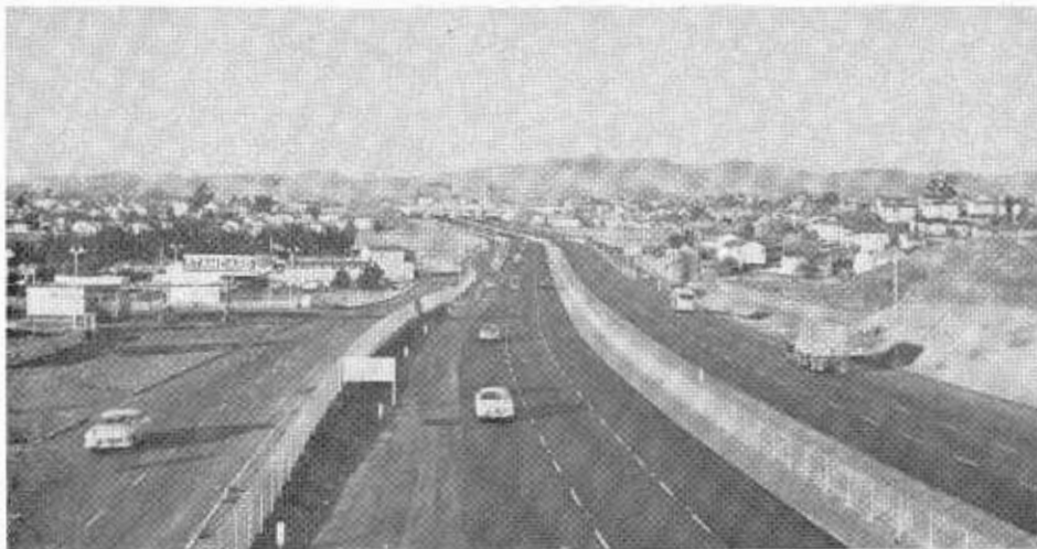
AFTER—A view of the same section of U.S. 40 following completion of the freeway.
