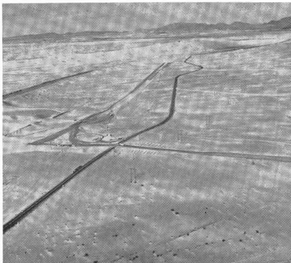
An aerial view of the haul road for construction equipment crossing the present highway.
