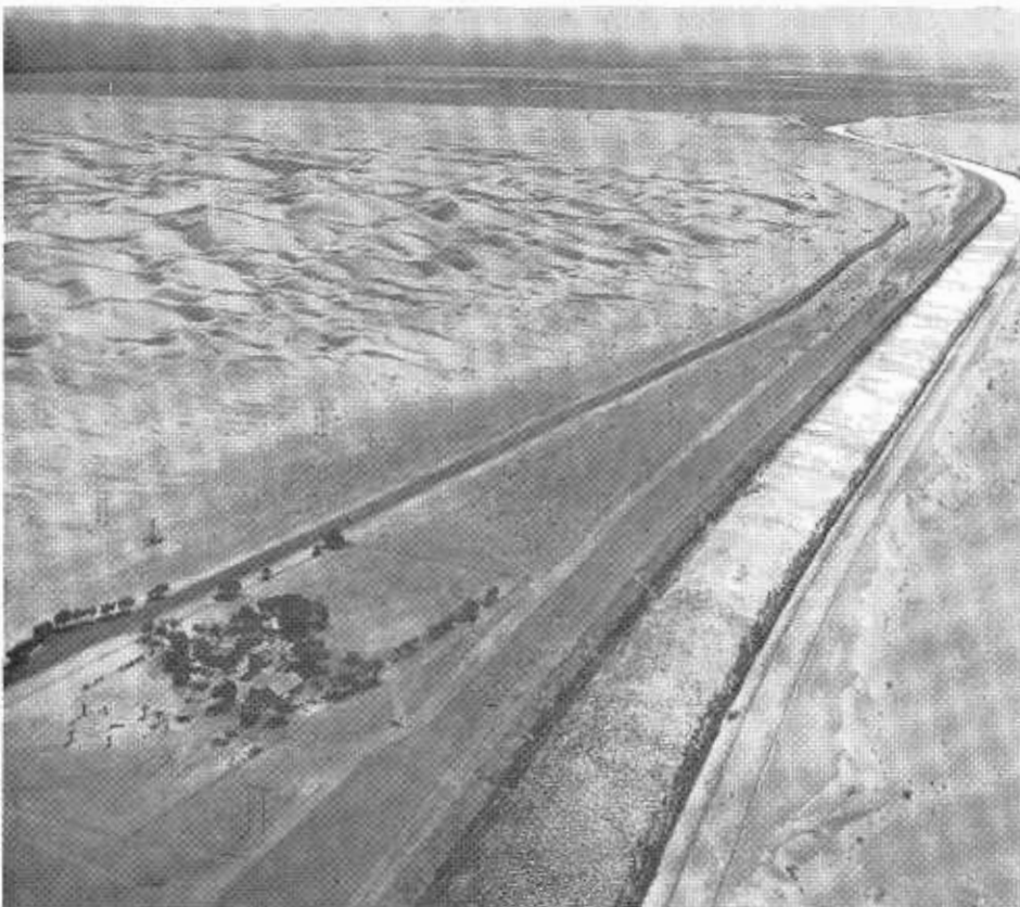
An aerial view of the All American Canal maintenance station and yard on the present highway which will be removed for construction of the new freeway.
