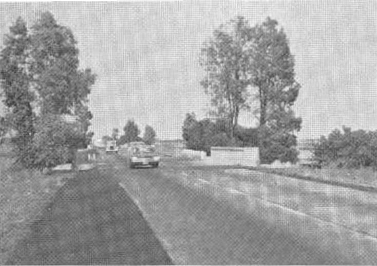
Eucalyptus and California Toyon used for delineation of series of short bridges on US 40 just south of Davis.
