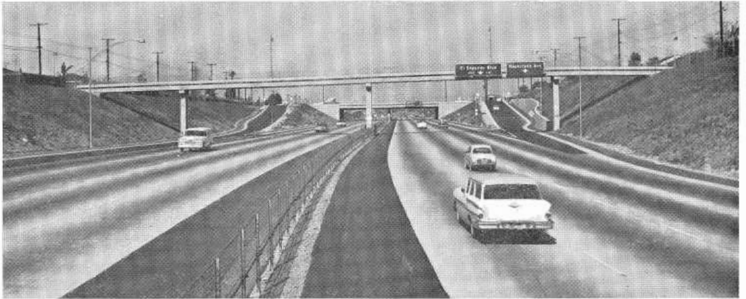
Looking northerly along recently completed portion of Harbor Freeway from 146th Street pedestrian overcrossing.
