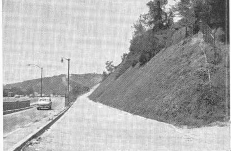
Example of Type A slope control in Cahuenga Pass section of Hollywood Freeway.
