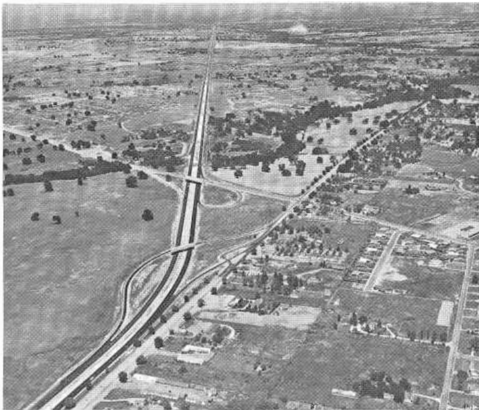
Looking east toward Roseville along the section of freeway covered by the study. The old highway is between the lines of trees to the right.
