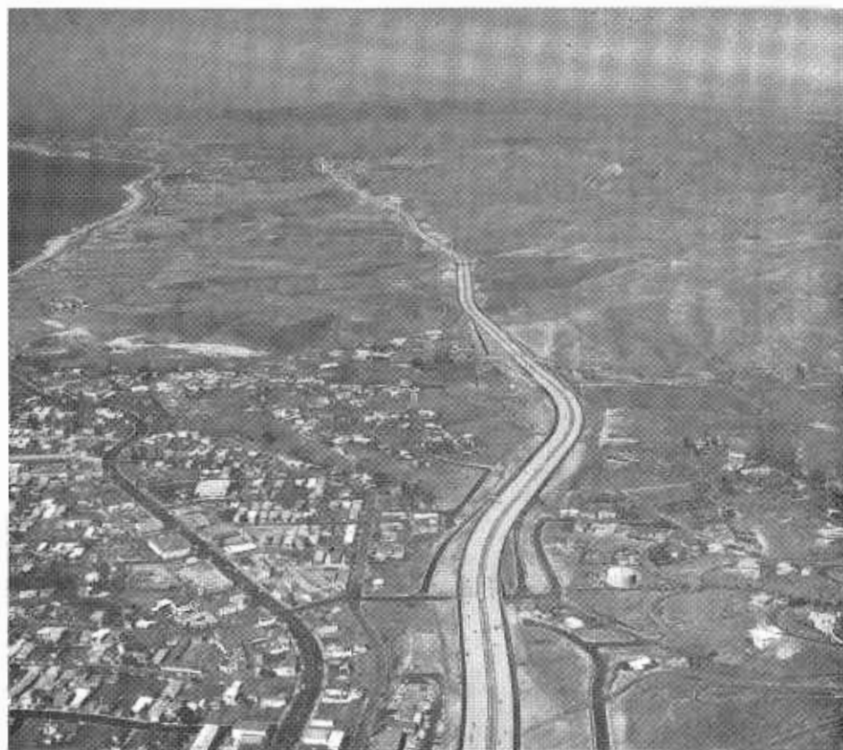
Looking north along newly completed portion of San Diego Freeway in San Clemente.
