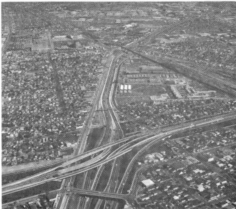
Looking south along Santa Ana Freeway at Long Beach Freeway interchange. White areas indicate added lanes on Santa Ana Freeway.
