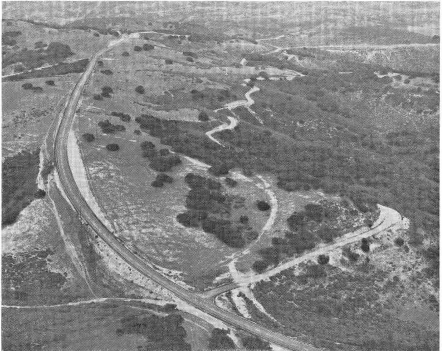
The Los Laureles Grade project, located east of Carmel and Monterey was constructed under the Federal Aid Secondary highway program and replaced a curving mountain road (sections visible in the center of the above photo) with a modern, two-lane highway. The old road has been renamed Toro Road. The view is south.
