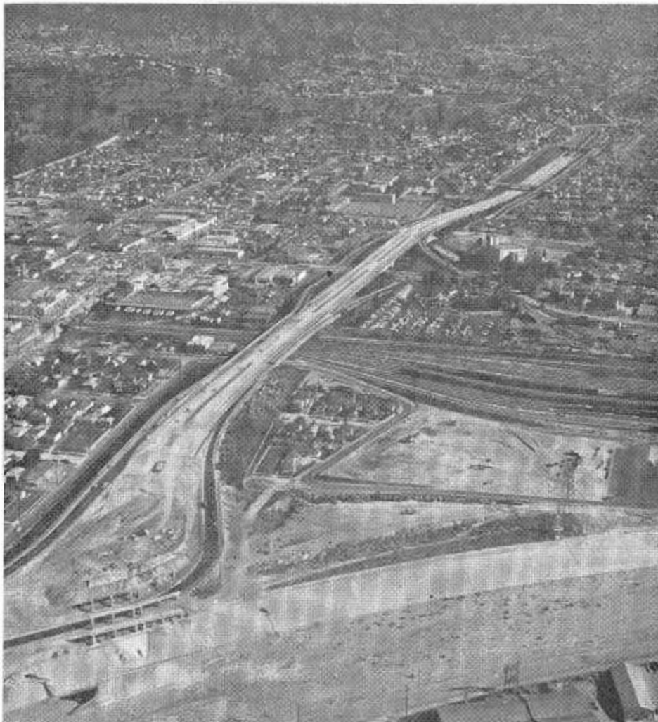
Looking easterly at completed portion of Glendale Freeway; foreground, bridges under construction connecting with interchange with Golden State Freeway.
