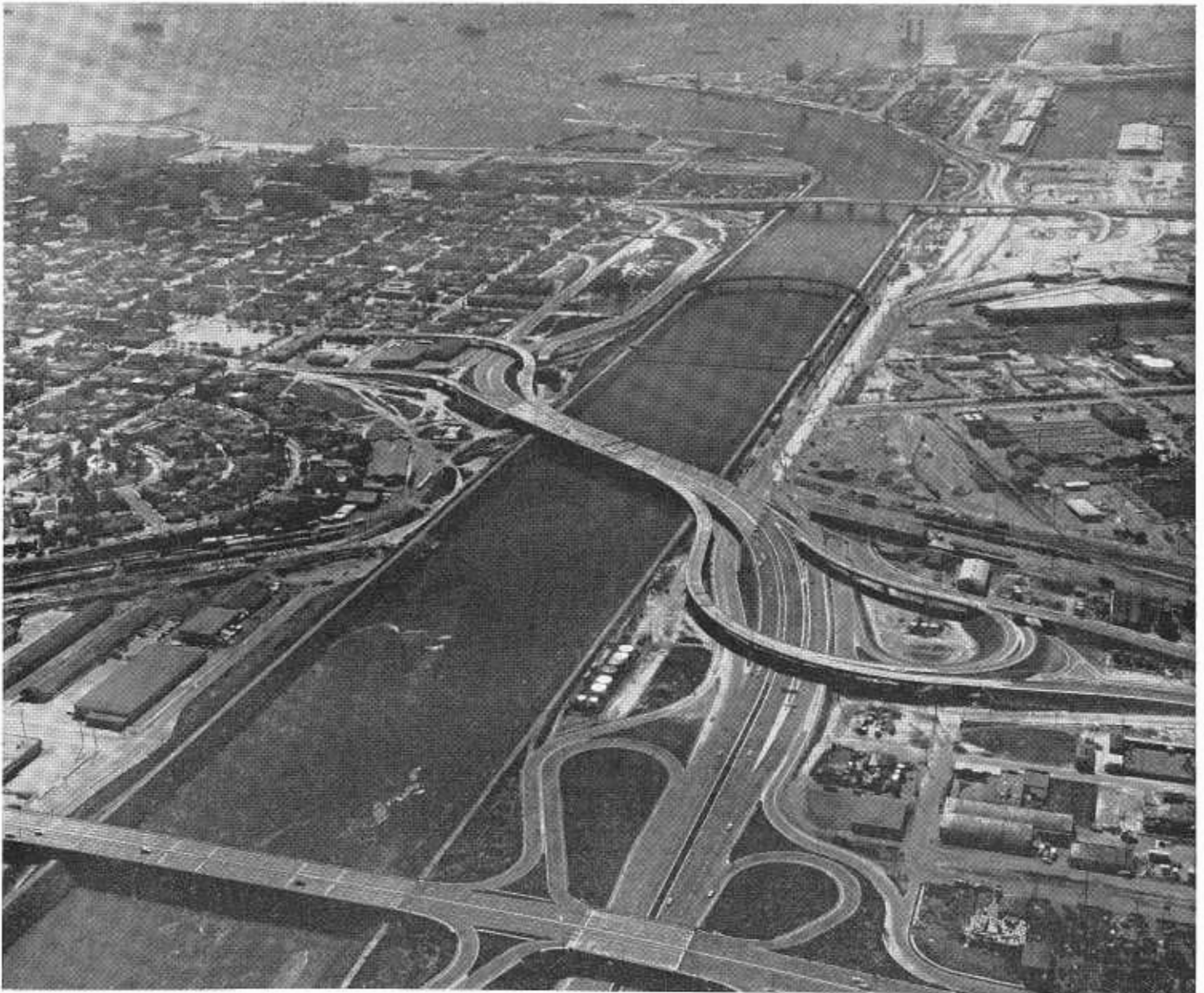
Long Beach Freeway terminus. Connections to Long Beach City Street System south of Anaheim Street, bottom.
