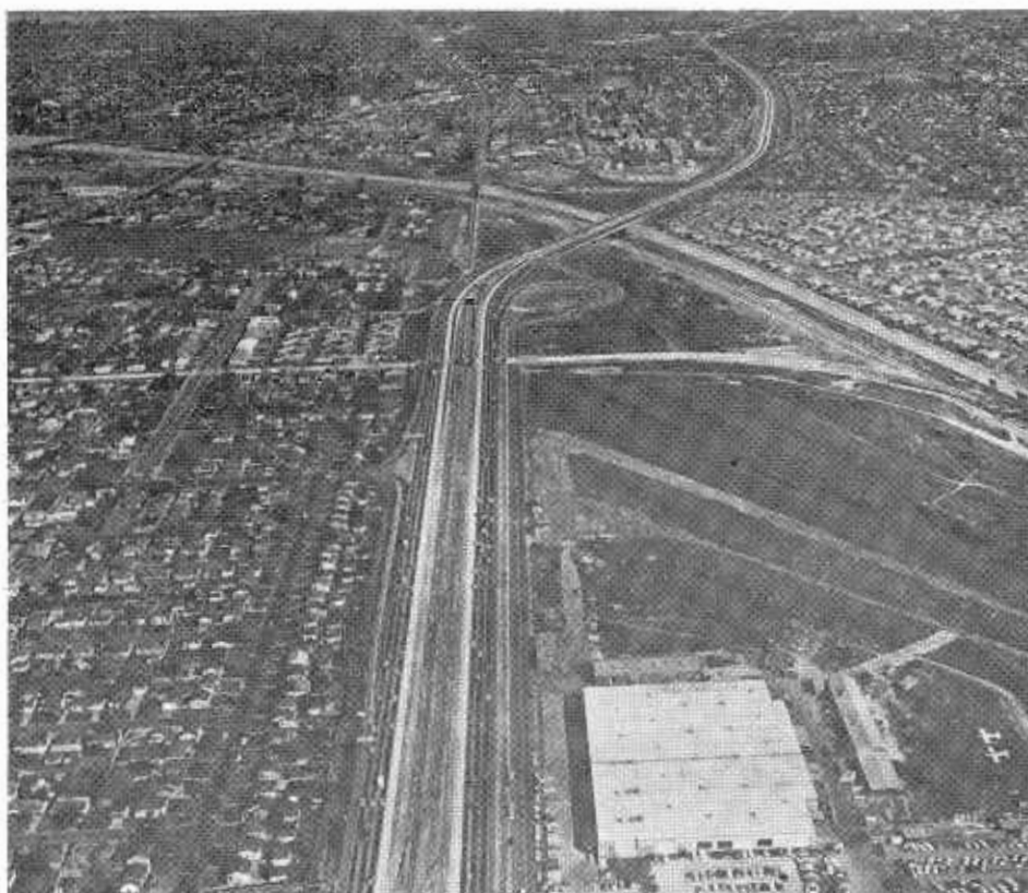
San Bernardino Freeway looking easterly at El Monte and the Baldwin Avenue interchange. The white areas in median are the newly constructed concrete pavement widening.
