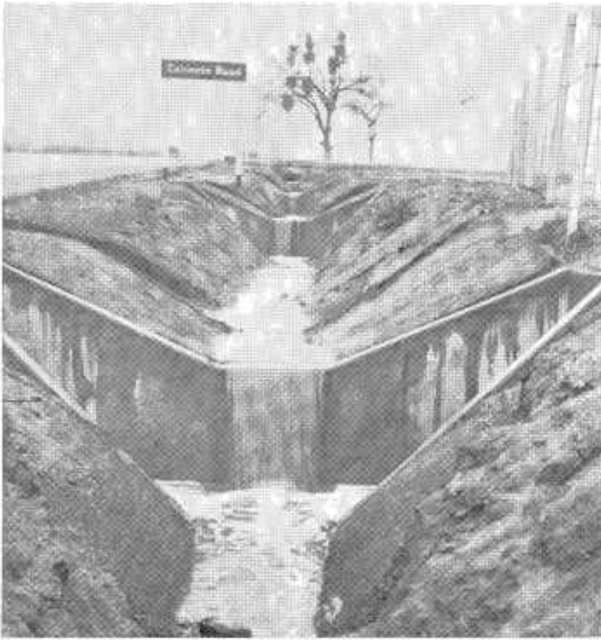
A typical reinforced concrete ditch-check series under operating conditions.
