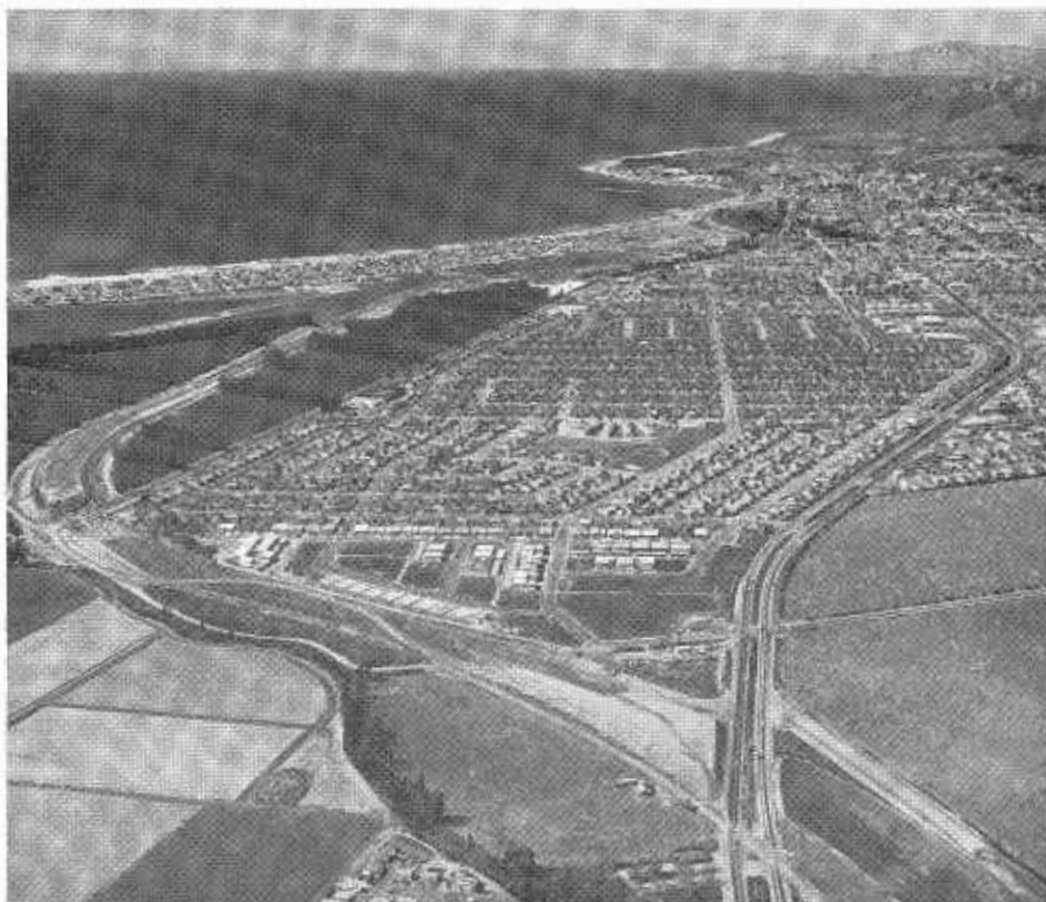
Looking northerly at construction in progress on the Ventura Freeway in the City of Ventura.
