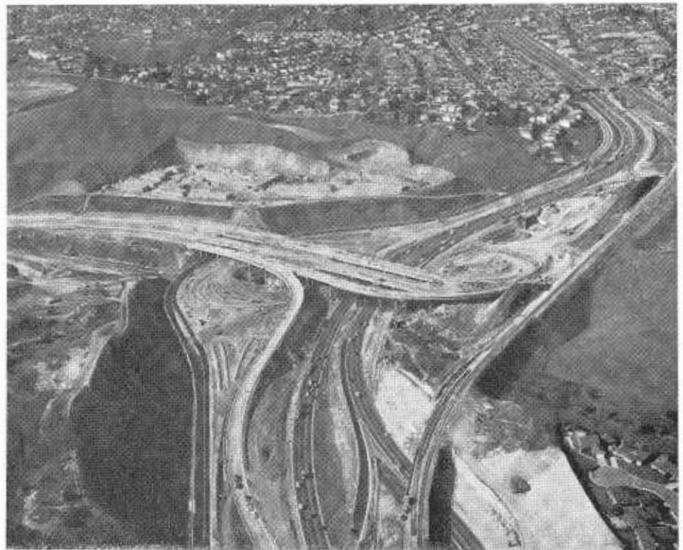
Long Beach-San Bernardino Freeway interchange looking westerly.
