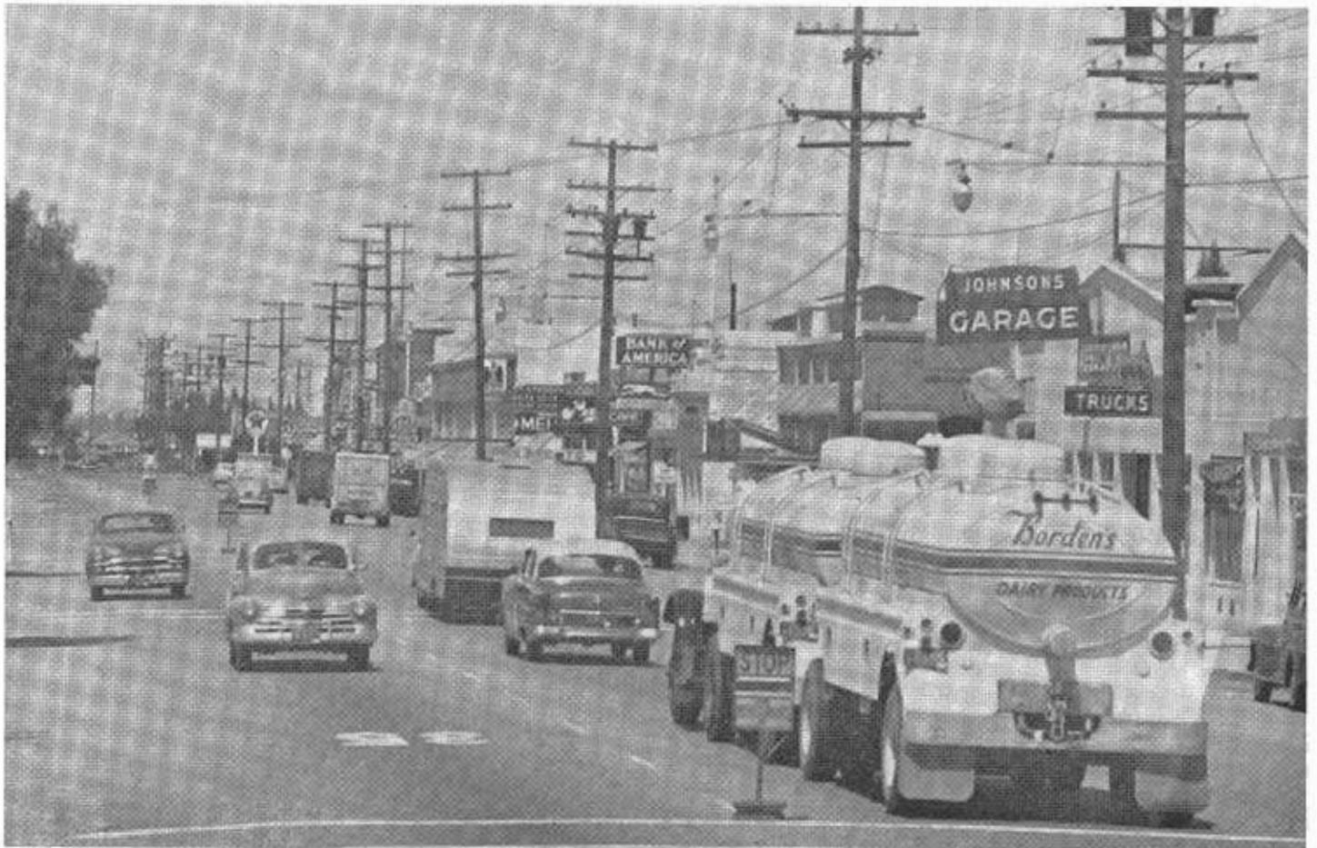
US 101 through the City of Soledad showing congestion typical of past years before construction of the freeway bypass.
