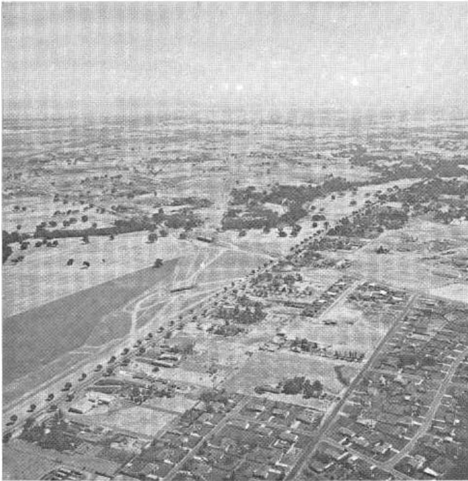
Looking toward Roseville when construction on the freeway was just beginning in 1954. Compare this photo with the one on page 31.
