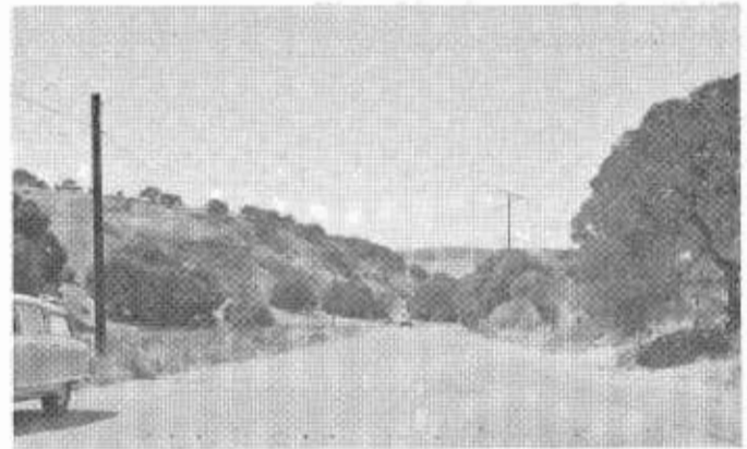
AFTER. The same section following completion of the project.
