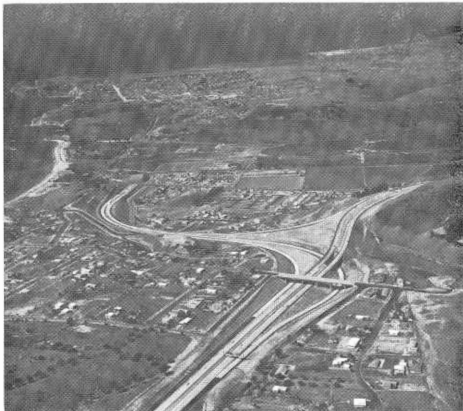
Looking north along completed San Diego Fwy. toward Dana Point, top, left. In foreground is connection at Serra Junction to existing Pacific Coast Highway.
