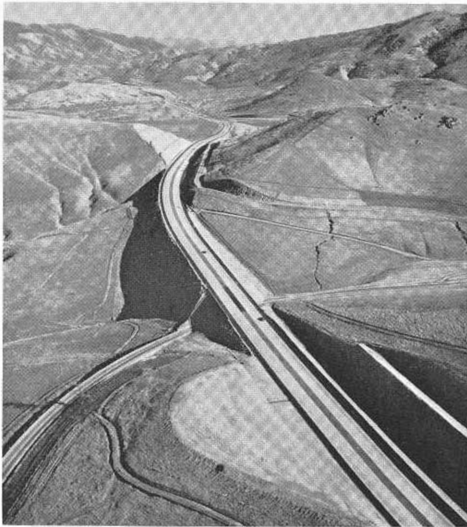
Looking east on US 466 about 1½ miles west of the Arvin Turnoff. Caliente Road passes under the freeway in the foreground.
