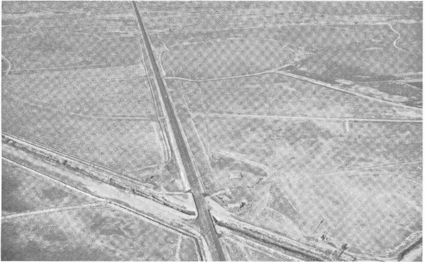
A northward view of the new Los Banos-Turlock Road showing the Santa Fe Canal crossing in the foreground.
