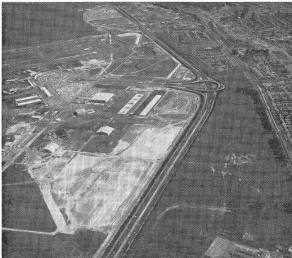
The Bayshore Freeway (looking south) near the International Airport where a fourth lane in each direction has recently been completed.
