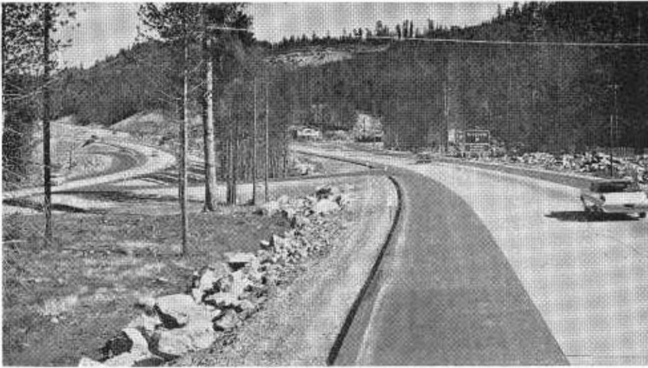
Section of U.S. 40 (Interstate 80) in the Sierra Nevada showing dike and cleared area outside it. Dike is essentially for control of runoff water, but also catches many cigarette butts.
