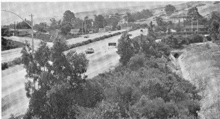
Dense growth of drought resistant plants on U.S. 101 in San Luis Obispo serves to delineate turnoffs, to lessen fire hazard, to keep down weeds, to screen and to beautify.
