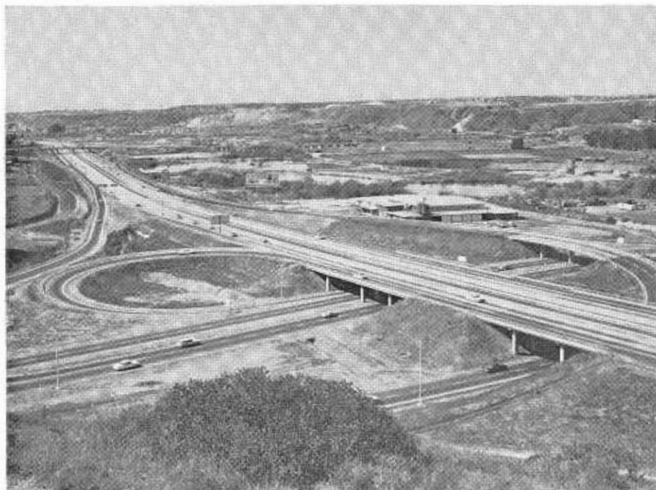
The Fairmount Avenue-U.S. 80 interchange, looking northwest.
