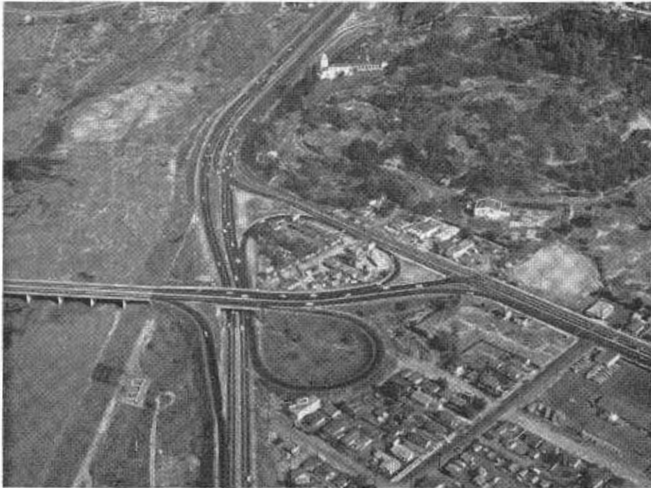
Looking eastward on U.S. 80 showing Morena Boulevard (overcrossing and bridge foreground) and Taylor Street (joining U.S. 80 from the right).
