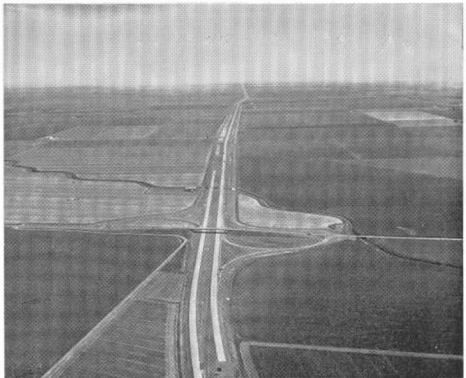
This aerial view showing the freeway under construction illustrates the intensive cultivation practiced in the area.
