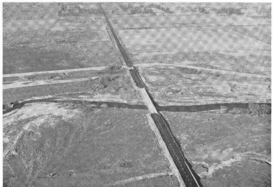
This bridge across the San Joaquin River is on the new Los Banos-Turlock Road constructed under the F.A.S. program in Merced County.
