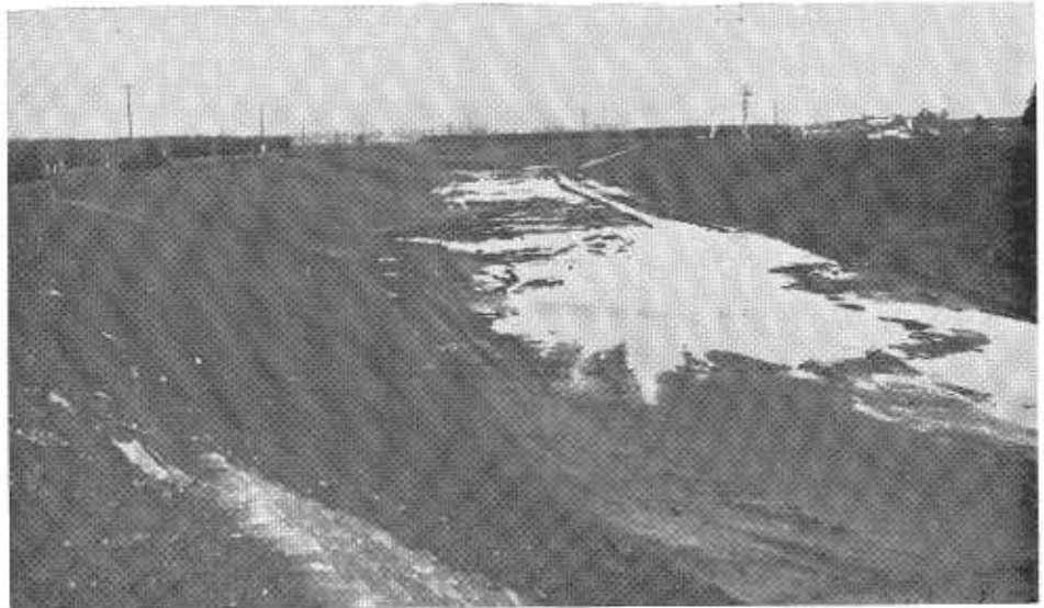
The Guadalupe River channel looking downstream from the Brokaw Road Bridge.
