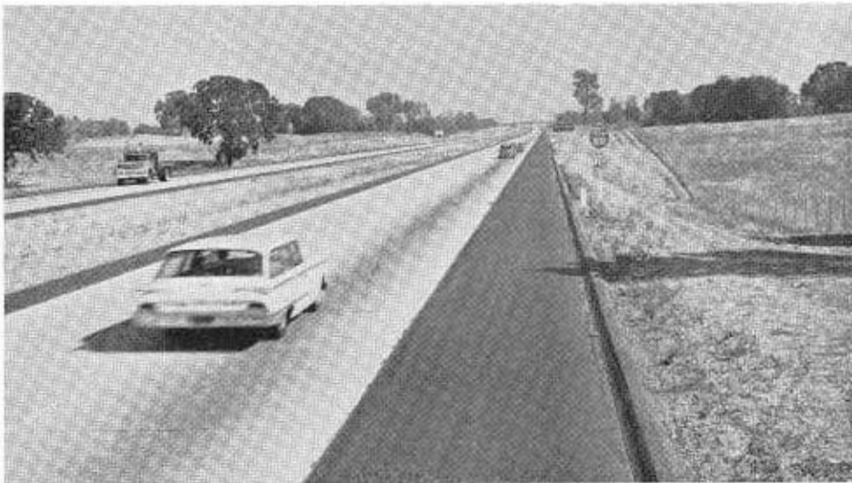
Neatly trimmed section of U.S. 40 near Roseville blends into surrounding landscape.
