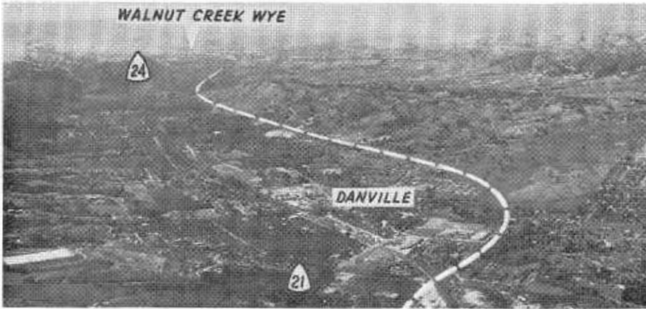
Looking north along existing Sign Route 21 showing Danville in the center. Dotted line shows adopted alignment for future construction.
