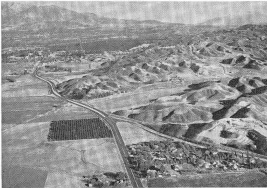
New section of county expressway on Washington Street and Barton Road in San Bernardino County, constructed under the FAS program.
