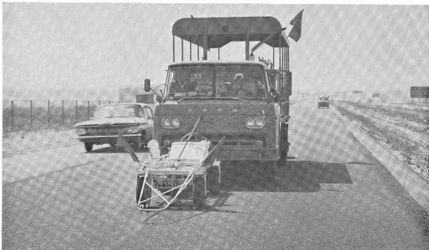
Pushbutton traffic striper used to paint the yellow and white lines on pavement.
