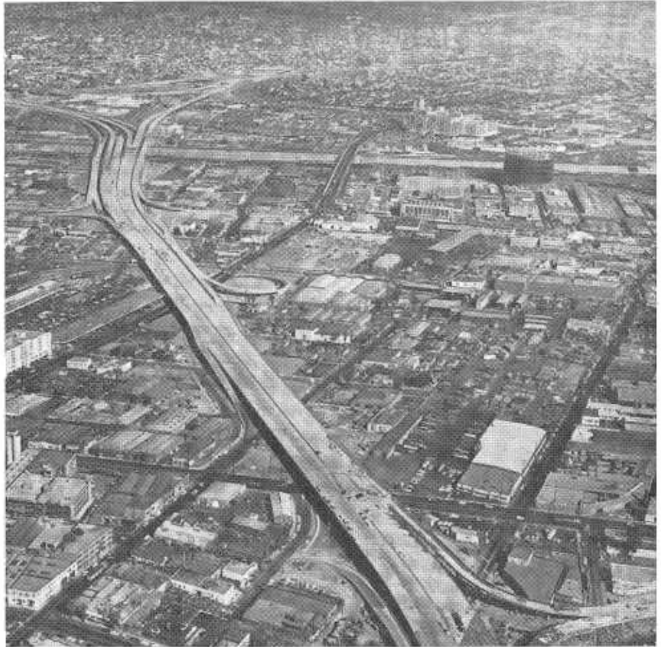
This recently completed section of Santa Monica Freeway viaduct will be part of the 29-mile "loop bypass" which will skirt downtown Los Angeles and provide relief from traffic pressure on other central district freeways. The Los Angeles River Bridge and the East Los Angeles Interchange are at upper left.
