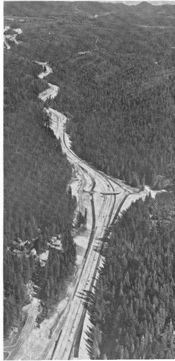
Interstate freeway construction on U.S. 40 near Baxter in the Sierra
