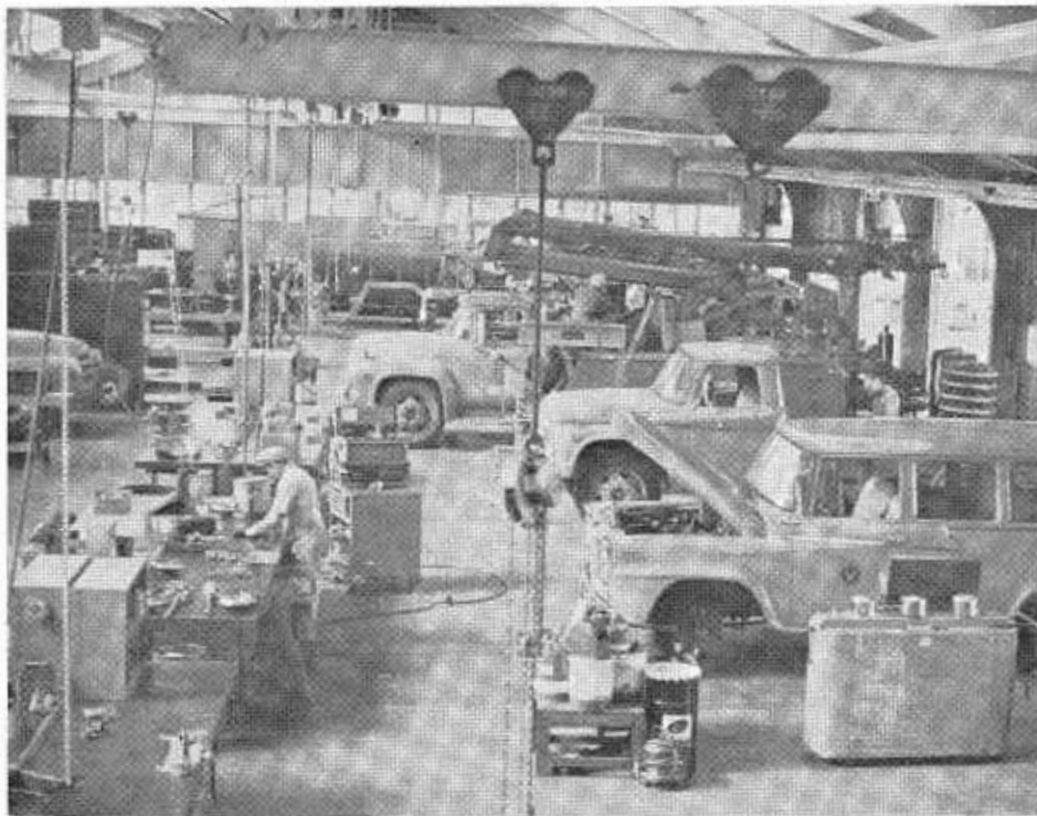
Interior view of Equipment Department's newly constructed truck shop in Sacramento.
