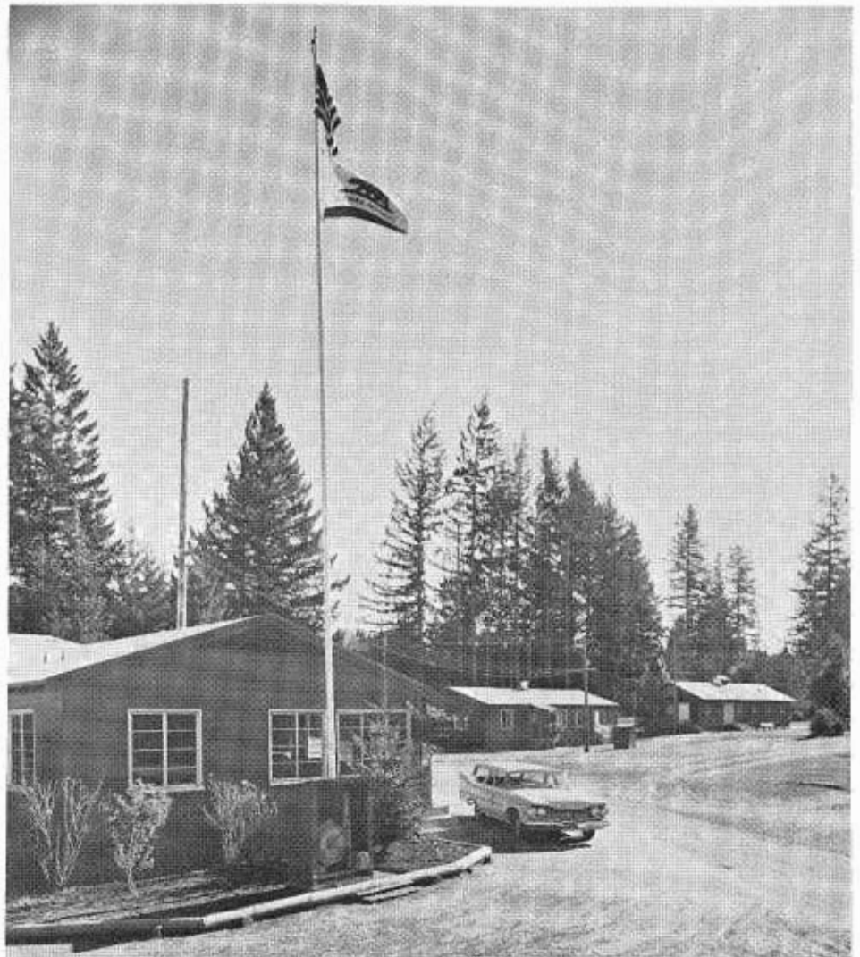
The Division of Highways and the Department of Corrections jointly operated road building Honor Camps at three remote locations during the fiscal year. Pictured here is Camp 42 in Humboldt County. At the end of the year, some 60 inmates were stationed at this camp for work on U. S. Highway 299.
