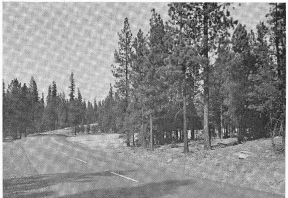
The Feather Lake Highway in Shasta and Lassen Counties was improved to modern standards under the Federal Aid Secondary County Road Program and recently became part of the State Highway System.
