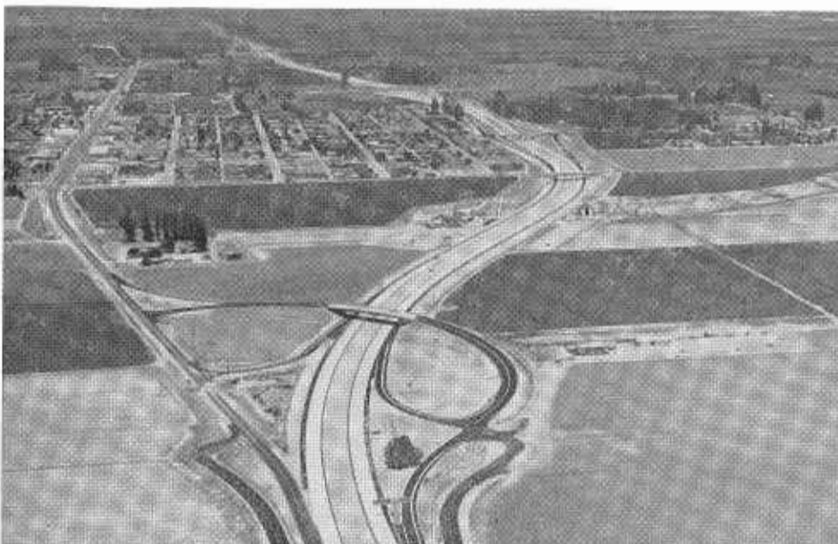
US Highway 101 is rapidly being converted to freeway and expressway standards. This new freeway bypass at Greenfield, Monterey County, is typical of the tremendous improvements which are being made.
