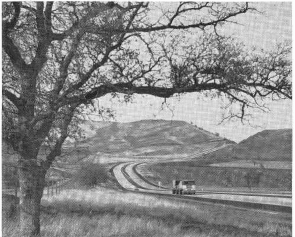
Cross-state traffic now rolls along on this new section of US 466 freeway in eastern Kern County, which was opened earlier this year.
