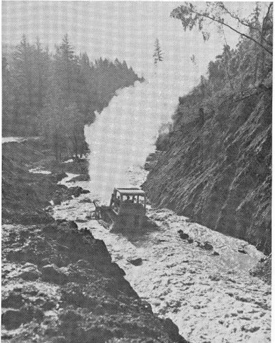
A bulldozer cuts a channel through a slide which blocked Long Valley Creek and caused flooding on U.S. Highway 101 in Mendocino County. (See picture on page 26.)
