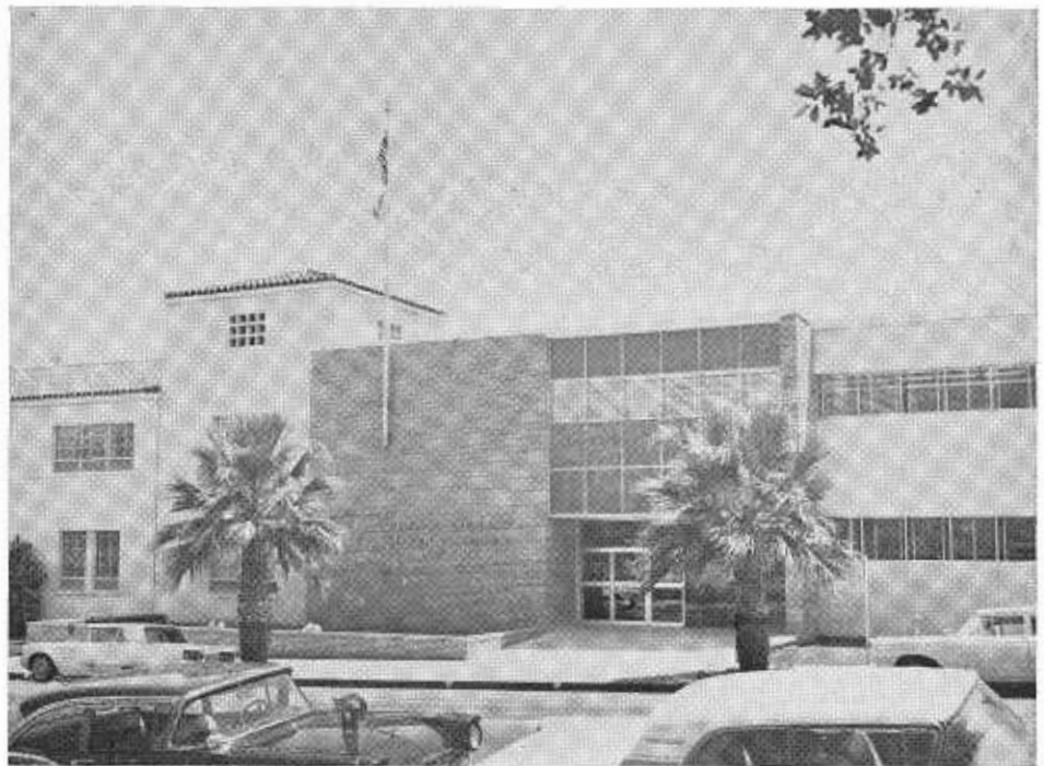
A view of the front entrance of the new Highways building in San Bernardino. Tiled-roof section to the left was constructed in 1952.
