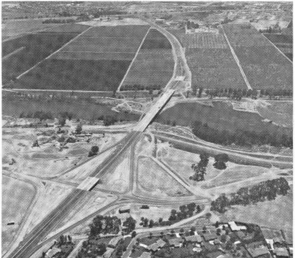
AFTER —The completed Watt Avenue Bridge and freeway section looking south toward U.S. 50. The structure immediately beyond the bridge will be part of an interchange to serve a proposed housing development on the south side of the river.
