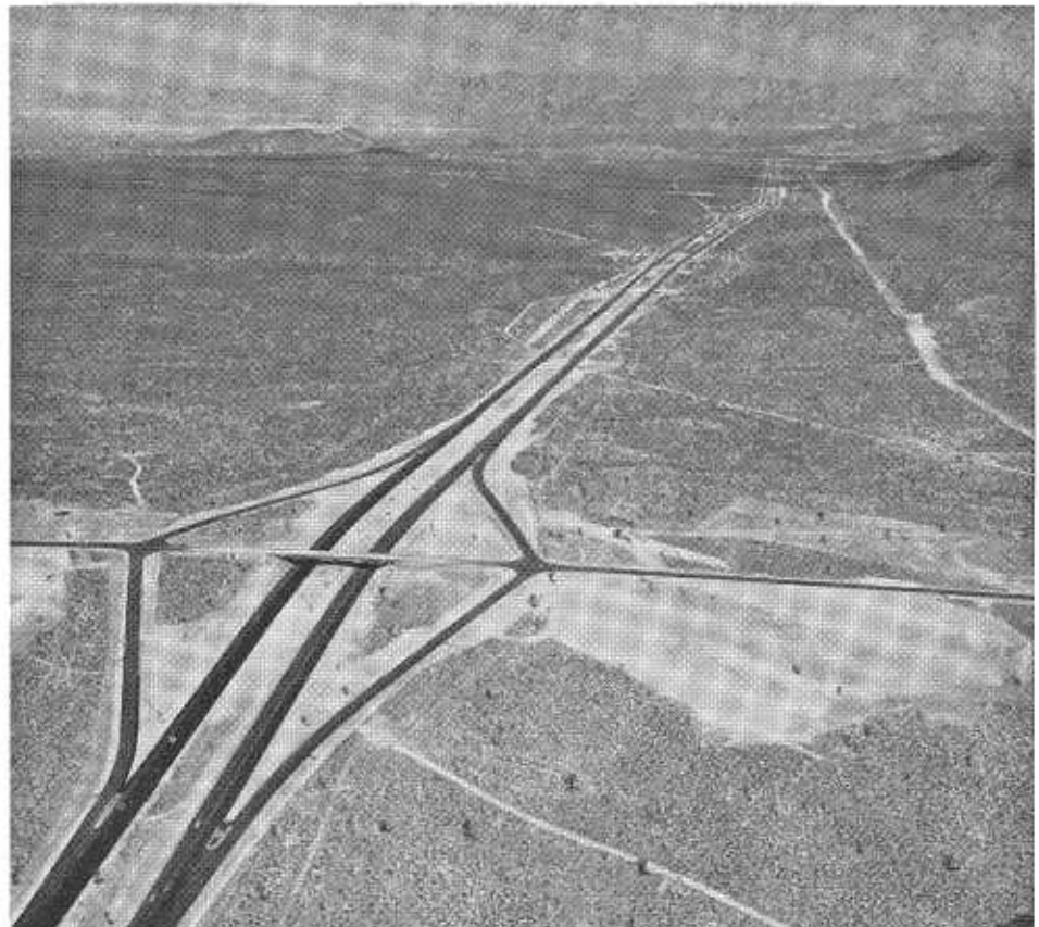
BELOW: Looking down the Baker Grade from Halloran Summit Overcrossing. Note the restoration planting of Joshua and native plants at the Interchange.
