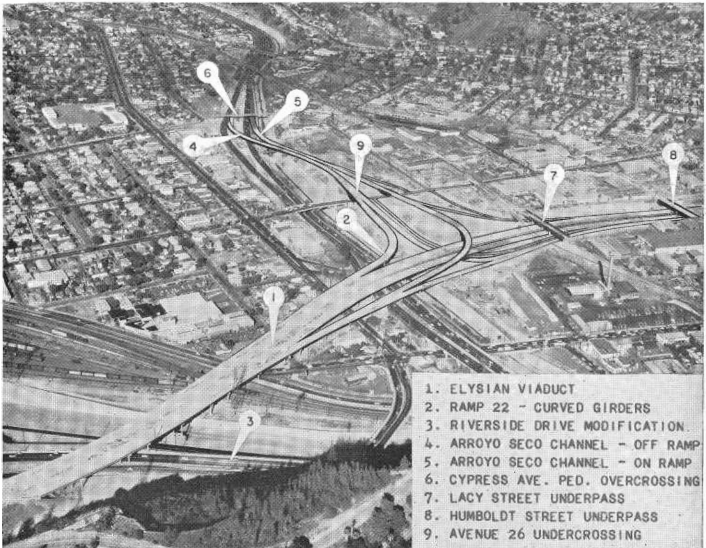
The numbers in the above photo indicate various construction features of the interchange.
