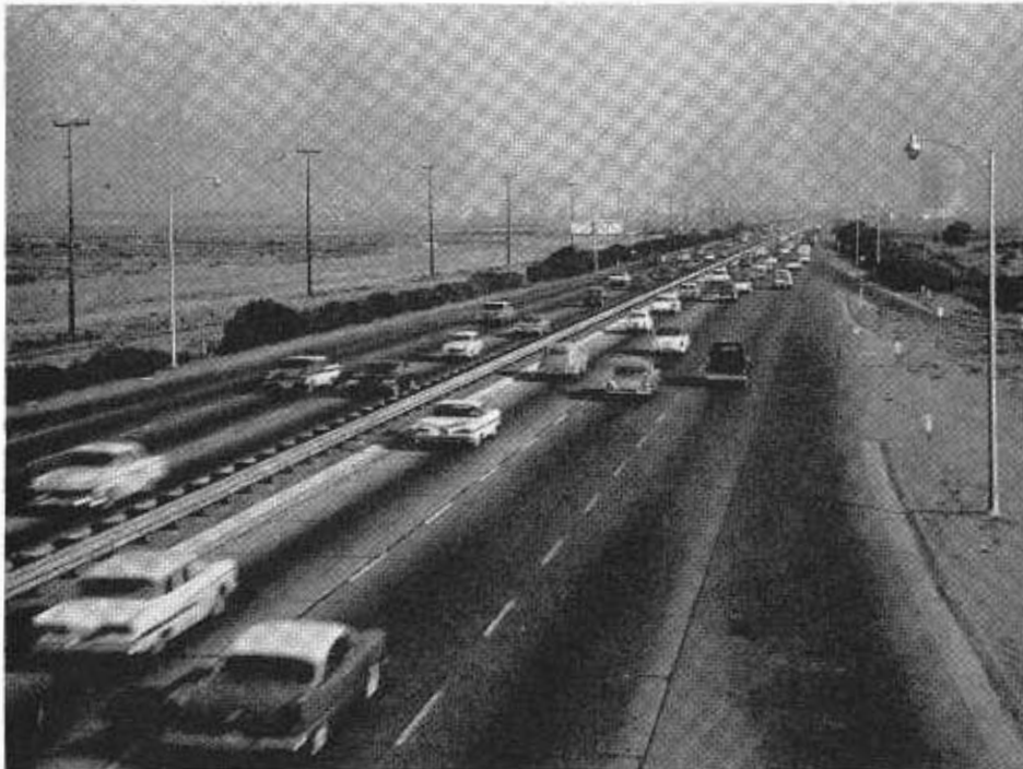
Beam barrier on a heavily-traveled section of the Nimitz Freeway in Alameda County.
