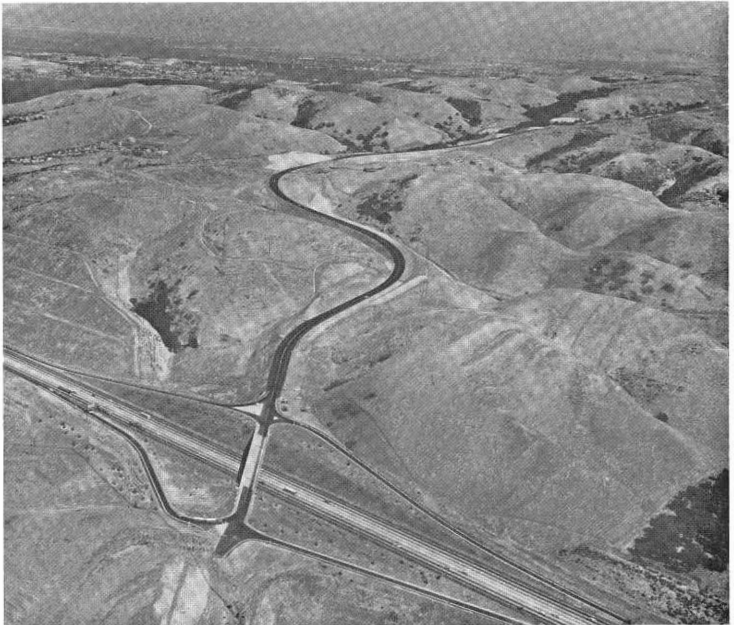
Looking eastward along the new section of the Cummings Skyway in Contra Costa County above the interchange connecting it with U.S. 40. Part of the "Big Cut" located just south of the twin Carquinez bridges can be seen to the left.
