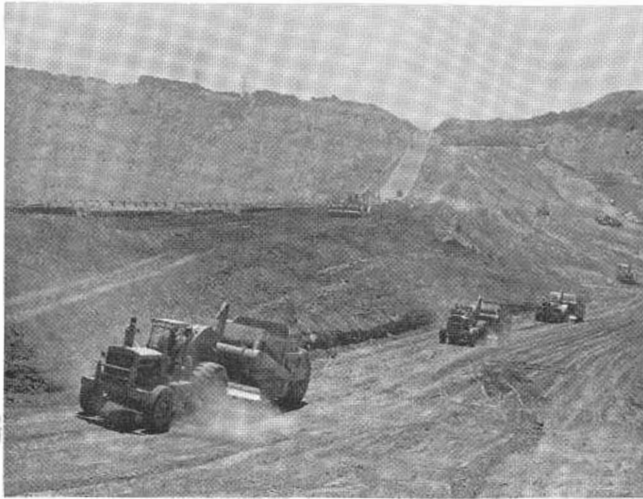
Scrapers move 1,500,000 cubic yards of material for embankment to widen U.S. 40 at American Canyon, and make this section eight lanes.
