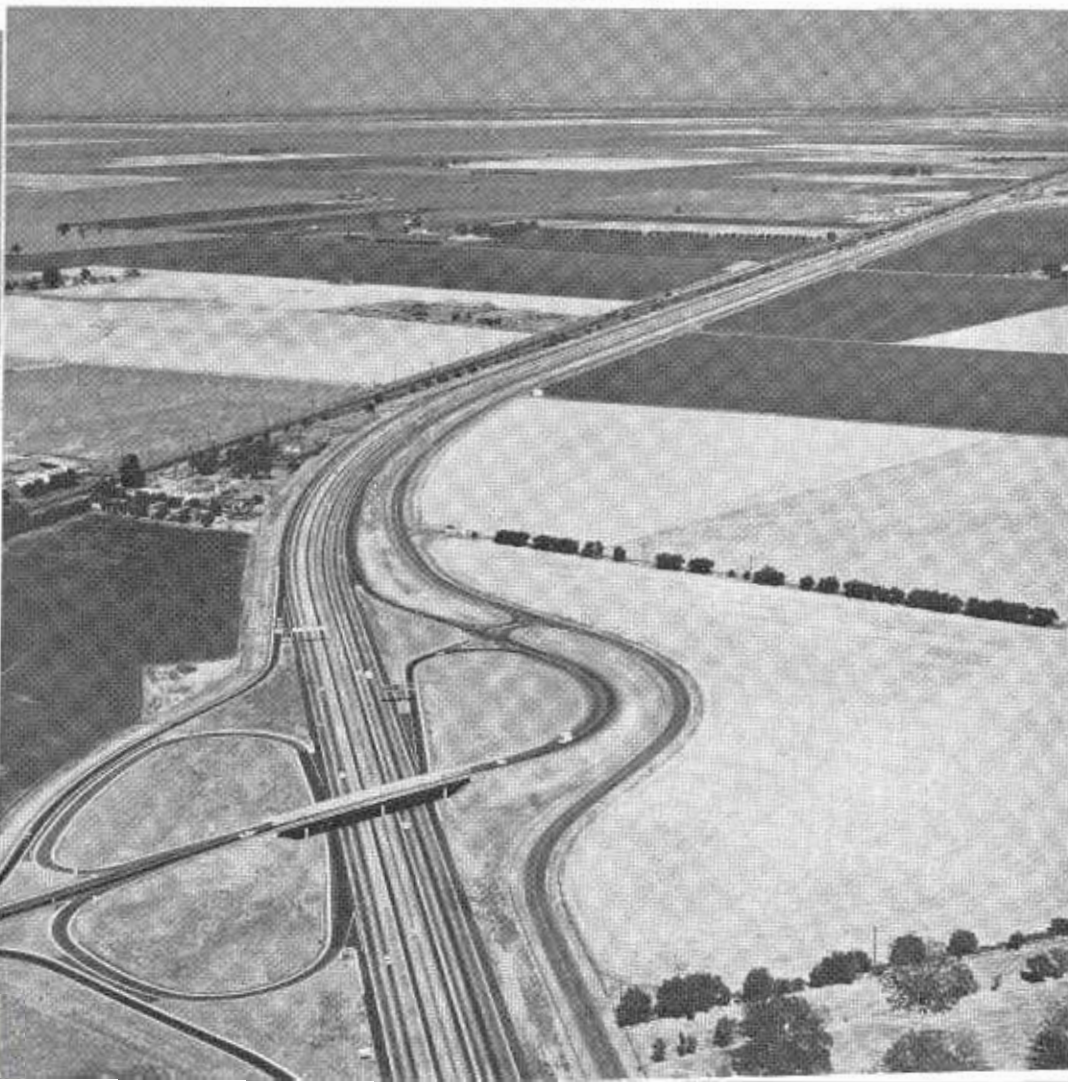
Looking east along completed section of six-lane freeway in Yolo County. Interchange connects with city of Davis.
