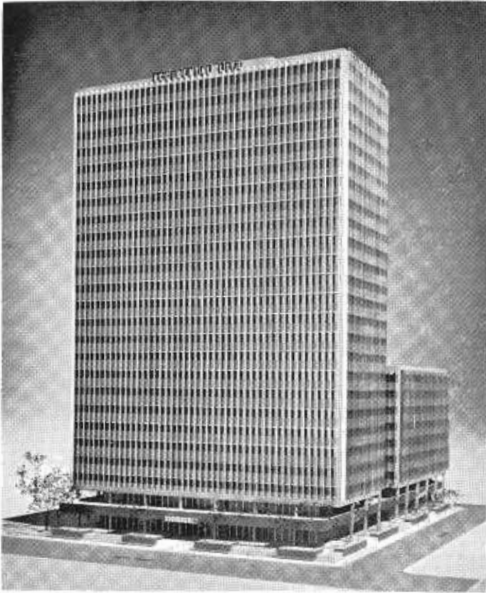
A model of the future Occidental Life Building in the downtown area. (Photo by Herbert Bruce Cross.)
