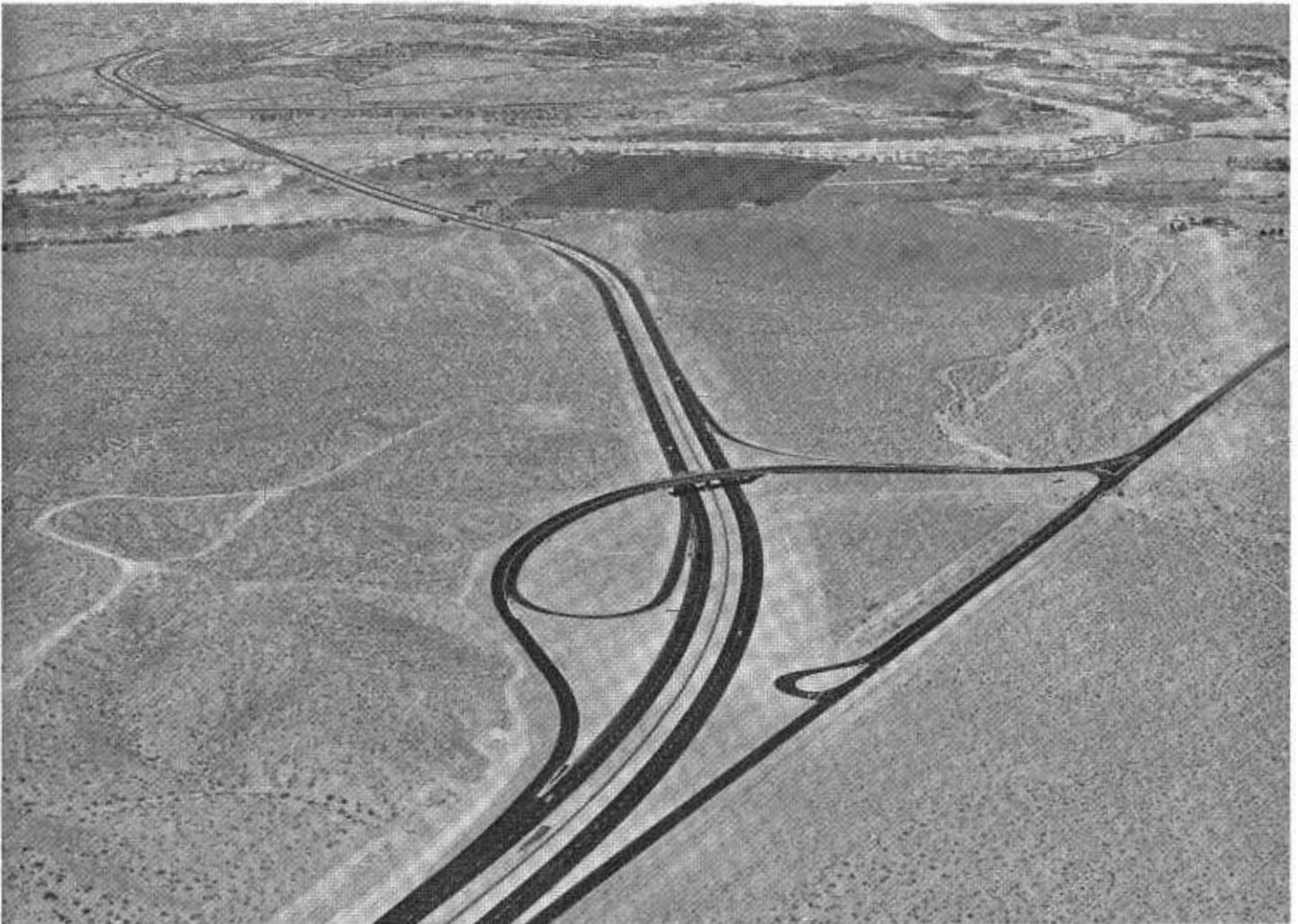
U.S. 91 and 466 crosses the Mojave River to the City of Barstow in the background. U.S. 466 separates to the right in the lower left portion of the photo.
