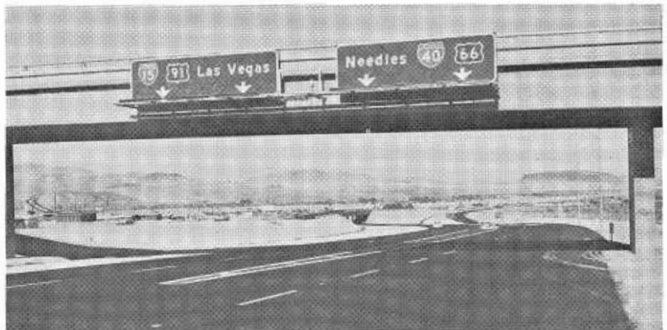
The junction of U.S. 66 and 91 on the new freeway. Muriel Avenue Overcrossing is in the immediate foreground.
