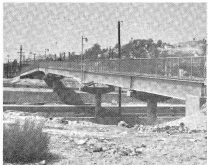
The Cypress Avenue Pedestrian Overcrossing is a welded steel structure, 440 feet long, which replaces an old timber truss structure.
