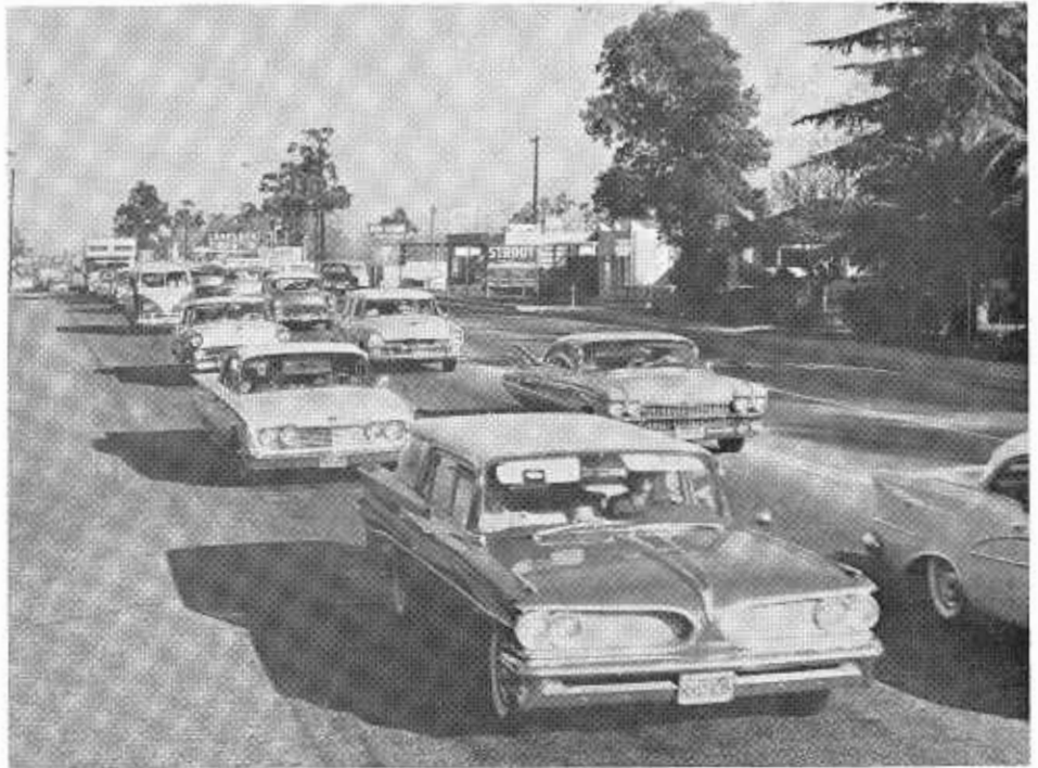
BEFORE —The Sixth and Magnolia Avenue intersection on US 60-70-99 in Beaumont taken in February of last year before the opening of the freeway. The view is eastward.
