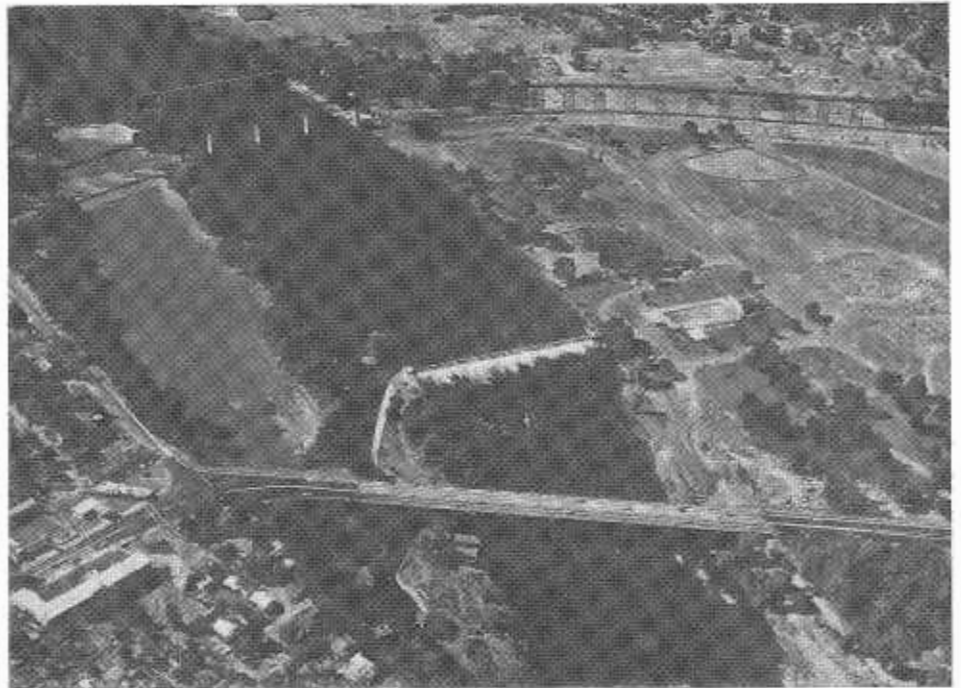
The structure in the foreground is the Highway US 99 bridge which spans the Sacramento River at Redding. Immediately upstream is the Anderson-Cottonwood Irrigation District diversion dam. The next upstream structure is the 4,353-foot Southern Pacific Railroad trestle. Farthest upstream is the Diestelhorst Bridge which carried Highway US 99 traffic across the river until replaced in 1935.
