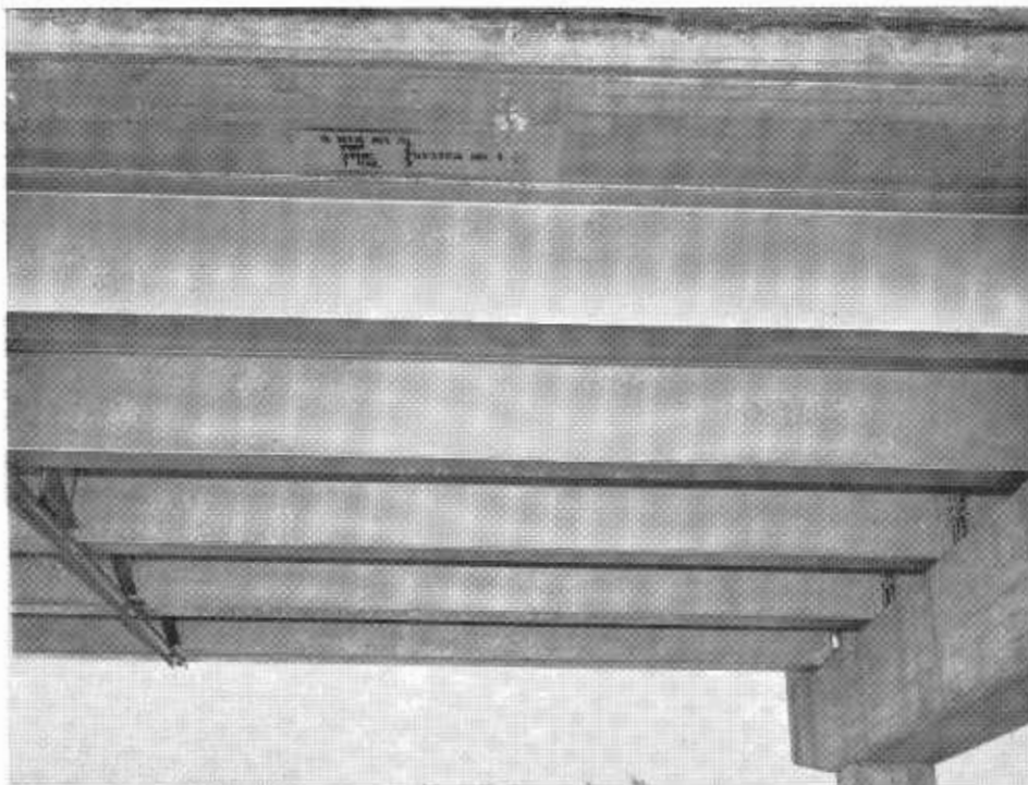
FIGURE 3—Under view of the south portion of Span 2 on which Painting System No. 1 was used.
