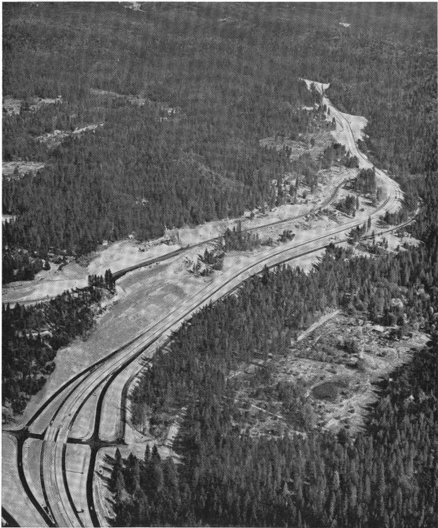
Recently opened new Interstate Section of US 40/Interstate 80 just above Monte Vista. Southern Pacific Lines run diagonally across photo above highway, in foreground is Towle interchange.
