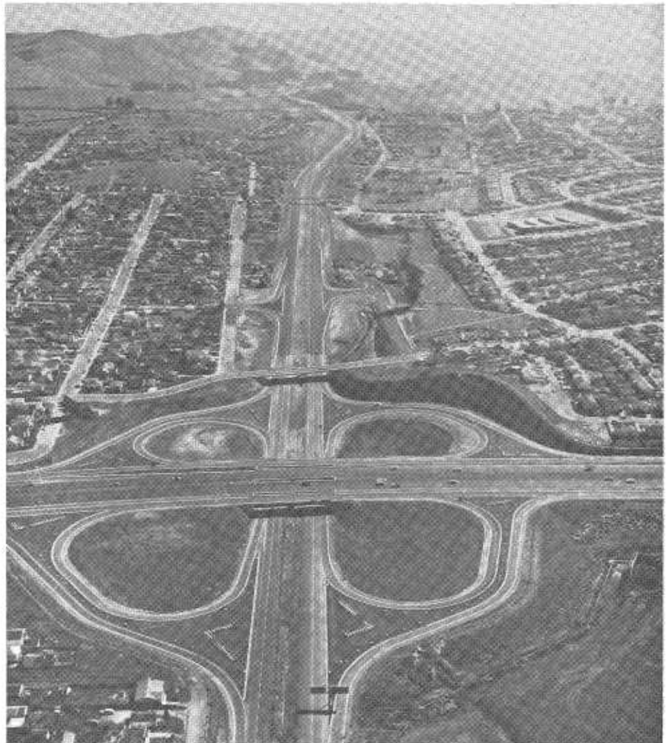
Looking east on Interstate Route 680 from above the cloverleaf intersection with US 40. Immediately beyond the cloverleaf is the Laurel Street-Cedar Street interchange. Both interchanges were constructed under a previous contract.
