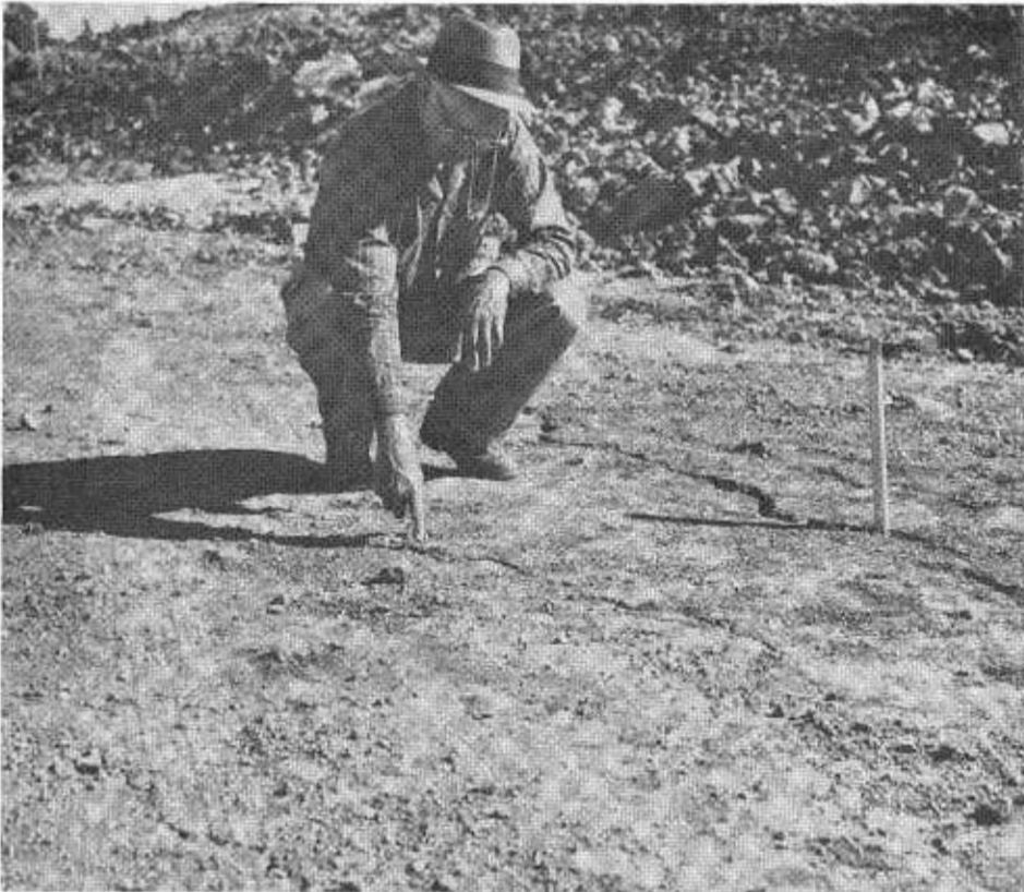
Settlement cracks in the earth strut along the north side of the sand drain area caused by the overload which is applied slowly (one foot per week).
