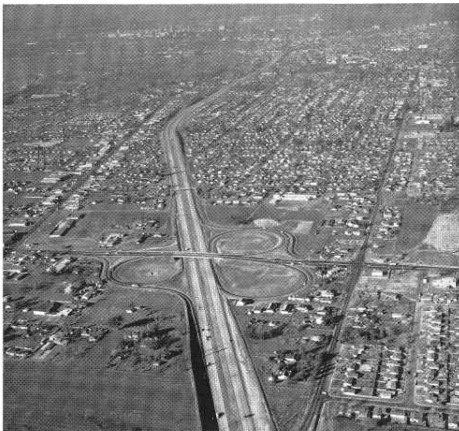
The new South Sacramento Freeway looking north toward the downtown area. The Fruitridge Road West interchange is in the foreground.
