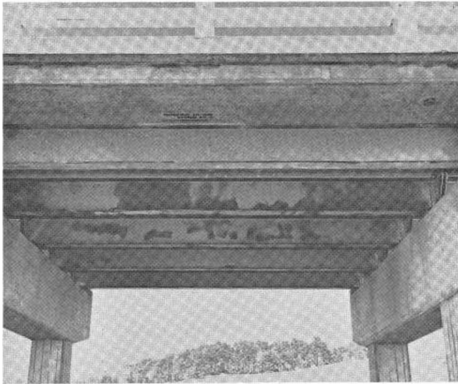
FIGURE 5—Under view of Span 3 on which Painting System No. 3 was used.
