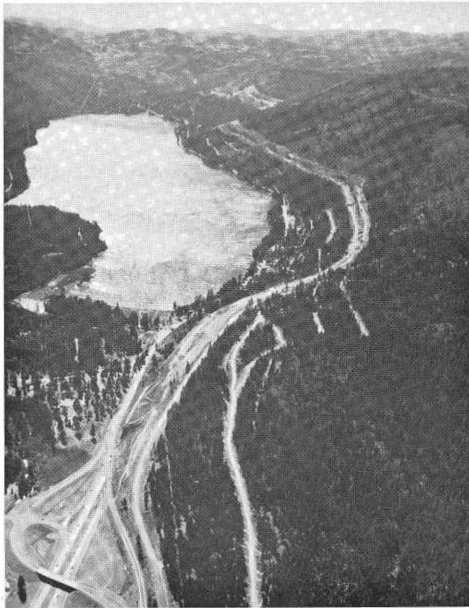
Looking west from outskirts of Truckee along US 40 Donner Lake at left and old Donner Summit upper left. Old roadway closely follows northern shore of lake, new alignment gradually gains altitude up ridge at right, then swings north and west again.
