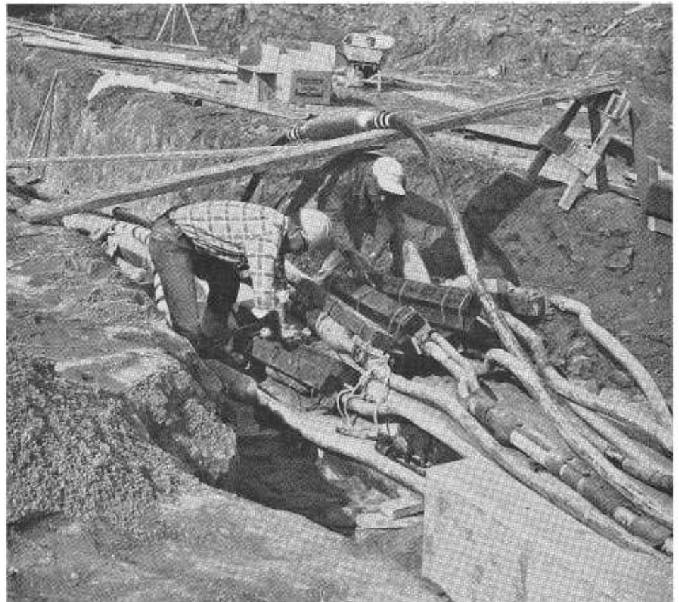
Timbers are lashed to the telephone cable splices for protection.
