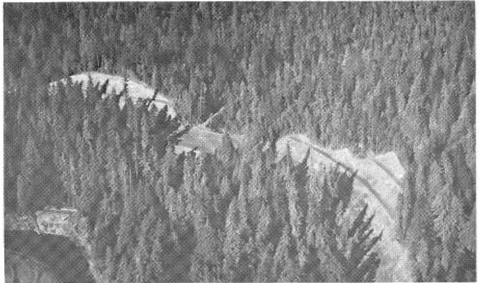
The freeway traverses rugged and heavily wooded terrain as can be seen from this aerial photo.
