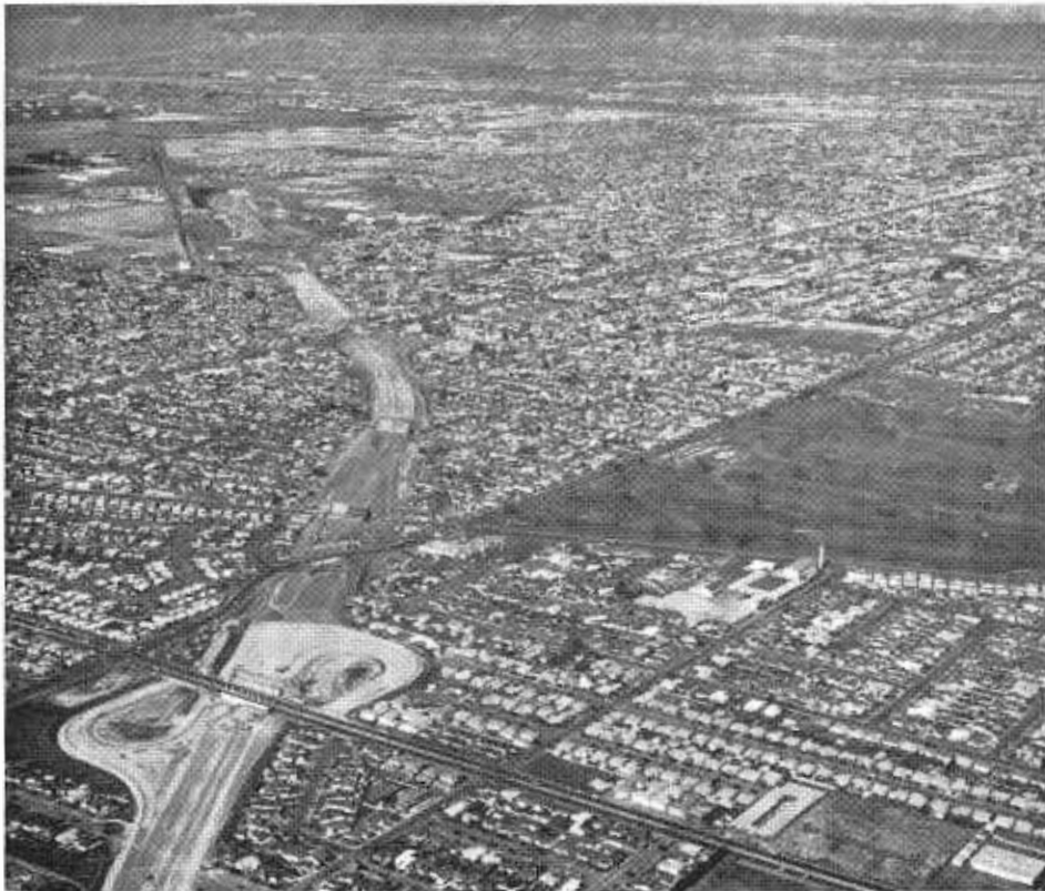
San Diego Freeway construction north from 174th Street.
