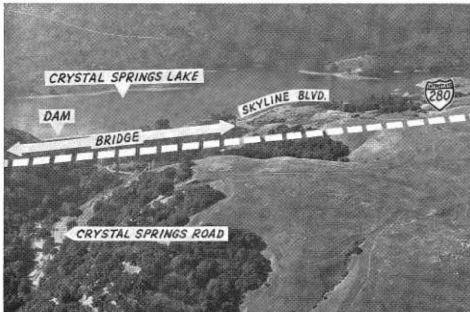
A westerly view of the Crystal Springs Lake and Dam showing the coastal hills in the background. The future bridge will be about 1,700 feet long across the canyon and about 100 feet above the dam.
