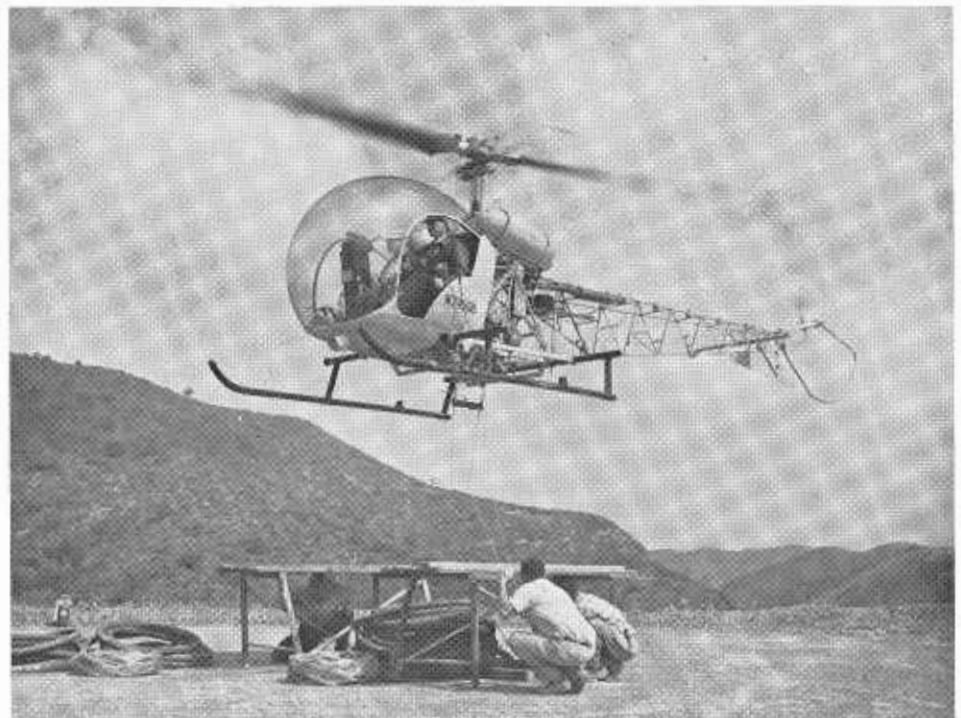
A helicopter hovers over the stand preparatory to picking up hose used to pump concrete for fence construction.
