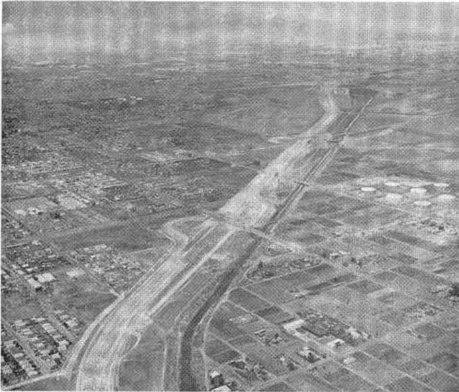
San Diego Freeway construction at Carson Street (center).
