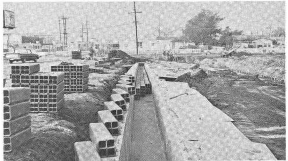
Multiple tile telephone duct installation in the new utility overcrossing bridge.
