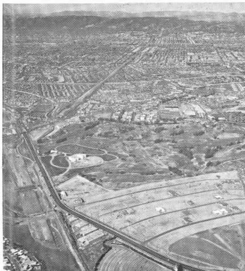
PHOTO BELOW LEFT—The temporary end of the San Diego Freeway (center) at Jefferson Boulevard. BELOW RIGHT—San Diego Freeway construction north from Rosecrans Avenue.
