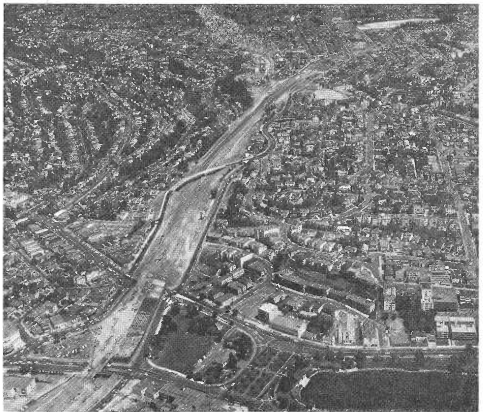
Westbound US 50 traffic is routed over the completed Lake Park overcrossing during construction.
