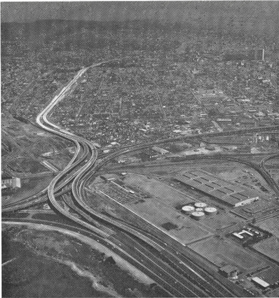
The MacArthur Freeway through Oakland looking east from the Distribution Structure. The Cypress Street Viaduct on the Nimitz Freeway curves out of the photo to the right.
