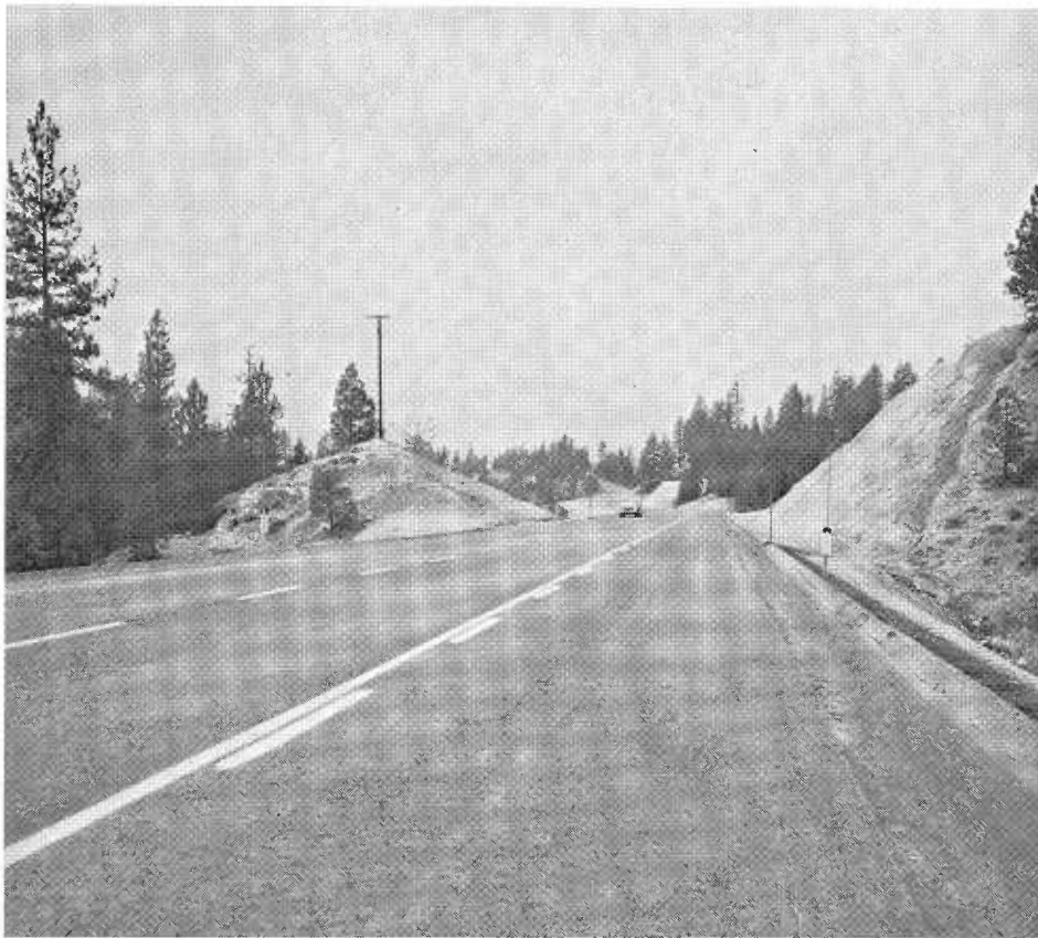
On two-lane expressways in the mountains, passing lanes are frequently provided on steep grades to alleviate tie-ups occasioned by slow-moving vehicles. Photo shows passing lane on US Highway 40 Alternate in Plumas County.
