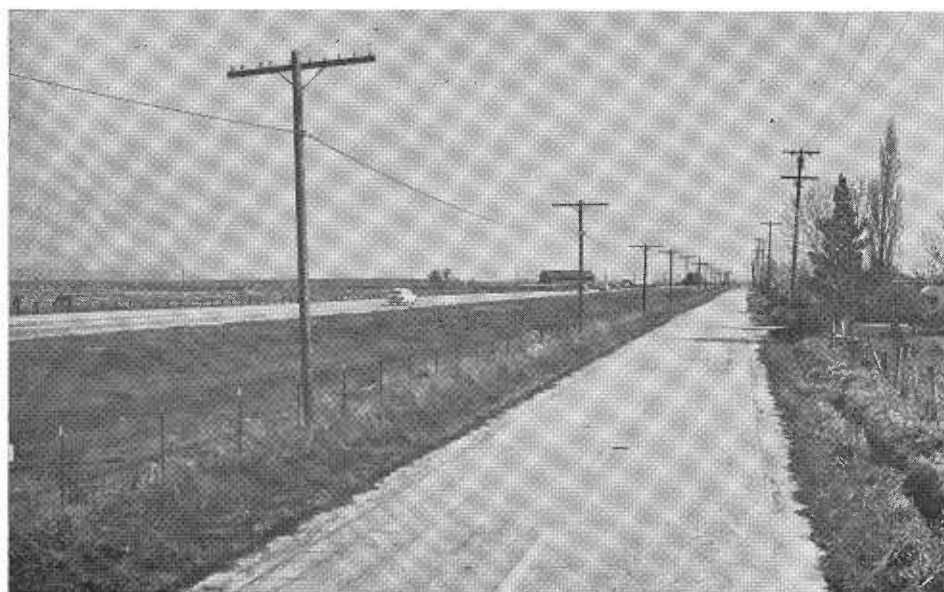
PHOTO TOP OF PAGE—Scenic two-lane expressway on State Sign Route 36 near Mineral in Tehama County. PHOTO LEFT—On this two-lane expressway section of Sign Route 120 near Oakdale, the old highway (foreground) now serves as a frontage road providing access to farms and homes.
