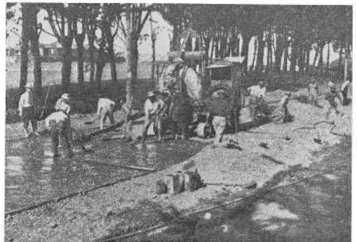
Work on El Camino Real near Burlingame, 1912.
