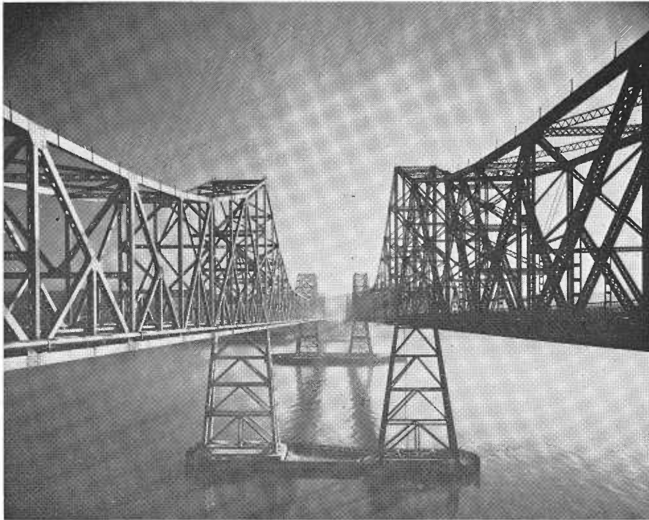
This view of the twin Carquinez Bridges shows the simple, more eye-pleasing structure made possible by the use of high-strength steels and modern welding techniques. The new structure, on the left, was built at a savings of $800,000 by using these materials and techniques.
