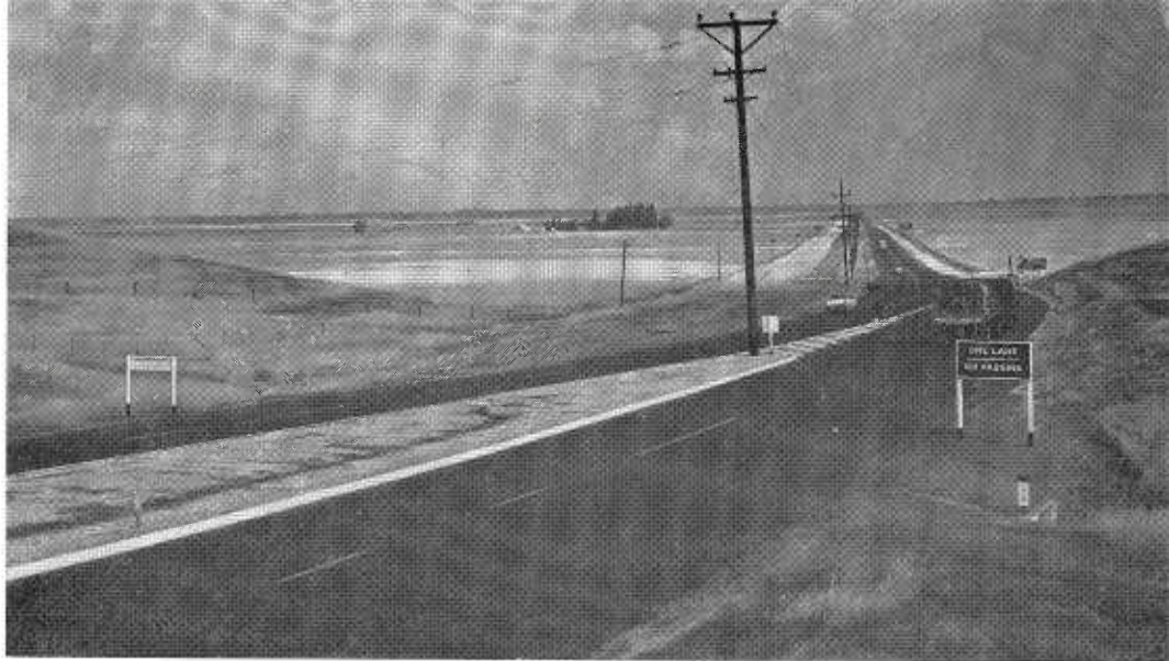
On US Highway 99E through farming country near Chico, Butte County, the unused right-of-way (left of tall utility poles) is held in reserve until four lanes are required to accommodate increased traffic volume. Shown in foreground is part of a four-lane segment at the busy Oroville turn-off intersection.
