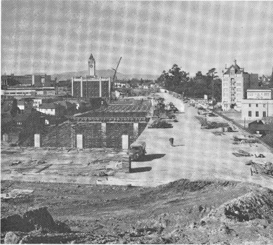
MacArthur Freeway construction at the Oakland-Harrison interchange.
