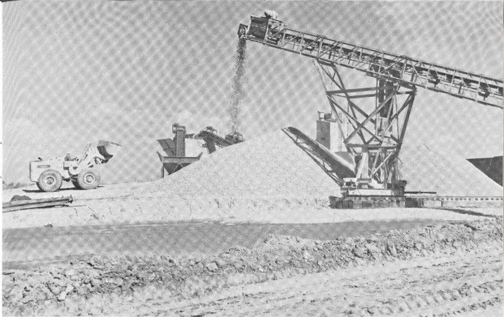
PHOTO ABOVE—The radial stacker conveyor stockpiles raw aggregates.
