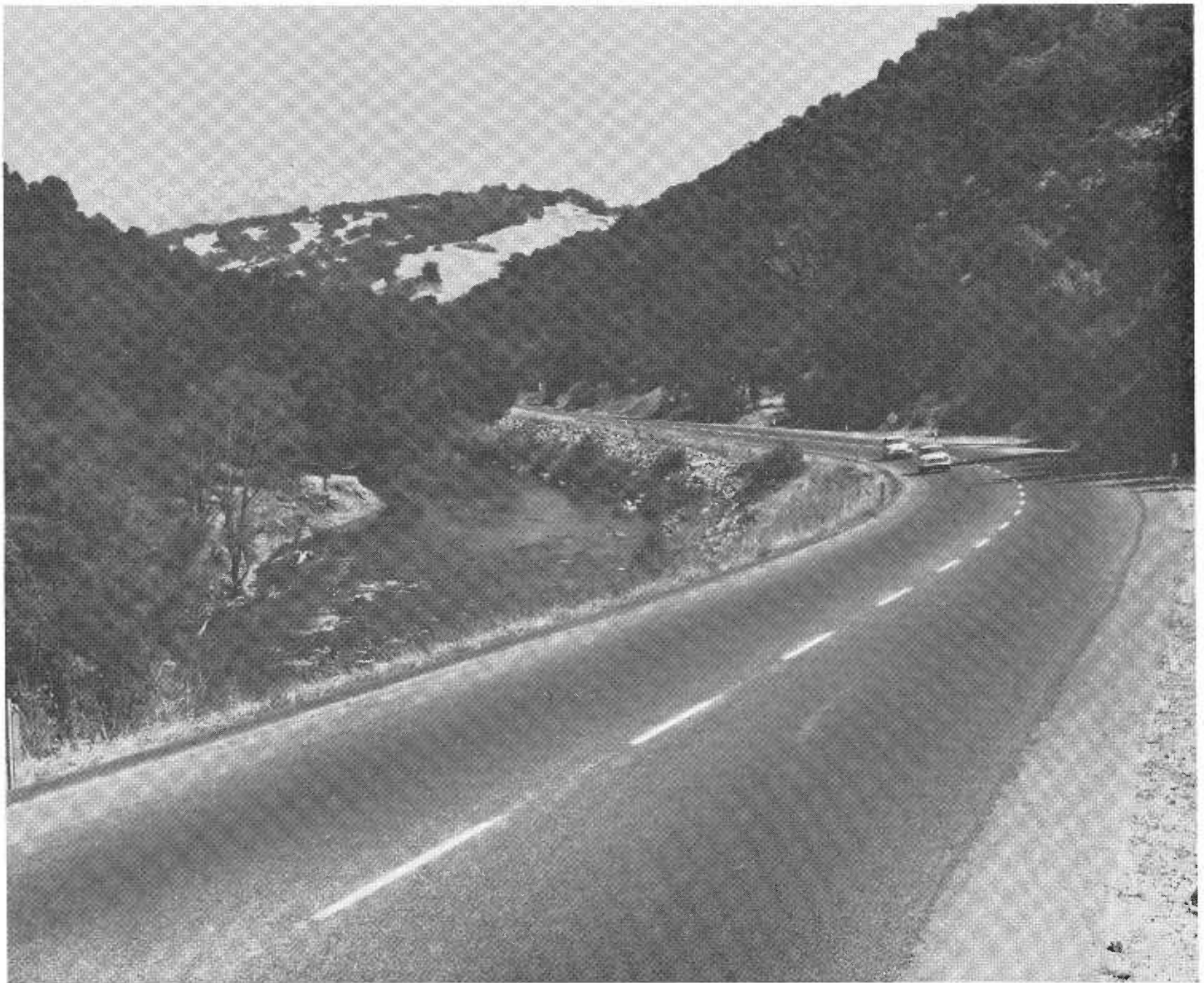
No special access-control measures have been required on this two-lane expressway section on Sign Route 20 in Mendocino County because natural terrain features—the stream and the steep wooded slope—already protect the right-of-way.
