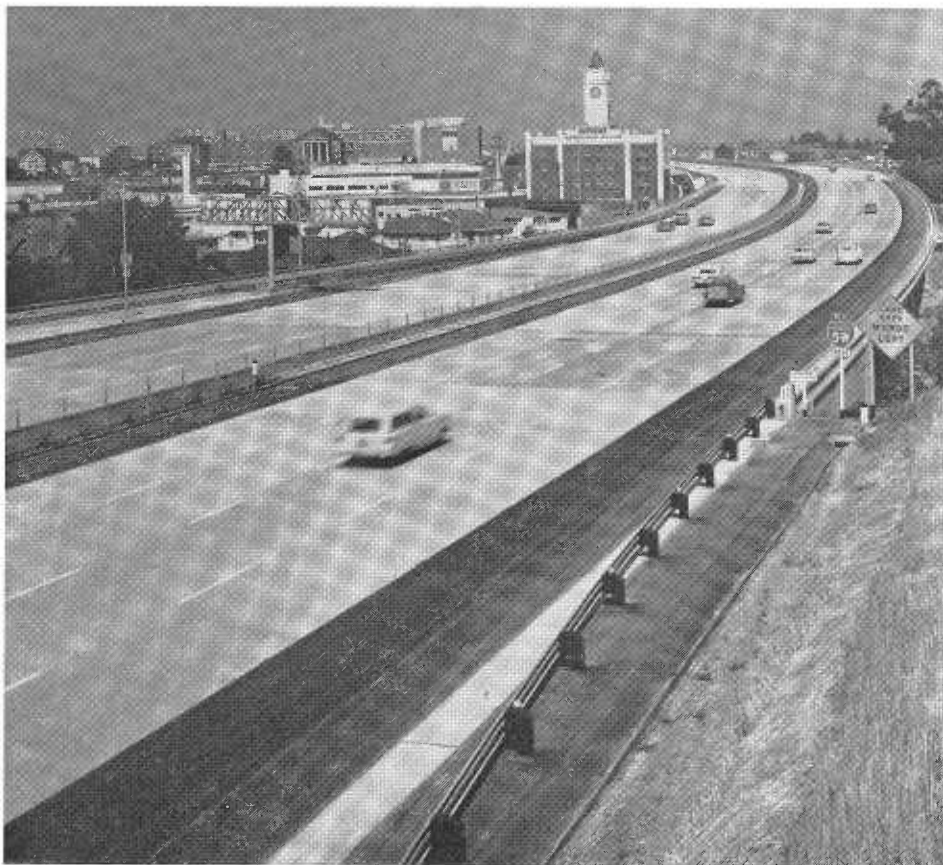
MacArthur Freeway in Oakland shortly after its completion. Broadway passes under the freeway by the building with the clock tower.
