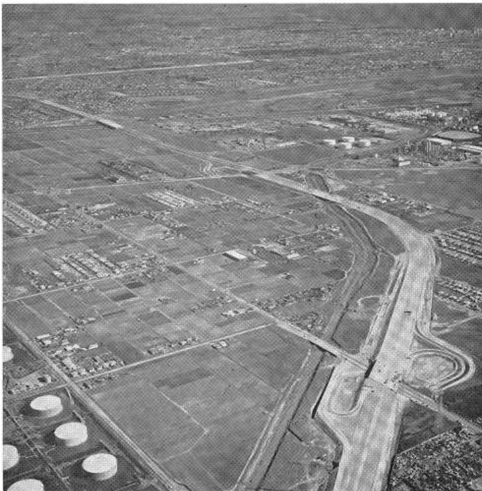
The San Diego Freeway with the Carson Street interchange in the foreground. The view is southward.
