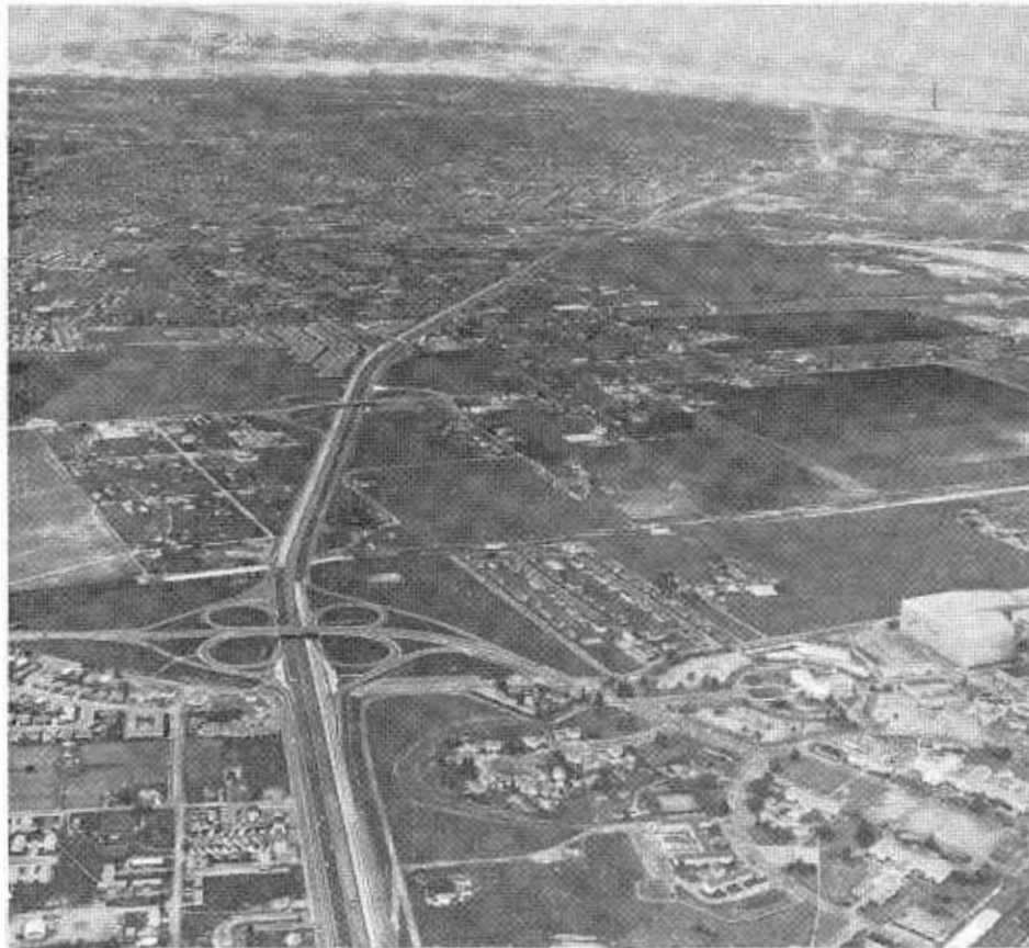
Bayshore Freeway looking northerly at a portion of the completed contract between Charleston Road and Morse Avenue. In the foreground is Moffett Field Interchange (not constructed in this contract).
