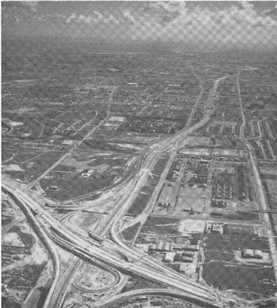
The San Diego-Harbor Freeway Interchange. The view is south along the Harbor Freeway.
