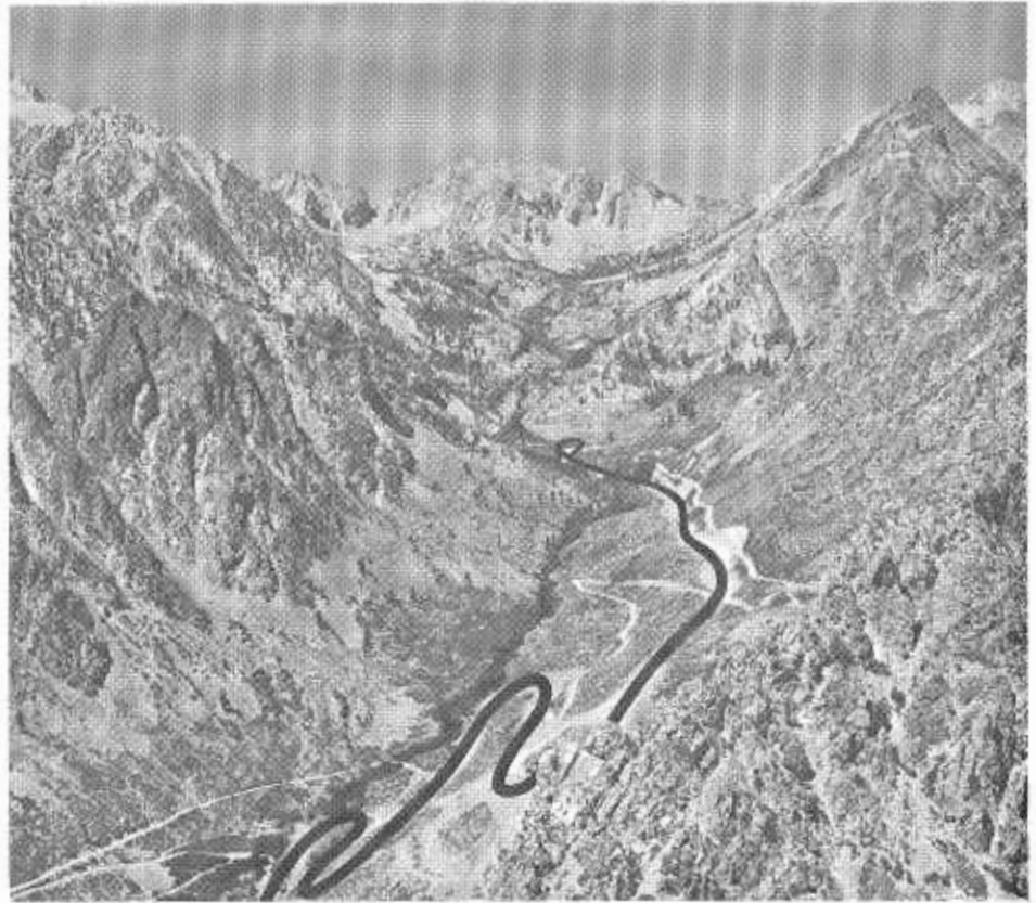
A view of F.A.S. Highway 1183 looking toward its western terminus in Onion Valley at the foot of the Kearsarge Pass Trail. Asphalt surfacing, not yet placed, has been delineated on the photo.
