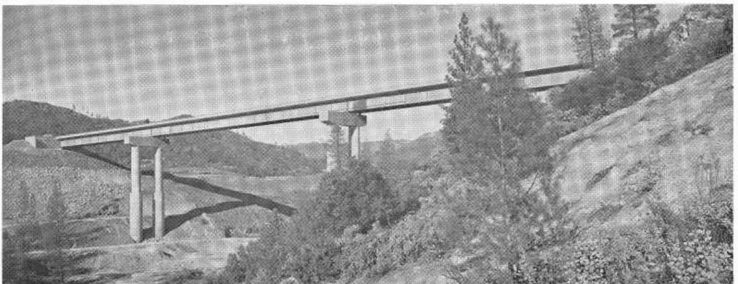
The new Whiskey Creek Bridge on the relocated section of U.S. 299 between Redding and Weaverville. The view is westward.
