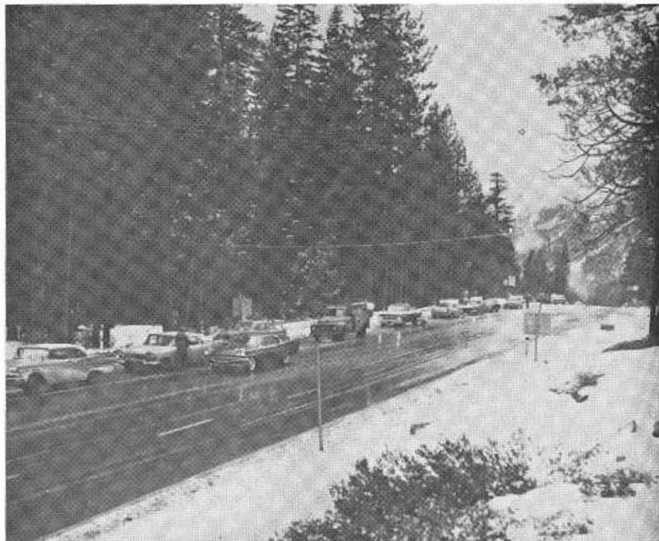
A portion of the Twin Bridges passing lanes being used as a chaining area for the climb over Echo Summit. The cars are headed east.
