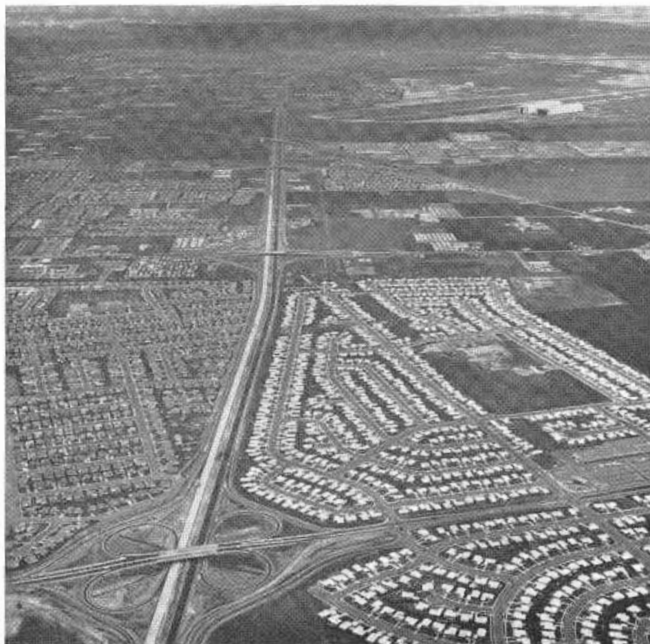
Lawrence Station Road Interchange on Bayshore Freeway between Morse Avenue and Brakaw Road, looking northerly. Beyond Fair Oaks Avenue Interchange in the center is the newly completed portion between Charleston Road and Morse Avenue.
