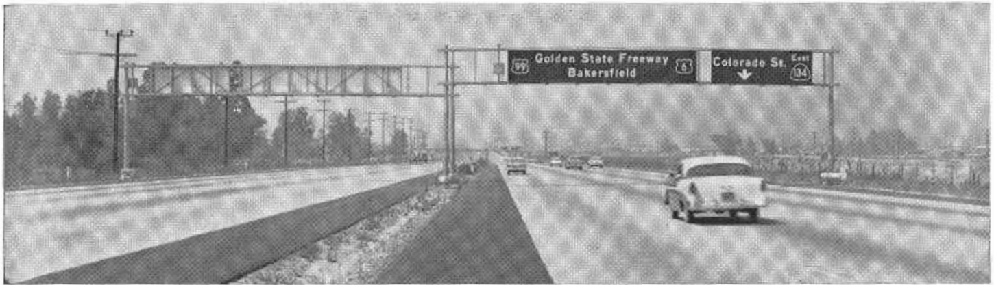
The Golden State Freeway in the Los Angeles area. This is an eight-lane freeway. The average daily traffic rate from 1957 to 1959 was 45,000. The accident rate for this period was 0.38 per million vehicle miles.
