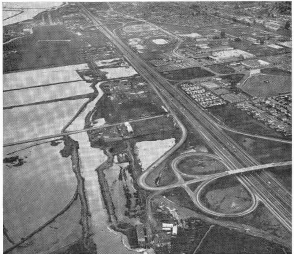
The Bayshore Freeway south of San Francisco. This is a six-lane freeway with an average daily traffic count of 59,400 vehicles and an accident rate of 0.75 per million vehicle miles.
