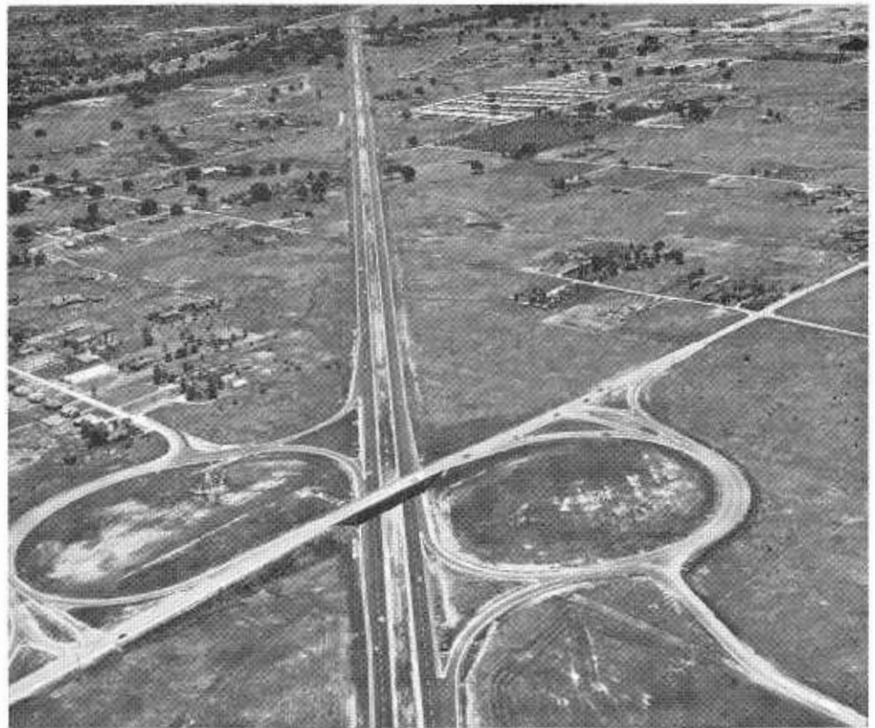
This section of the Roseville Freeway (US 40-99) north of Sacramento has an average daily traffic count of 22,200 and an accident rate of 0.51 per million vehicle miles.
