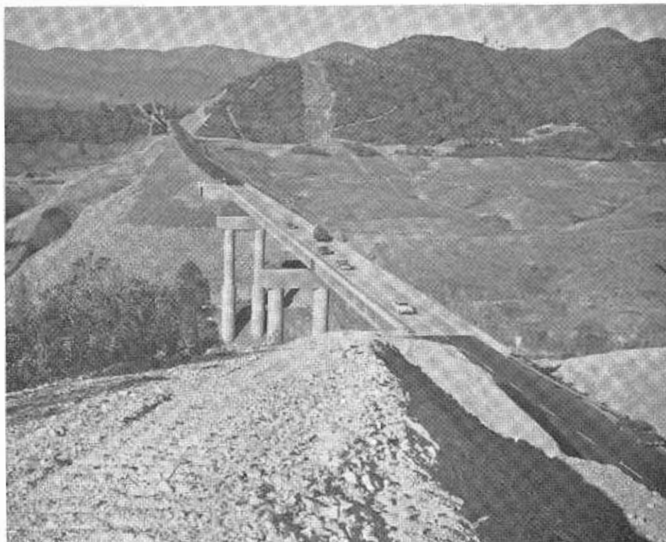
The new Whiskey Creek Bridge showing the completed roadway with provision for future expansion to four lanes.
