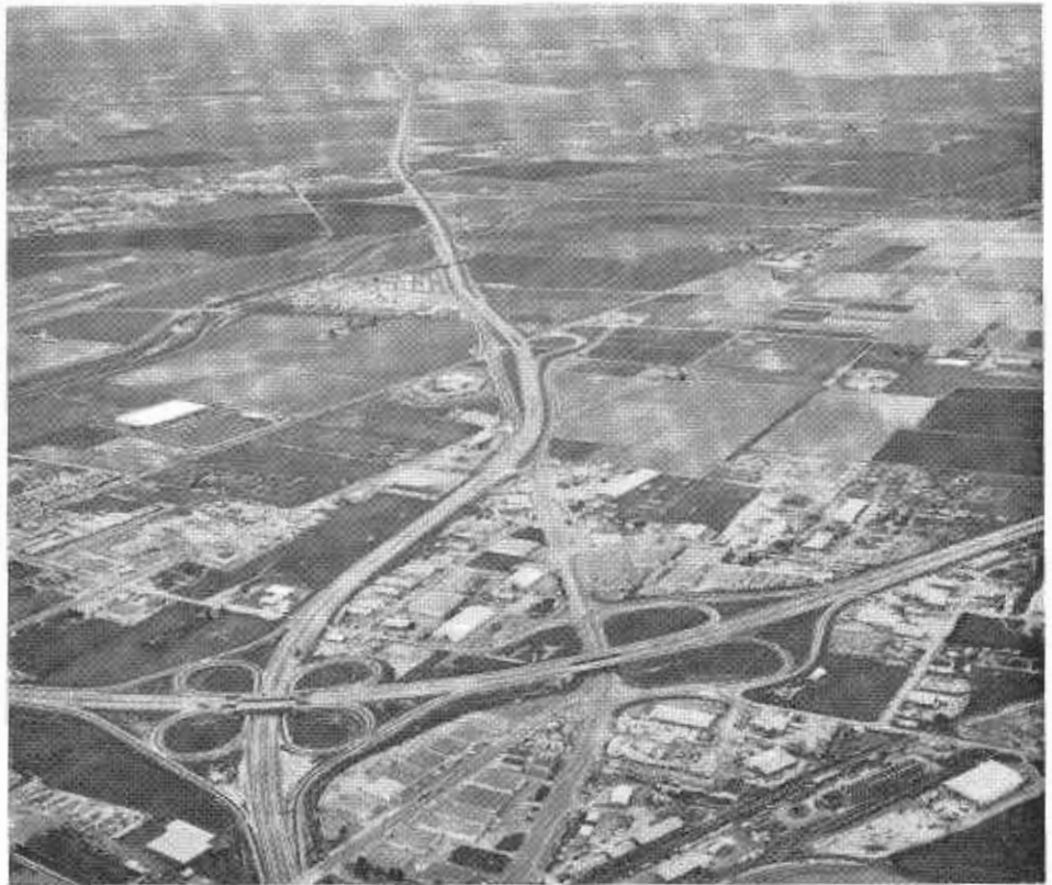
Looking northerly from Junction of Interstate 680 and US 101 Bypass at the newly completed portion of Bayshore Freeway between Morse Avenue and Brokaw Road. Guadalupe Parkway Overcrossing structure in center of photograph.
