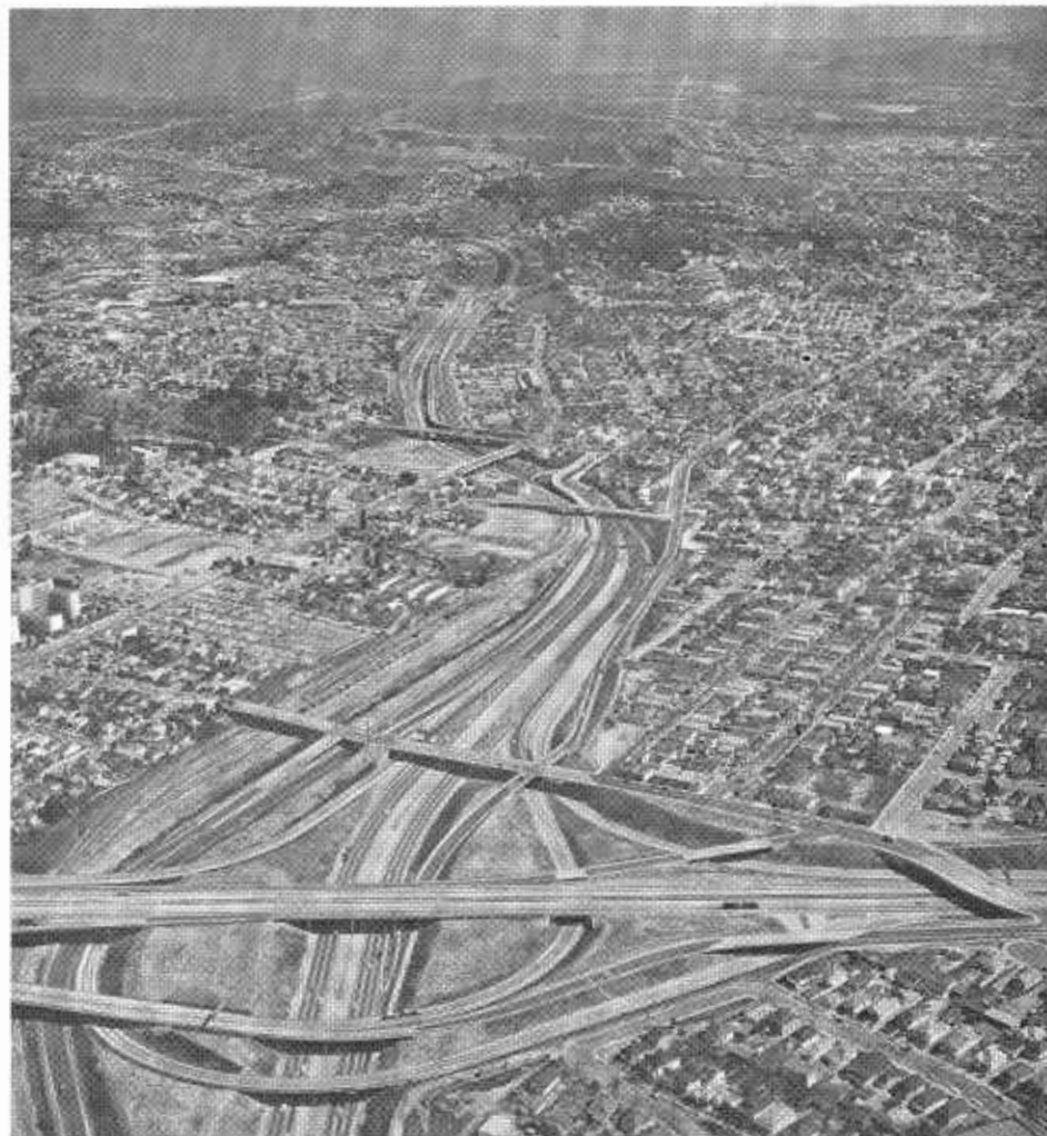
The San Bernardino-Golden State Interchange. The view is east along the San Bernardino Freeway.
