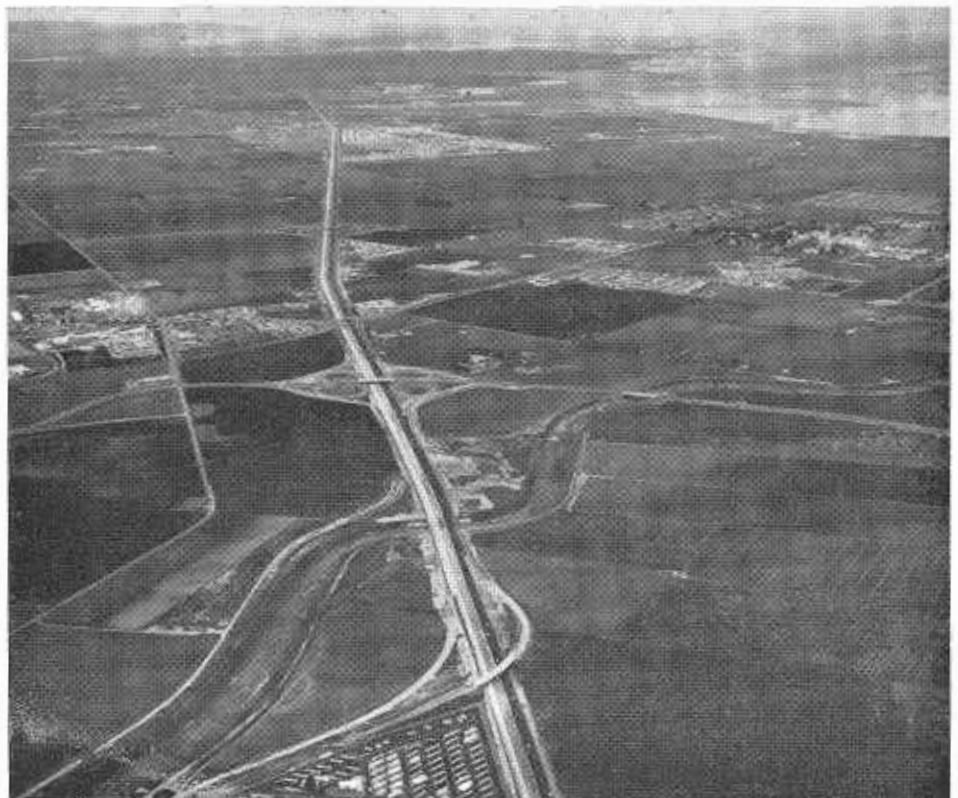
Bayshore Freeway between Morse Avenue and Brokaw Road, showing the structure for the future Guadalupe Parkway in the foreground and the four-quadrant cloverleaf at Trimble Road-De LaCruz Boulevard.
