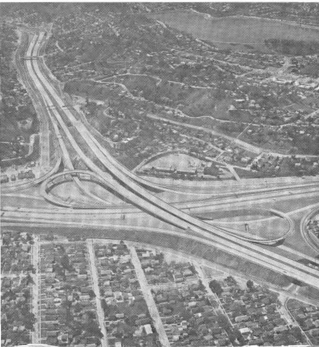
The completed Glendale Freeway, looking southwest to Glendale Boulevard. In the foreground is the Glendale-Golden State Freeway Interchange.
