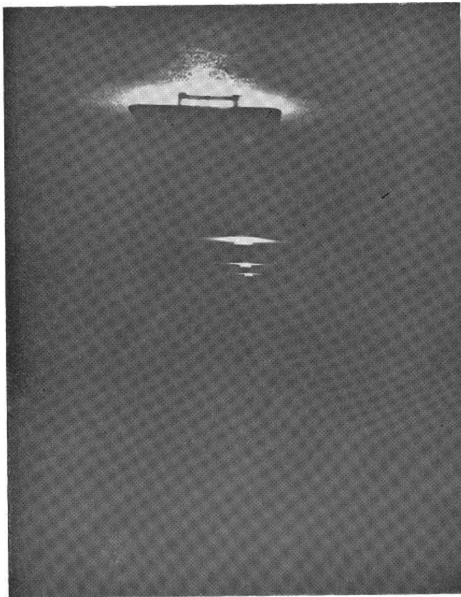
BEFORE—A night photo of lighting inside the Miner Avenue Pedestrian Undercrossing in Stockton prior to the experimental installation of the fluorescent fixtures.
