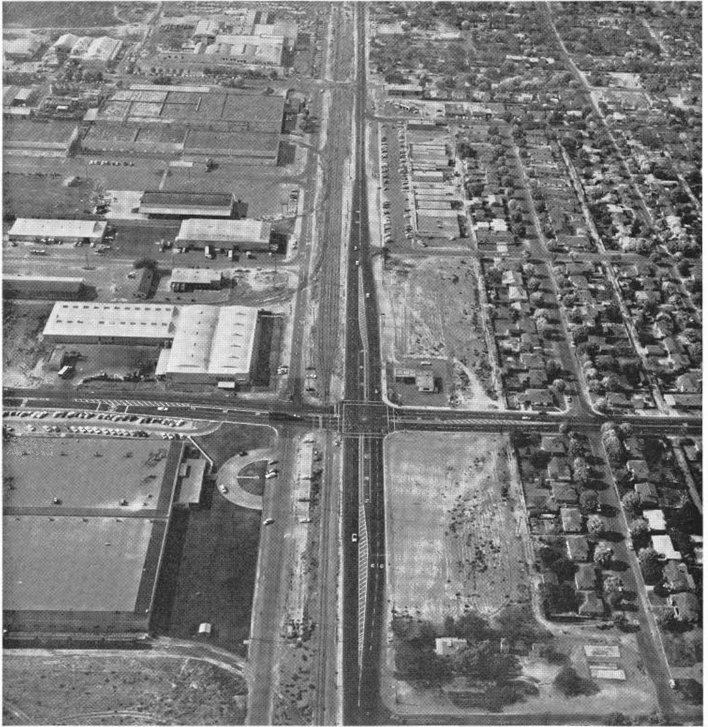
AFTER—The completed project looking west along Yosemite Boulevard (State Sign Route 132) toward the City of Modesto. (See photo previous page.)
