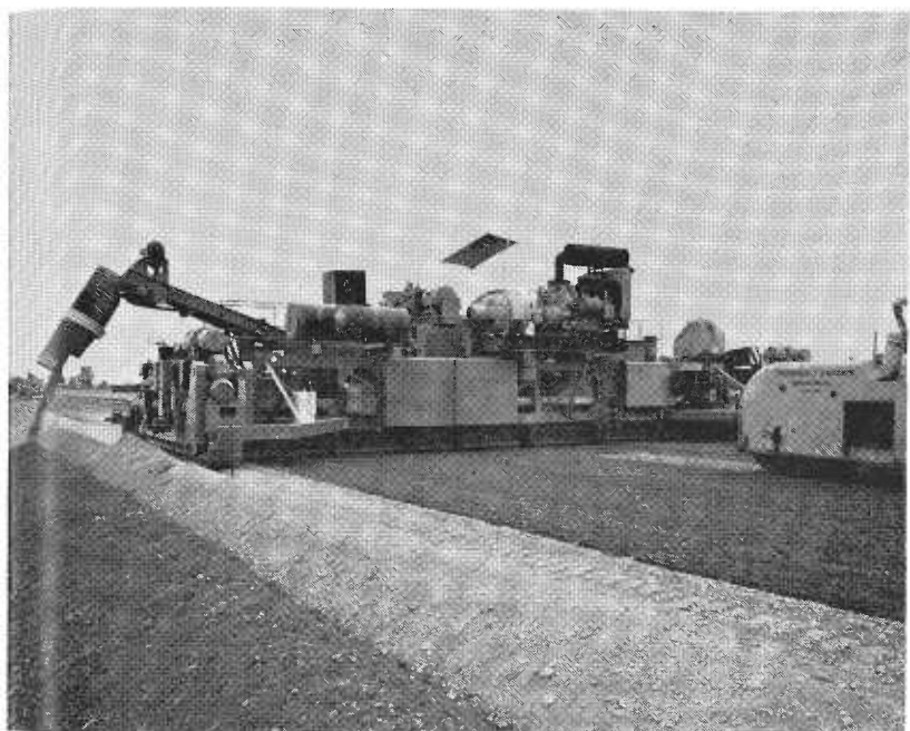
ABOVE—Rear view of the "Road Builder" trimming cement treated base. BELOW—Steel deck unit forms being prepared for concrete pour.
