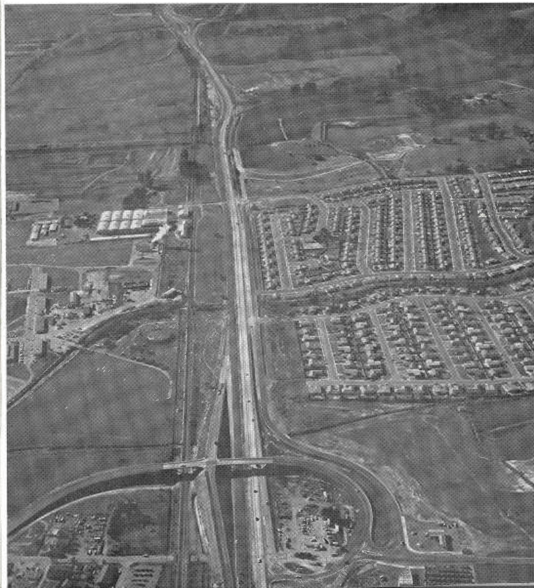
The Fairview overcrossing (center front) connects U.S. 101 with the University of California at Santa Barbara. The view is westward.
