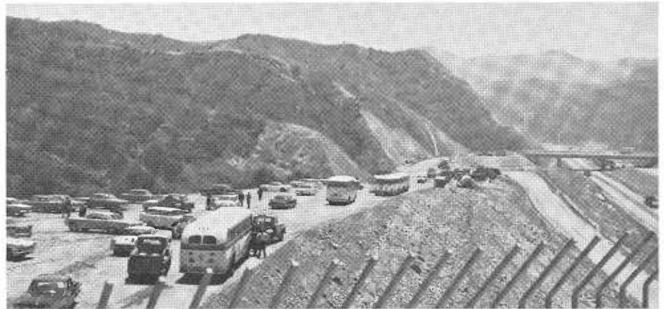
Below: Some of the buses and cars used to transport the tour participants. View is south in the cut area from Mulholland Drive Overcrossing. Bridge in middle distance is Rimerton Road Overcrossing.
