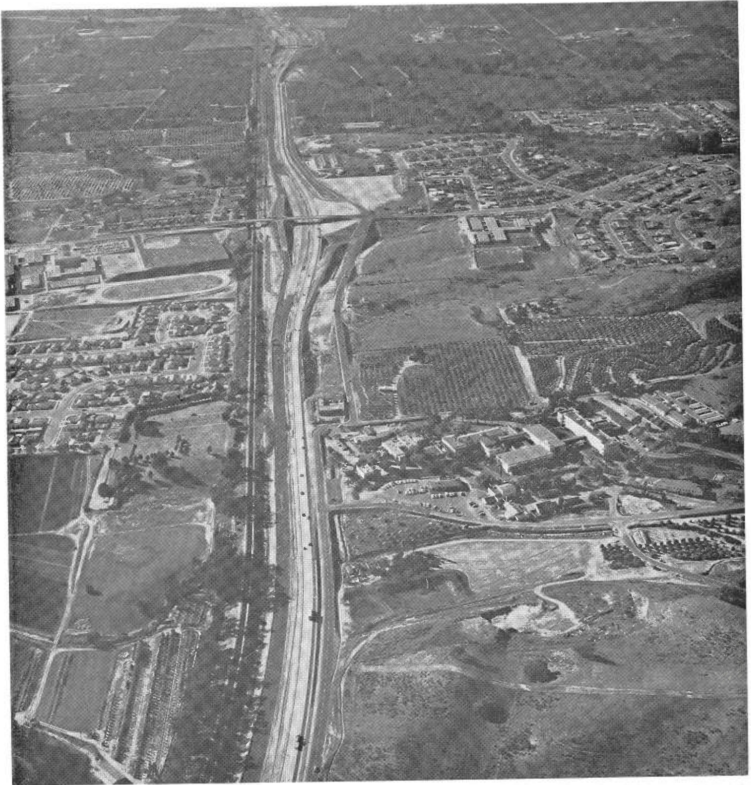
The Turnpike Road overcrossing passes over the freeway at the center of the photo with the San Marcos High School to the left of the overcrossing and the Cathedral Oaks Elementary School to the right. Group of buildings in the right foreground is the Santa Barbara County Hospital.
