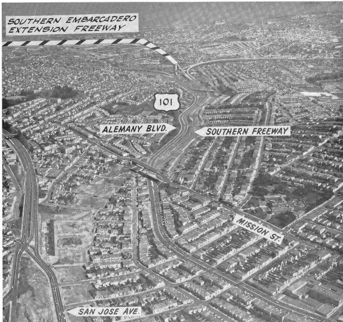
The Southern Freeway on US 101 in San Francisco. The future location of the Southern-Embarcadero Freeway extension is shown in the background. The portion between the James Lick-Southern Freeway Interchange and Mission Street is under construction and the right of way west of Mission Street has been cleared.
