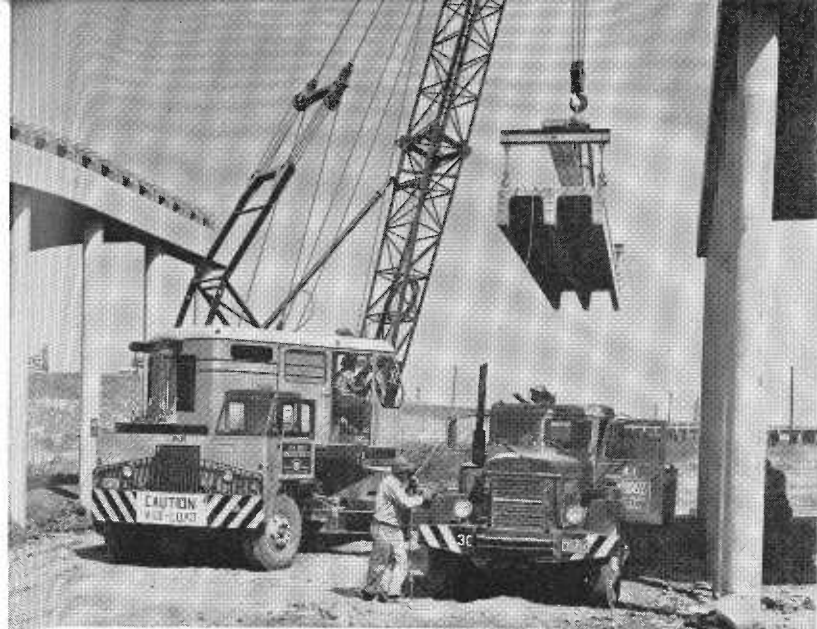
Erecting the deck units on the west Yolo Causeway.
