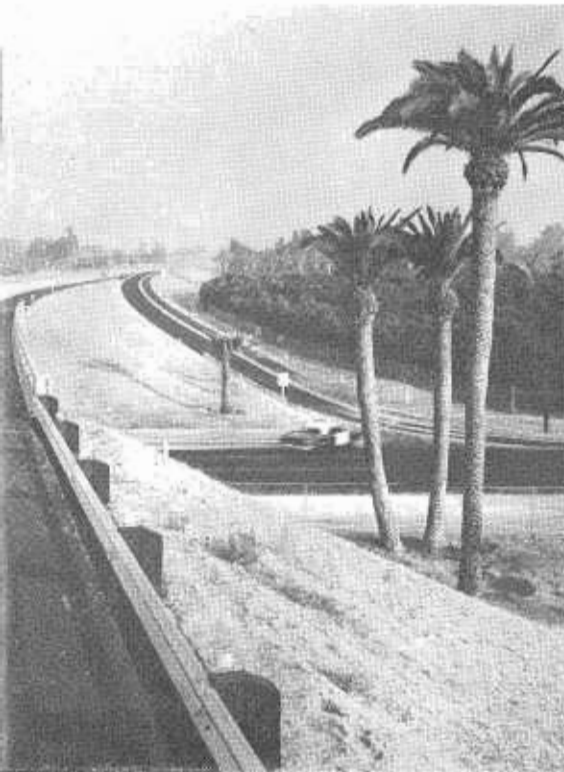
FRONT COVER—Part of the freeway through Redlands on U.S. 70-99 (Interstate 10) at the Cypress Avenue Undercrossing, completed in August 1962. The golden straw on the embankments provides erosion protection pending planting of trees, shrubs and periwinkles. The palm trees were transplanted to their present location (photo by Robert Dunn).
