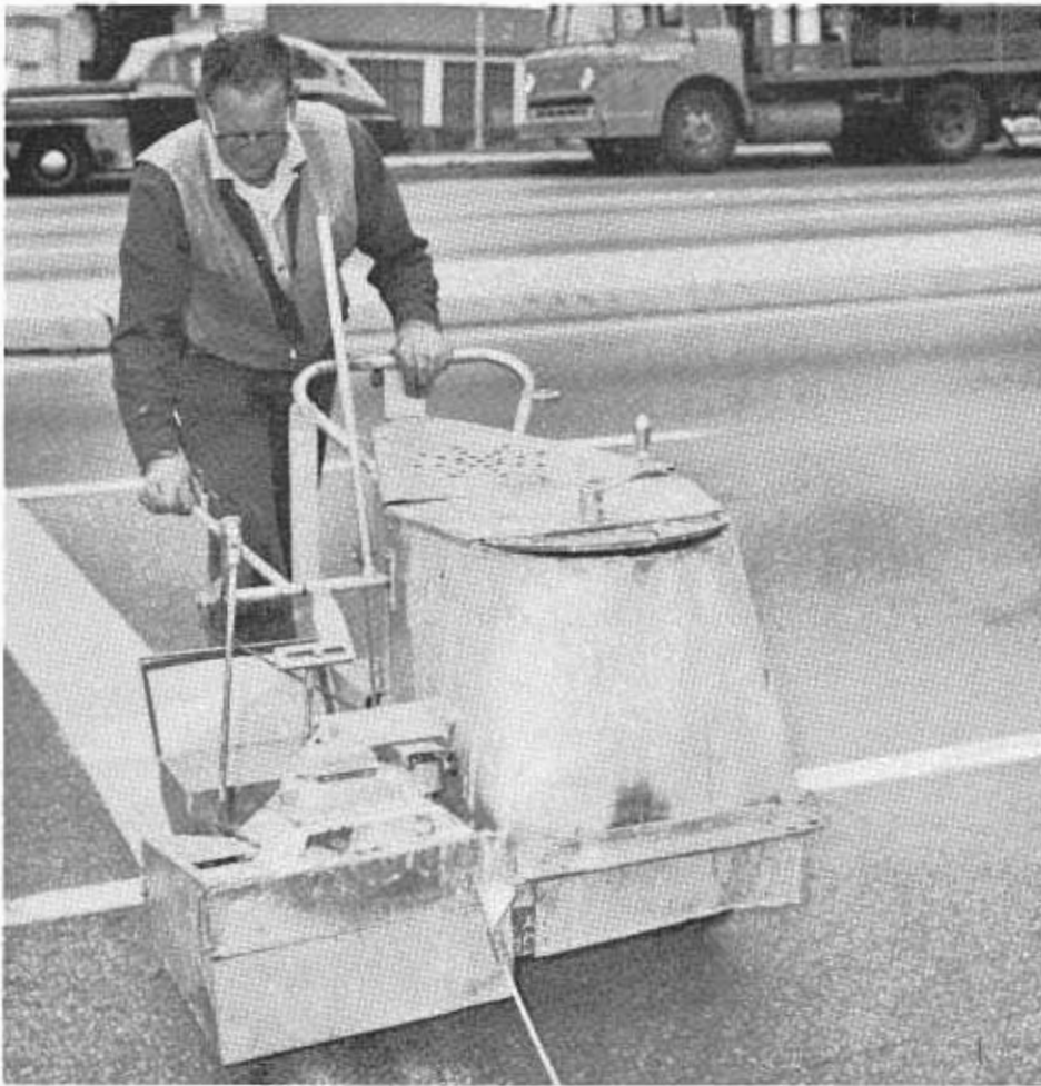
Thermoplastic striping unit placing crosswalk markings.
