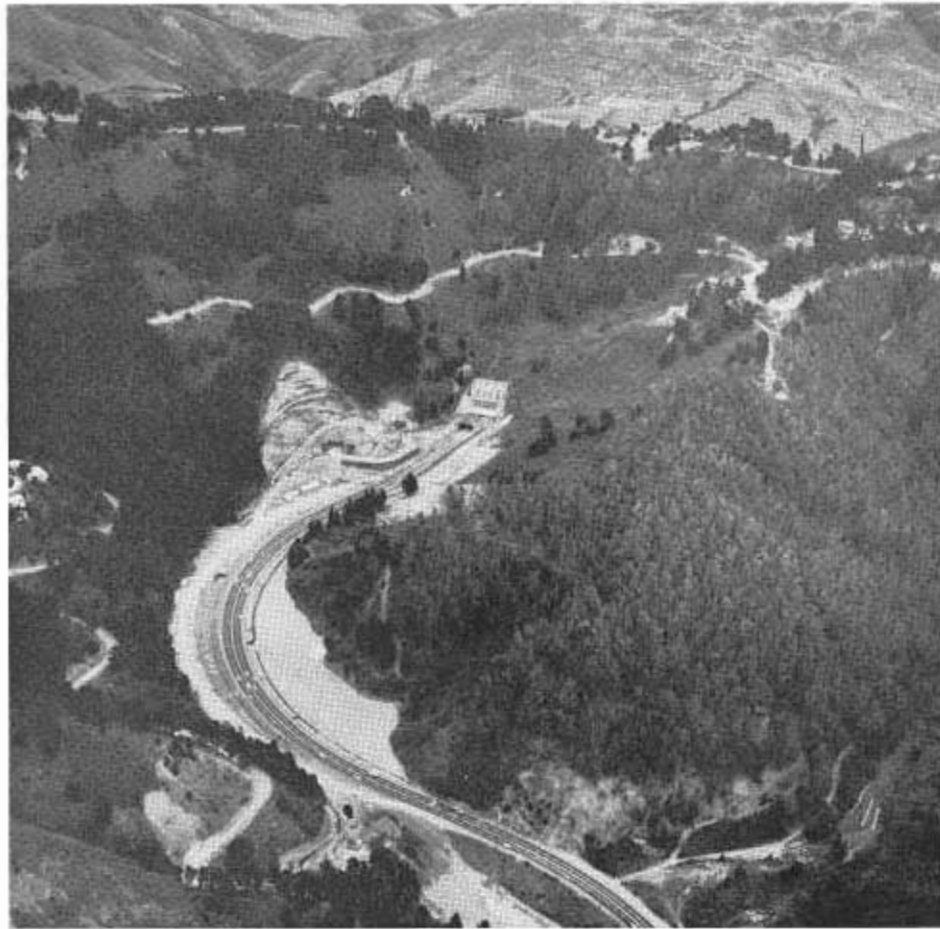
The west portal of the Caldecott Tunnel on Sign Route 24 east of Berkeley.
