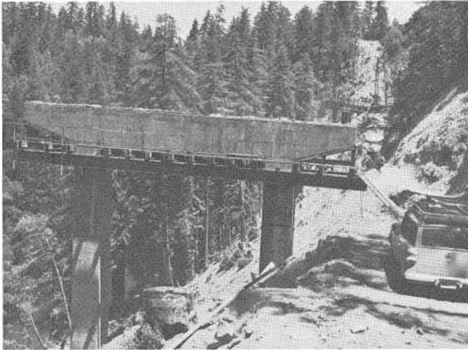
Illustrating some of the problems encountered in the construction of the Redwood Parks Freeway through rugged country is this view of the Eagle Point Viaduct in Humboldt County. This 16-span bridge structure will carry four freeway lanes on a 56-foot roadway for a quarter-mile.
