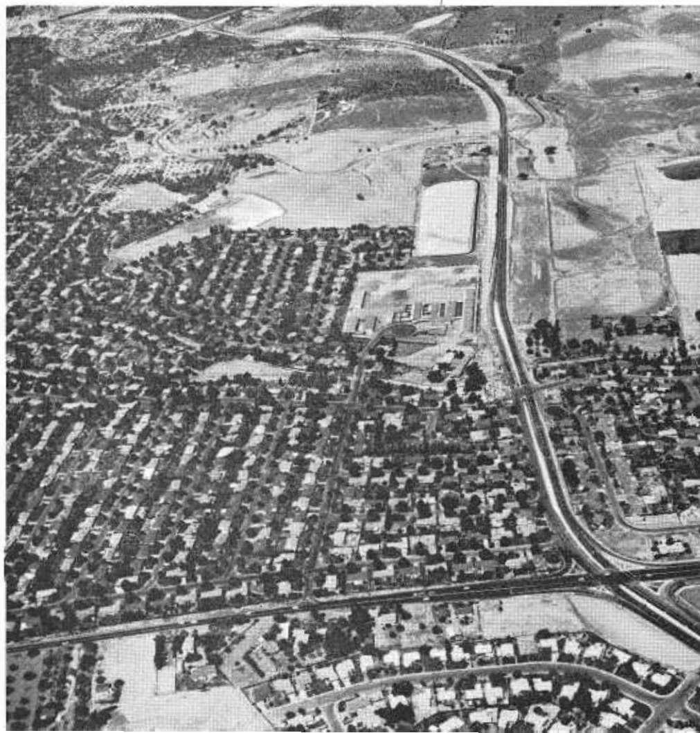
Taylor Boulevard, a new Contra Costa County freeway near Concord, constructed under the federal-aid secondary and F.A.S. urban extension programs.
