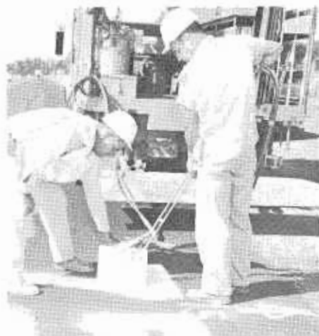
A mileage marker for aerial surveillance is painted on U.S. 40 near Davis.
