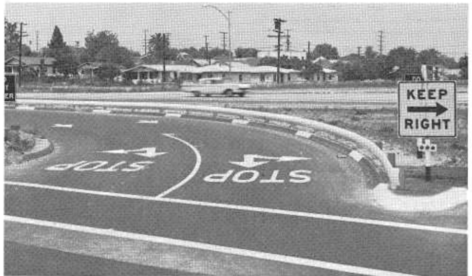
Restrictive pavement markings are painted at the ends of freeway offramps to prevent wrong-way entrances.
