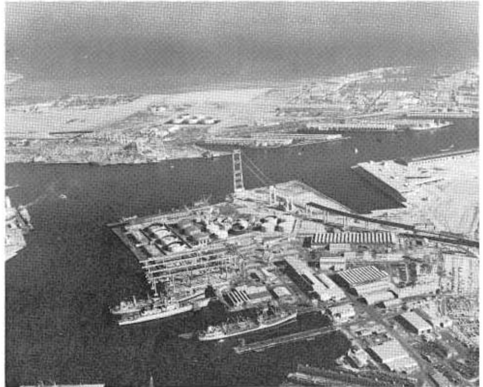
An aerial of the San Pedro-Terminal Island Bridge just after the stringing of the suspension cables over the towers began.
