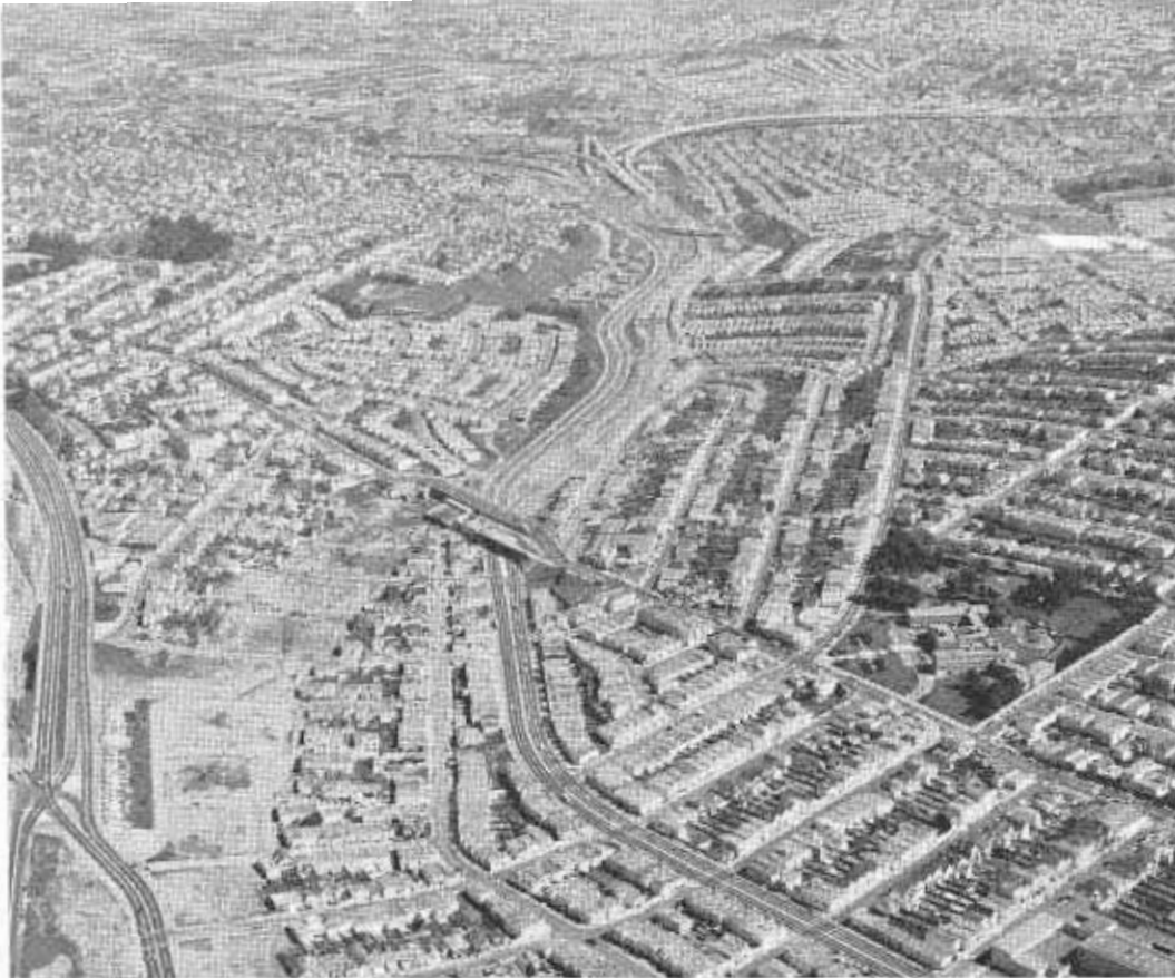
ABOVE —The Southern Freeway in San Francisco, which will roughly parallel Alemany Boulevard, is under construction from the James Lick Memorial (Bayshore) Freeway (upper center) to Orizaba Avenue. It will be continued by funds in the new budget to connect with the Junipero Serra Freeway (Interstate 280) in Daly City.
