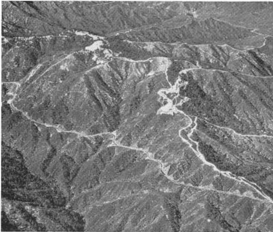
The road winding up the mountainside from left center is the recently completed Angeles Crest Highway in Los Angeles County. Barley Flat recreation area is off to right of photo. Higher level road is a former access road used during highway construction.
