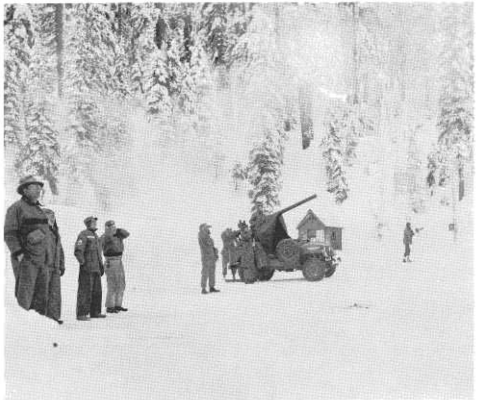
California National Guard shooting down snow cornices to prevent snow slides on U.S. 50 at Sierra Ski Ranch.
