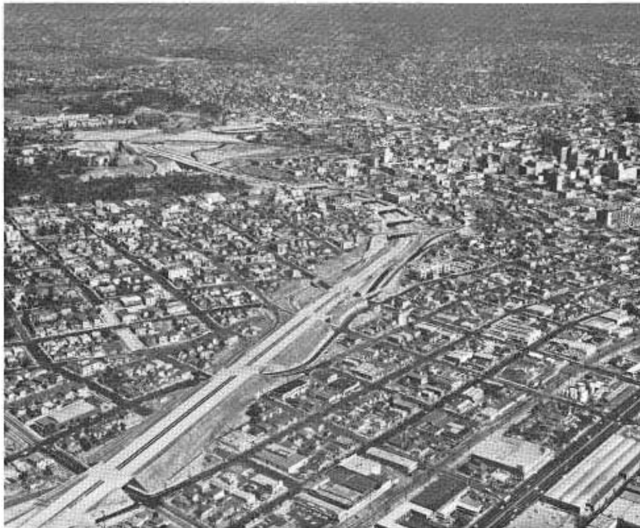
Shown above is a section of the Crosstown Freeway in San Diego which was opened to traffic in June. It turns left at center of photo to interchange with the Cabrillo Freeway (U.S. 395) at the south end of Balboa Park (left center). The Crosstown is a section of the San Diego Freeway which eventually will run from the San Fernando Valley in Los Angeles County to the Mexican border.
