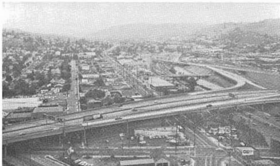
Part of the panorama from the Elysian Park view point in Los Angeles showing part of the viaduct (foreground).
