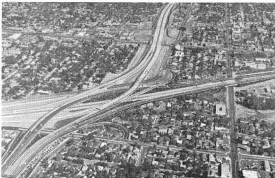
Looking east along the newly opened Ventura Freeway extension from above the interchange with the Hollywood Freeway in North Hollywood.
