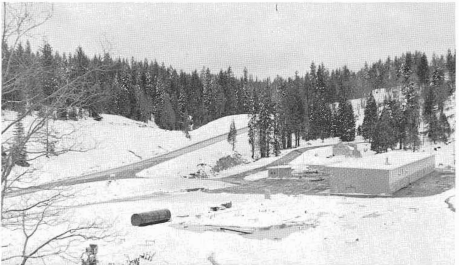
The new Whitmore Maintenance Station on U.S. 40 east of Baxter will facilitate maintenance work along this important stretch of trans-Sierra freeway.
