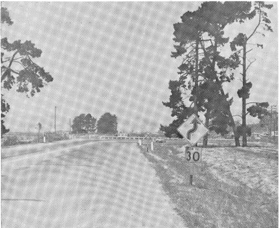
Looking north at the Alton Railroad Grade Crossing on the old highway. Note the poor alignment and sight distance.
