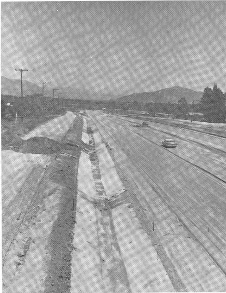
This drainage channel flanks the Sign Route 126 Freeway.
