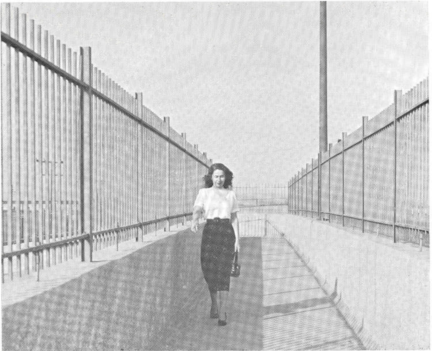
This railing was much better looking than the chain link fence but was too attractive to climb on, both inside and outside, and provided little interference to the rock and bottle droppers.
