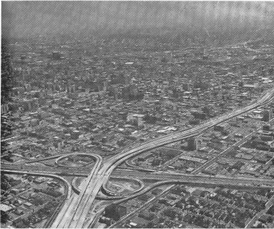
The Santa Monica-Harbor Freeway Interchange, a part of the Loop. The view is eastward. The section of the Santa Monica Freeway in the final stages of construction when this photo was taken (foreground) is now open to traffic as far as Vermont Avenue.
