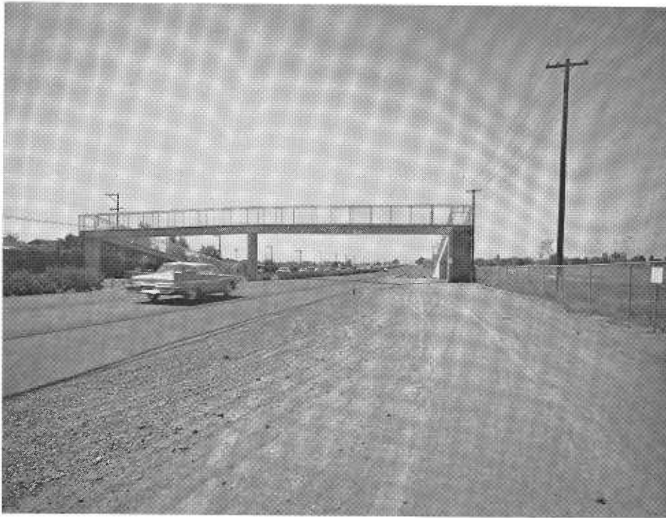
Completely enclosed, even on the ramps, this pedestrian structure near Sacramento looks very well protected. This apparently is regarded merely as a challenge by the children. The entire length of the roof of the cage across the freeway and down the ramps, is beaten down where countless children have crossed and bounced on the top of the cage instead of staying inside where they should be. (See photo below.)
