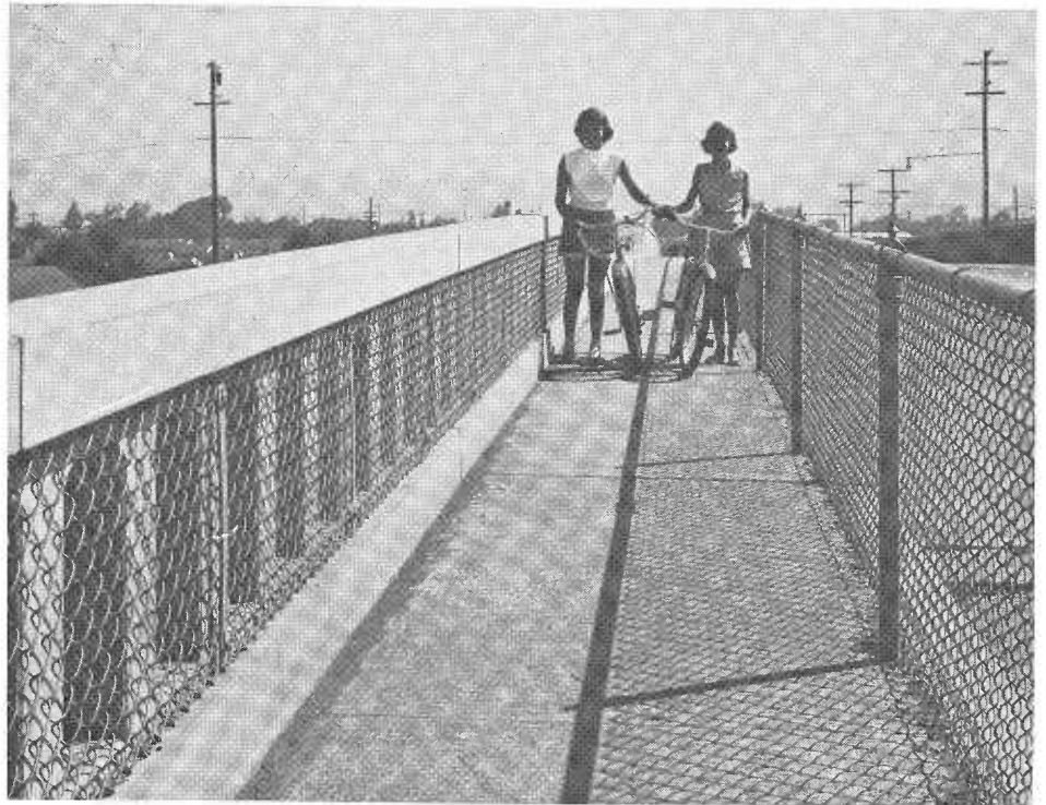
Here the concrete railing has been faced with a chain link fence so children cannot climb out through the windows and an additional fence has been placed on the edge of the sidewalk to keep them from jumping out into the street.
