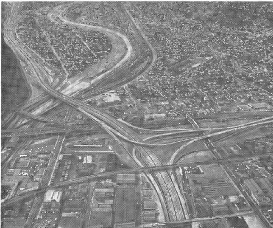
Looking north along the Golden State Freeway section of the Loop. In the foreground is the Elysian Viaduct and Pasadena Freeway Interchange.
