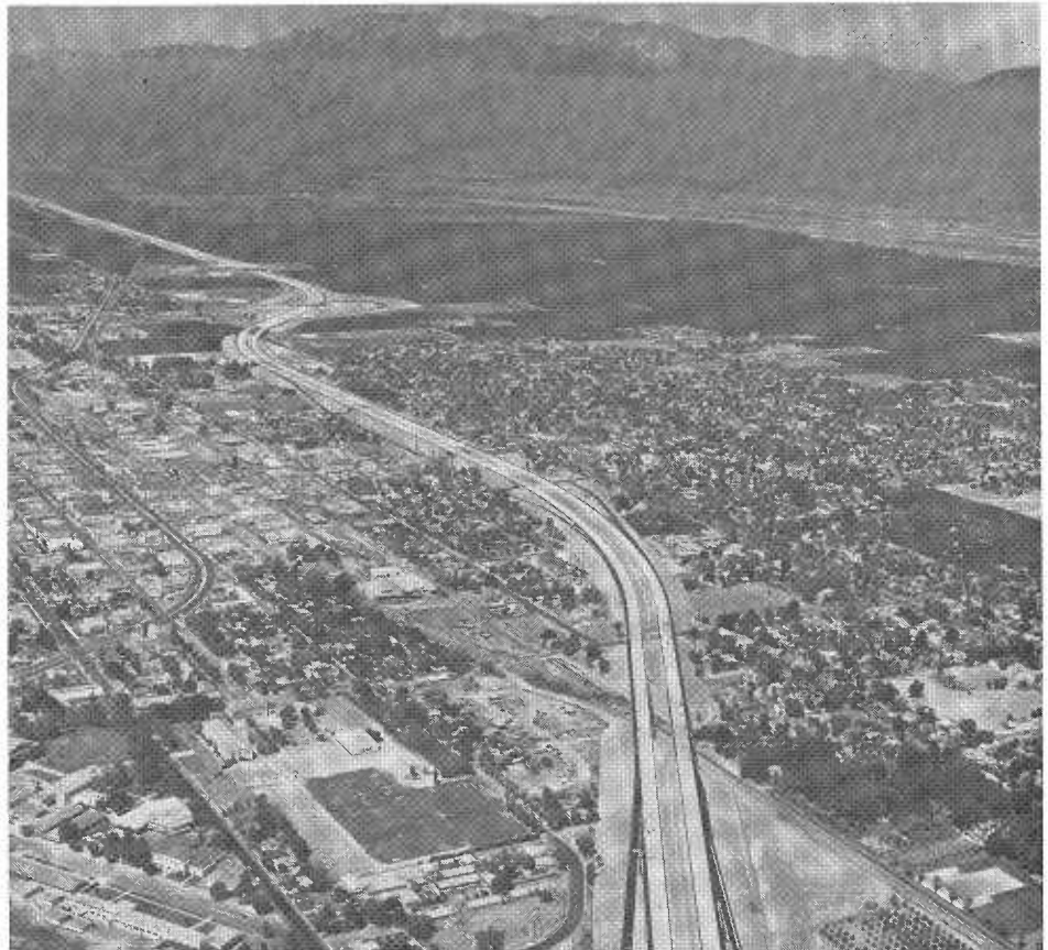
This aerial, looking northwest from above the University Street undercrossing, shows the completed freeway through Redlands and the San Bernardino Valley in the distance. The old four-lane highway is to the left.
