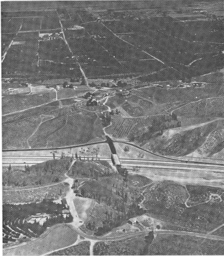
Looking north over the Wabash Avenue Interchange. The new freeway in this section (left to right) follows the general alignment of Reservoir Canyon.
