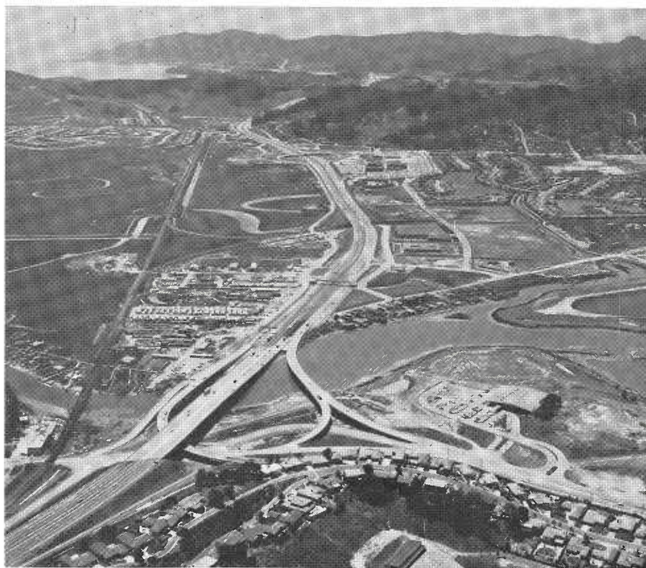
PRIMARY—US 101, the Redwood Highway, in Marin County is on the Federal-Aid Primary System. This view is looking south across the Greenbrae Interchange and Corte Madera Creek.
