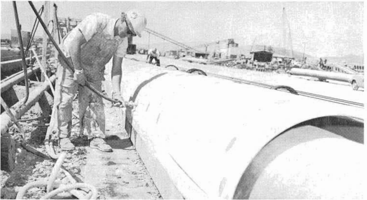
CONCRETE PILE CURING showing cover for initial heat curing.
