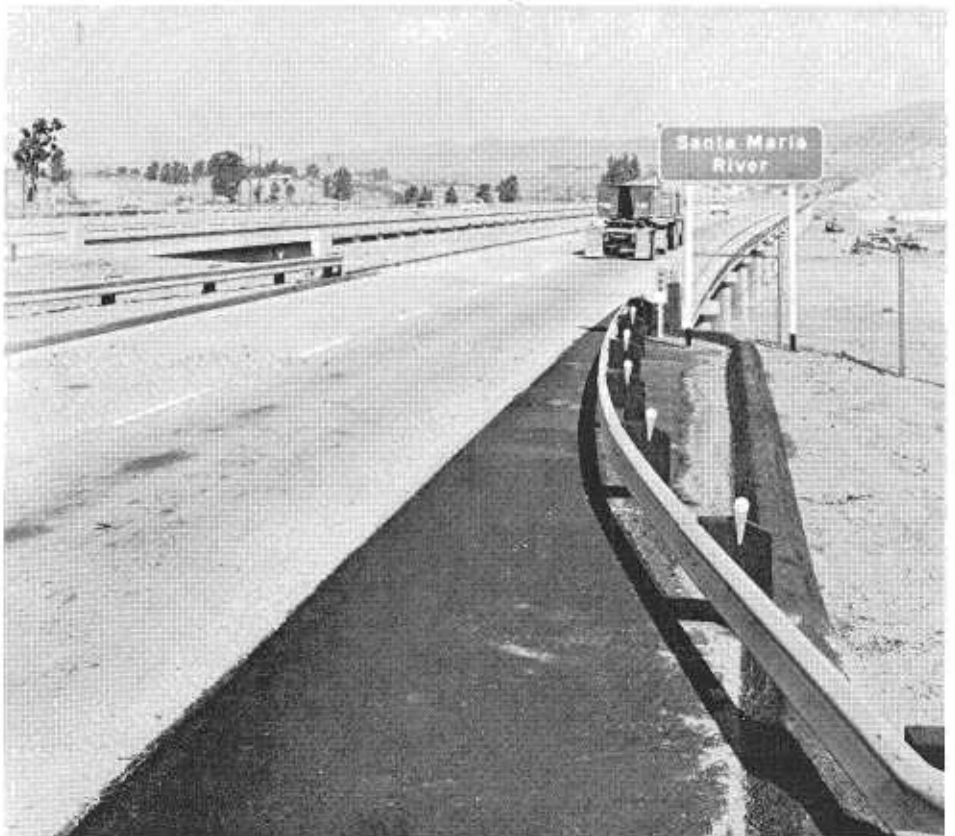
AFTER. These twin bridges now carry traffic on the new freeway across the Santa Maria River channel.
