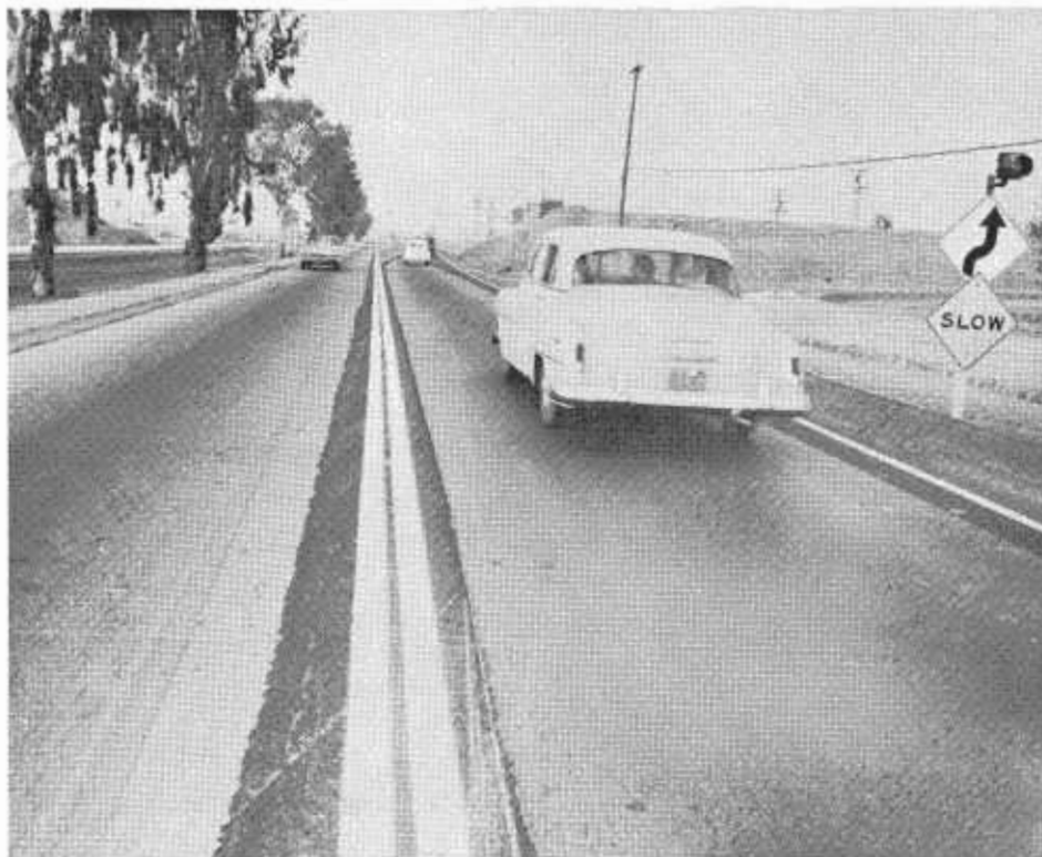
This photo shows temporary "no passing" pad down the center of the roadway.
