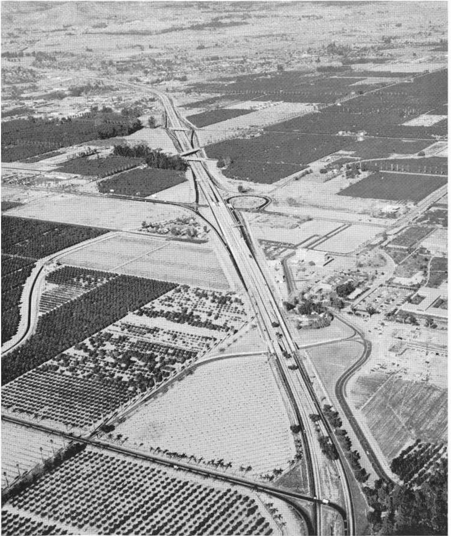
Looking northwest along the new alignment of U.S. Highway 60 from the University of California (right foreground) at the east city limits of Riverside, showing the Eighth Street Undercrossing, Linden Street, Iowa Avenue, and Blaine Street Overcrossings.
