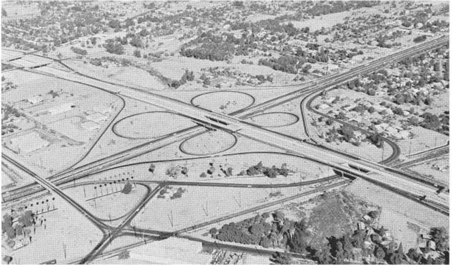
The U.S. Highway 60/395 Interchange with the Main Street and Orange Street Overcrossings at the extreme left and the Down Street Overhead at the right. Many of the transplanted palm trees are visible in the contour-graded areas.
