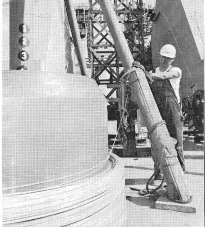
PHOTO ABOVE. The picture shows a single wire being reeled from a swift to one of the top sheaves of the floating sheave tower. PHOTO BELOW. Looking east from near the top of the Terminal Island tower, several of the 19 strands have been spun. The 19 strands will be squeezed into one compact cable 13 3/4 inches in diameter, then after full dead load from the supported roadway below has been imposed the cables will be tightly wrapped with galvanized wire and painted.
