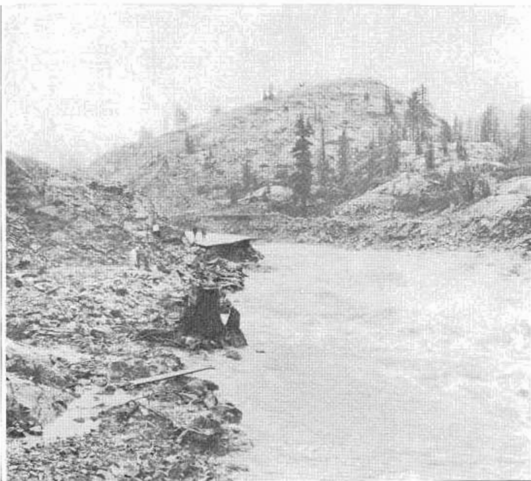
Above: Slipout on eastbound lanes, U.S. 40/Interstate 80 at Whitmore Maintenance Station, at about 5,000 feet altitude. Blue Canyon, a few miles east, recorded 16 inches of rain in 3 days. Below: Waters of Yuba River south fork near Cisco here partly receded after having savagely torn out several hundred yards of paving, subpaving, and fill on U.S. 40.
