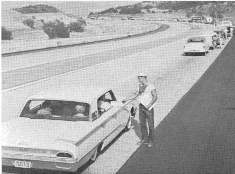
PHOTO ABOVE. During the earlier construction phases of the project flagmen handed out leaflets explaining the reasons for traffic delays ahead. BELOW. View of completed roadway. Note concrete lined ditches above cuts to prevent erosion.
