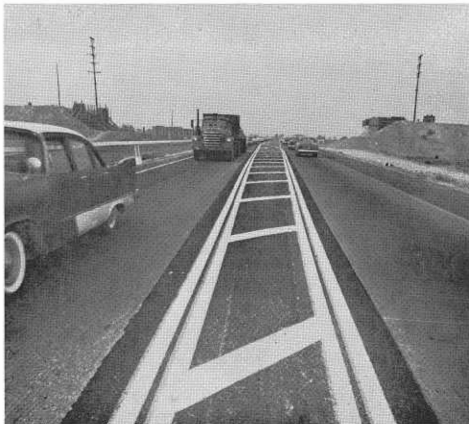
Channelized intersection delineation on asphalt concrete overlay.
