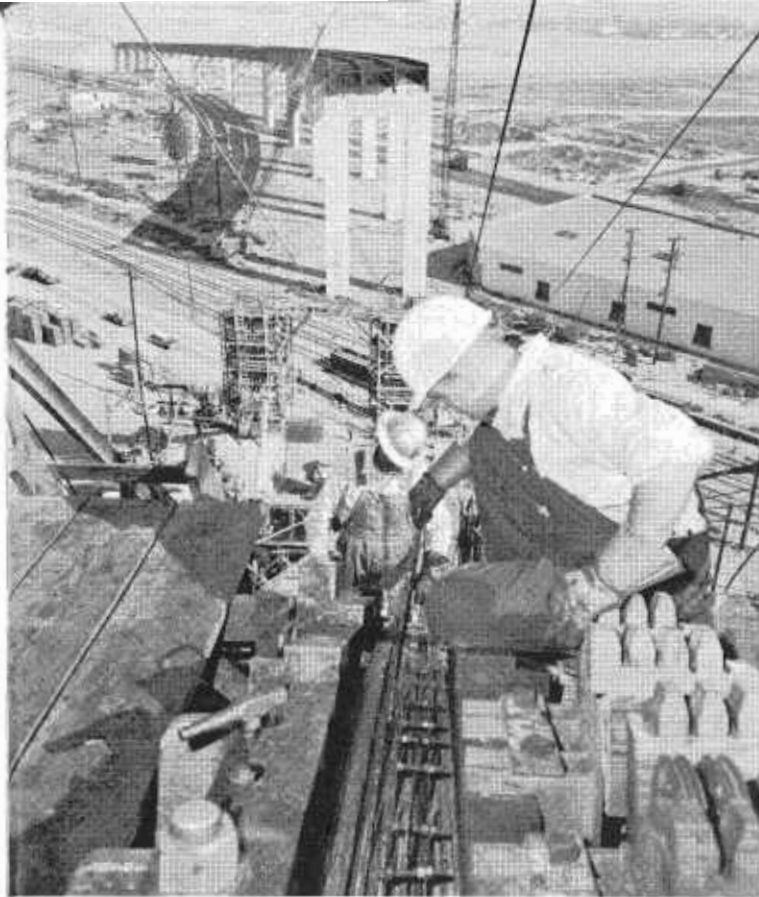
PHOTO ABOVE. Looking east from the top of the Terminal Island cable bent. After the wires are pulled along the bridge from anchorage to anchorage, they are tested for sag from the guide wire and then positioned one by one in the large steel tower shoes. PHOTO BELOW. This picture, taken at the Terminal Island anchorage, shows the splay of the cable strands from the splay casting at the top of anchorage to the circular strand shoes at the bottom. This portion of anchorage will be boxed in with concrete.
