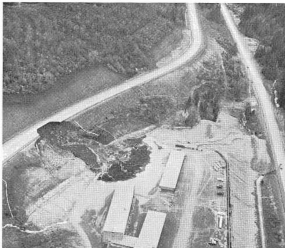
Above: Slipout on eastbound lanes, U.S. 40/Interstate 80 at Whitmore Maintenance Station, at about 5,000 feet altitude. Blue Canyon, a few miles east, recorded 16 inches of rain in 3 days. Below: Waters of Yuba River south fork near Cisco here partly receded after having savagely torn out several hundred yards of paving, subpaving, and fill on U.S. 40.
