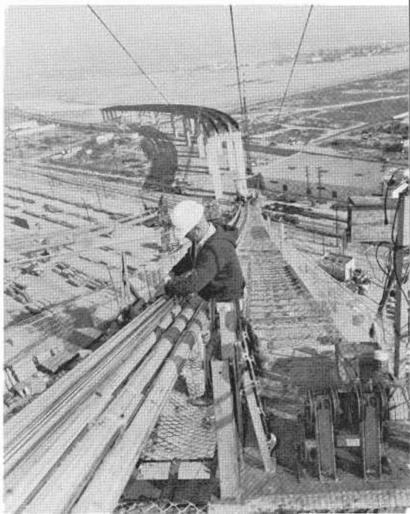
PHOTO ABOVE. The picture shows a single wire being reeled from a swift to one of the top sheaves of the floating sheave tower. PHOTO BELOW. Looking east from near the top of the Terminal Island tower, several of the 19 strands have been spun. The 19 strands will be squeezed into one compact cable 13 3/4 inches in diameter, then after full dead load from the supported roadway below has been imposed the cables will be tightly wrapped with galvanized wire and painted.
