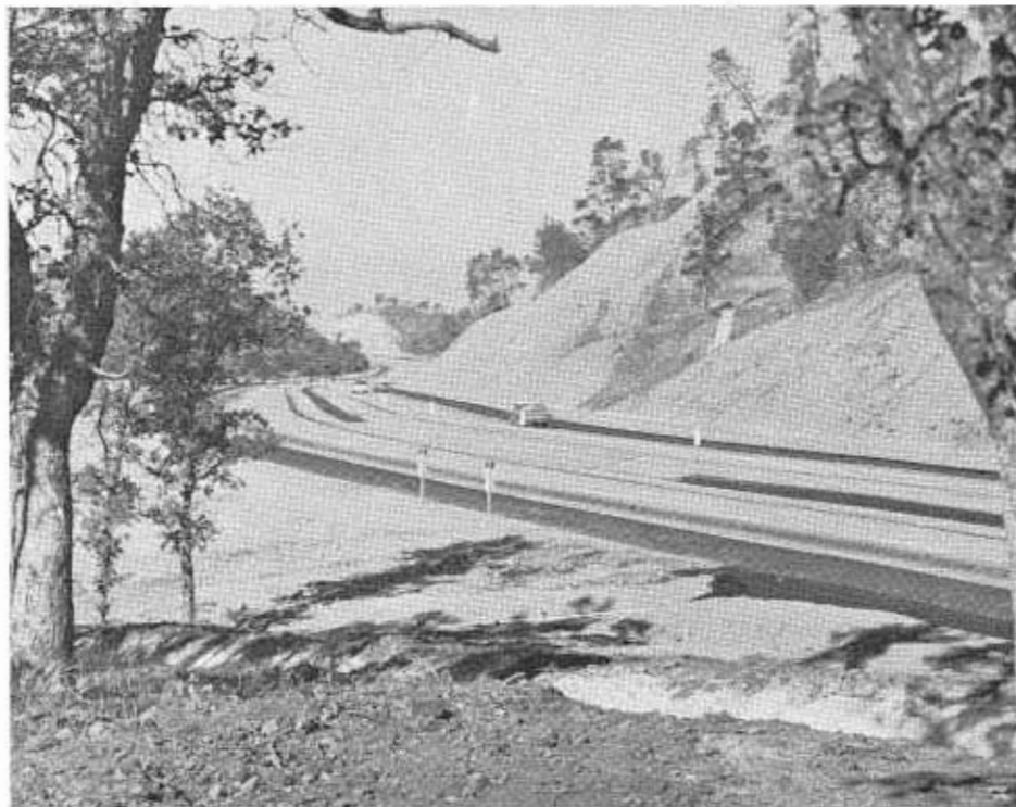
PHOTO ABOVE. During the earlier construction phases of the project flagmen handed out leaflets explaining the reasons for traffic delays ahead. BELOW. View of completed roadway. Note concrete lined ditches above cuts to prevent erosion.
