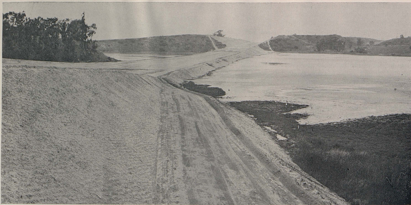
The settlement fill across Batiqitos Lagoon, strut in the right foreground.
