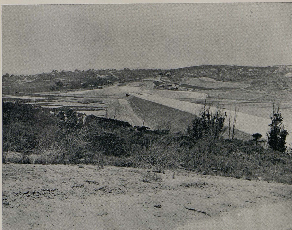
Another view of the fill at the San Elijo Lagoon showing the strut to the left.
