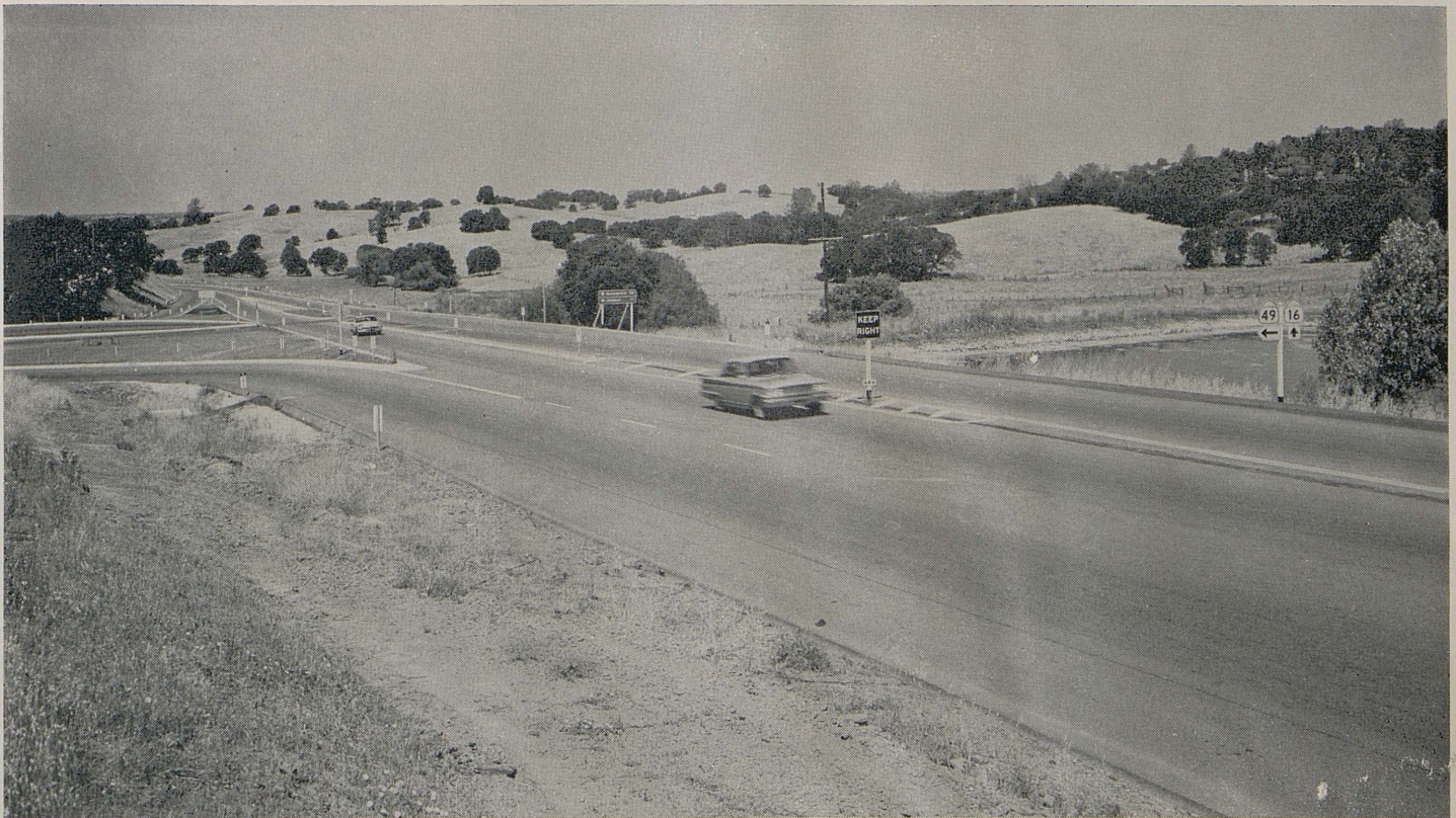
The highway has been made safer by channelization and widening of once hazardous intersections. This is the intersection of Sign Routes 49 and 16 north of Drytown, Amador County.
