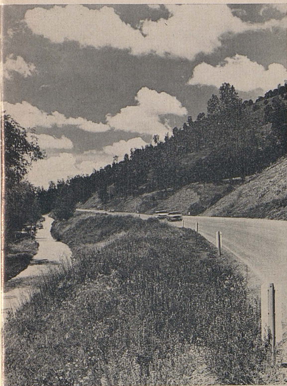
FRONT COVER: When a section of Sign Route 49 (Mother Lode Highway) near Jacksonville, south of Sonora, was realigned and constructed to modern standards in 1957 a portion of the old highway was left in place to serve local property owners. In the spring, with wild flowers in bloom, it offers a particularly inviting rest or picnic stop. Entrance is available to southbound traffic only. Photo by Bill Ruland.
