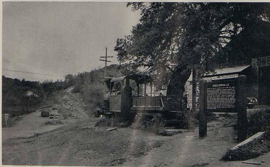
An ancient locomotive once used in the Mary Harrison mine seems to have a pensive regard for evidence of more modern transportation as it overlooks construction for relocation of Sign Route 49 near Coulterville.
