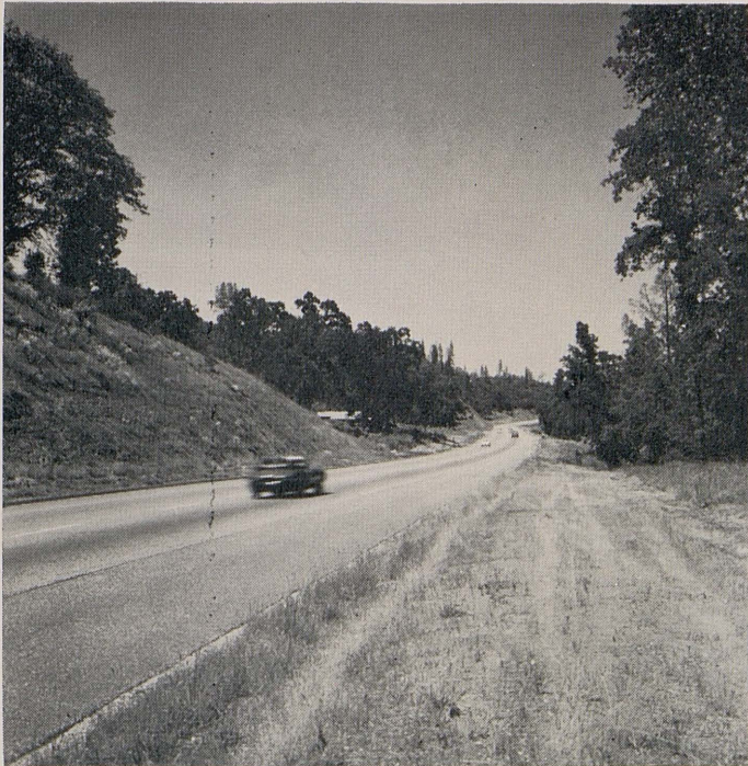
A section of modern two-lane expressway speeds the traveler between Auburn and Grass Valley.
