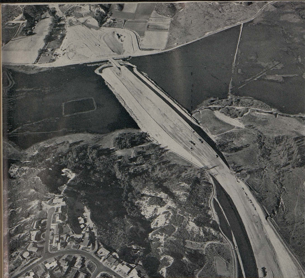
ABOVE PHOTO. Aerial of the San Elijo Lagoon showing the surcharge fill and struts looking north. BELOW. Another aerial of the San Elijo Lagoon fill taken higher up and looking south along the coastline.
