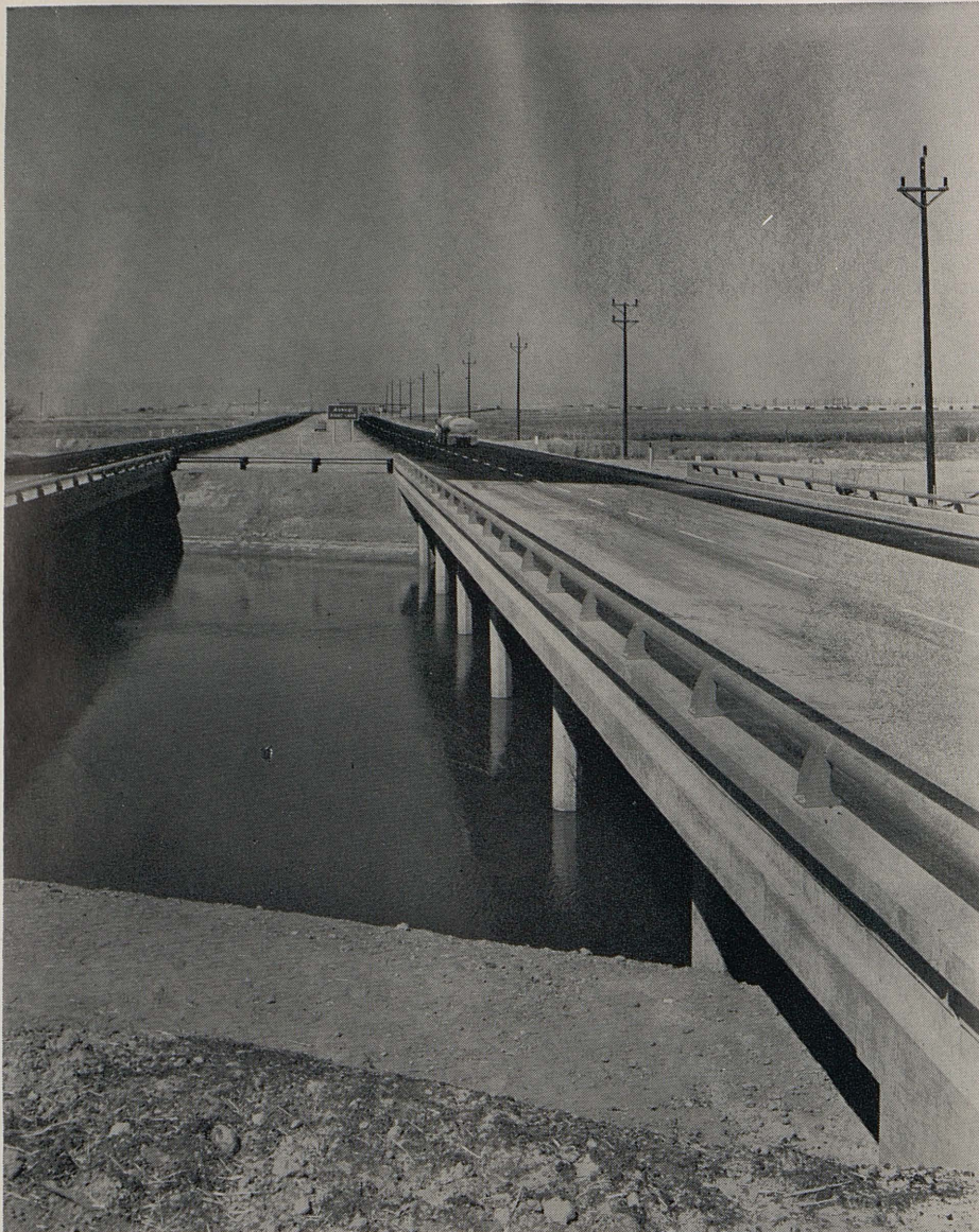
The twin bridges across the Kings River looking west.
