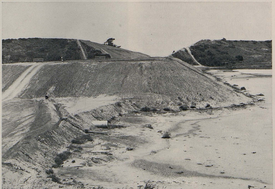
The north bridge cone embankment at Batiquitos Lagoon.
