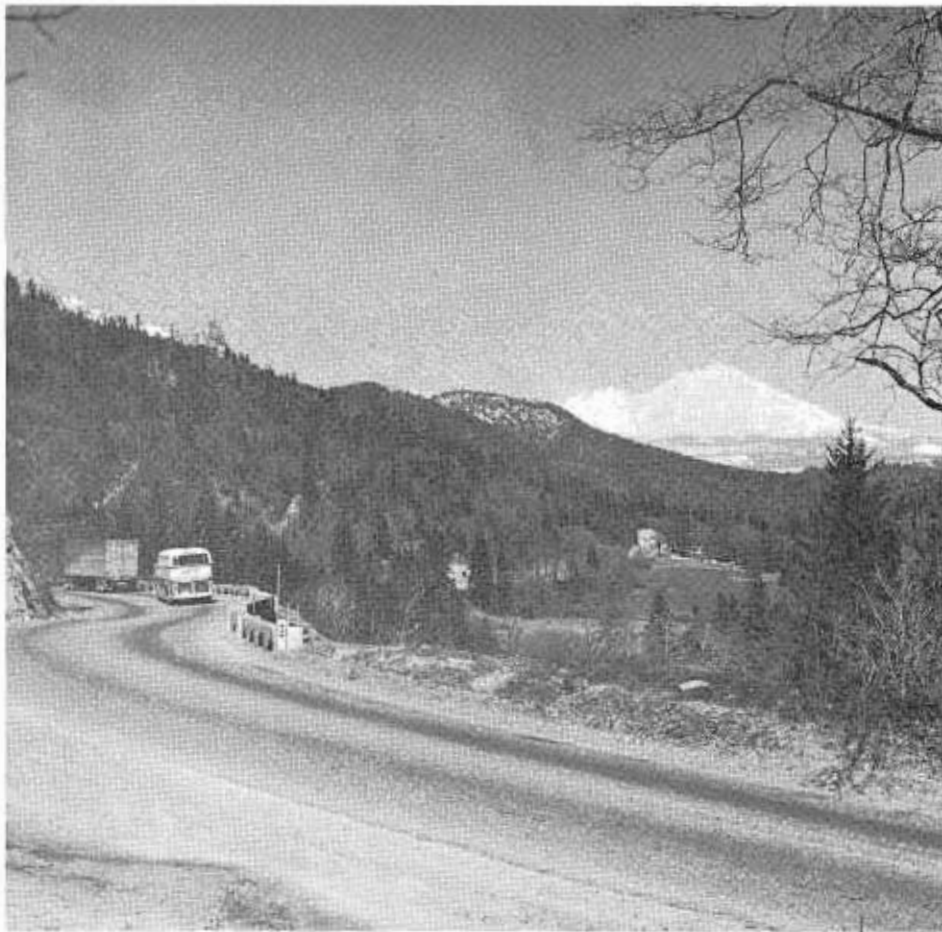
BEFORE. Section of old highway near Sweetbrier. Mount Shasta in background. Note retaining walls on right to prevent encroachment on railroad.
