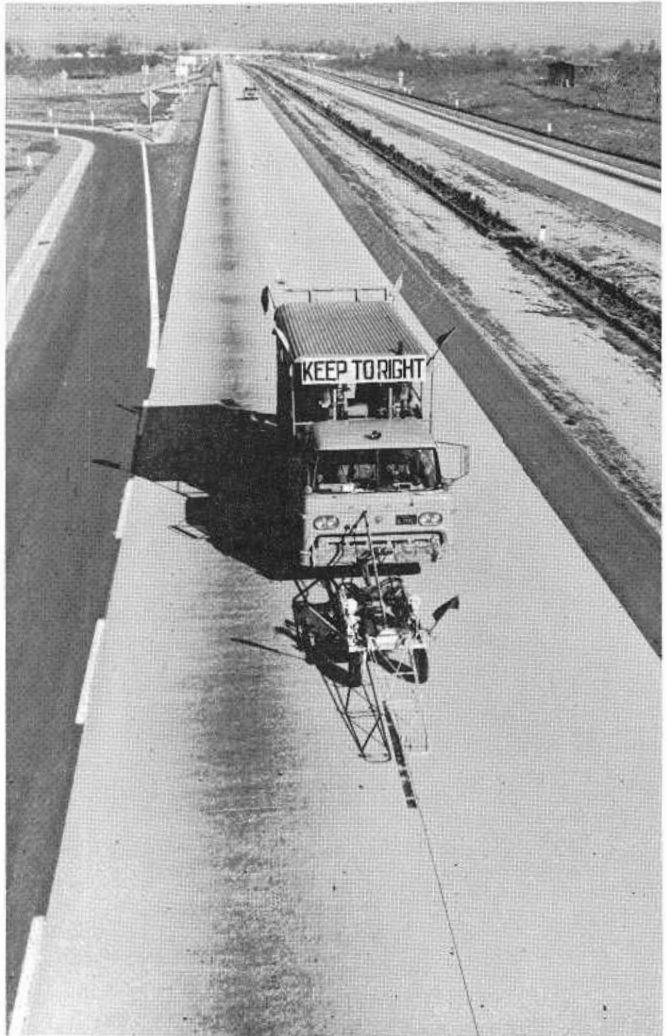
New unit in operation on U.S. 40 east of Roseville.
