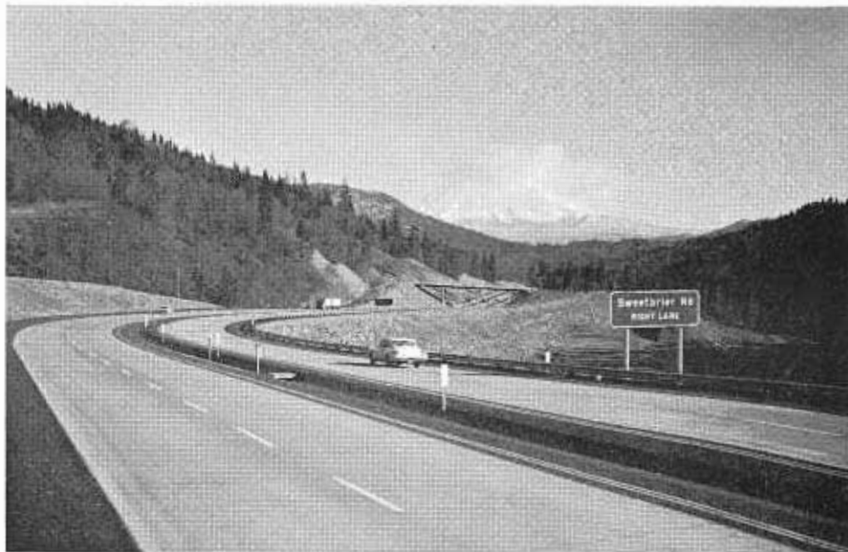
AFTER. Same section as above after freeway was completed. Sweetbrier Interchange in background. Clouds veil Mount Shasta in distance.
