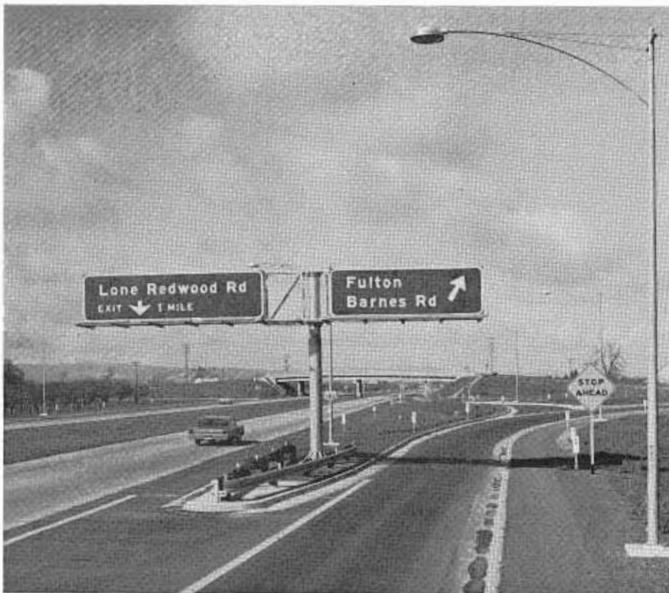
New freeway section of U.S. 101 in Sonoma County at the East Fulton Road overcrossing, completed in 1962.
