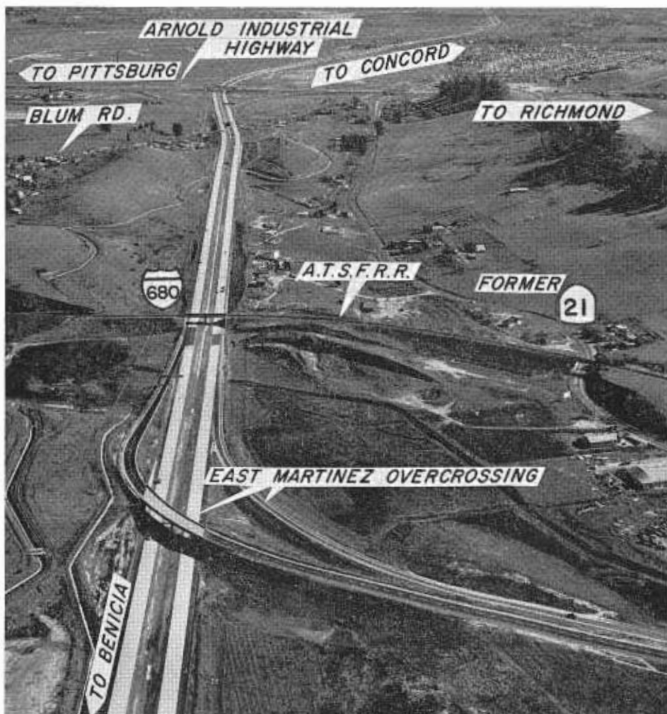
Looking southerly from vicinity of Arthur Road to recently completed section of Interstate 680 between Willow Pass Road and Benicia-Martinez Toll Bridge.
