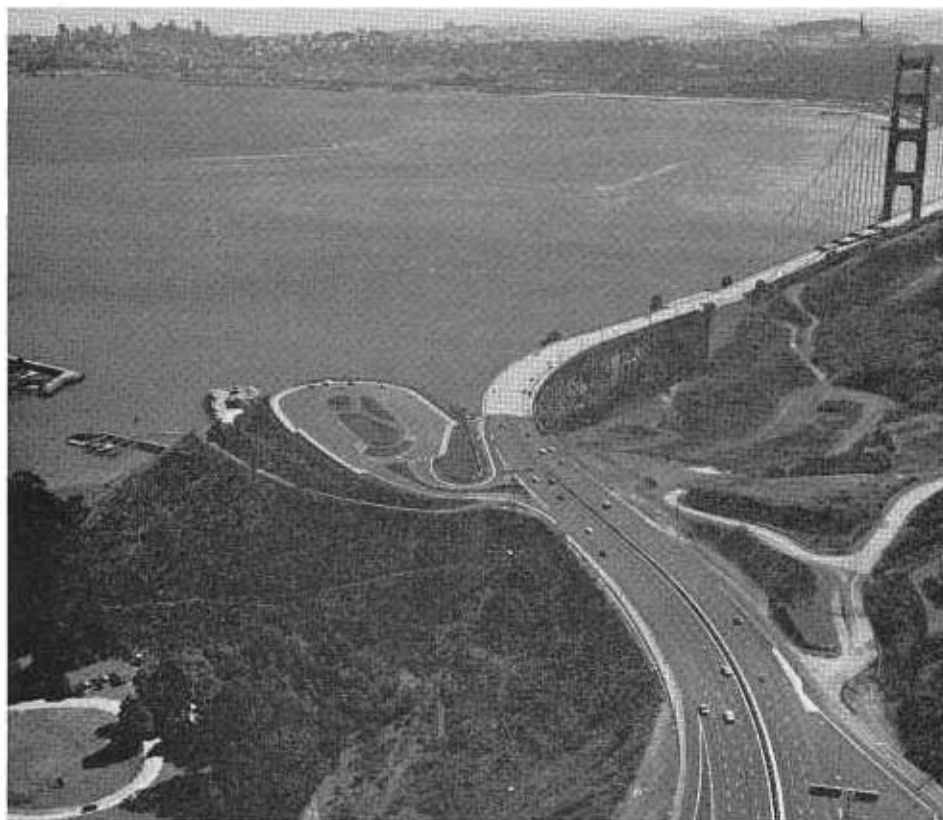
Looking southerly to the recently completed Vista Point and reconstruction at the north end of the Golden Gate Bridge. The City of San Francisco in the background.
