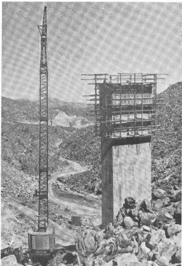
Piers were slip-form construction.
