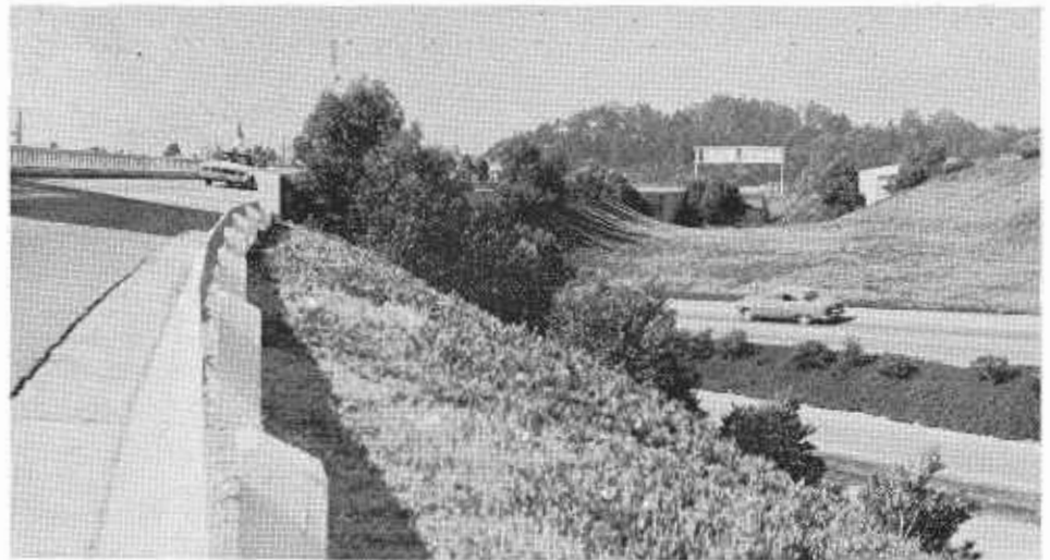
A fine example of landscaping in District IV near the City of Santa Cruz. In the coastal air the iceplant is particularly well adapted.
