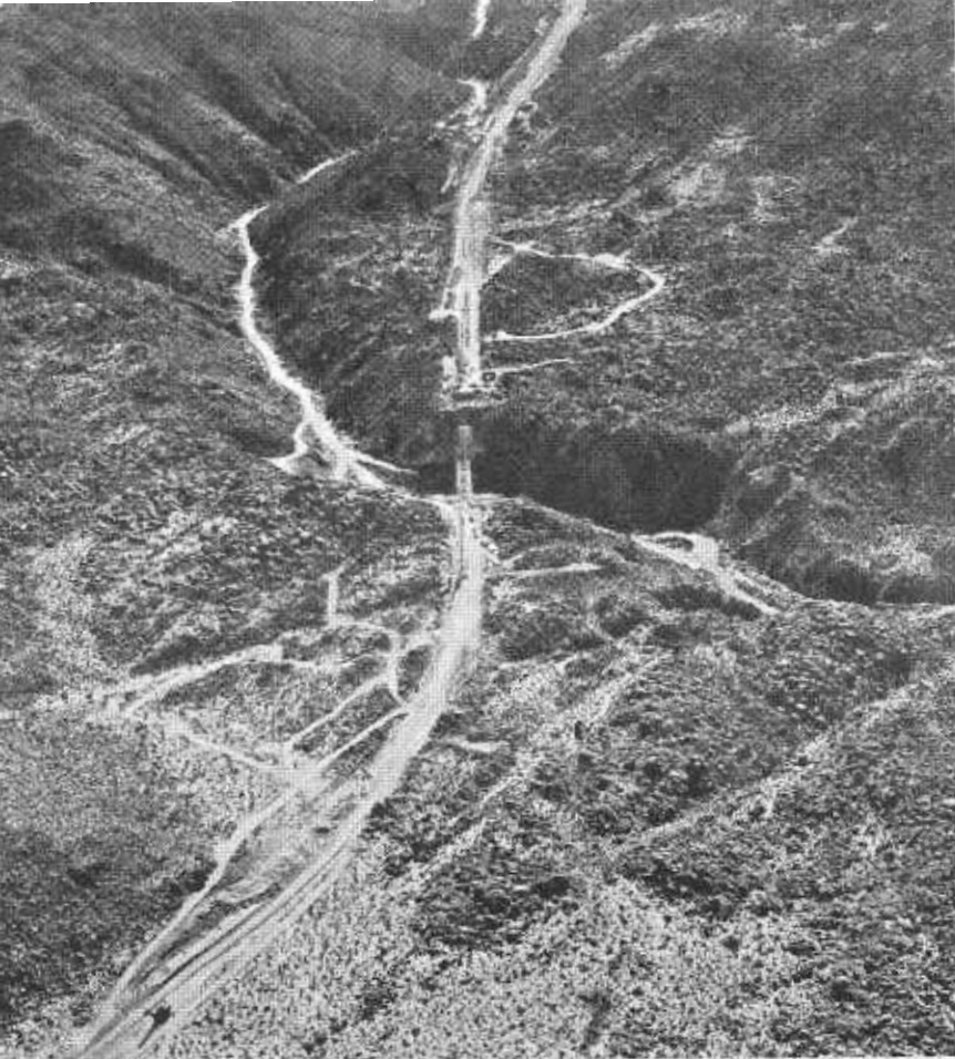
Aerial view of site.
