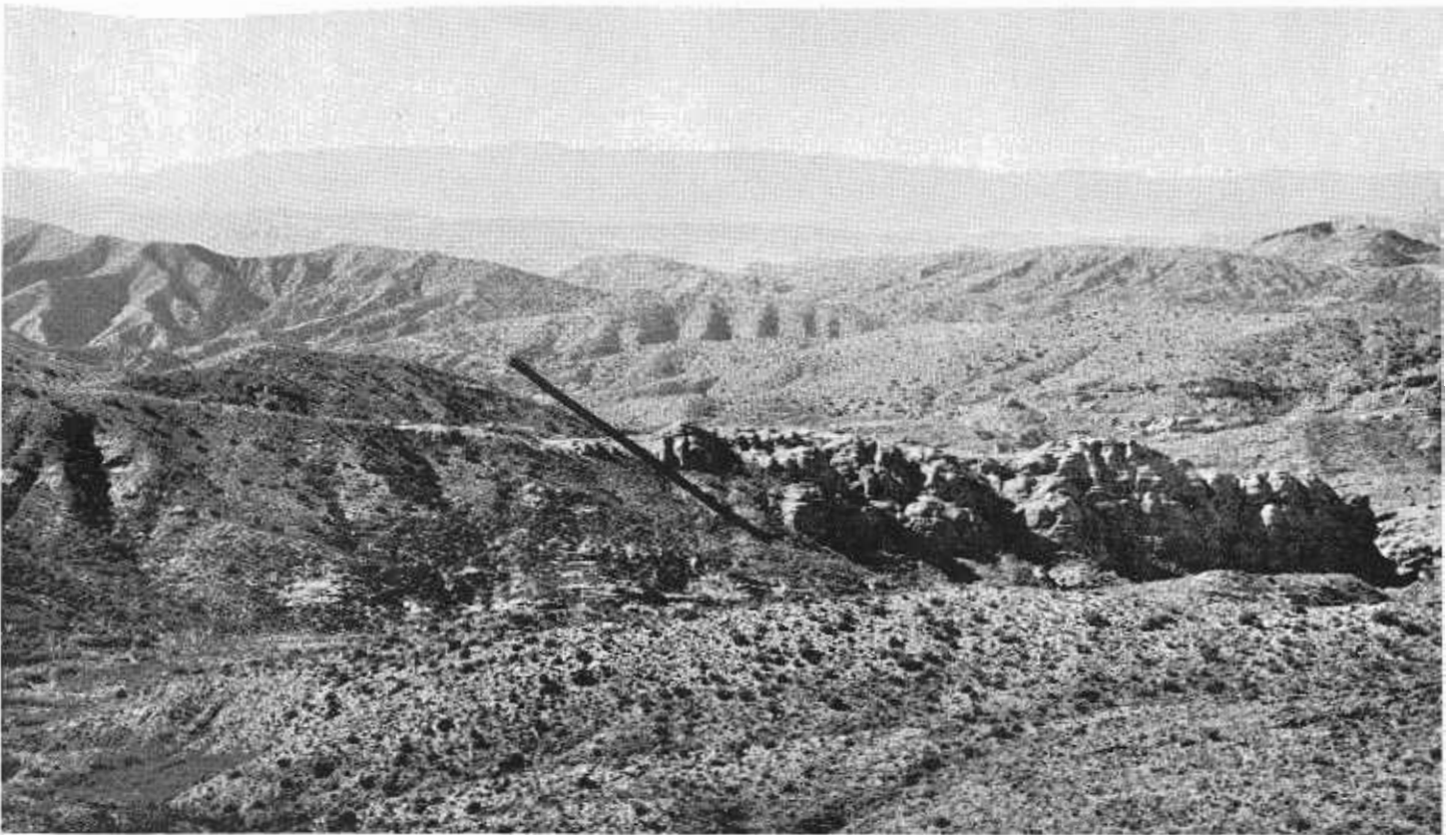
A 1960 photo looking west along the proposed location of the Antelope Valley Freeway indicated by the superimposed line. Some 800,000 cubic yards of material were removed from the cut through this bluff.
