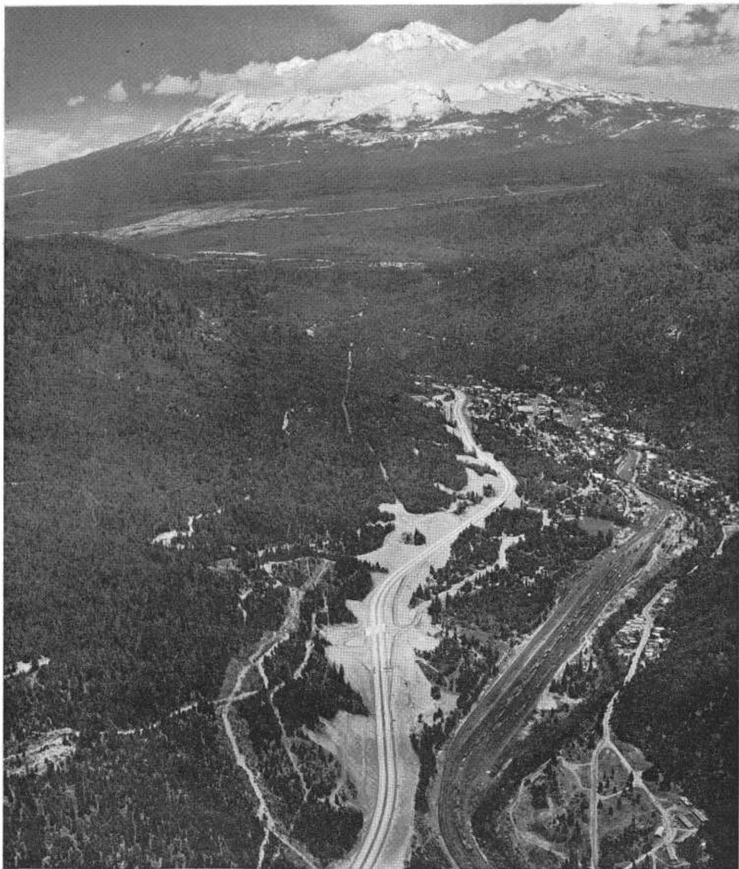
Looking north along the new freeway toward Mount Shasta with the City of Dunsmuir in the middleground.
