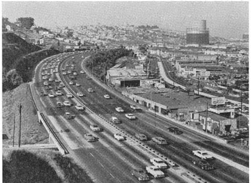
AFTER. The present Bayshore Freeway looking northward toward the Army Street interchange. (See photo above.)
