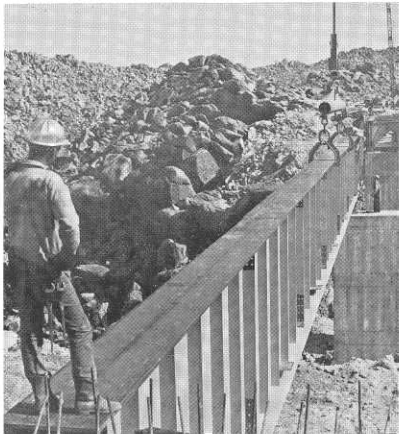
Closeup of girder placement.
