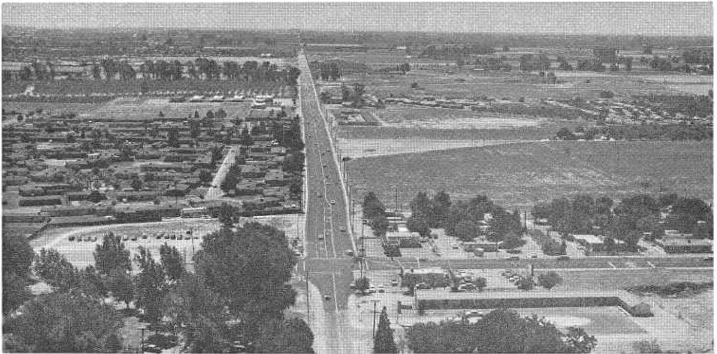
This recently completed widening of Bellevue Road between Buhach and Shaffer Roads in Atwater, Merced County, was financed with federal, state, county and city highway user tax funds.
