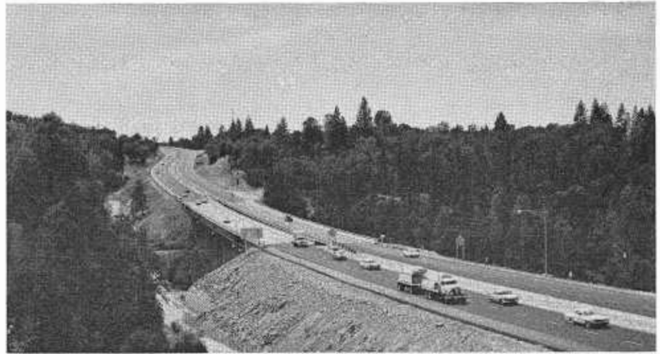
Shown is a freeway section of U.S. 50 west of Placerville completed in September. An expressway section west of Camino and a 5.5-mile freeway near Pollock Pines on this route will be completed in 1964.
