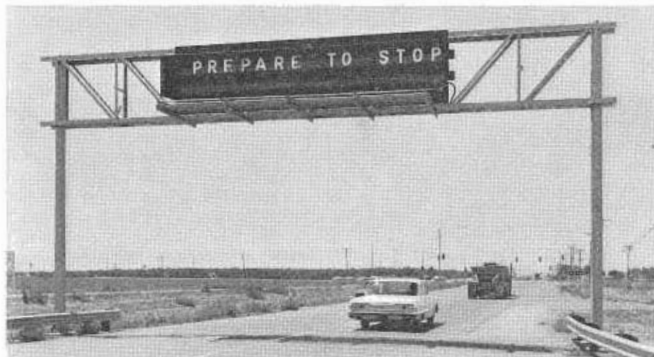
An experimental illuminated sign with a changing message to warn fast traffic of a stop or slow moving traffic ahead at the signalized intersection of U.S. 50 and Sign Route 33 near Tracy.
