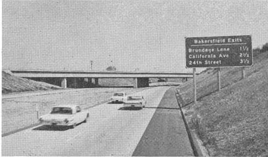
The $13,000,000, 17-mile Bakersfield Freeway on U.S. 99 was completed last summer. Most of its length had been opened to southbound traffic in 1962.
