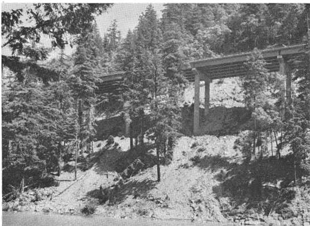
The Eagle Point Viaduct carries the Redwood Parks Freeway (U.S. 101) traffic on part of a 5.7-mile freeway section completed in October south of Myers Flat.
