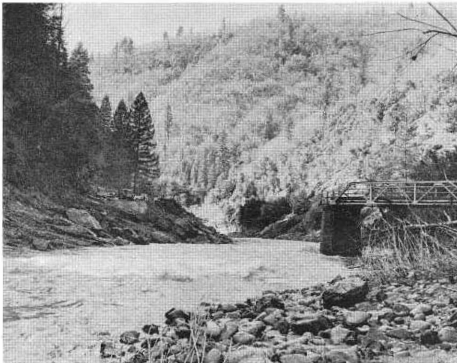
The high water on January 31, 1963, destroyed the Yuba River Bridge on Sign Route 49 west of Downieville. Thirteen days later a single 120-foot welded plate girder replacement span had been designed and constructed and was carrying traffic.
