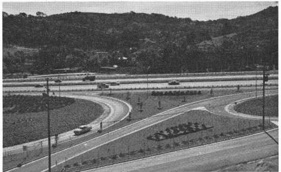
The Lafayette Bypass landscaping showing paved traffic islands with shrubs massed in geometric patterns. This treatment provides adequate sight distance for the motorist and at the same time minimizes maintenance costs.
