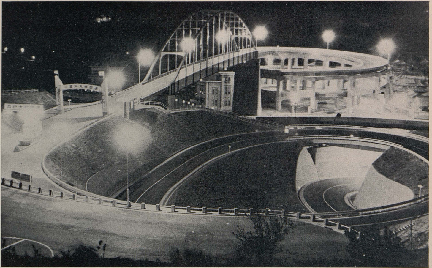
Spiral approaches to the Ondo Ohashi Bridge are shown at night.
