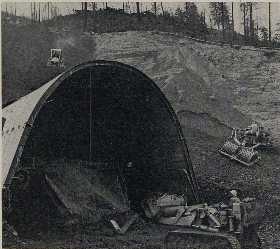
Grading and backfilling over the tunnel at the north portal.
