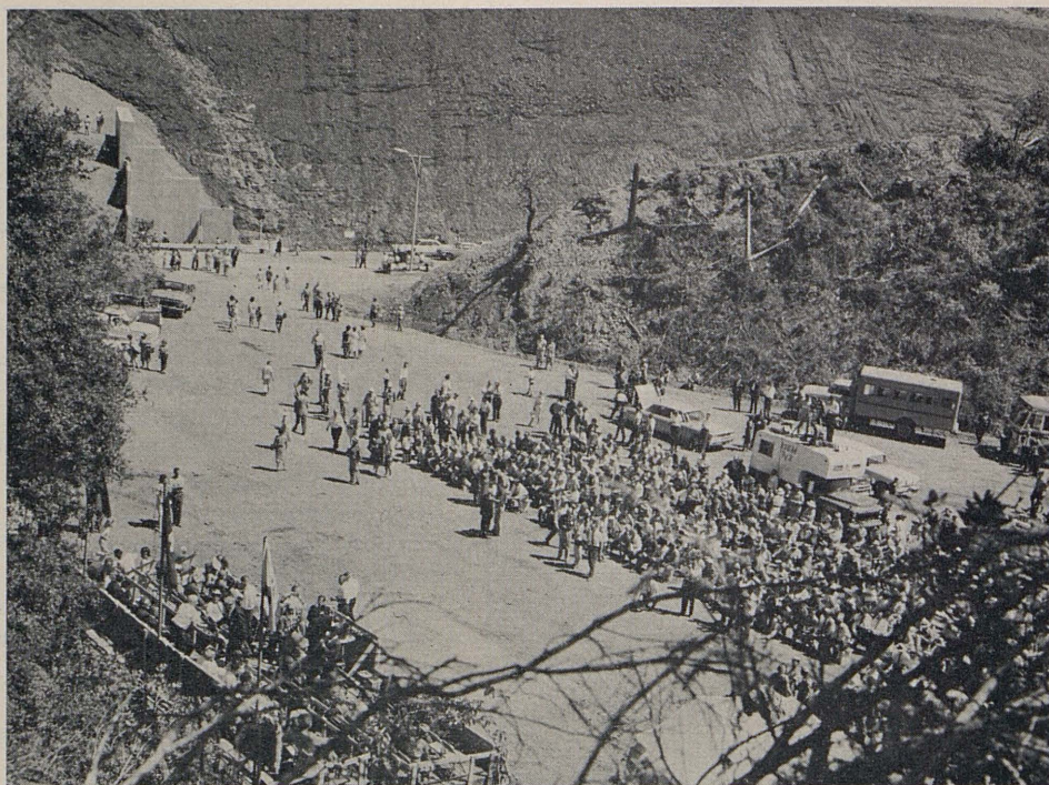
Dedication of the tunnel on July 20 drew hundreds of people and many dignitaries from California, Oregon and Nevada to honor veteran State Senator Randolph Collier in ceremonies near the south portal.
