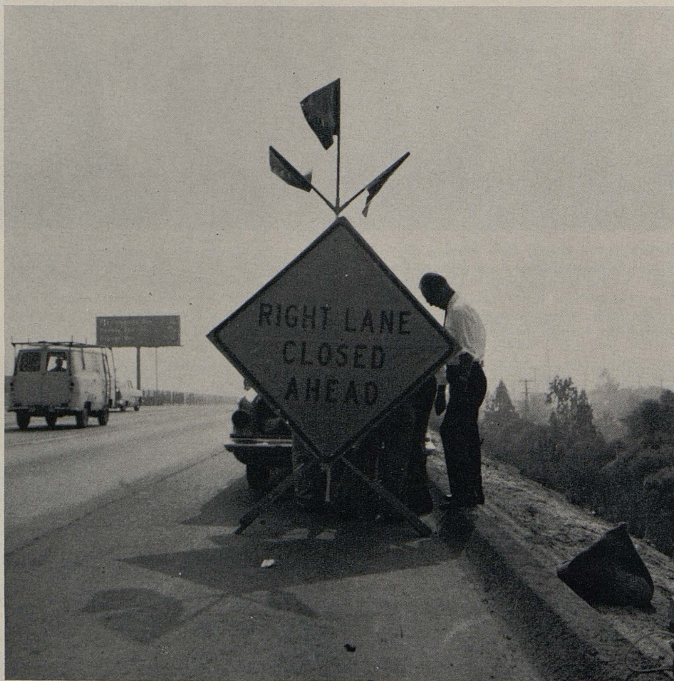
This high standard with its pattern of three flags can be seen over the top of the average car. Here, it is being used as a support for a 48-inch federal standard sign. The sign is made of nylon material and can be dismantled and transported in rolled condition.
