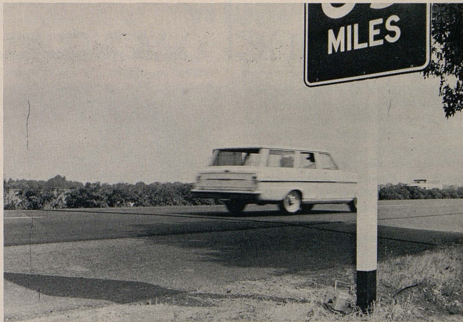
A typical junior counter installation, this one on the Roseville Freeway north of Sacramento. Note the counter chained to the base of the sign post and counter hose stretched across the pavement.
