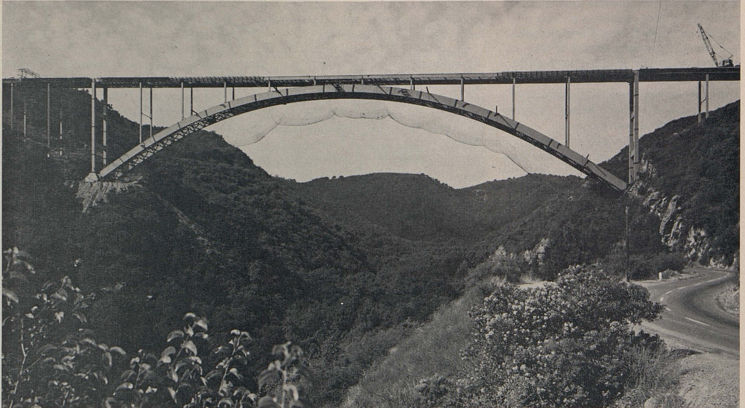
The steel structure as seen from downstream. The deck and railing remain to be completed. The bridge will be painted green as a final operation. The existing road can be seen in right foreground.
