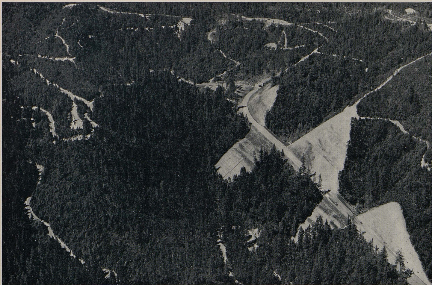
An aerial of the project looking toward the south portal of the tunnel. The old highway (left) winds through the Oregon Mountain forest and Hazelview Summit
