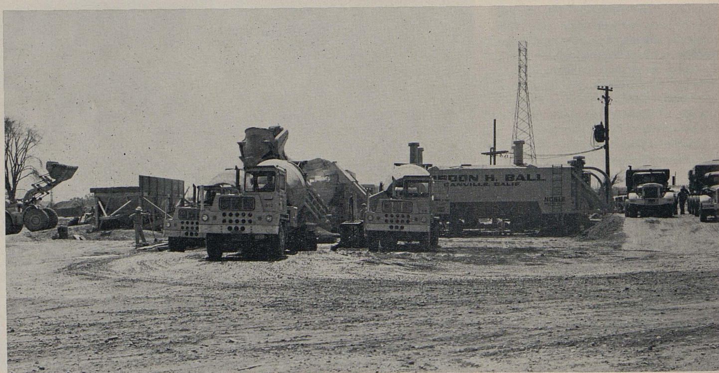
The new low profile portable batch plant is capable of batching all ingredients for 450 to 500 cubic yards per hour.
