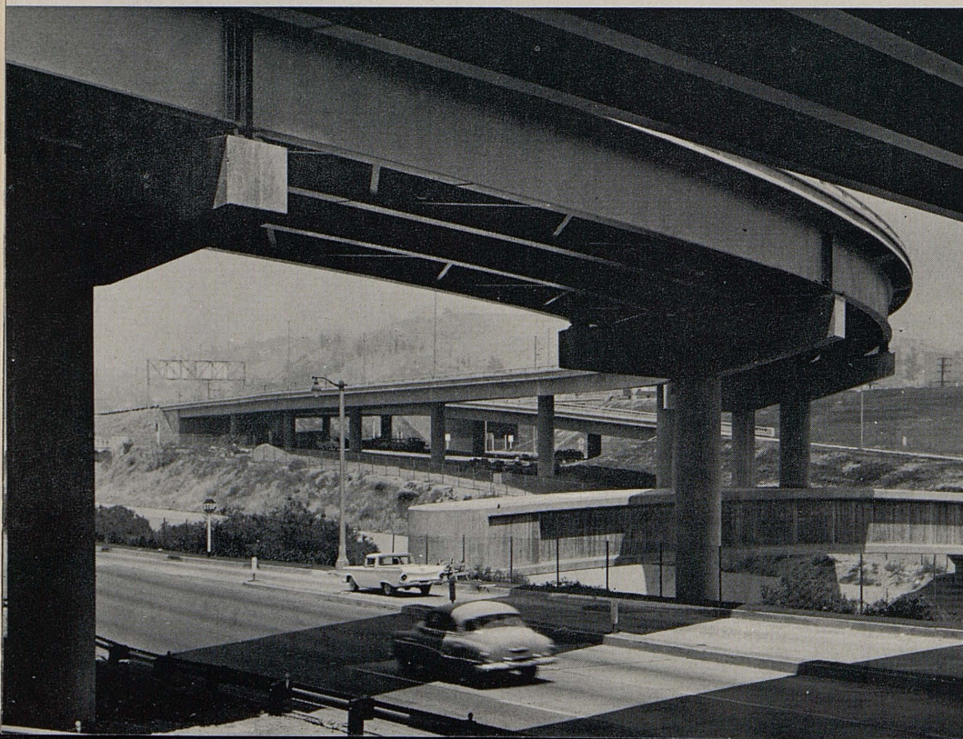
BELOW. The Elysian viaduct in Los Angeles using curved steel girders and all-welded construction, won an award in the 1962 contest. (See back cover, California Highways and Public Works, November-December 1963.)
