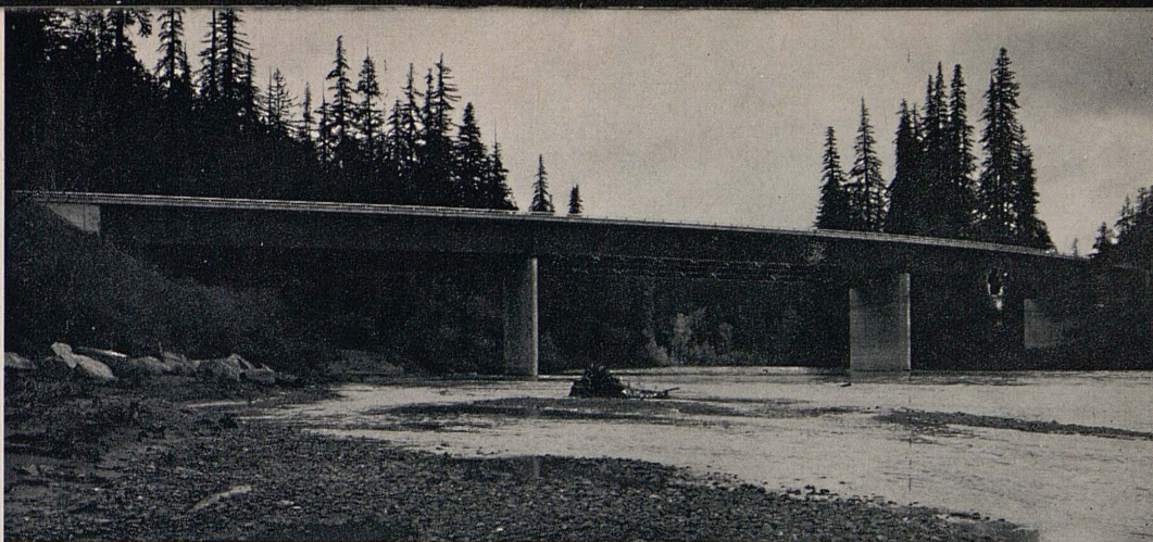
ABOVE. The George J. Cole Memorial Bridge across the Eel River at Myers Flat, a very attractive steel structure in the redwood country which received a first prize in 1962.
