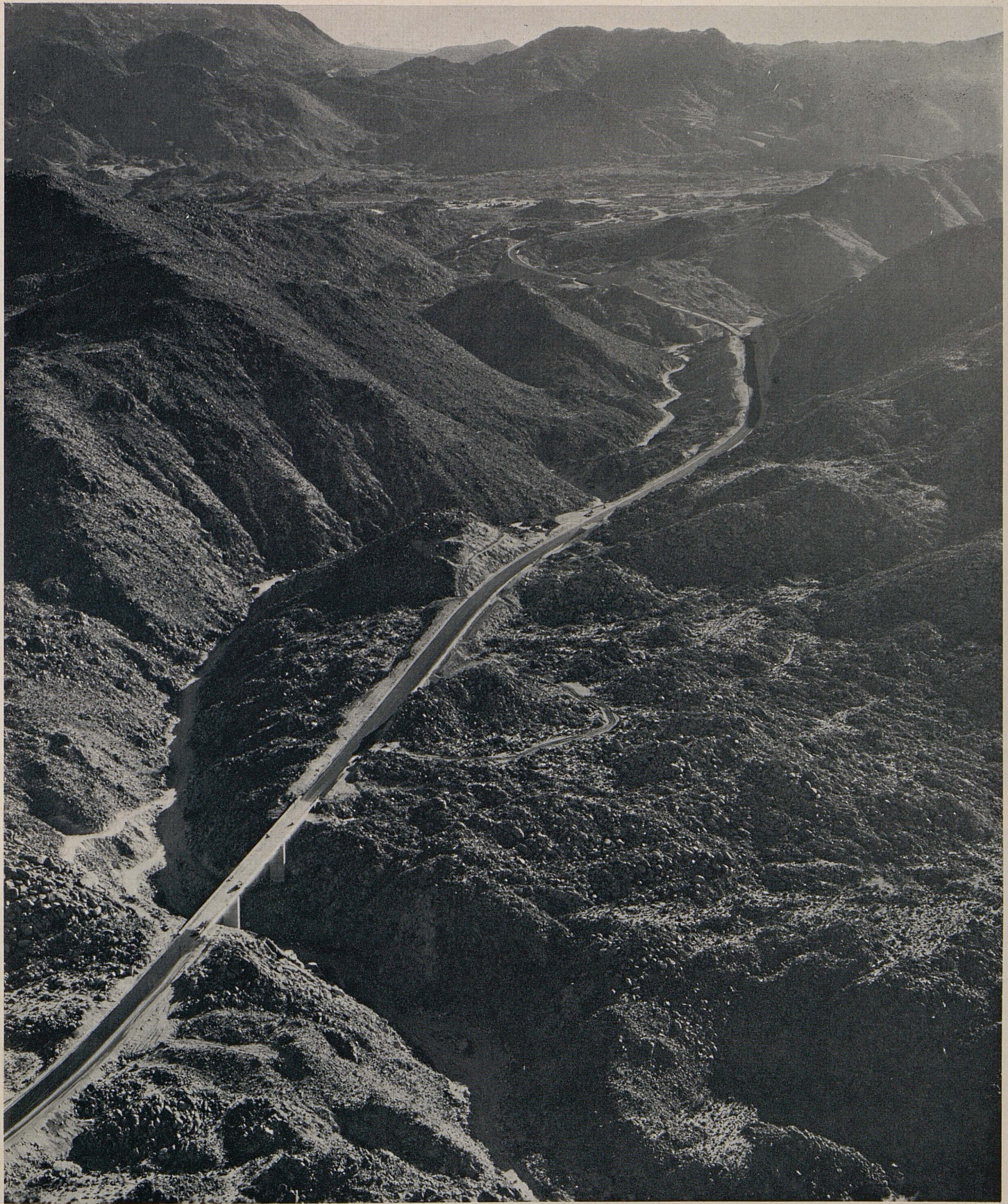
Looking south over the Mountain View—Devil's Canyon area. Bridge No. 2 is in the left foreground; Bridge No. 1 in right background. Community of Mountain Springs is visible in center background.
