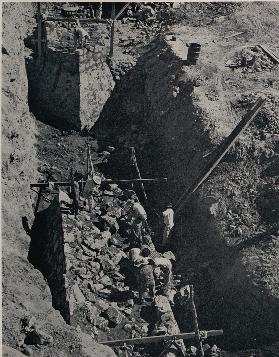
Workmen construct a native stone bridge pier.
