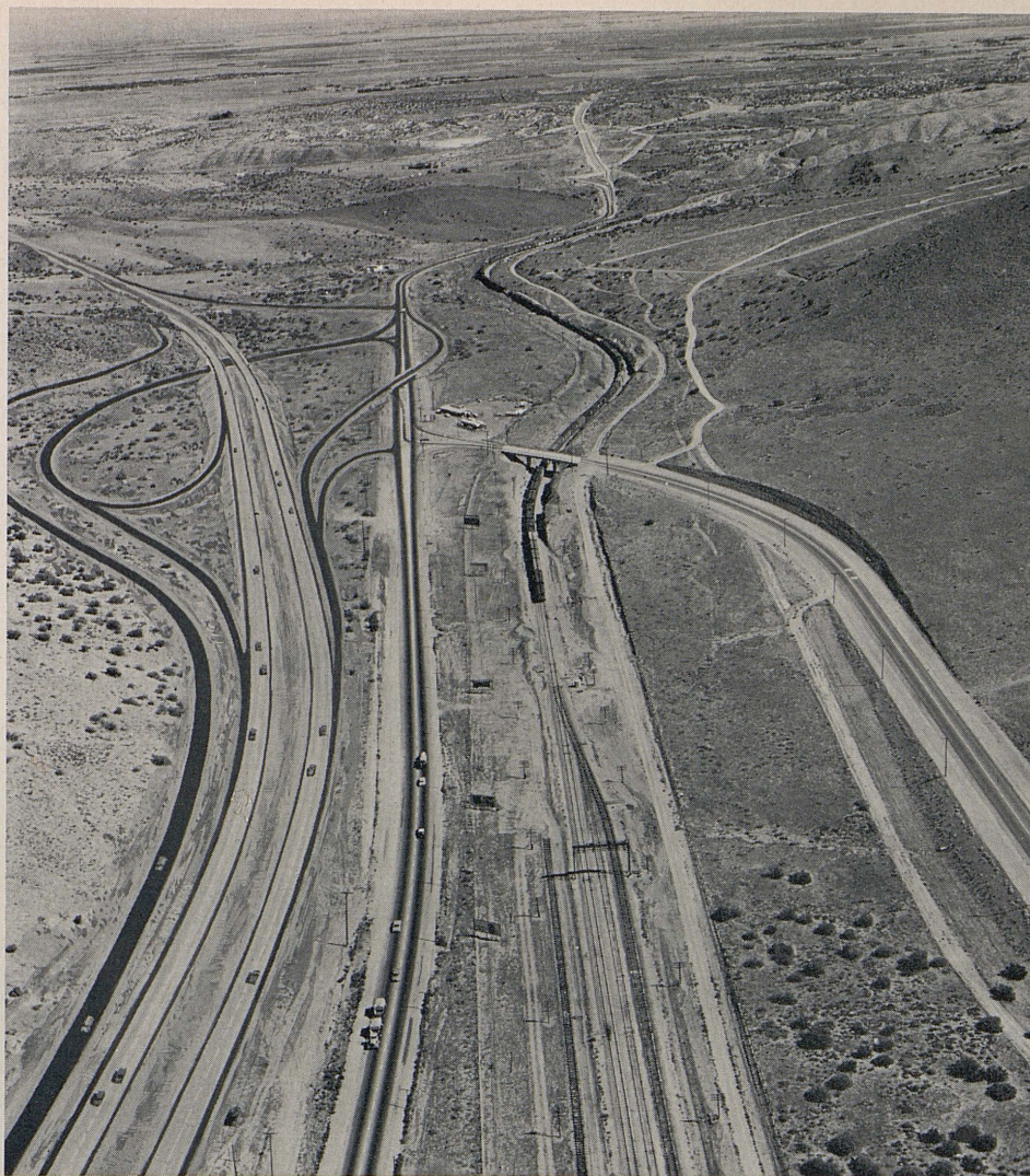
Now under construction, the Antelope Valley Freeway (artist's rendering at left) will contrast sharply with the two existing roadways at right. Sierra Highway is center with the Angeles Forest Highway coming in from the right. This busy junction is located near Vincent.
