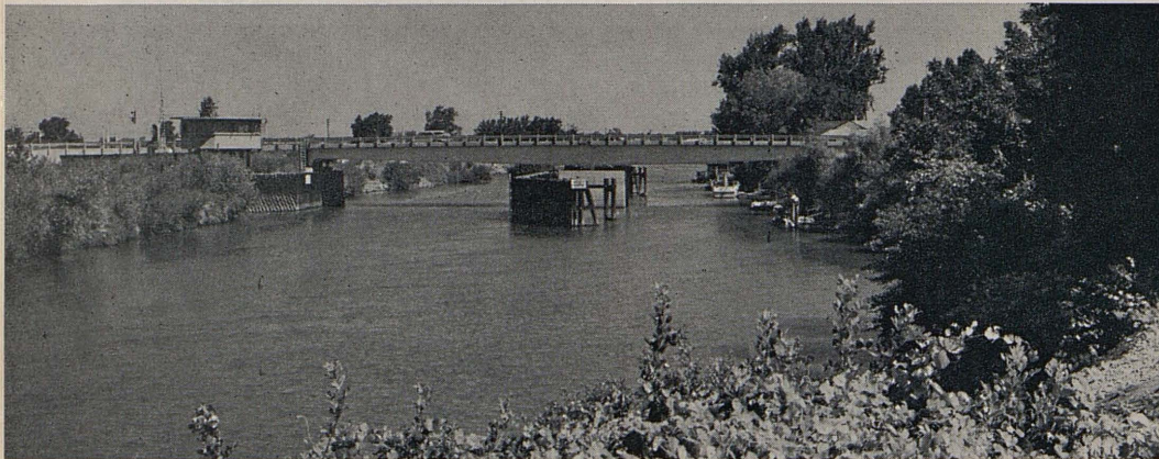
ABOVE. The Georgiana Slough Bridge at Walnut Grove over an arm of the Sacramento River. This structure, designed and built by Sacramento County with the collaboration of the Division of Highways, won the first prize for movable bridges in the 1962 competition.
