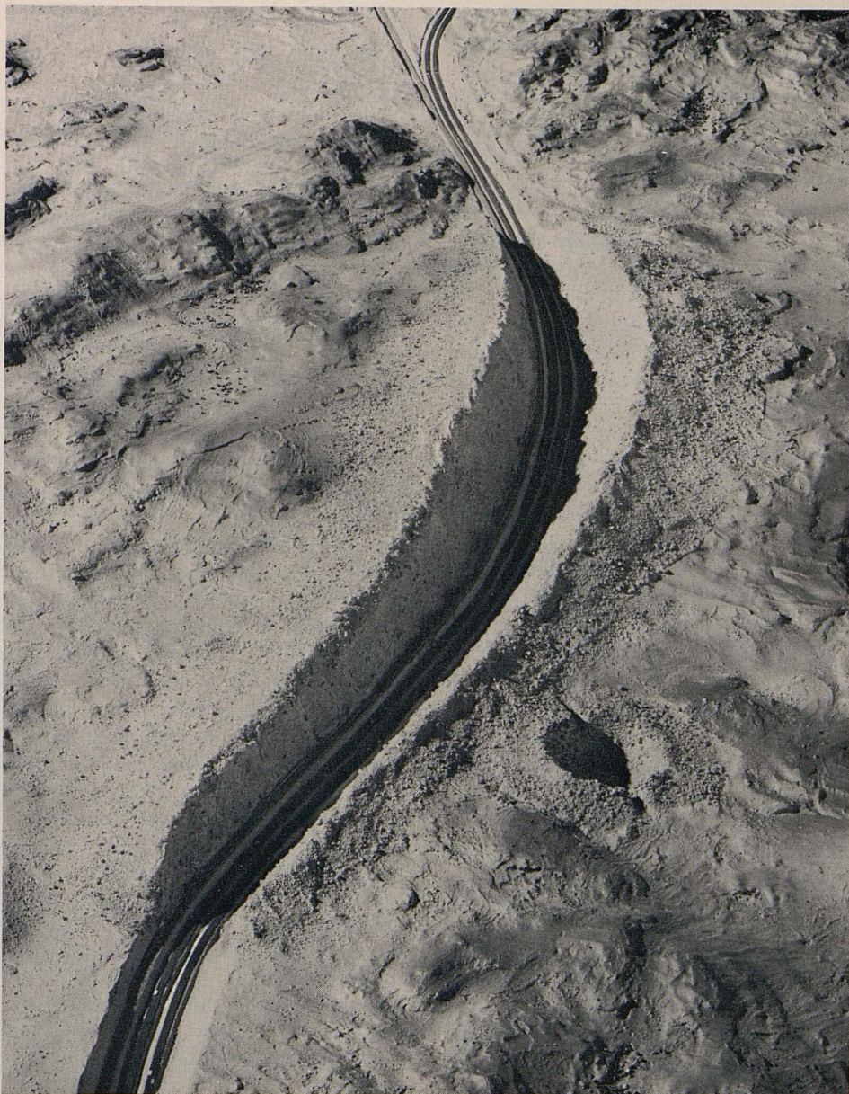
A closeup of a section of the Project Carryall model showing the roadway excavation and the drainage crater (right foreground).
