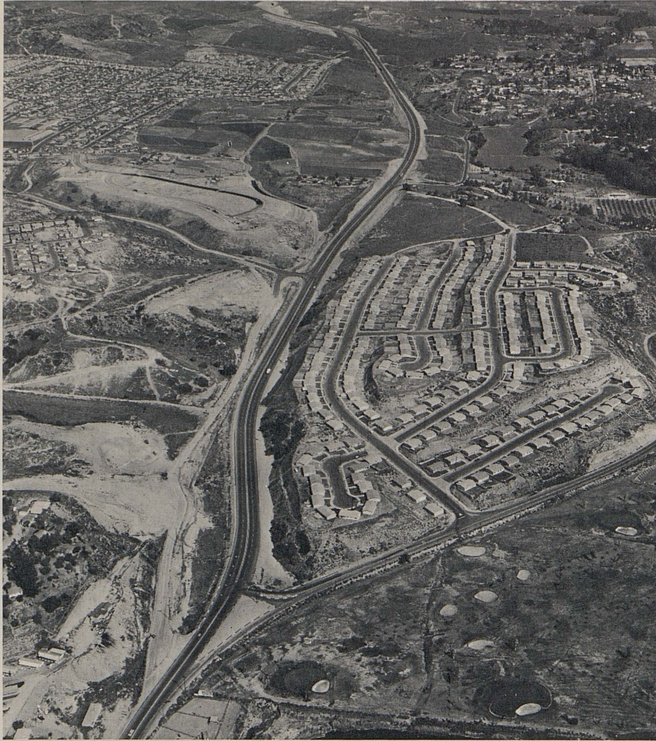
Looking northeast from Sweetwater Road at the National City end of the project. Photo on following page continues view of the freeway starting with section visible in far distance of above aerial.
