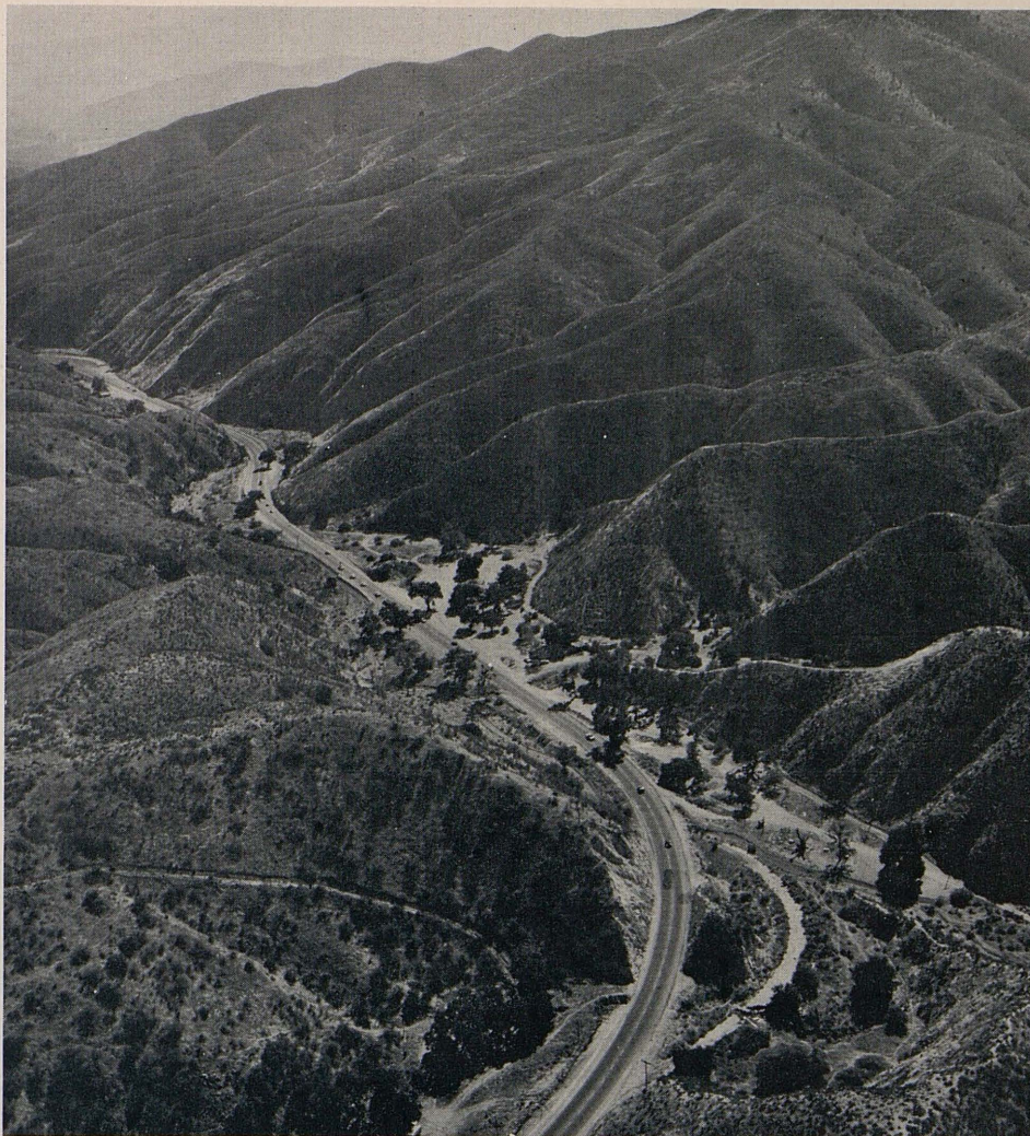
OLD. Traffic using Sierra Highway last August, before opening of the Antelope Valley Freeway, was often slowed by hills and curves through the mountains, such as on this section through Mint Canyon northeast of Solemint.
