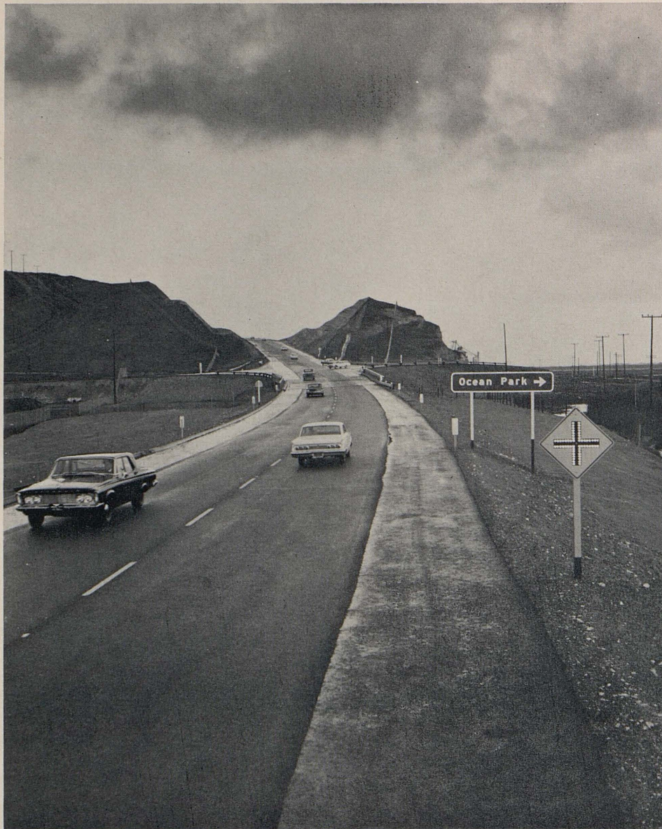
Looking west along a new section of Sign Route 154 toward the seaside community of Surf. This highway also carries traffic to the Point Arguello naval missile facilities.
