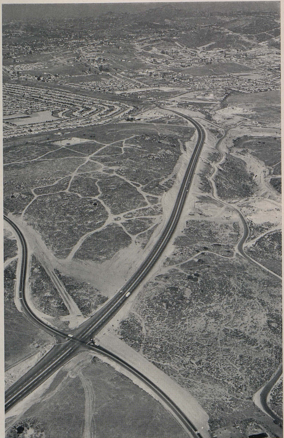
Looking northeast from Sweetwater Road crossing toward reentry into Sweetwater Road at the northeast end of the project. Both large rock cuts show clearly.
