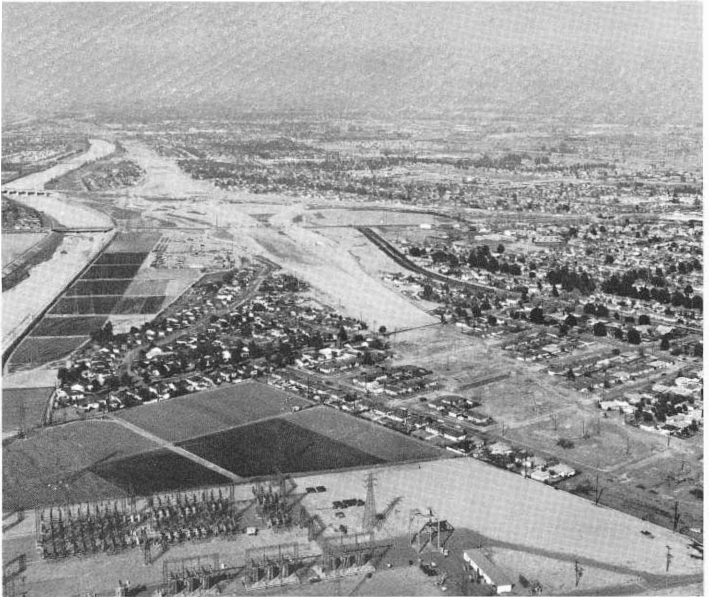
Aerial view shows future Interstate 605 Freeway course northward through a corner of Downey. Southern California Edison Company installation is at lower left. The three bridges across the San Gabriel River show the locations of Florence Avenue, the Santa Ana Freeway, and Telegraph Road. Beyond Telegraph Road, the river divides Pico Rivera on the west from Santa Fe Springs on the east.
