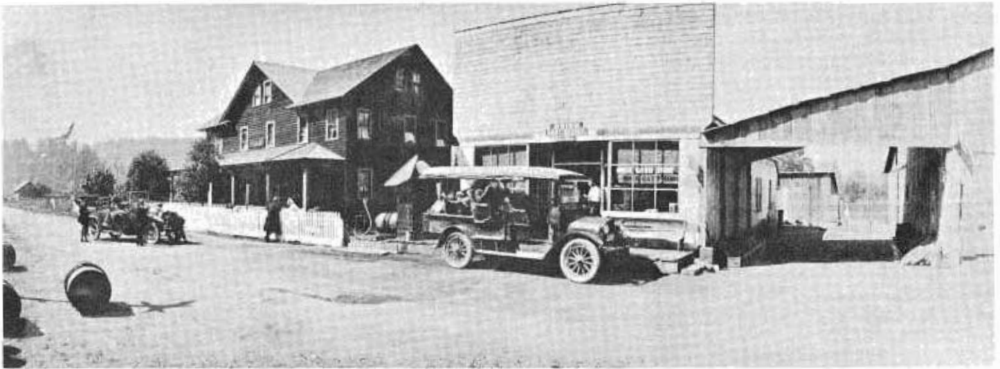
Orick, northern Humboldt County, about 1925. Vehicle stopped at post office is "stage" running between Crescent City and Eureka at that time. Note big wheels and high clearance. Gasoline in more primitive areas at that time was hauled in steel drums seen at extreme left, and attached, a drum at a time, to pump at service station. Signs say "Orick Post Office," "Notary Public," and "Orick Cash Store."
