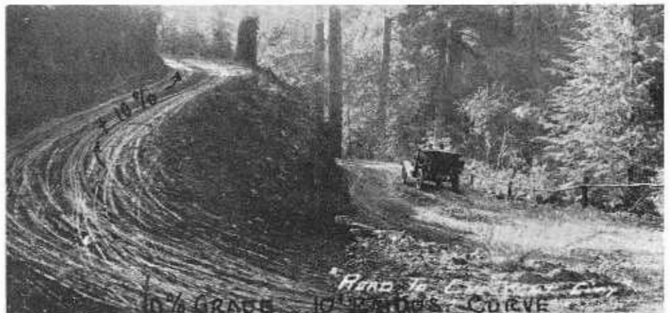
Below: The Redwood Highway just south of Crescent City in Del Norte County. Grade at left is 10 percent. Photo made on Lincoln's Birthday, 1915.
