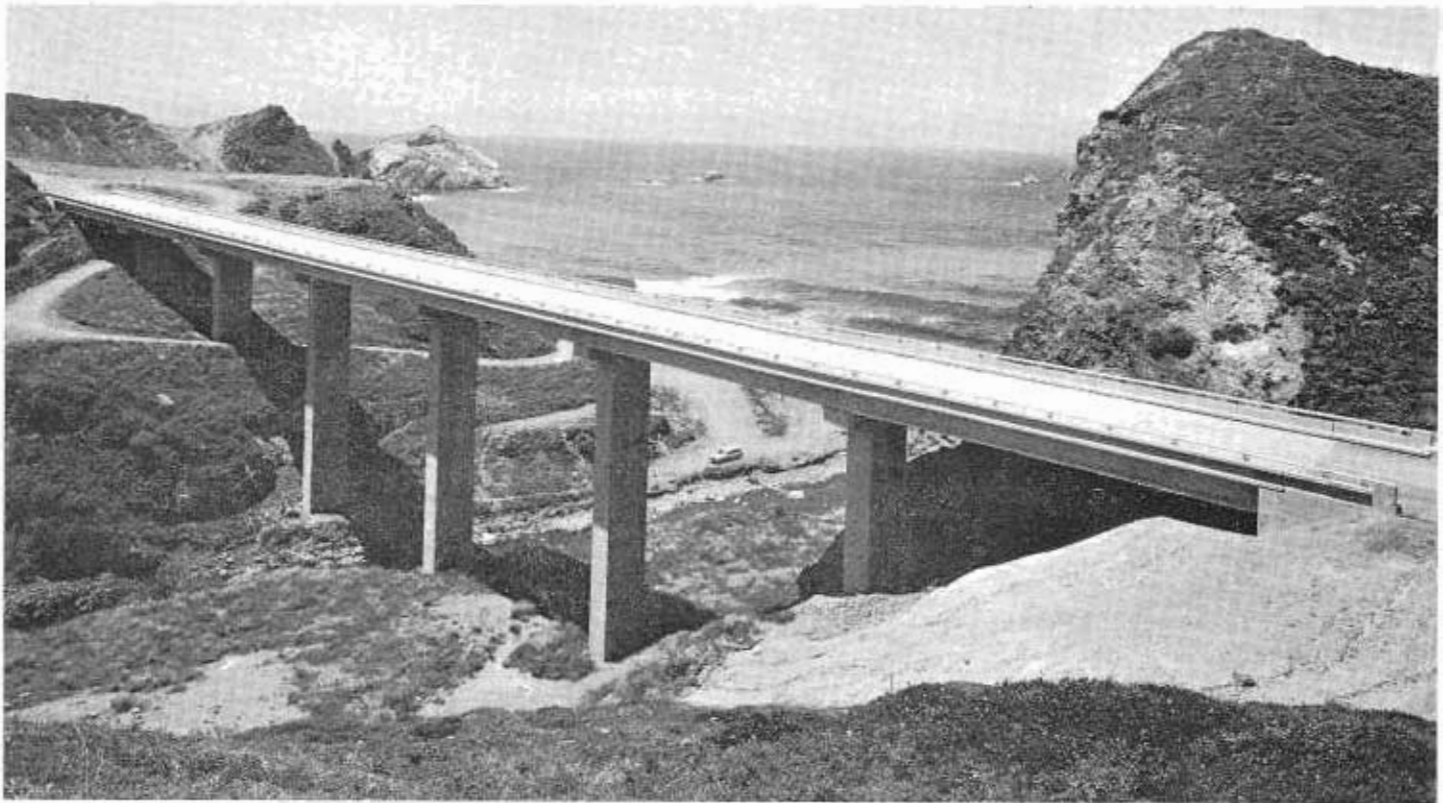
The Willow Creek Bridge on Sign Route 1 some 65 miles south of Monterey. The prestressed beams create a thin, light-appearing structure in an attractive setting beside the ocean.
