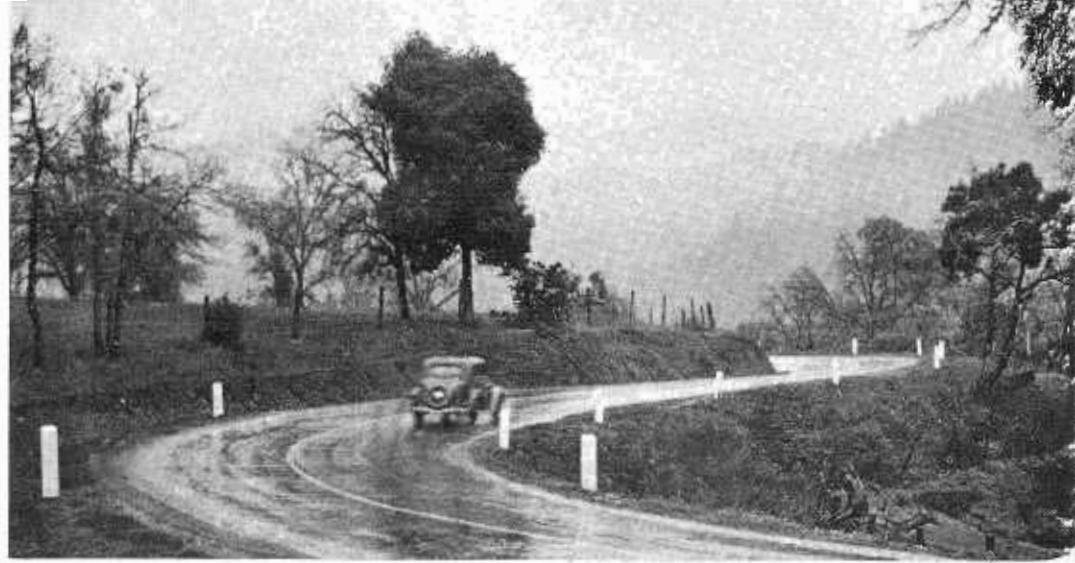
This view of the old Ridgewood Summit road south of Willits in 1938 is typical of old "reversing curve" type of construction used in those days. Earthmoving was slow and costly, and road had to follow the contours. This road has been realigned and widened to four lanes, but many miles of the Redwood Highway still follow contours.
