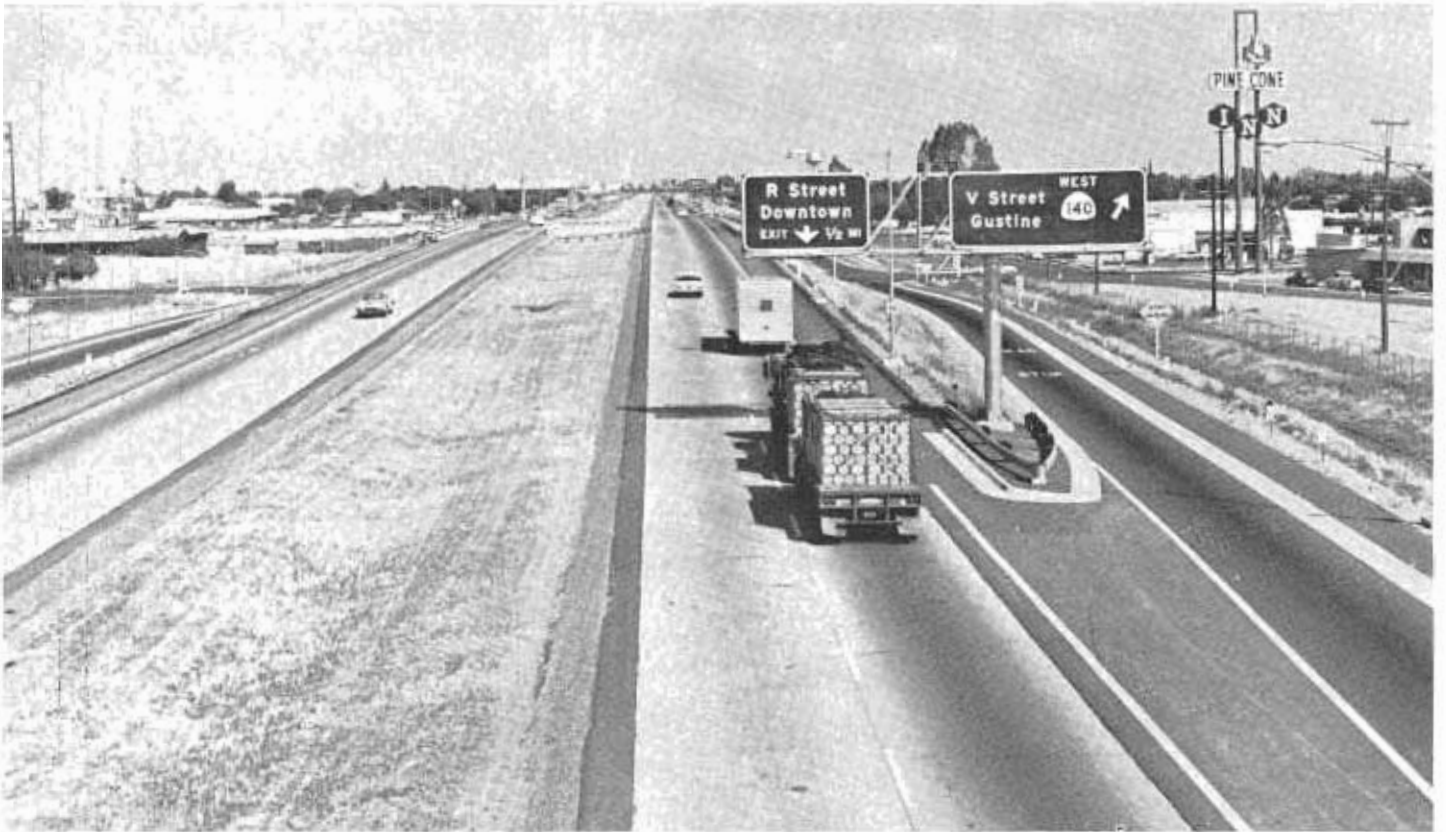
A view of the freeway at the Sign Route 140 ("V" Street) interchange.
