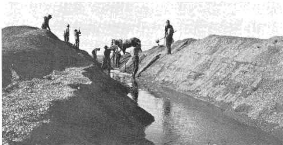
Above: Bar at Big Lagoon in 1920's was so high, lagoon could not drain into sea, and water rose to level of causeway, necessitating drainage ditch to get water into ocean.
