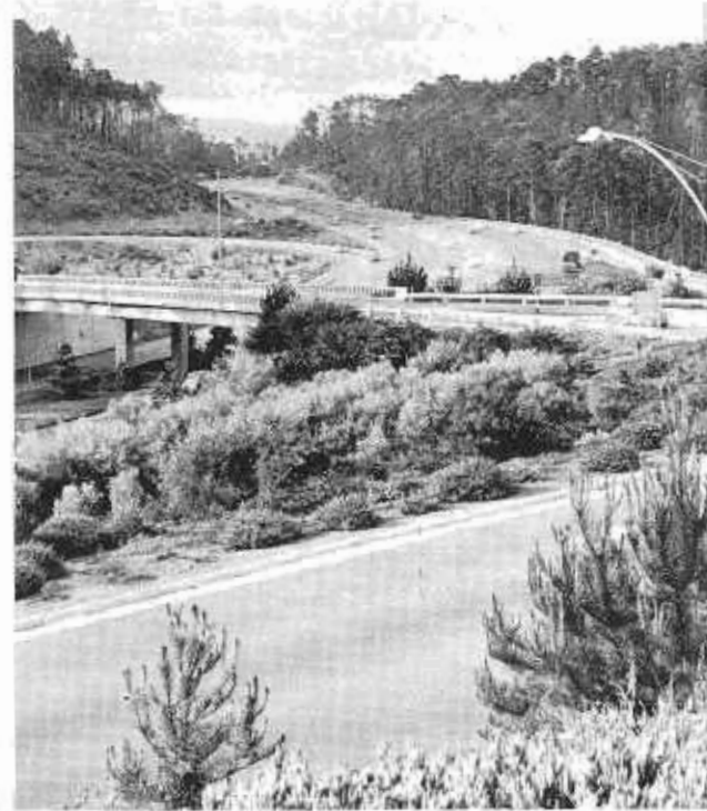
FRONT COVER. State Sign Route 1, looking southward from the Carmel-Pacific Grove Highway and 17-Mile Drive interchange. The landscaping includes such native plants as Monterey Pine, Monterey Cypress, Gowen Cypress, California Live Oak and Carmel Creeper. Photo by John Meyerpeter.
