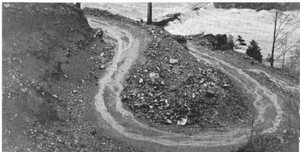
Above: Damage was great when the Smith River rose to unprecedented heights in 1920's just after the Crescent City-State Line section was taken into the state system.
