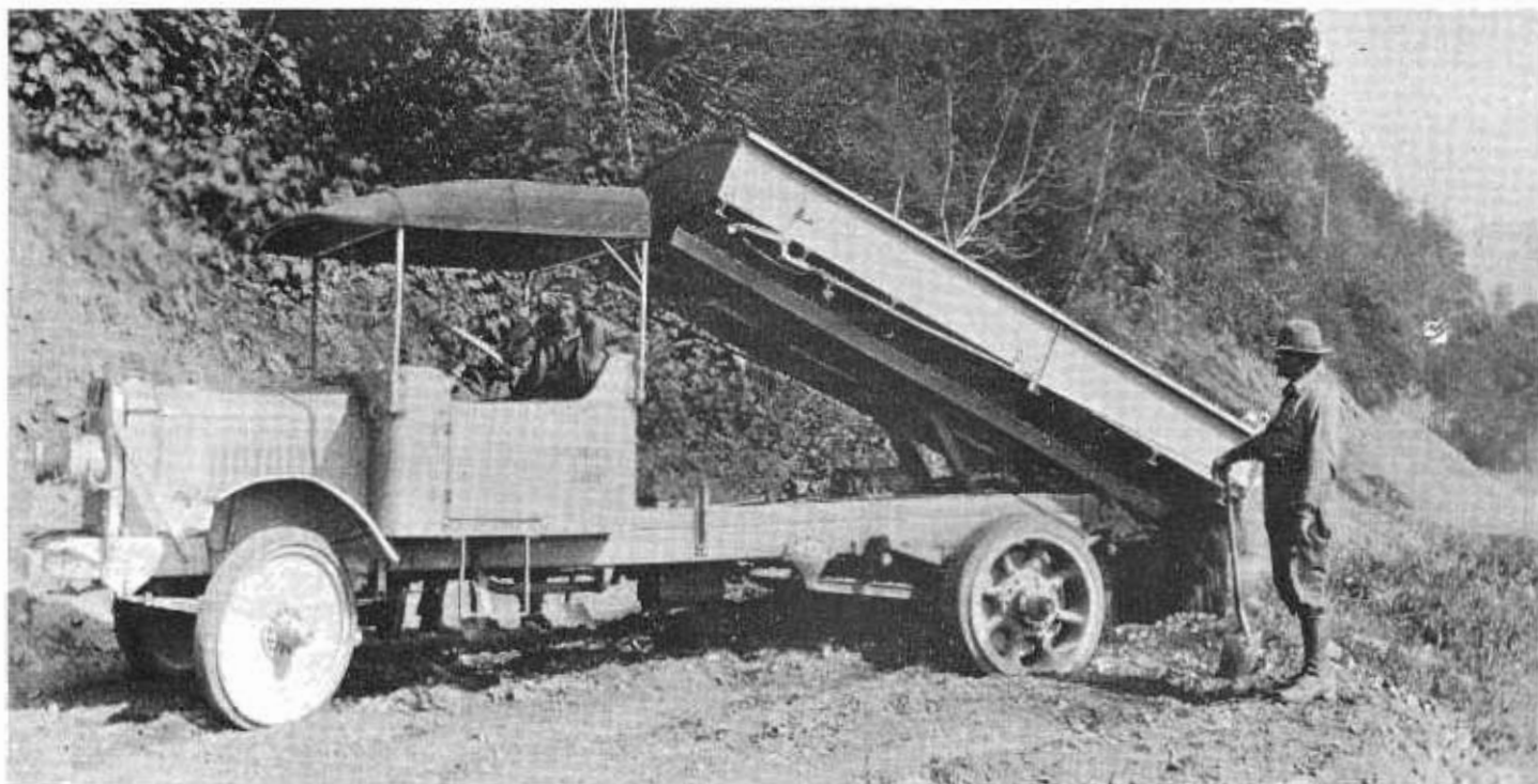
Even when powered equipment such as this Liberty dump truck could get to site, it could carry little more load than mules and wagon, and repairs after slides were slow and laborious.
