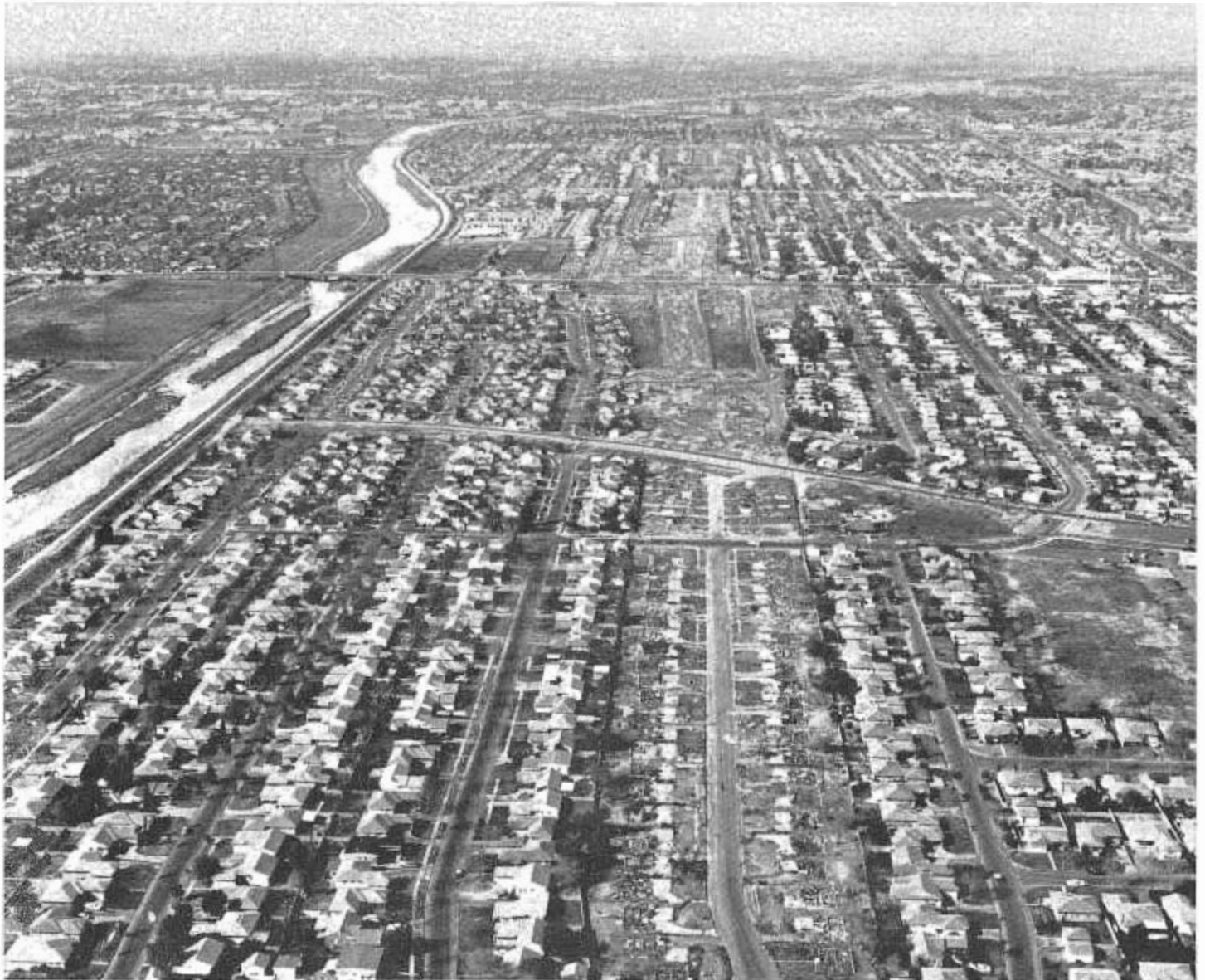
Between rows of tract houses in Norwalk, the cleared land of the Interstate 605 Freeway right-of-way extends northward paralleling the San Gabriel River. Bridges cross the river at Rosacrans Avenue and Imperial Highway.
