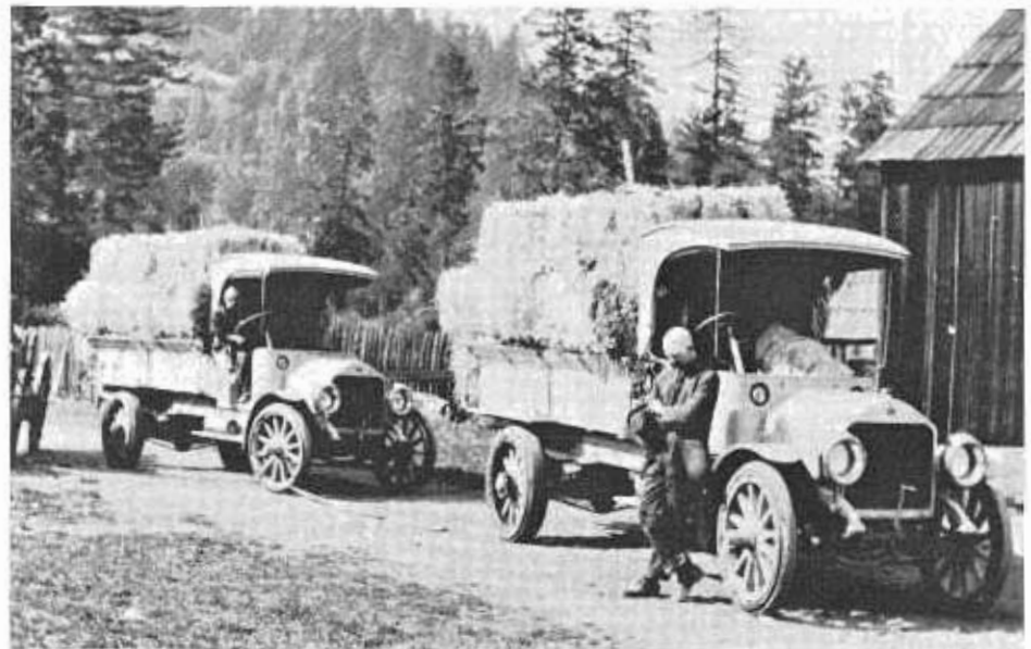
Mechanized equipment used on a job in early days of modernization of Redwood Highway near Cummings, Mendocino County. Note right hand drive on trucks, and loads of hay for mules and horses.
