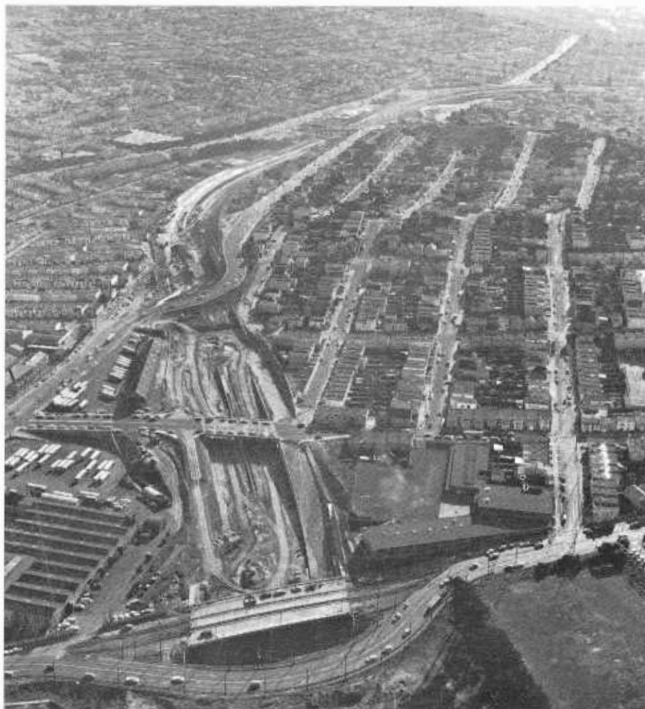
This view shows the Ocean Avenue overcrossing in the foreground with traffic routed around construction. In order can be seen the Geneva Avenue overcrossing and the San Jose Avenue detour.
