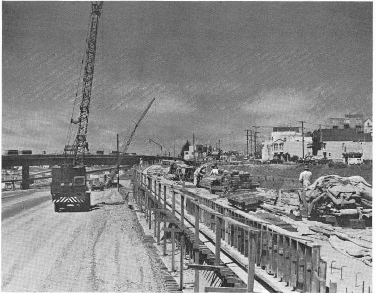
Looking westerly toward Monterey Boulevard and access ramp construction.
