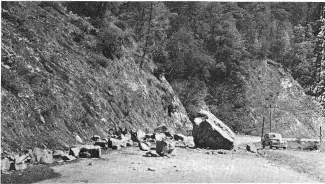
Below: Rock slide in road, Redwood Highway north of Leggett, April 7, 1948.
