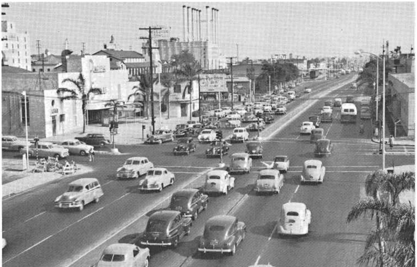
The old Pacific Highway, looking south, at Ash Street. The new freeway eliminates 16 traffic signals and 30 railroad siding crossings.
