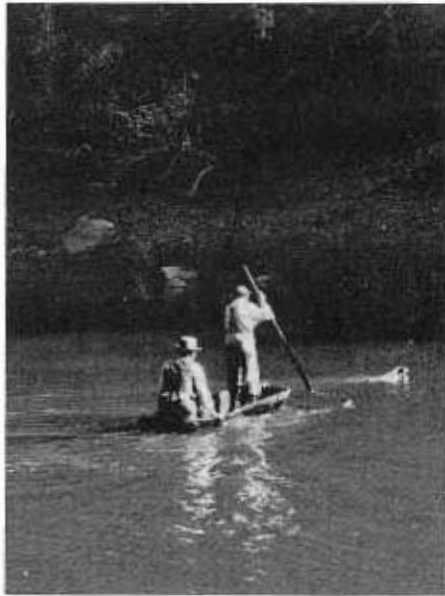
Survey crews fording the Eel River while laying out the original Redwood Highway route through the South Fork Canyon.
