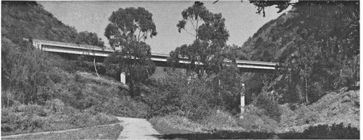
A view of the Hot Springs Creek Bridge from the streambed. To minimize disturbance to native shrubbery and for economy, the structure is supported on single, six-foot round column pier shafts mined into the rock of the steep canyon slopes.
