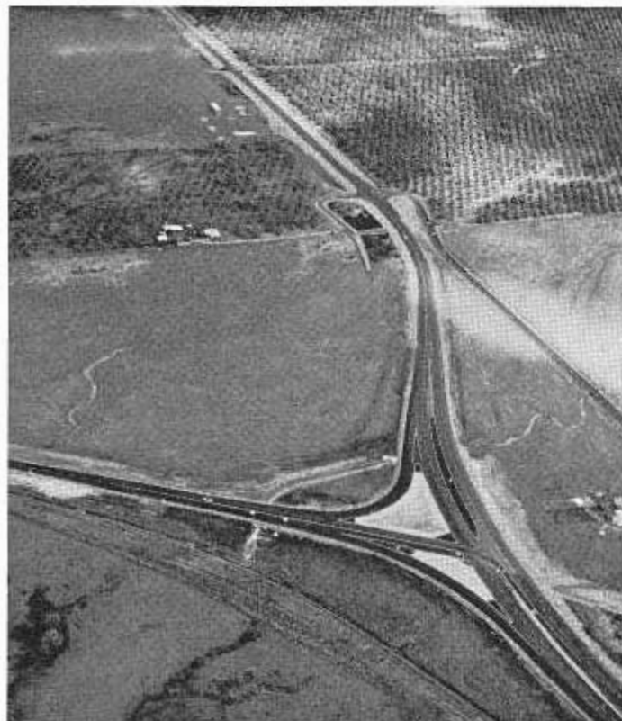
Aerial of completed Wicks Corner intersection. Old road is at right. Freeway makes transition from four lanes to two and continues toward Garbo Gap as an expressway. Road at left goes to Chico.
