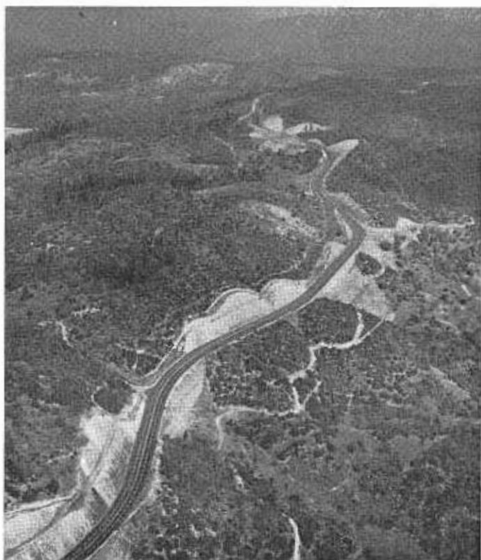
Aerial shows four-lane section northeast of the West Branch bridge.
