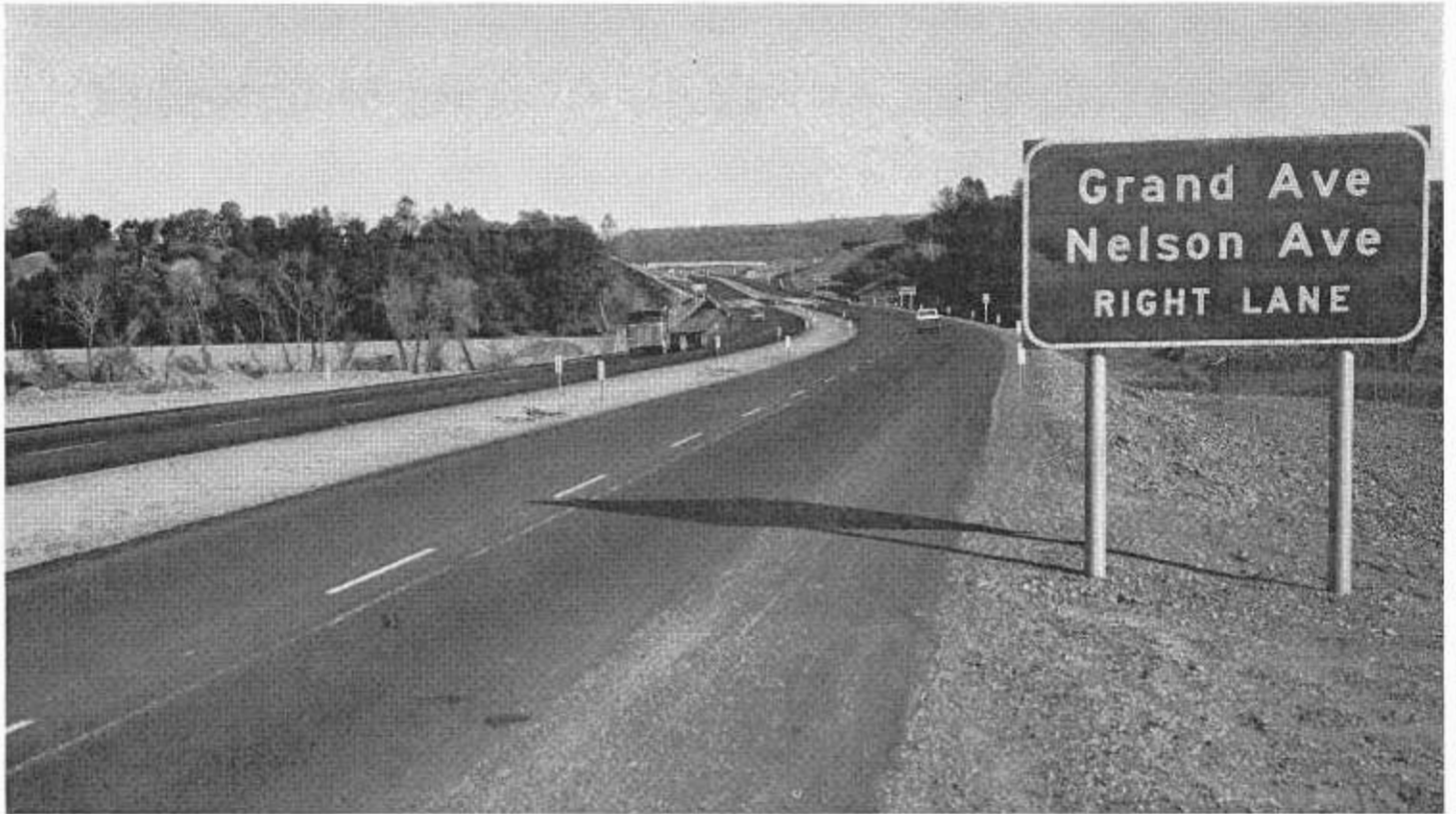
Typical view of the Oroville-Wicks Corner freeway. This one is approaching the Grand Avenue interchange in Oroville from the south, located about one-half mile north of the Feather River.
