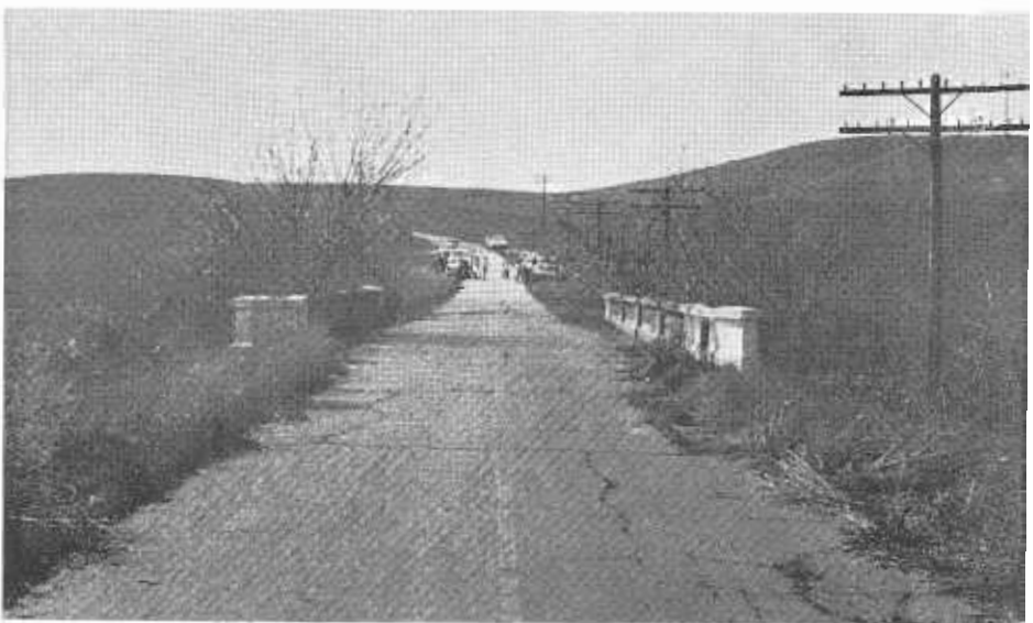
ABOVE: Same view taken three years later. The roadbed was graded and a portland cement concrete slab 15 feet wide and 6 inches thick was installed. This pavement remained in use for 30 years. In 1949 when Highway 16 was realigned, this section was abandoned but not obliterated. Today a portion serves as an access road to the famous old landmark, Sloughhouse. BELOW: Easter Sunday, 1964, 45 years after the pavement was placed. The group in the background is enjoying an old fashioned Easter egg hunt.
