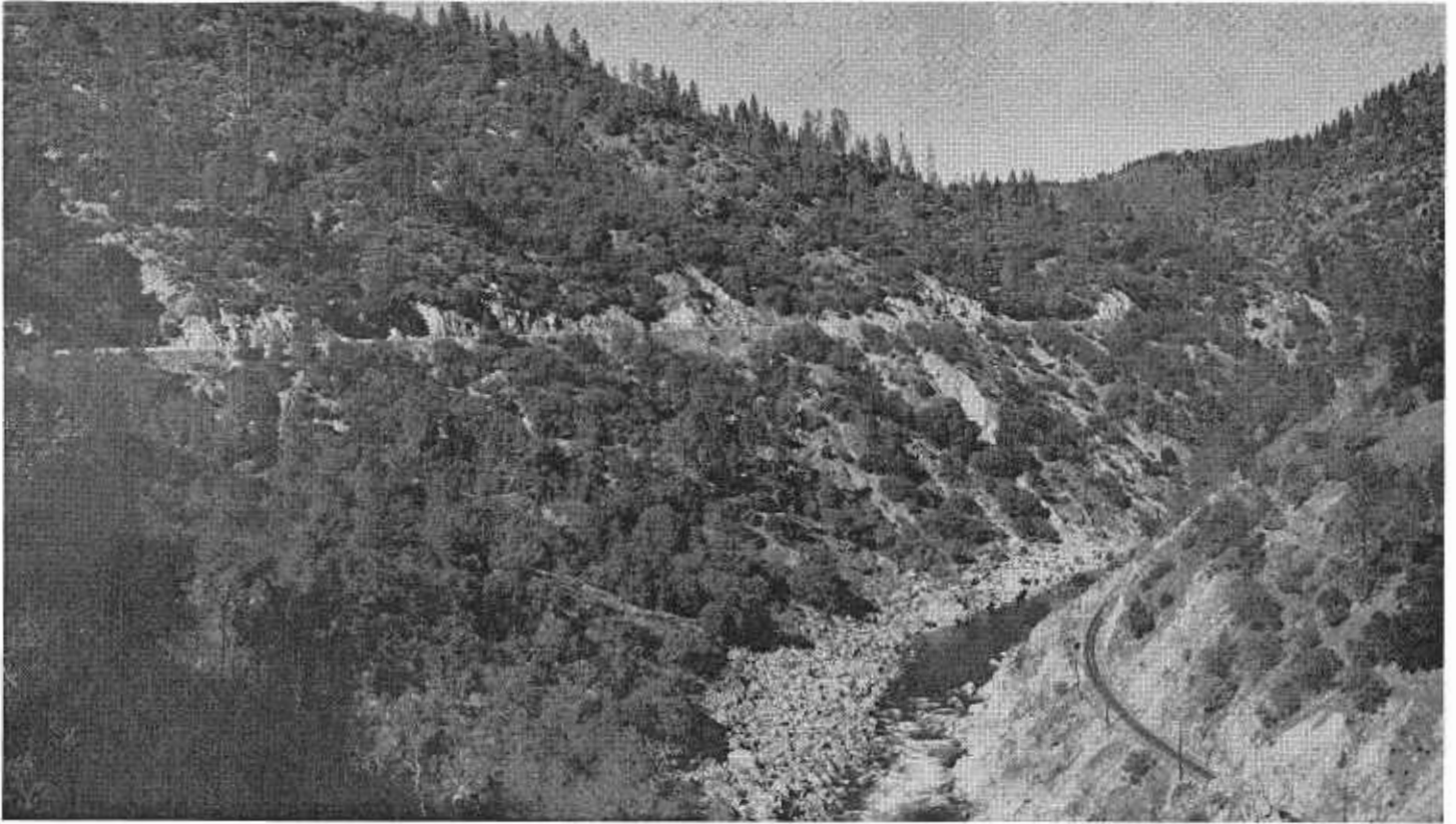
A typical view up the narrow North Fork Feather River Canyon. Old road upper left, abandoned railroad lower right. All will be inundated when reservoir is full.
