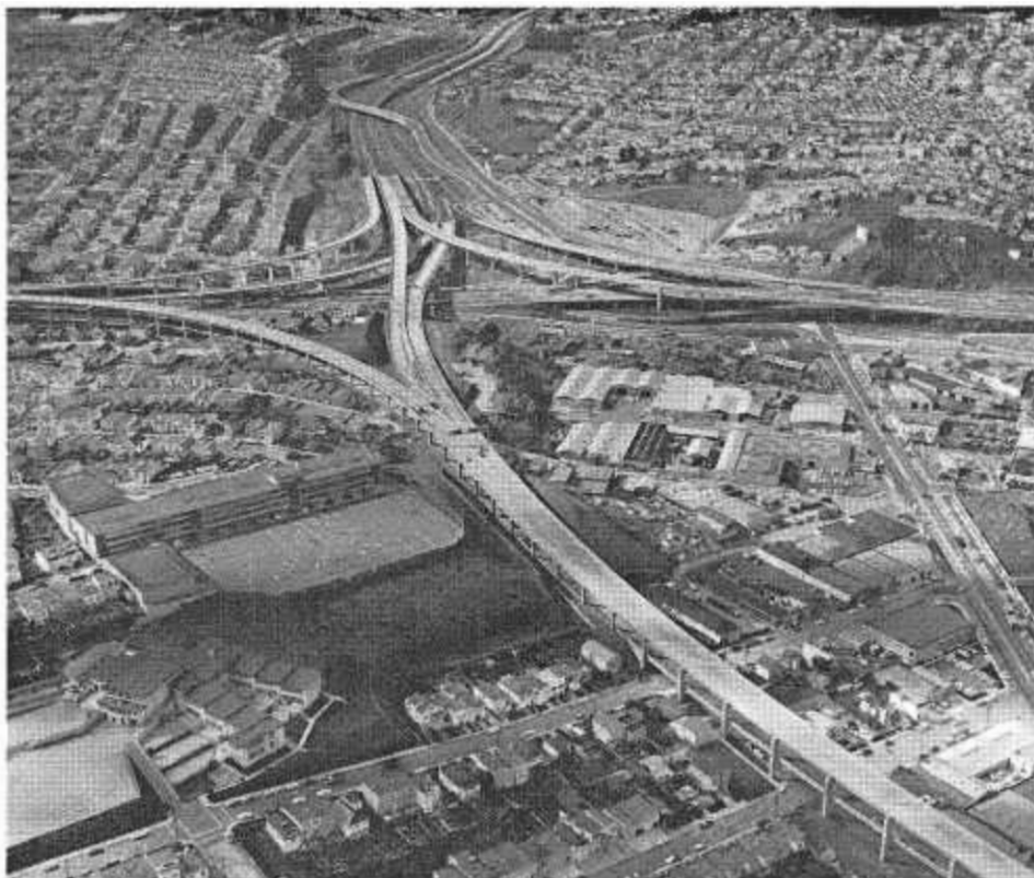
Aerial photo looks west from the vicinity of Newcomb Street toward the intersection with James Lick (Rayshore) Freeway showing the section of double-deck viaduct that was completed in February. This unit will not be usable until the next section, extending to Army Street, is constructed.
