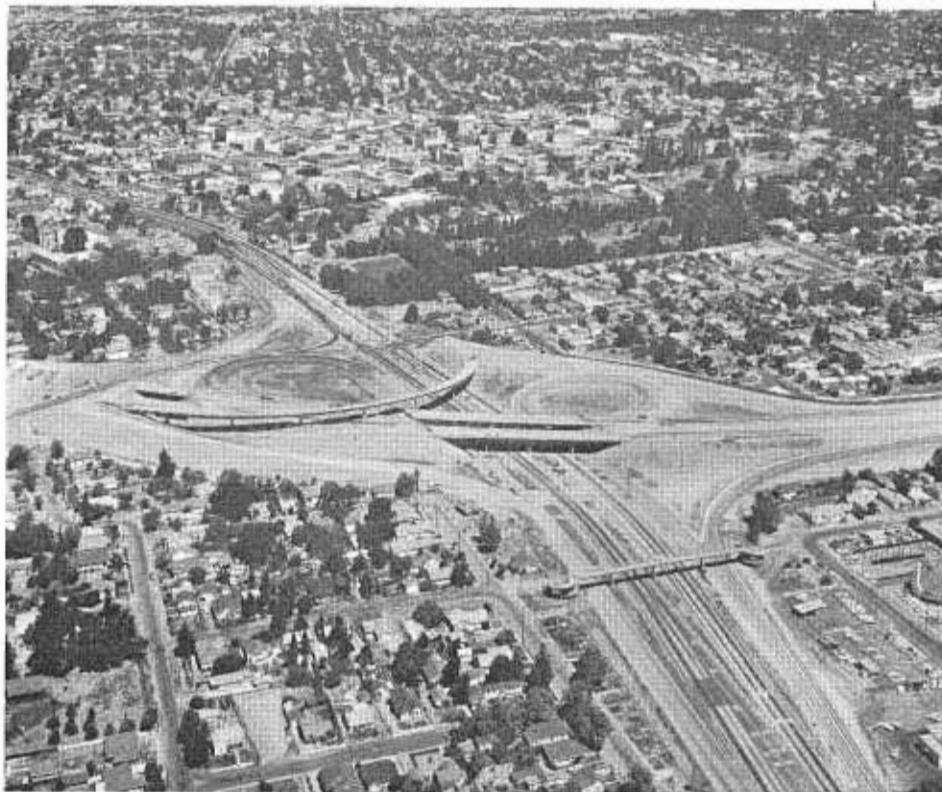
Photo shows the new three-level interchange of Routes 101 and 12 in Santa Rosa. The Earle Street Pedestrian Overcrossing is in the foreground.
