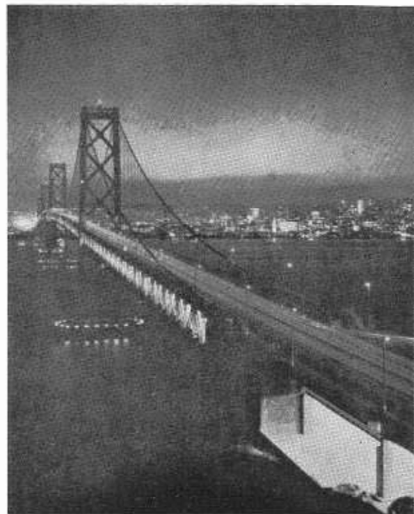
FRONT COVER: One way to illustrate the new traffic flow on the remodeled San Francisco-Oakland Bay Bridge is to photograph it at night. Westbound traffic on the upper deck shows only its tail lights, while the lower deck is illuminated by the headlights of eastbound cars. Bright area lower right was once occupied by commute train rails. See "Bay Area Report," page 24. (Photo by Bill Ruland.)
