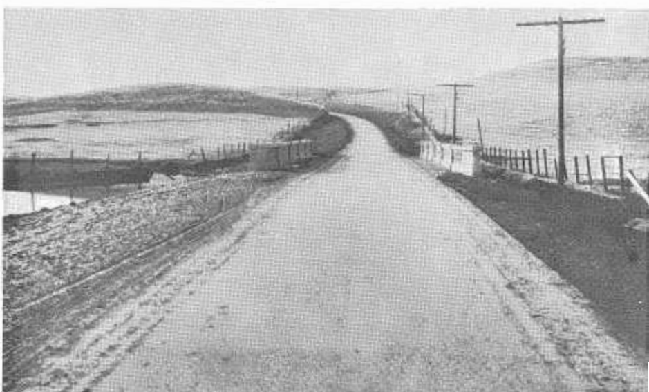
ABOVE: Same view taken three years later. The roadbed was graded and a portland cement concrete slab 15 feet wide and 6 inches thick was installed. This pavement remained in use for 30 years. In 1949 when Highway 16 was realigned, this section was abandoned but not obliterated. Today a portion serves as an access road to the famous old landmark, Sloughhouse. BELOW: Easter Sunday, 1964, 45 years after the pavement was placed. The group in the background is enjoying an old fashioned Easter egg hunt.
