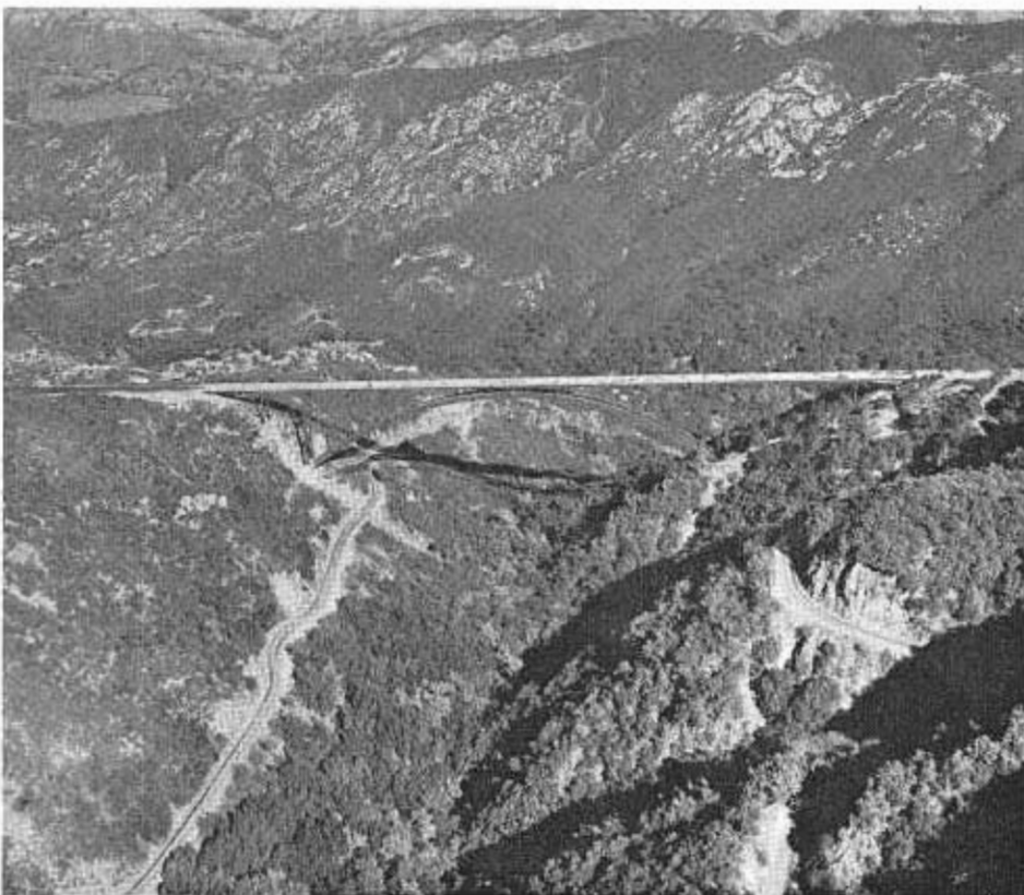
A view of the Cold Springs Canyon Bridge when nearly completed, showing the alignment of the old road beneath.
