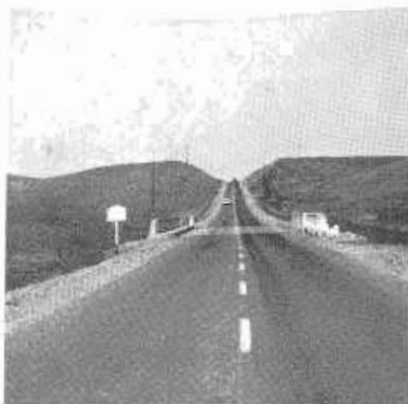
State Sign Route 16 as it looks today. The present highway was realigned several hundred feet to the north of the original route in 1949, eliminating the curves, and reducing the steep grade by cutting through the hill in the background. Note that this hill is visible to the right in the older photographs.
