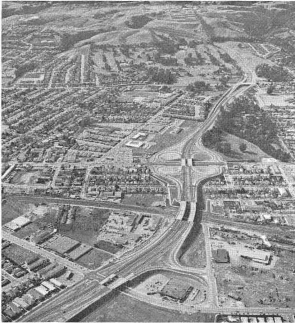
Aerial view of the completed four-lane elevated freeway through the City of San Mateo on Route 92 looks west showing the cloverleaf interchange with Route 82, El Camino Real, in the center.
