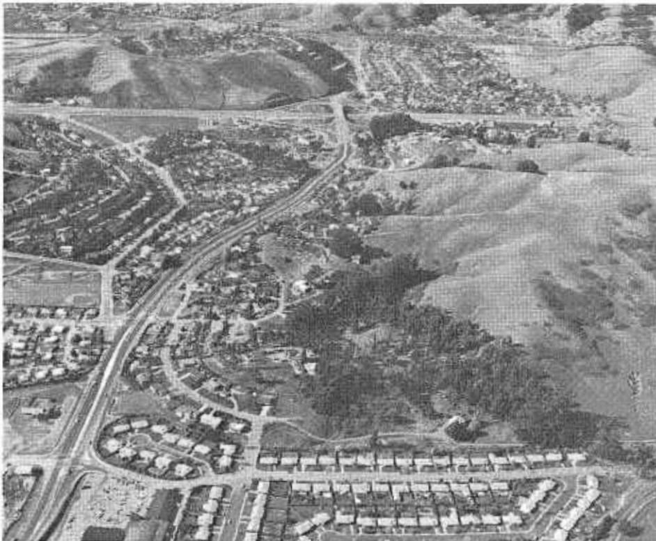
Aerial view of the recently completed section of Route 131, Tiburon Boulevard, looks west to the Alto Wye Interchange at Route 101.
