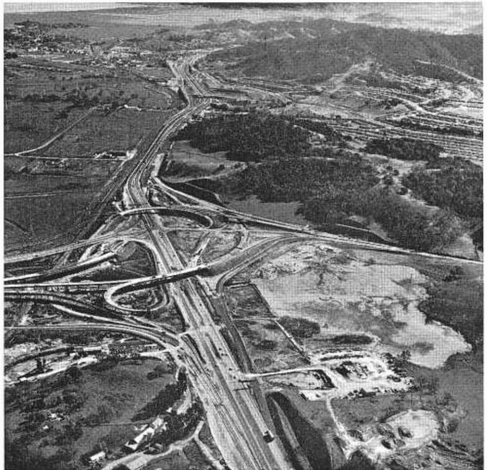
This view of the Ignacio Wye Interchange project on Route 101, the Redwood Highway, at Route 37 looks southerly toward Hamilton Air Force Base.
