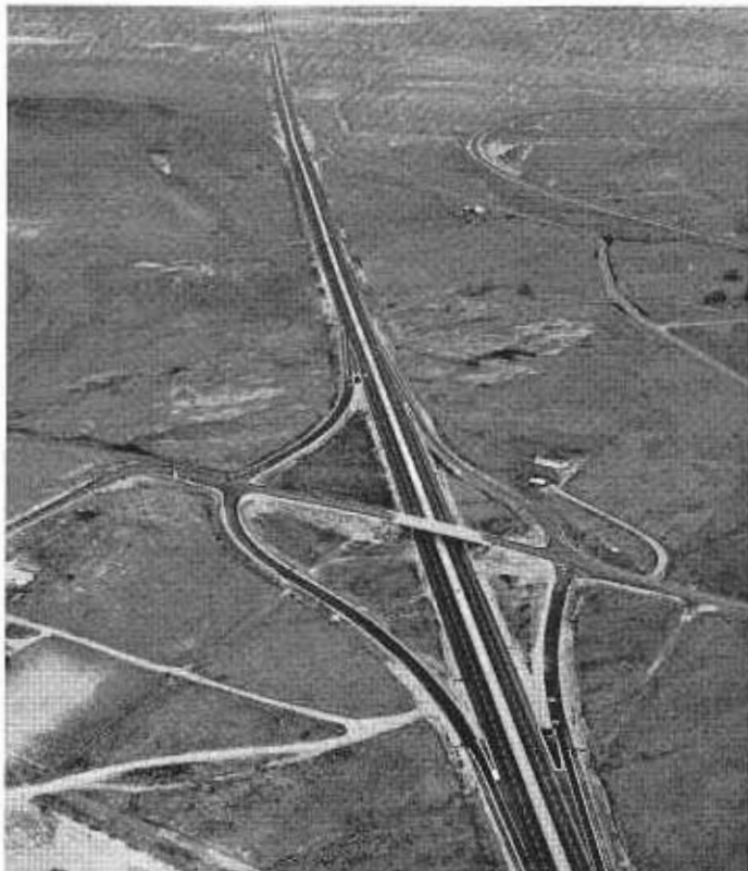
Aerial of the Garden Avenue interchange about one mile northwest of Oroville. The old Oroville-Chico road is at right as is a loop of the relocated Western Pacific railroad. Wicks Corner in upper center background.
