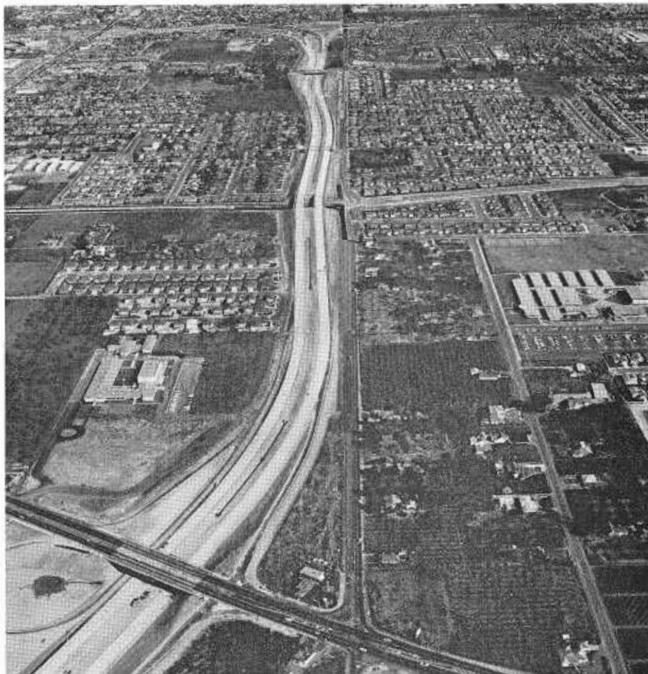
Aerial view looks east at a section of Interstate Route 280 which was opened to traffic on March 16, 1964. The Saratoga Avenue Interchange is shown in the foreground.
