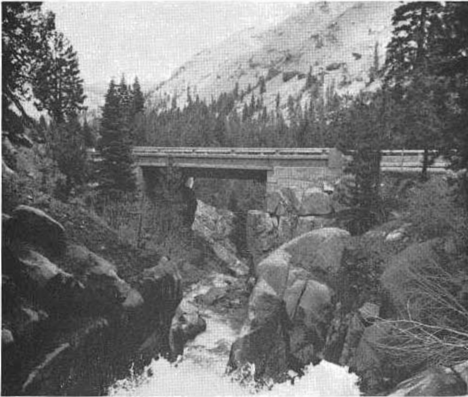
The new concrete bridge across Raymond Meadow Creek on Route 4 in the rugged terrain of Alpine County.
