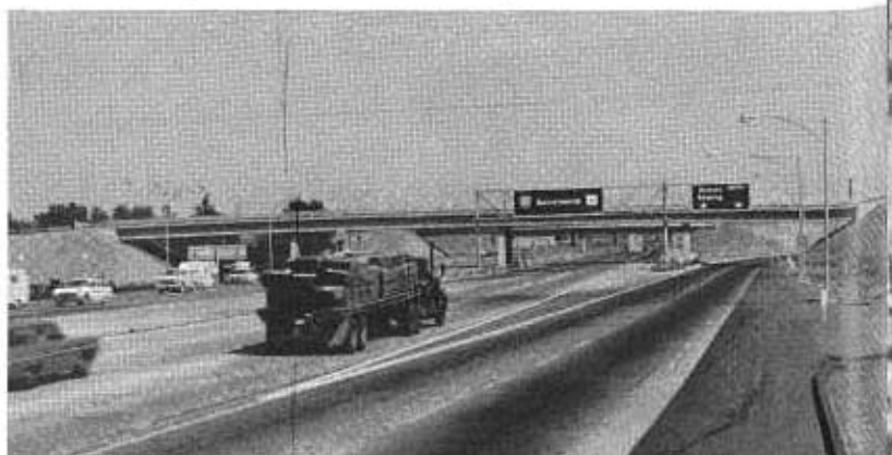
Shown is part of a recently completed 5.1-mile freeway section on Interstate 80 between Vacaville and northeast of Route 505 in Solano County. Another 7.1 miles of this route southwest of Vacaville will be converted from four-lane expressway to six-lane freeway by the end of 1965, and a 3.7-mile six-lane freeway northeast of Route 505 will be opened to traffic next fall.
