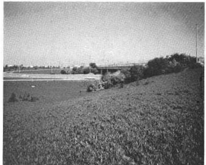
Good contour grading combined with simplicity in planting design provide effective landscaping at the interchange of the Nimitz Freeway (Route 17) with Route 92 near Hayward.
