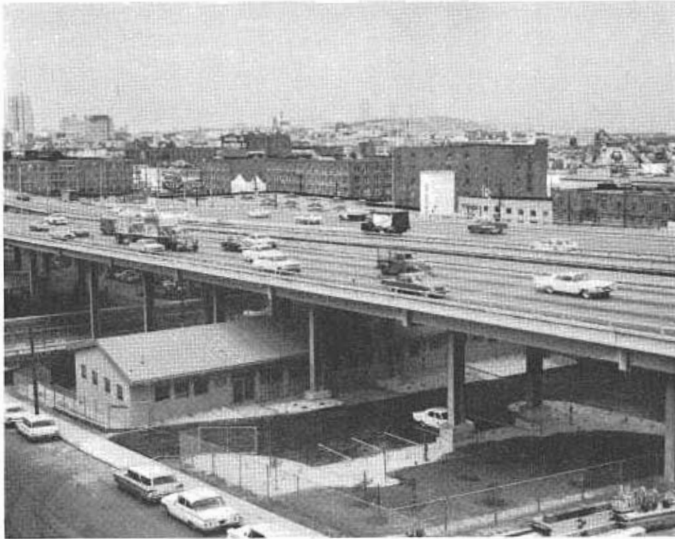
District 4's unique new materials laboratory, constructed under the James Lick Memorial Freeway in San Francisco, is well equipped to handle the large volumes of samples that must be tested.
