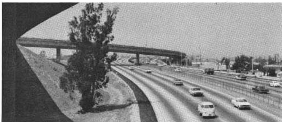
The Santa Monica-San Diego Freeway interchange in Los Angeles. The view is northward along the San Diego Freeway.
