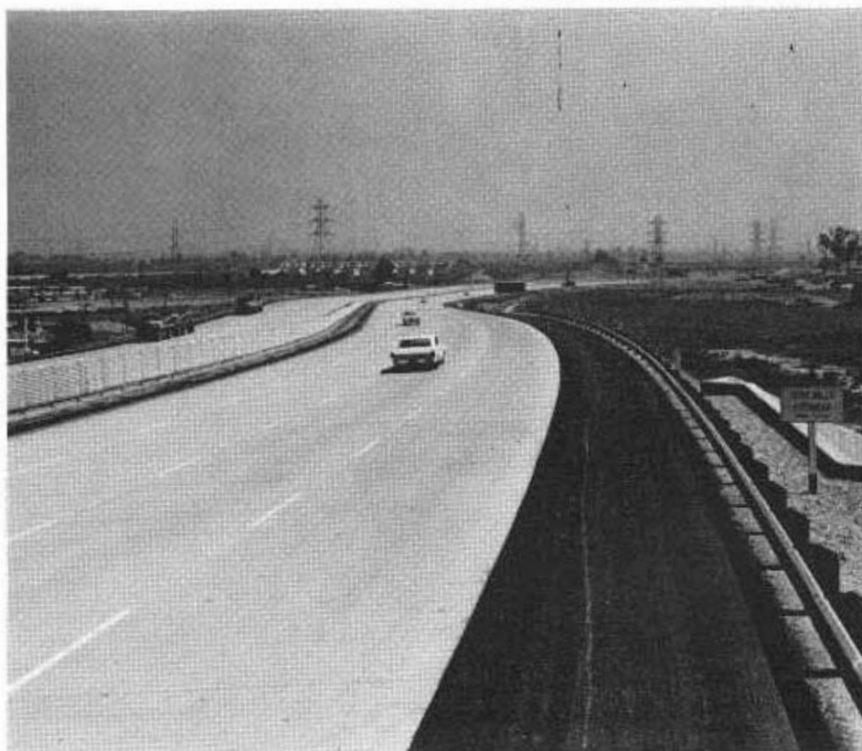
Looking north along a recently opened section of Interstate 605 north of Whittier. Median barrier is supplemented by aluminum glare shield.
