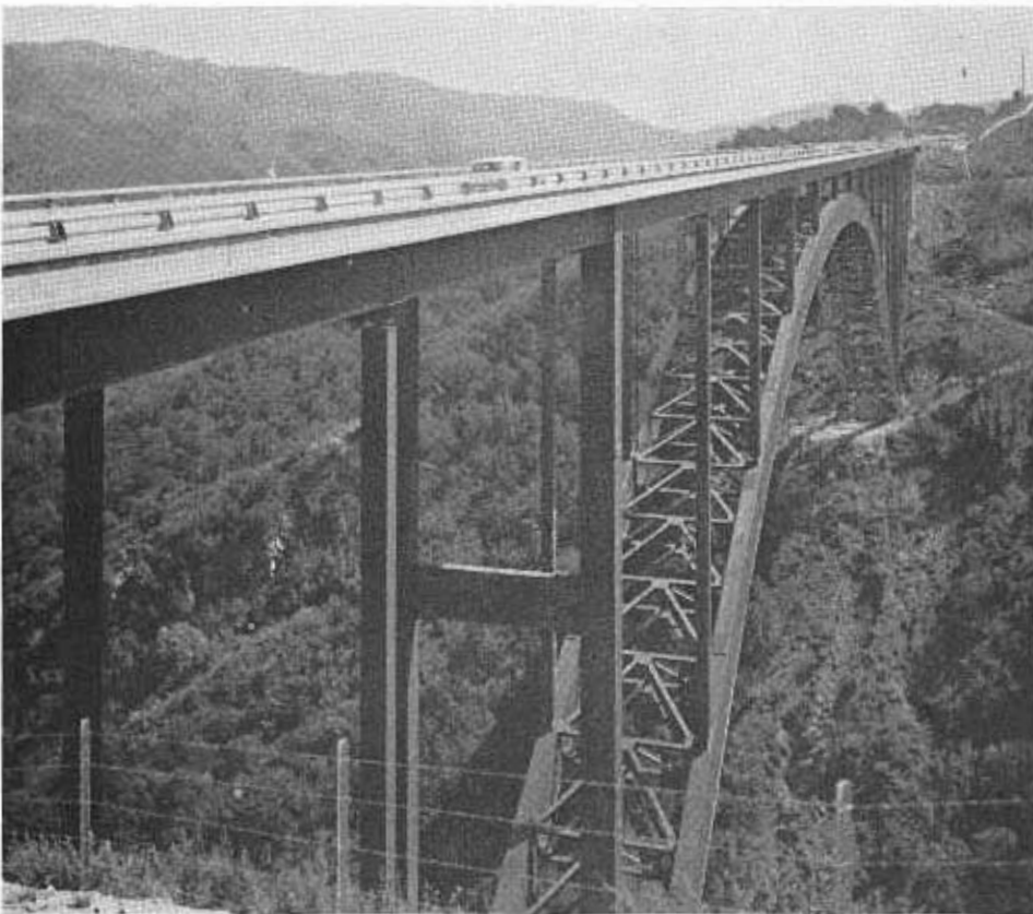
The 700-foot steel arch span across Cold Springs Canyon on Route 154 between Santa Barbara and Santa Ynez.
