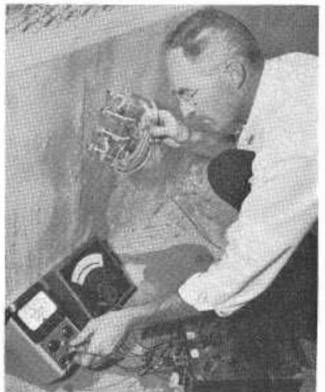
The electrical resistivity of concrete is measured to determine the relative conditions of corrosion potential to reinforcing steel by this instrument developed by the Materials and Research Laboratory.
