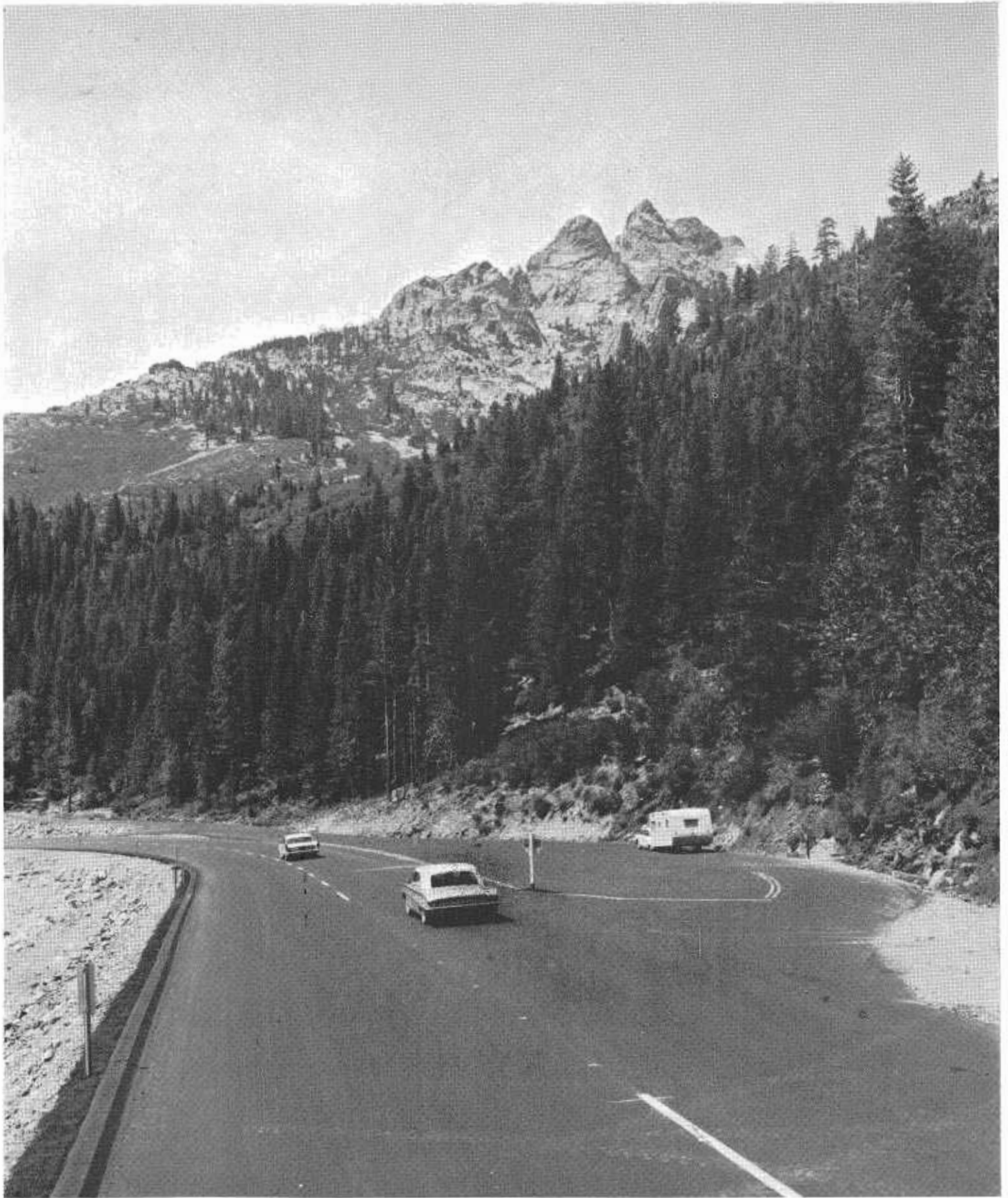
A safety roadside rest on the two-lane Route 49 expressway east of Sierra City in Sierra County. It is one of 24 such facilities throughout the state now used by motorists. Seven more are under construction and work is scheduled to begin on an additional 26 in 1965.
