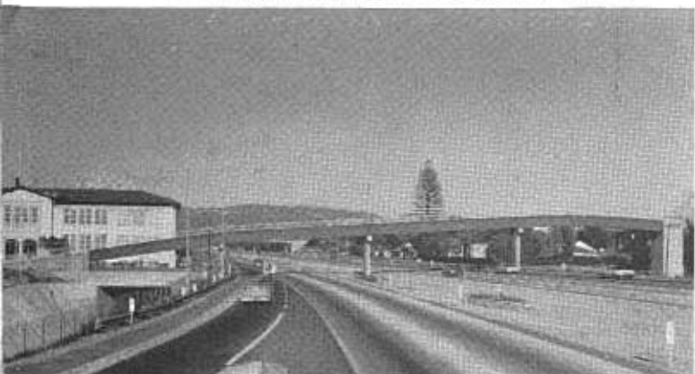
Construction of the US 101 Freeway in the City of Santa Barbara, completed last January, was complicated by the proximity of a railroad (at left), Mission Creek (at right of the freeway fence) and Wilson School.
