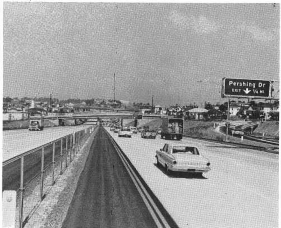
A section of Interstate 5 in the City of San Diego, with steel cable barrier in the median.
