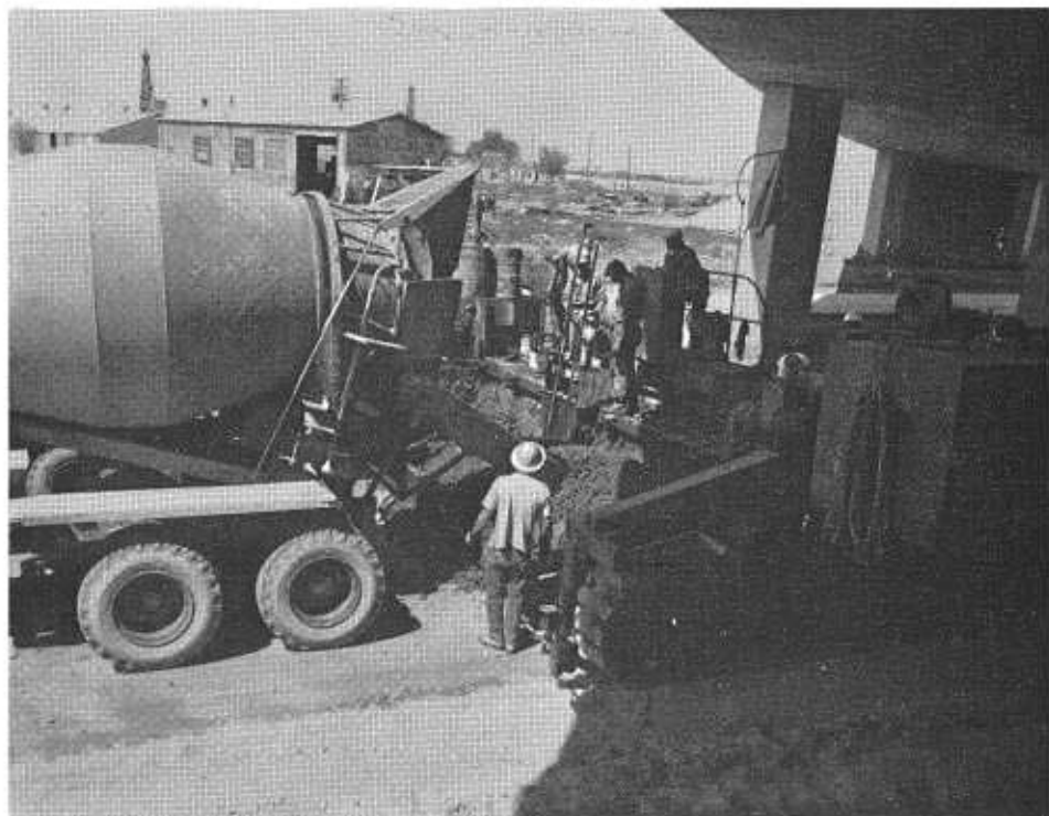
Placing 24-foot-wide portland cement concrete highway pavements with an automatically controlled slip form paver. At top, end-dump truck delivers concrete mixed in a stationary tilt-drum central mix plant away from the construction scene. At bottom, tilt-drum truck paving mixers deliver concrete mixed in transit to the job site.
