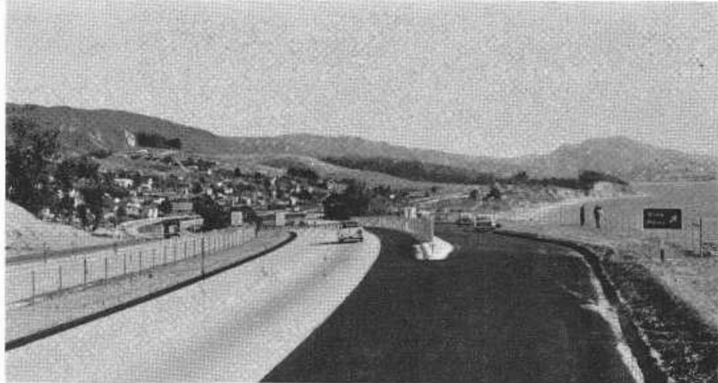
One of the illustrations in a recent manual of design standards for scenic highways, this photograph of US 101 at Ortega Hill east of Santa Barbara shows how turnouts may be provided for vista points at suitable locations.
