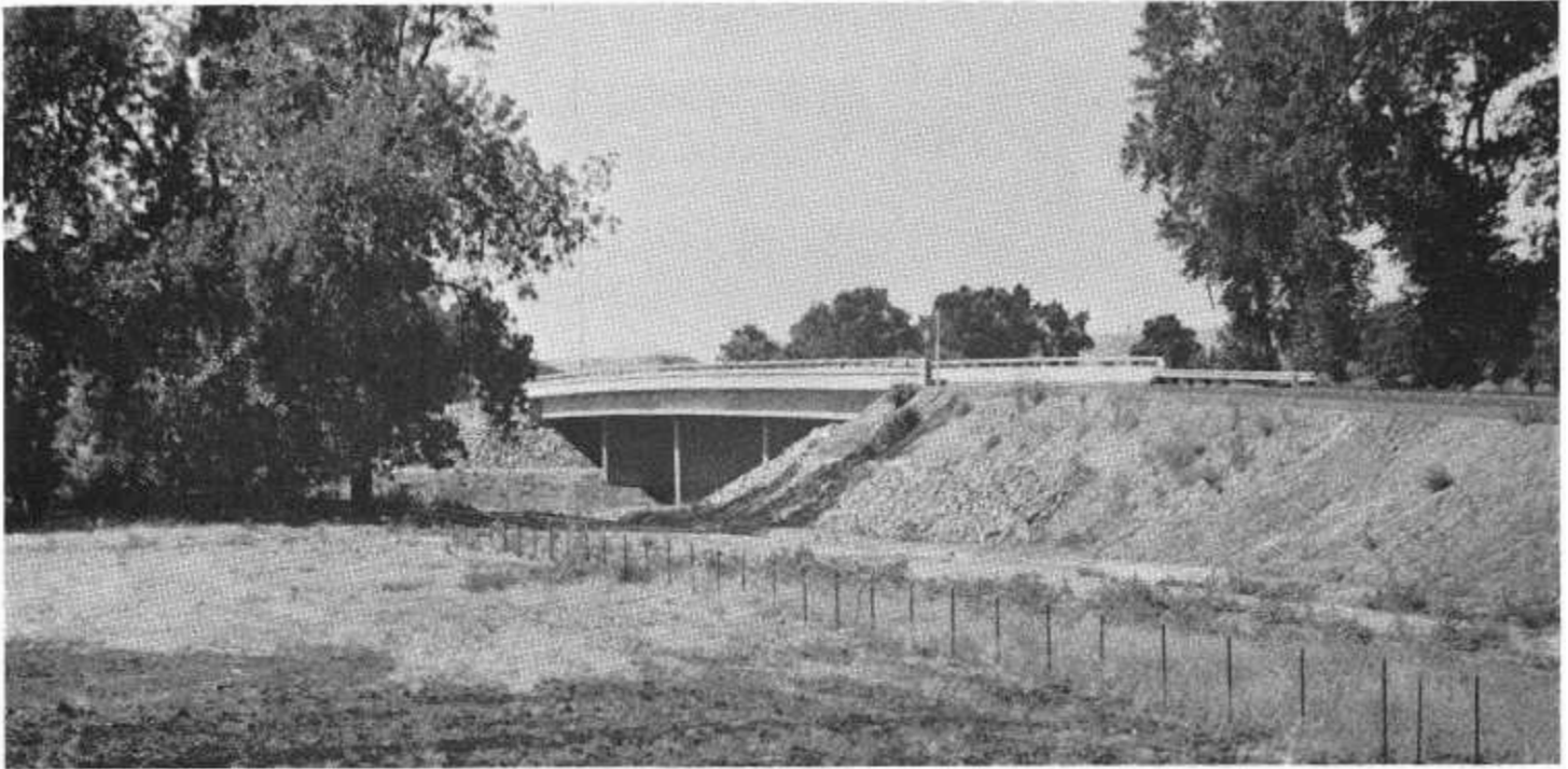
This new bridge across the Cosumnes River near Sloughouse in Sacramento County was built with federal aid secondary funds, replacing an old steel truss span built in 1906.
