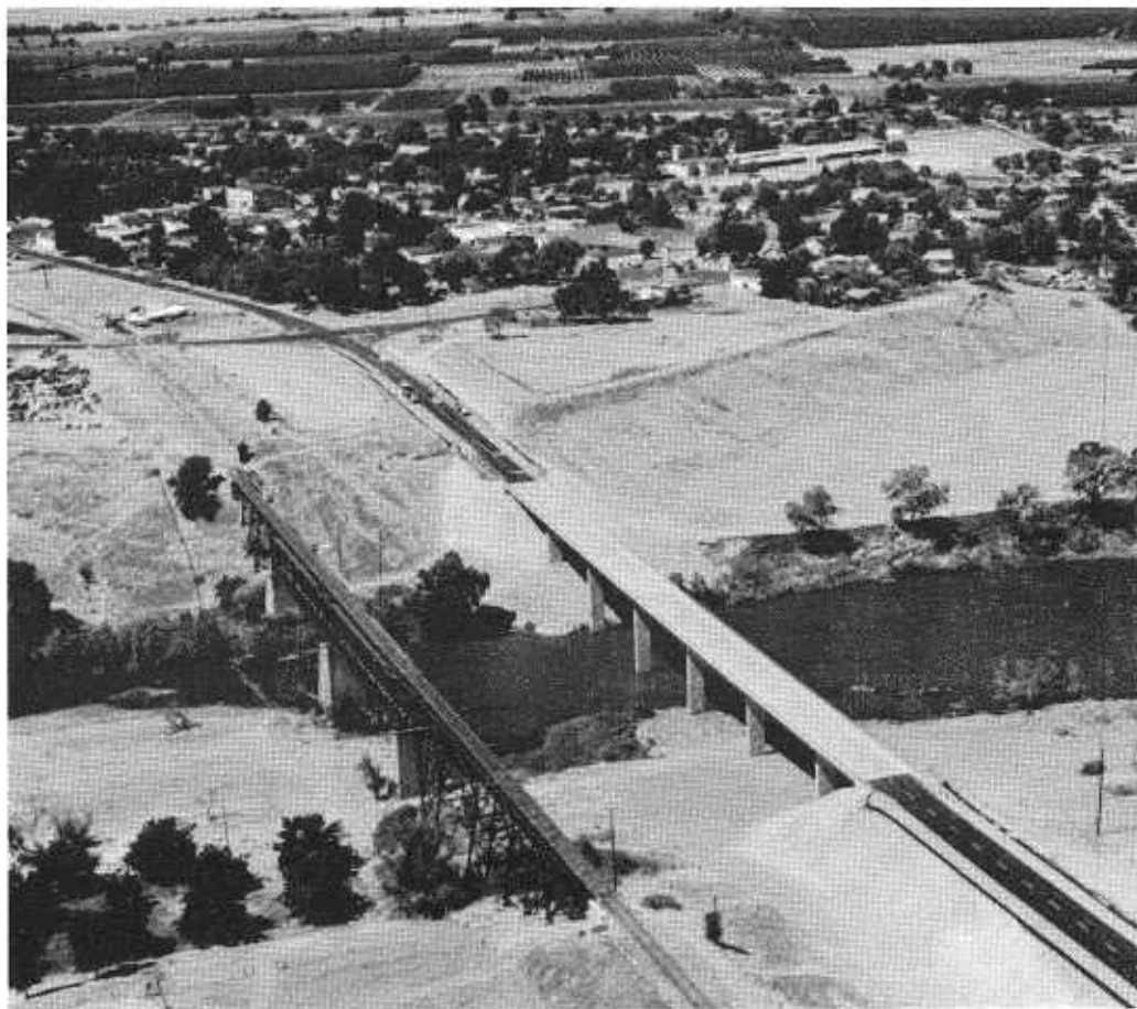
Bridge (right) was constructed on new alignment over the Tuolumne River near Waterford by Stanislaus County under the federal aid secondary program. It replaces a bridge built in 1914 which is now inadequate for present day traffic.
