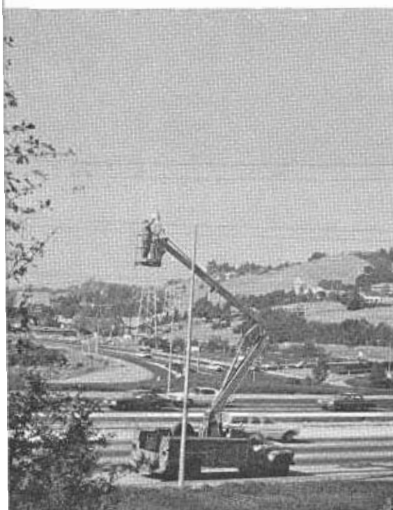
"Giraffe" is used to relamp an electrolier on freeway.
