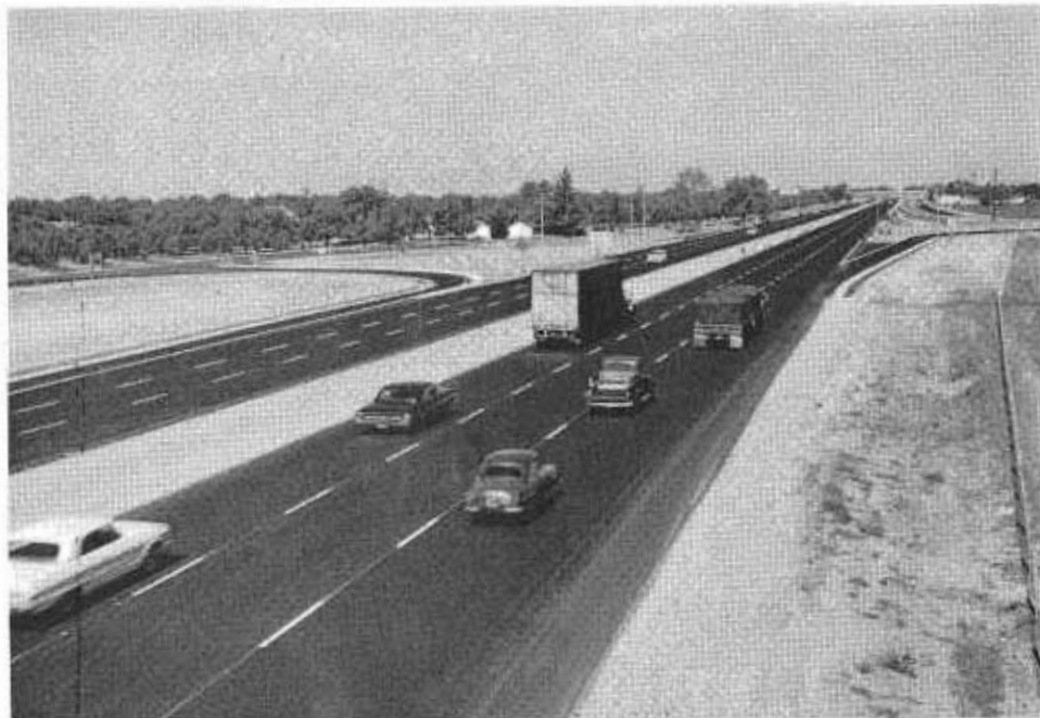
Looking northerly from the Calaveras River Overcrossing toward the Hammer Lane Overcrossing and Lodi on the new freeway between Stockton and Lodi.
