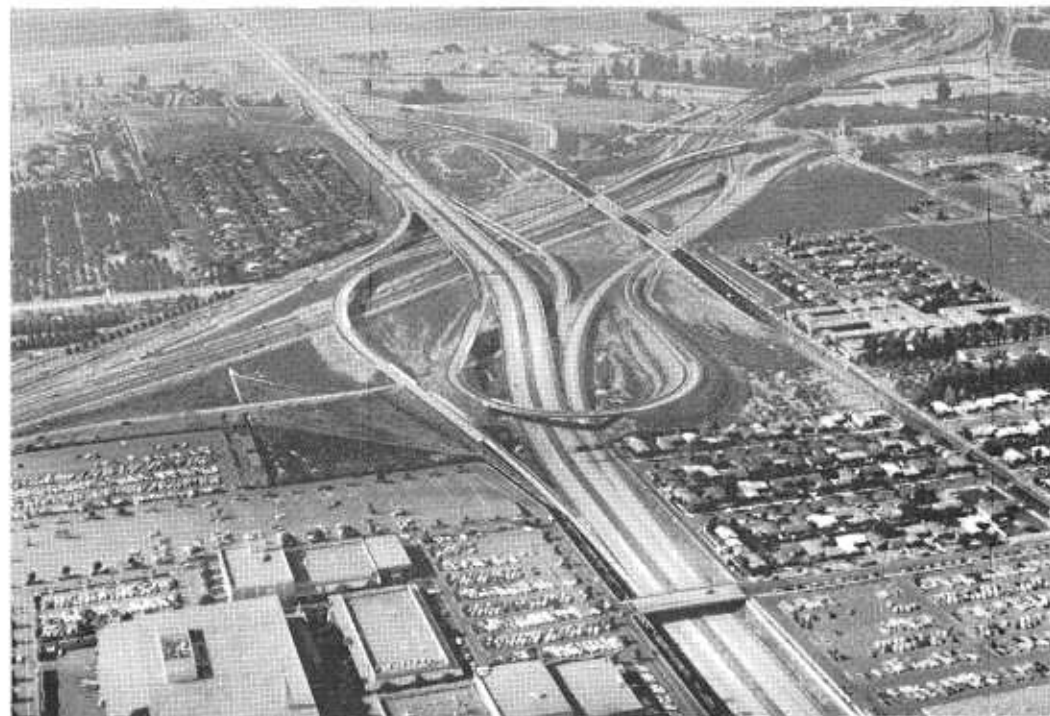
The interchange between the Garden Grove (Route 22) Freeway (upper) and the Interstate 5 (Santa Ana) Freeway in the Orange-Santa Ana area was completed in September. The former freeway is now under construction between the Santa Ana and the Interstate 405 (San Diego) Freeways.
