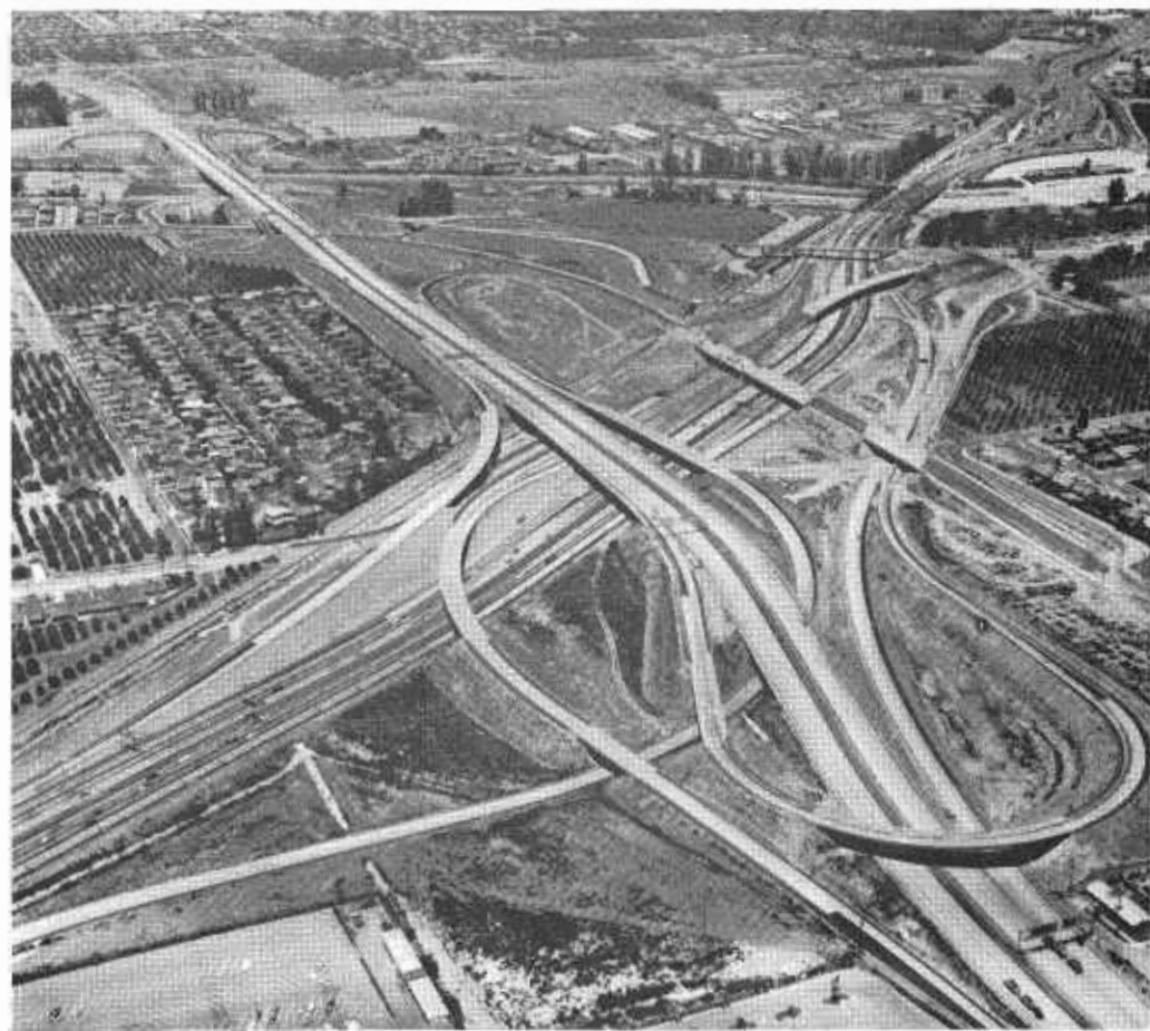
Looking west along the Garden Grove Freeway at the interchange which carries it over the Santa Ana Freeway.
