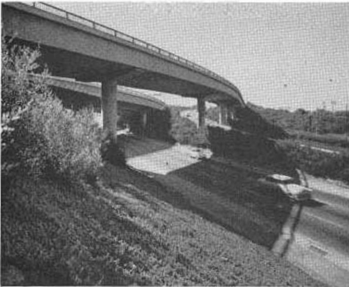
The interchange of the Santa Ana and Long Beach Freeways in Los Angeles illustrates the dual role of low-maintenance shrubs and ground cover to control erosion on slopes and to complement bridge structures.
