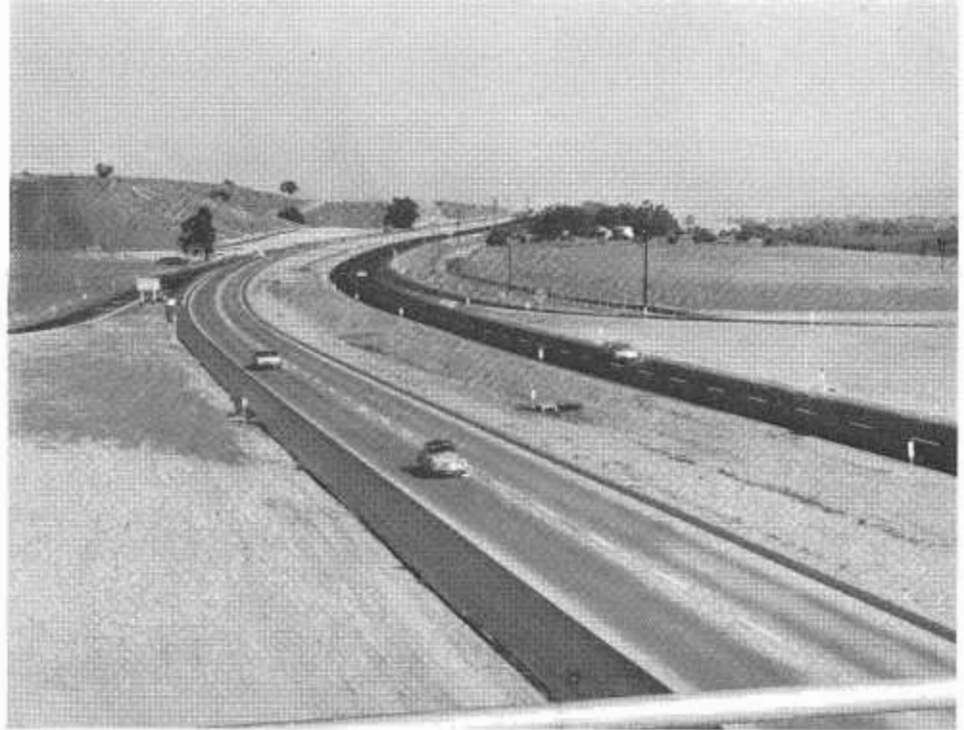
Shown is a portion of the 11.3-mile freeway section of US 101 between south of San Ardo and north of Bradley in Monterey County which was completed in August. This section connects on the south with a 6.7-mile freeway project, which will be opened to traffic next fall. The latter, in turn, connects with a recently completed 4.8-mile freeway section extending to north of San Miguel in San Luis Obispo County.
