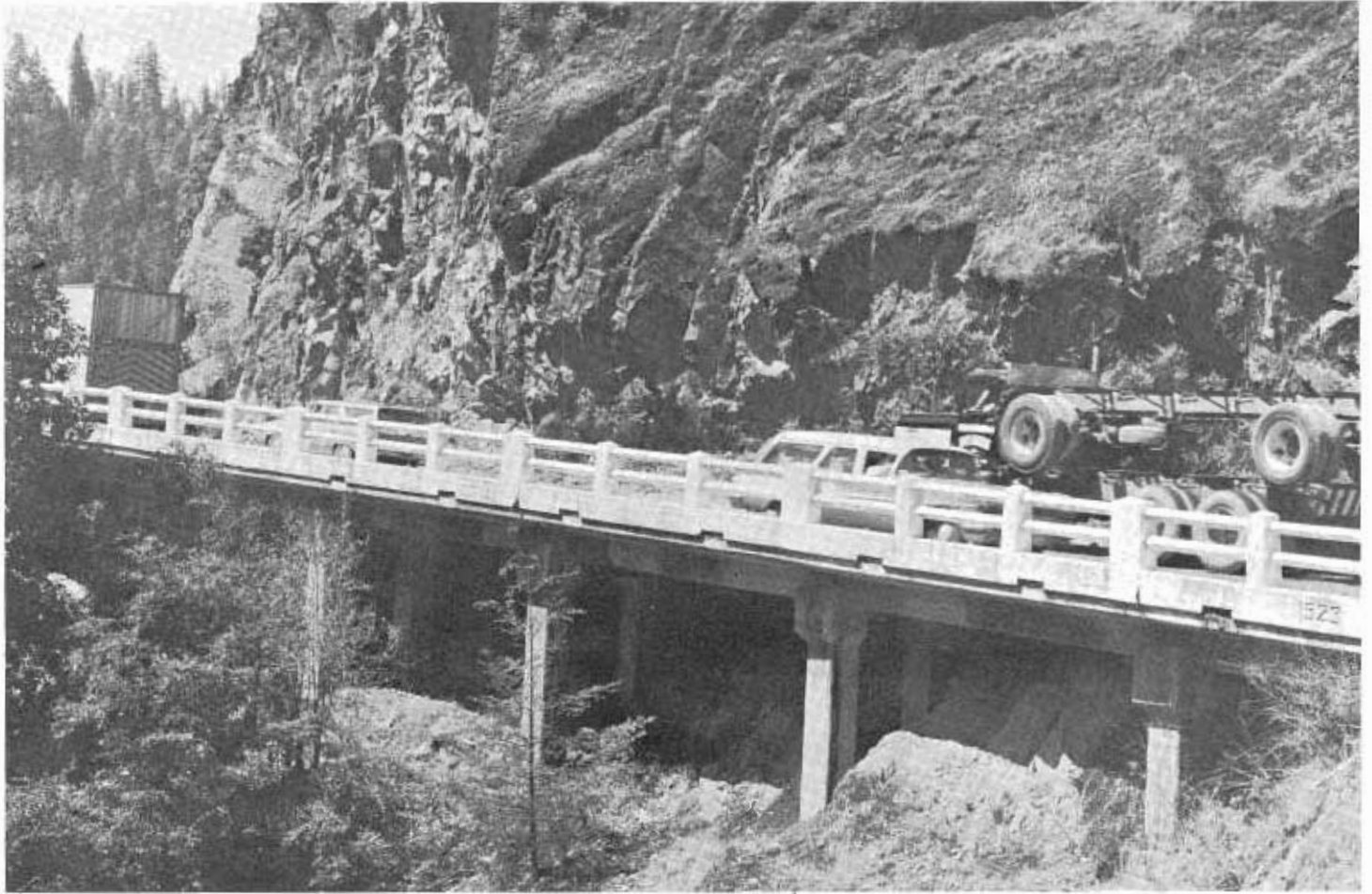
Motorists negotiating this narrow viaduct built into the steep terrain in northern Mendocino County can't see the "1923" date on the structure, but it wouldn't surprise them.
