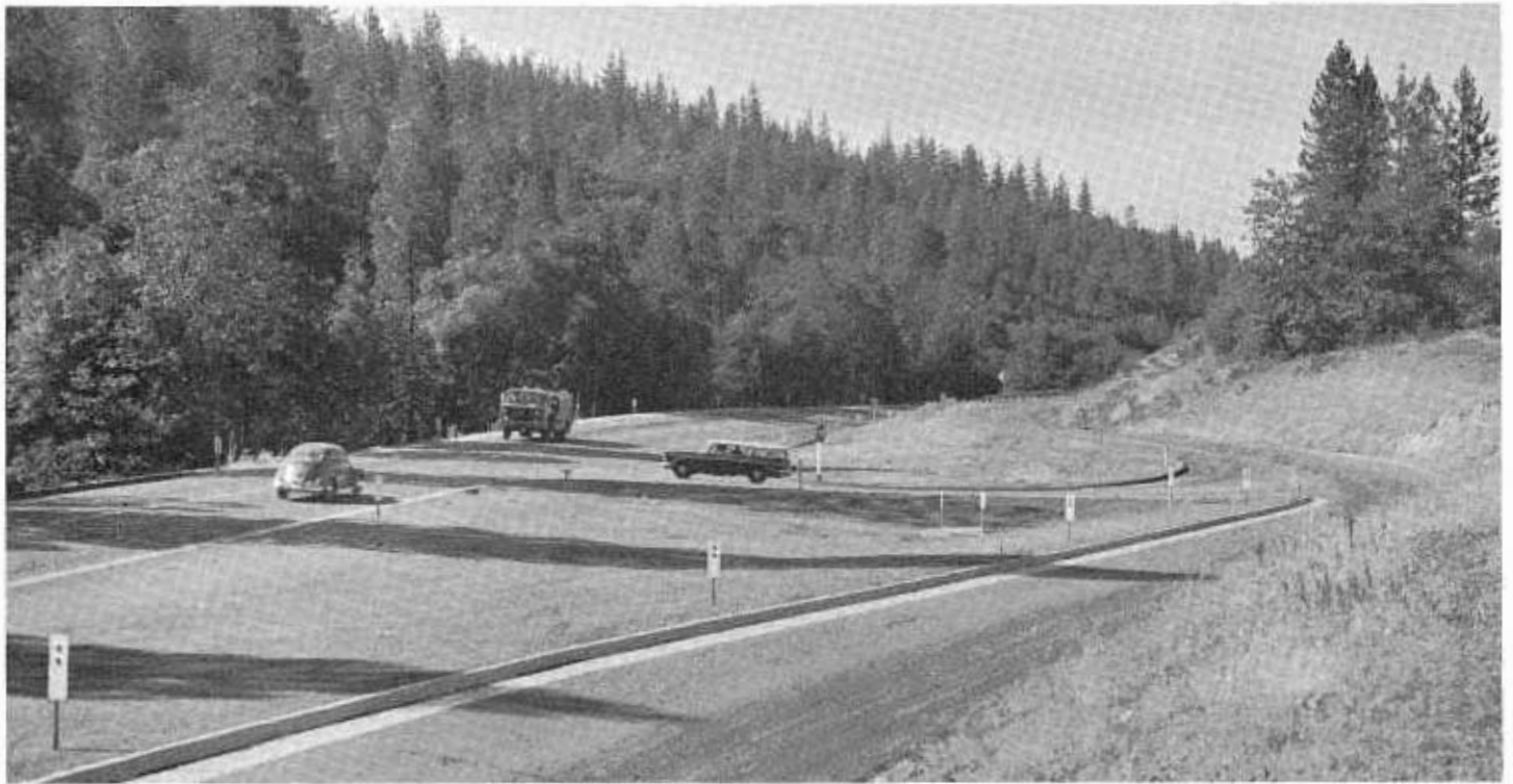
The once hazardous junction of Climax Road and Highway 88 has been made safer by channelization and widening.
