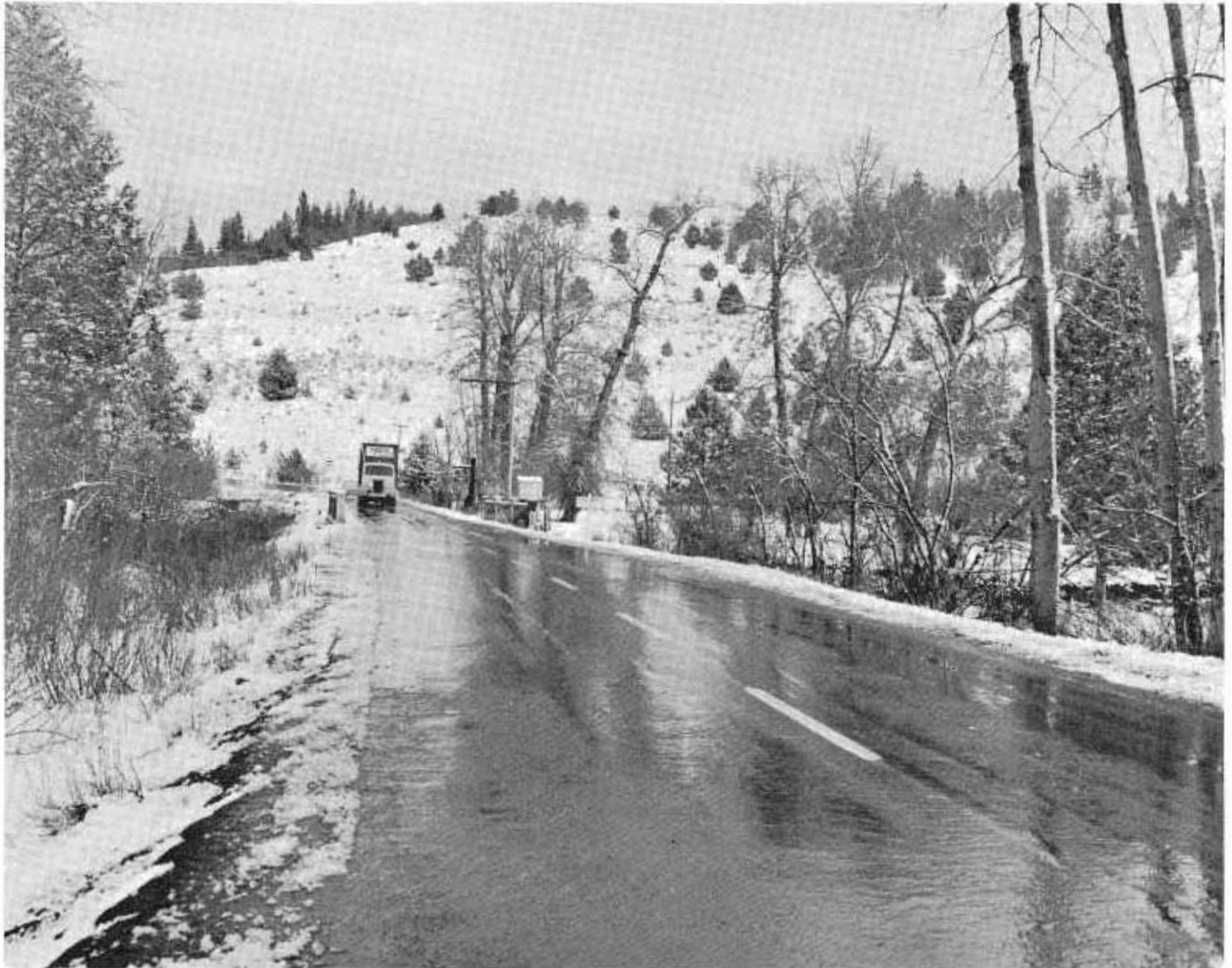
A winter view of Route 299 at Rush Creek before reconstruction.
