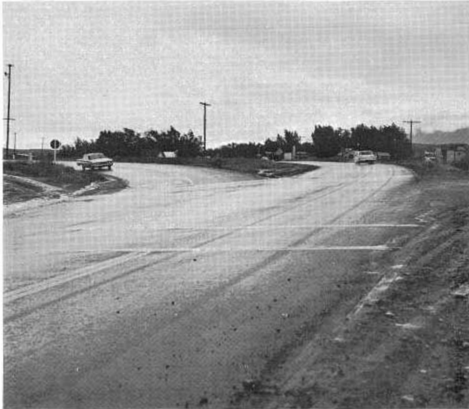
BEFORE. The old intersection of Routes 36 and 395 prior to relocation.
