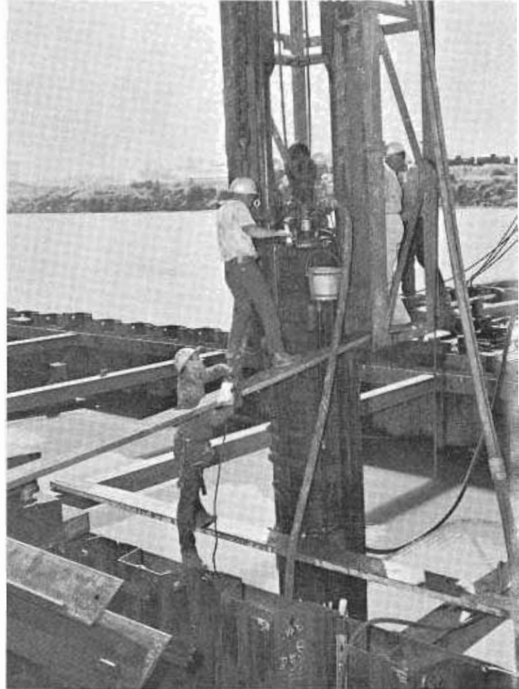
PHOTO ABOVE—An underwater hammer used for driving foundation piles to 35 tons of bearing value per pile. PHOTO BELOW—Driving 50-foot timber piles with underwater hammer.
