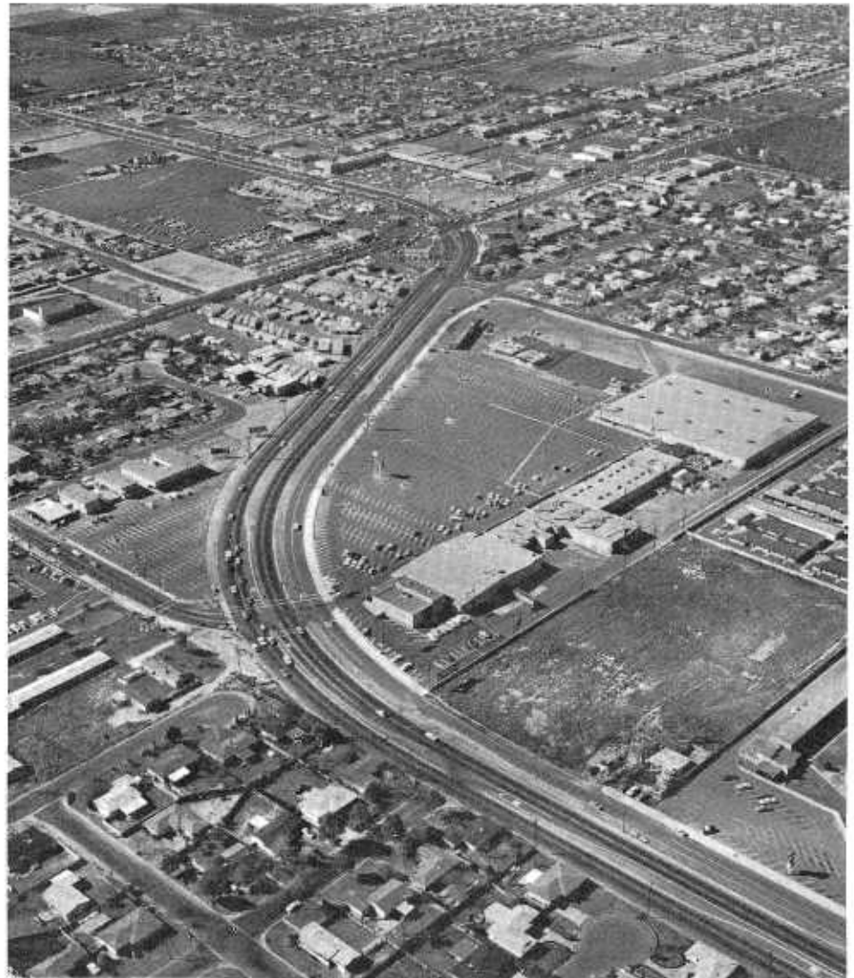
Harbor Boulevard reconstruction looking southwest. Garden Grove Boulevard crosses Harbor Boulevard at an angle in the middleground. The shopping center in the foreground is served by a frontage road. Access is provided by a signalized intersection with a public street (foreground).
