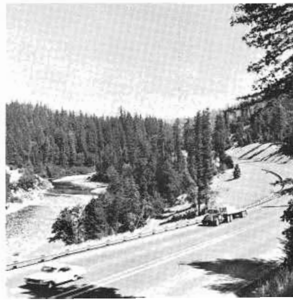
BACK COVER: The recently completed US 101 Freeway about a mile south of Myers Flat passes near the Lansdale Bar recreation area on the Eel River. The Avenue of the Giants, which the freeway has replaced as a through route, is visible in the left center of the picture. (Photo by John Meyerpeter.)
