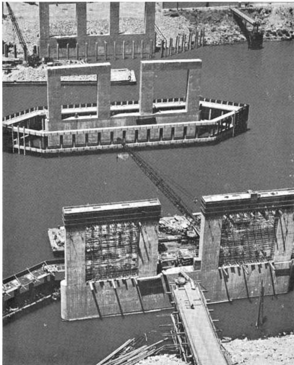
PHOTO ABOVE—Final stages of pier construction. At Pier No. 1 (background) rock riprap is being placed. Center pier is complete except for treated timber sheeting being placed at the near side. At Pier No. 3 (foreground) the fender system is being constructed. Photo by Sacramento Bee. PHOTO BELOW—Looking downstream and across the Sacramento River to Yolo County at the nearly completed substructure of the bridge.
