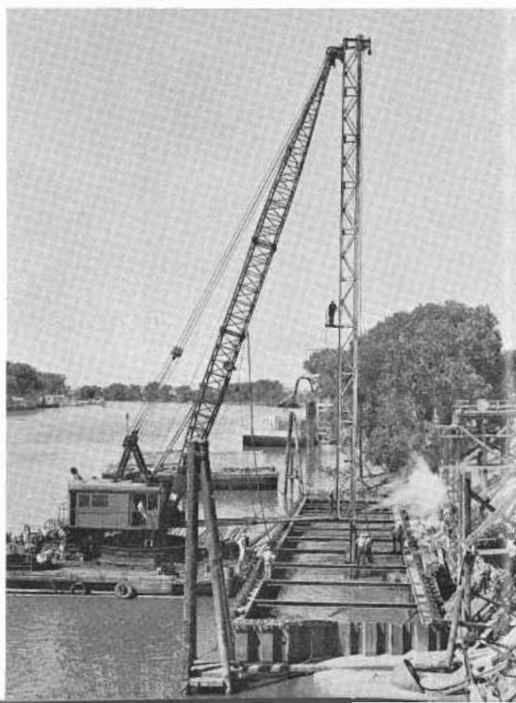
PHOTO ABOVE—An underwater hammer used for driving foundation piles to 35 tons of bearing value per pile. PHOTO BELOW—Driving 50-foot timber piles with underwater hammer.
