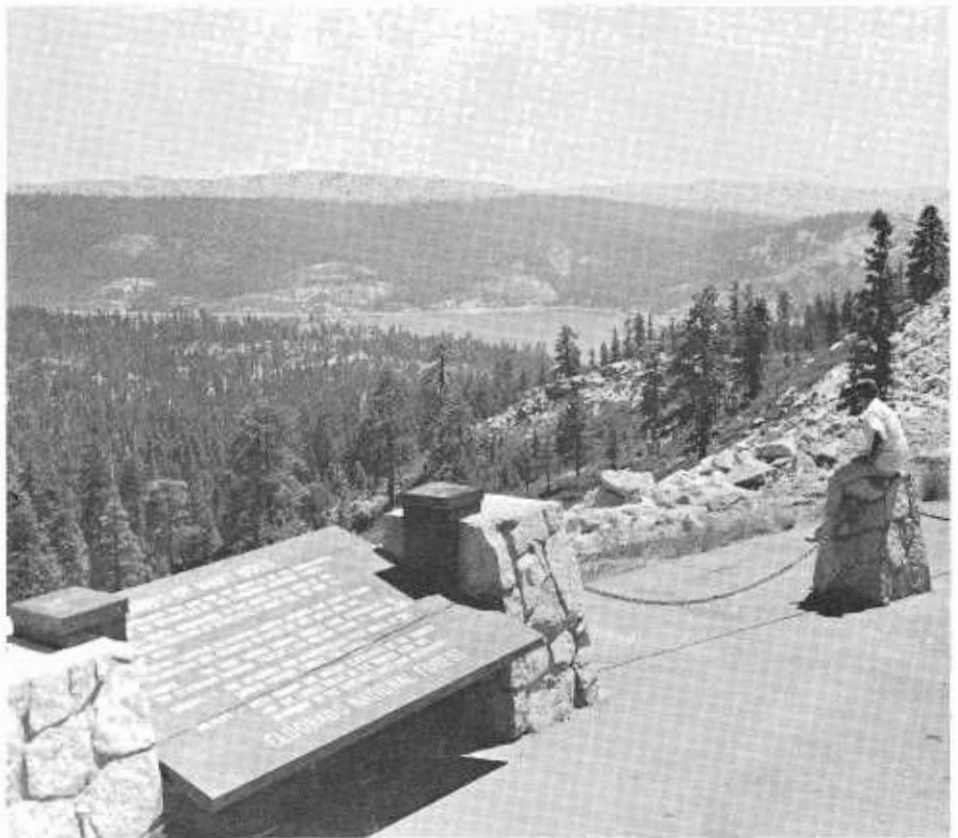
The Bear River Reservoir viewed from the U.S. Forest Service vista point at Peddler Hill.
