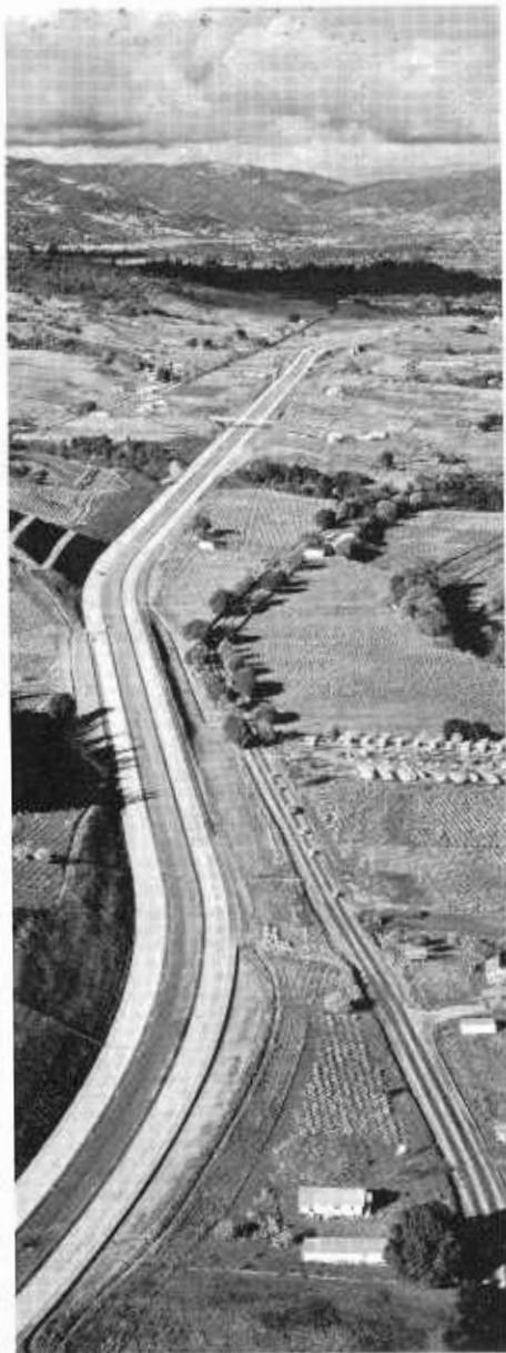
Aerial view of new freeway section just north of Ukiah, looking north along the Russian River valley toward Ridgewood Summit.
