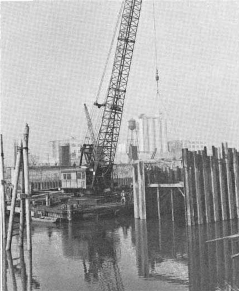
PHOTO ABOVE—Final stages of closing the sheet pile cofferdam (Sacramento side of the river). PHOTO BELOW—One of two large derrick barges lowers a 64-ton water system.
