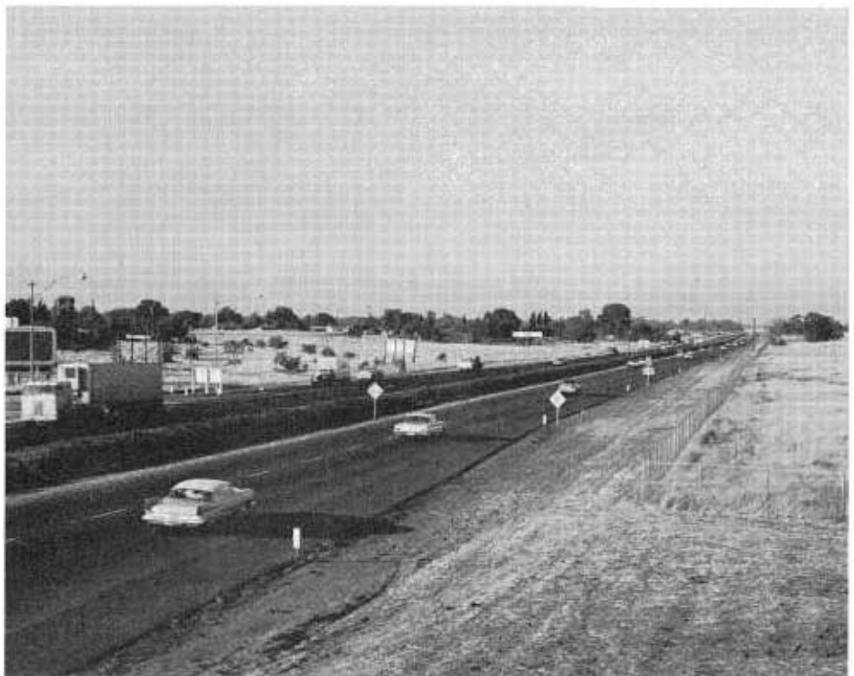
Interstate 80 (old US 40-99) north of Sacramento was the center of a case in 1949 in which the constitutionality of the freeway statute was affirmed by the State Supreme Court.
