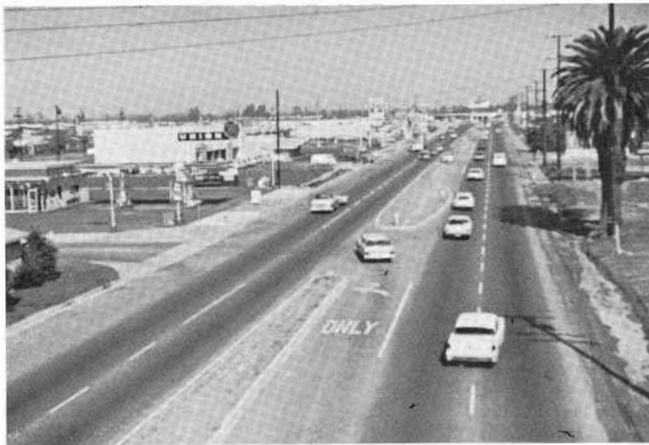
AFTER—Harbor Boulevard following improvement with divided roadways and left turn lanes. Accidents have been reduced by more than 50 percent.
