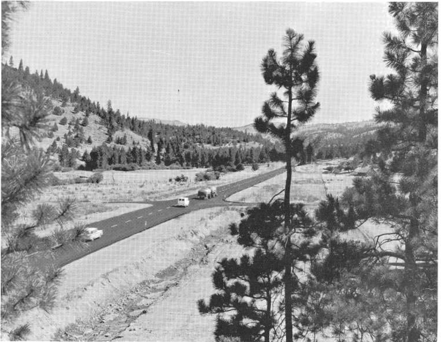
The completed expressway through this mountainous area is constructed to a design speed of 70 miles an hour.
