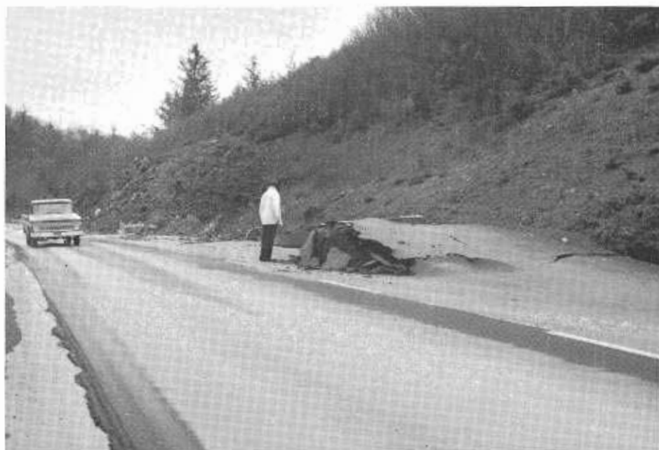
ABOVE: This paving damage was caused by pressure of sliding material on slope at right, forcing its way between road surface and foundation. BELOW: Man in photo has right hand at high-water mark which South Fork of Eel reached here near Phillippsville. This stretch of freeway, recently completed, was constructed five feet above high-water line of 1955 flood.
