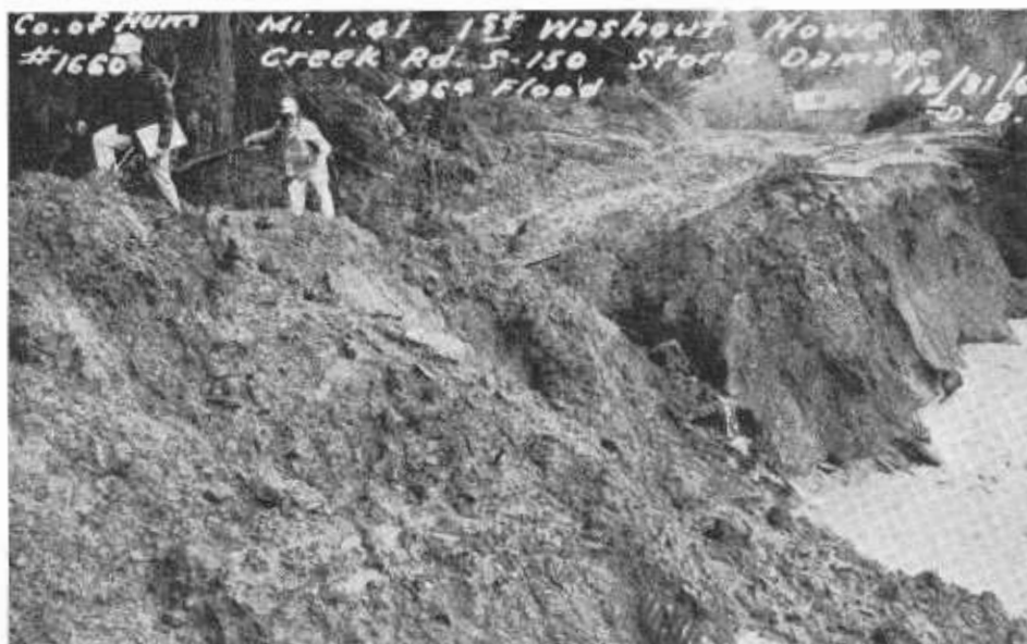
Engineers surveying damage on county road in Humboldt County, seeking route into Rio Dell, struggle through knee-deep mud along banks of the Eel River. This route is now being used temporarily as part of the Redwood Highway.
