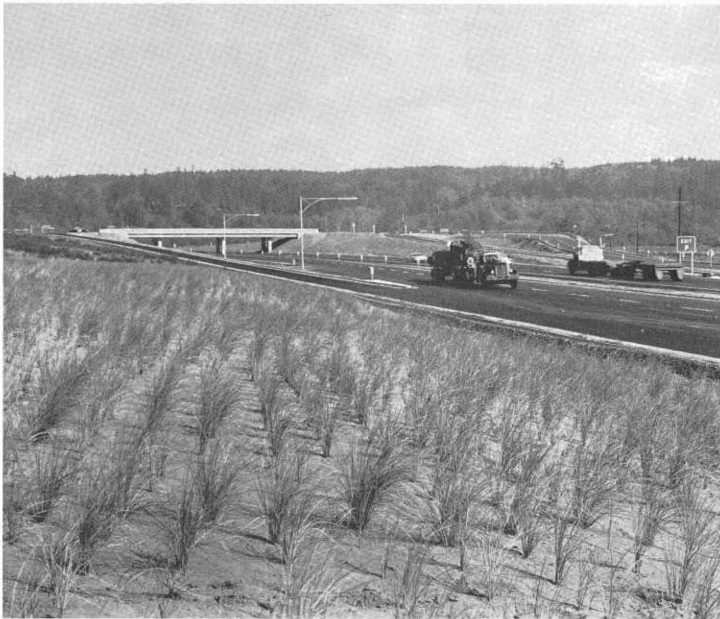
The Crannell Interchange, looking north, showing typical lumber industry truck traffic. Planting of beach grass in foreground prevents drifting sand in the dune areas.
