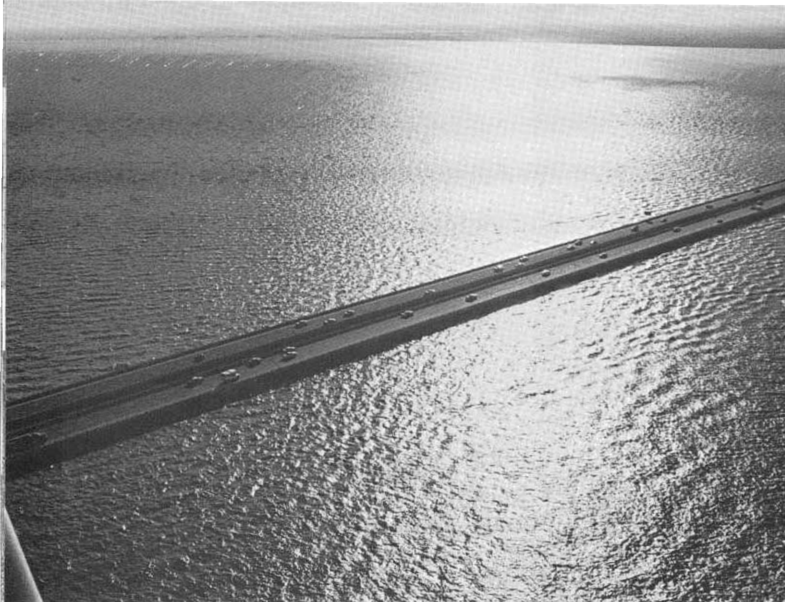
Overflow water from Sacramento River passing over weirs into Yolo Bypass during week of Christmas Flood makes Interstate 80 look like causeway to Key West. (Photo courtesy of Vernon Giles, Carmichael Times.)
