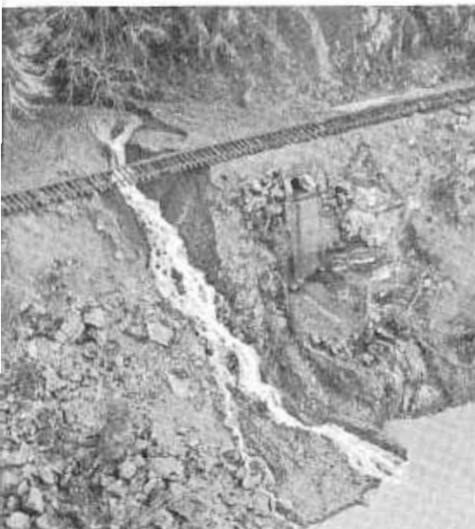
ABOVE: In this photo of roadbed destruction on Northwestern Pacific Railroad debris washed down the slope has filled the culvert and the stream has cut a new bed. (Photo courtesy of Northwestern Pacific Railroad.) BELOW: Destruction here is by slipout, or, in other words, a slide of the supporting slope below the roadbed.
