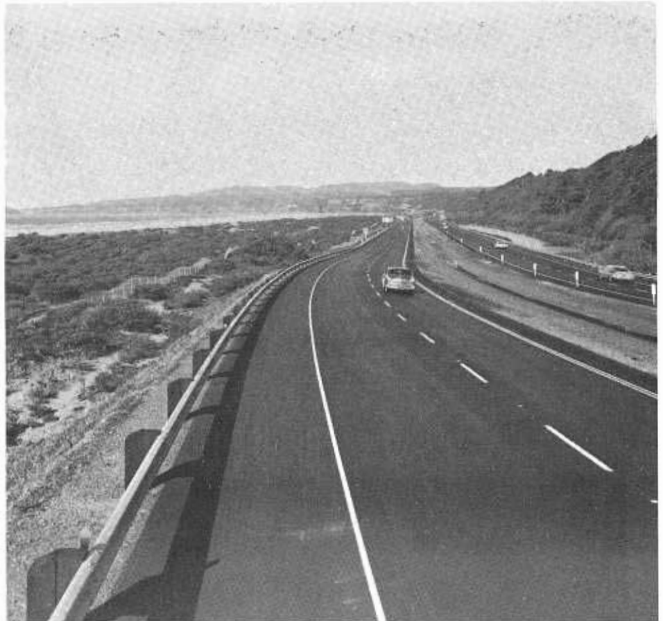
Looking north along the new McKinleyville Freeway section of US 101 in Humboldt County.
