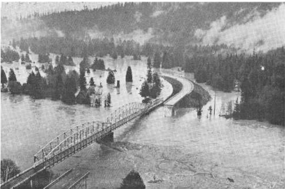
ABOVE: Debris deposited by flood on US 101 in redwood groves just upstream from Pepperwood. Barn with cupolas came from site across river and several miles upstream. BELOW: Downstream bridge of pair on Redwood Highway at South Scotia was also flood victim. Older bridge at left of through-truss design, survived flood because it was high enough to avoid debris which collected on truss below deck of newer bridge now missing at right. (Photo courtesy of Eureka Newspapers, Inc.)
