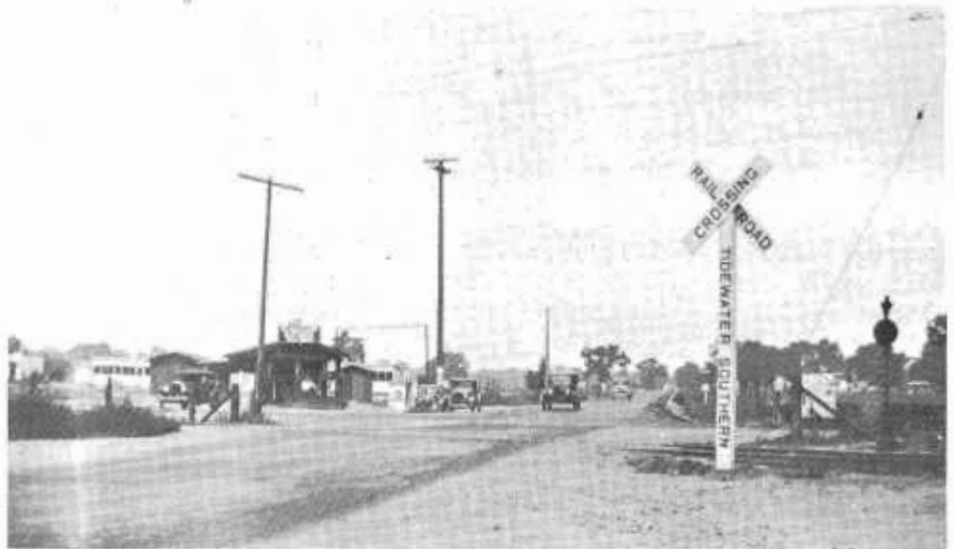
The US 99 crossing of the Tidewater Southern Railroad tracks near Turner Station in 1929, looking north.
