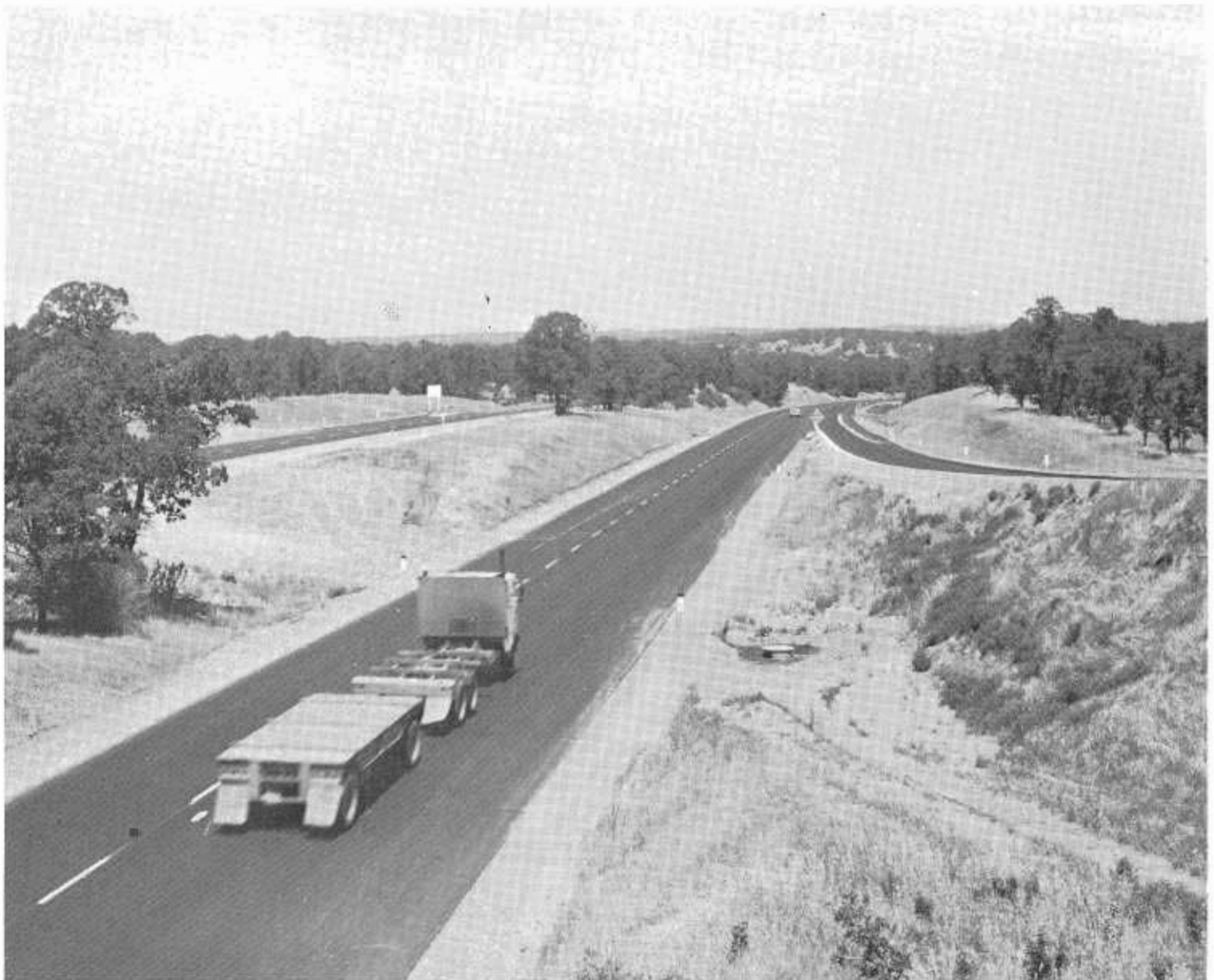
A section of the new Interstate 5 freeway near Cottonwood in Shasta County. Note the wide, contoured grading of side slopes and median with split-level roadways and trees preserved and made part of the highway picture in the wide median separator.
