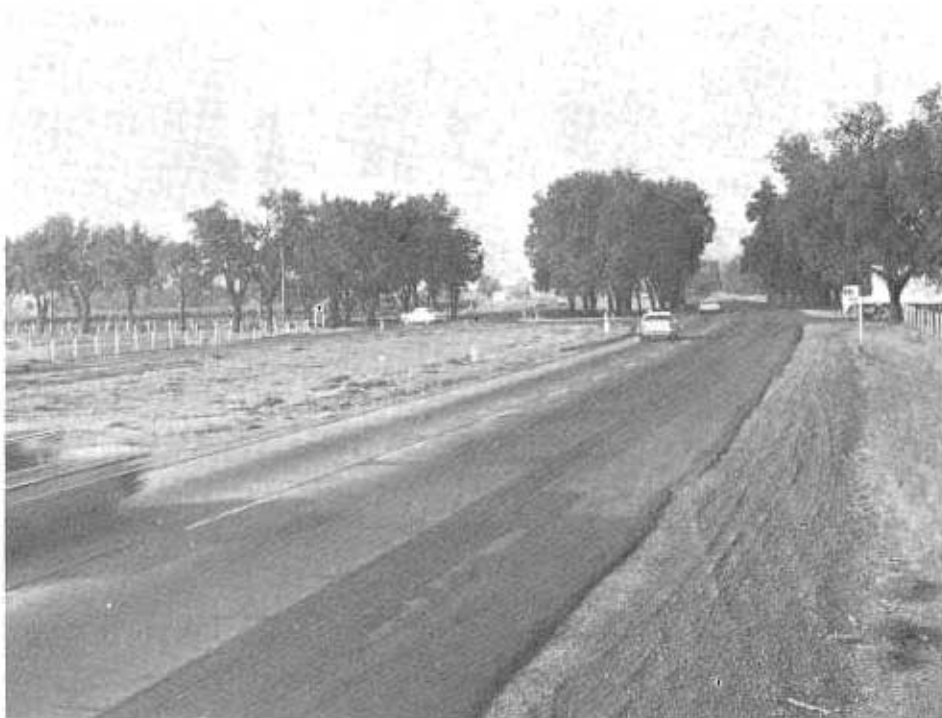
When Interstate 80 is widened near the Yolo County Line, this at-grade intersection adjacent to the University of California Davis campus will be eliminated.
