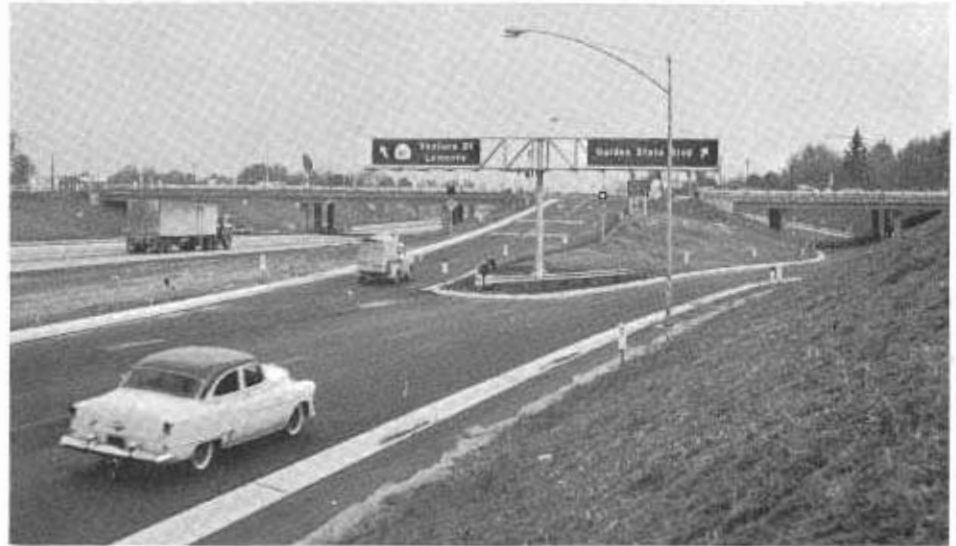
The north (Fresno) end of overall project, showing the direct connection to Golden State Boulevard, the superseded highway.
