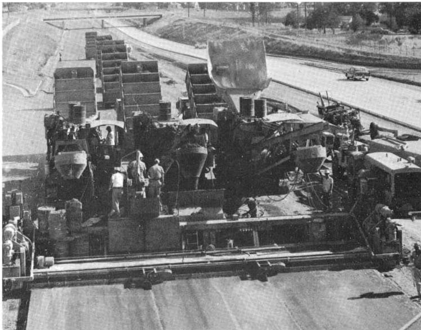
FIGURE 6—A photo of the three-lane, 36-foot highway slipform paver in operation.
