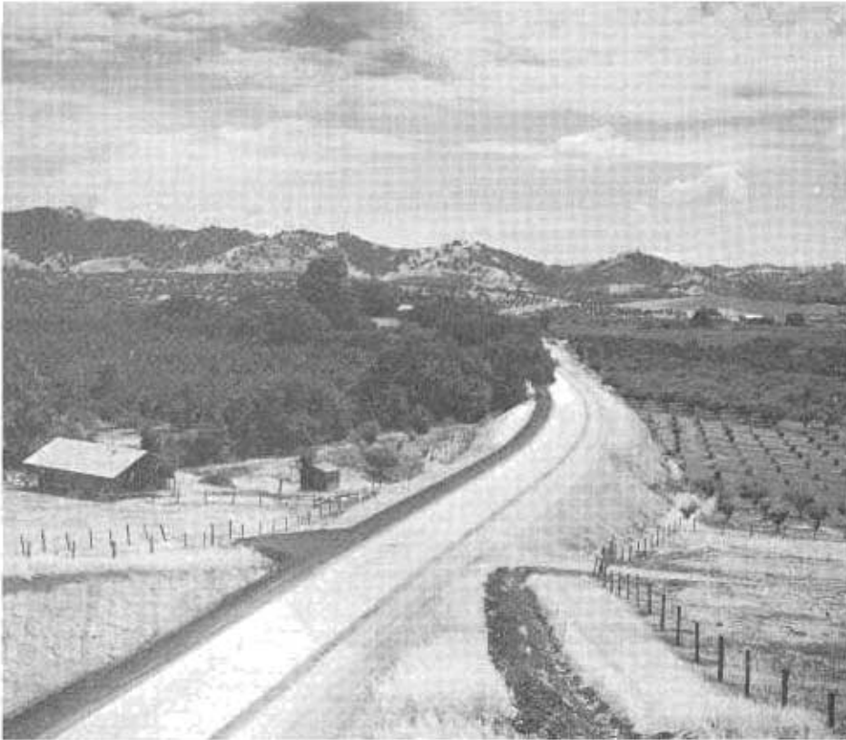
In 1937 looking toward Vacaville, formerly Route 7 and which twisted through Vaca Valley, has been realigned and reconstructed as Interstate 80 freeway.
