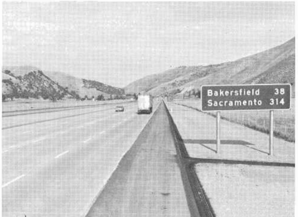
A view northward along the new eight-lane Interstate 5 Freeway between Lebec and Fort Tejon on the Ridge Route.
