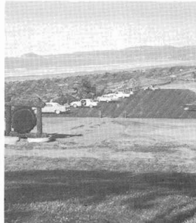
FRONT COVER: The first glimpse of the Pacific Ocean on US 101, after the motorist leaves the Golden Gate Bridge in the northerly direction, occurs 300 miles later on this new stretch of four-lane highway which bypasses McKinleyville. Here he is afforded unrestricted access to the magnificent beach for a distance of one and a half miles via frontage roads. The roadside rest features a wooden plaque dedicated to this area "Where the Majesty of the Redwoods Meets the Beauty of the Sea" and an exceptional view of Trinidad Head. See "McKinleyville Freeway," page 31. (Photo by Robert Mulno.)
