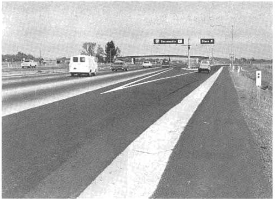
This grade separation carries Dixon-Grant Road traffic over Interstate 80.
