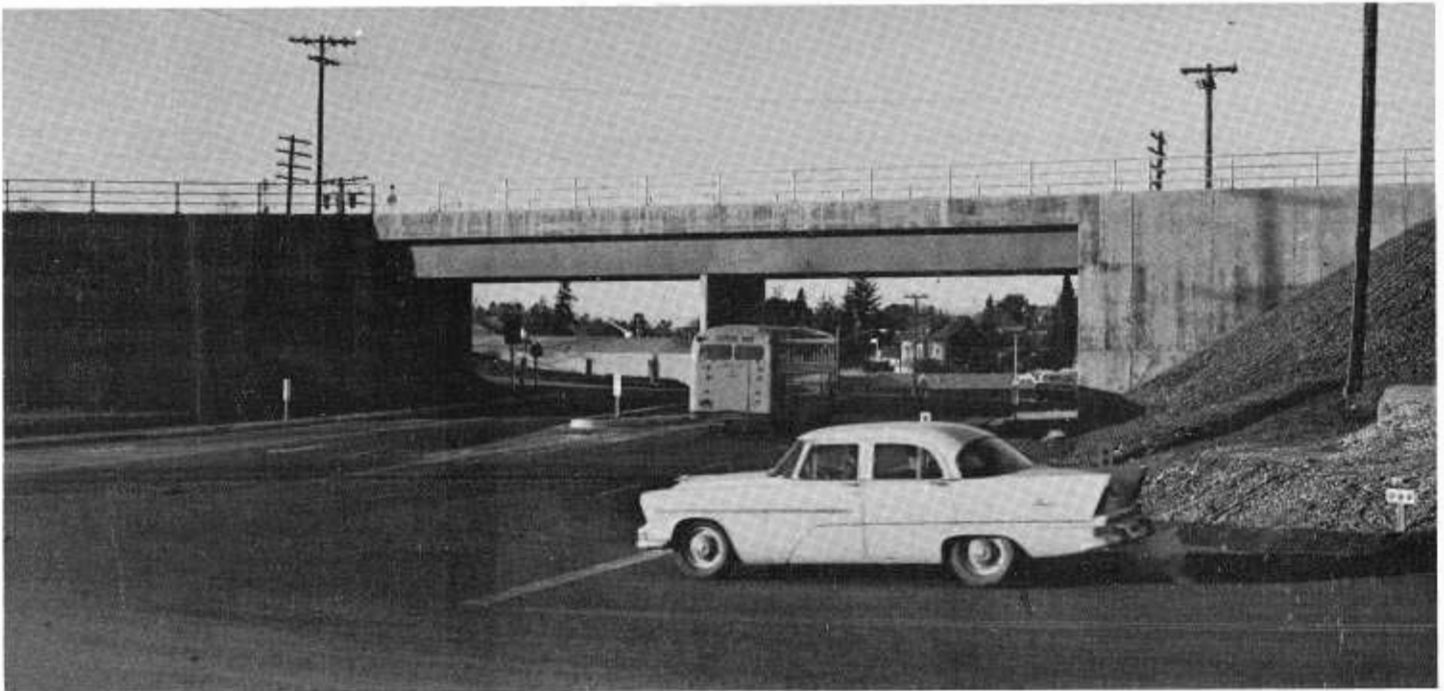
The new East Auburn Underpass is a two-span reinforced concrete box girder bridge over a four-lane highway. It was constructed on new alignment.
