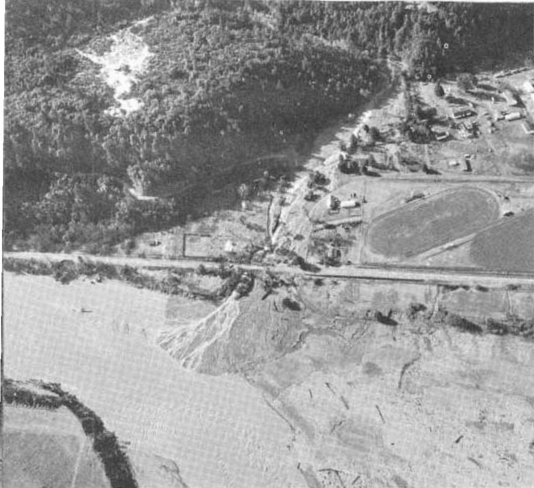
Hospital Creek on Trinity River near Hoopa brought down so much debris it filled channel, and covered highway with gravel several feet thick. This was a common type of damage in this storm, and required reestablishment of the channel in each case. Note creek "delta" in river.
