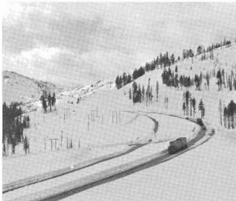
The eastbound roadway and frontage road shortly after they had been cleared of heavy snow near Donner Summit. The westbound lane is visible part way up the slope to the right.
