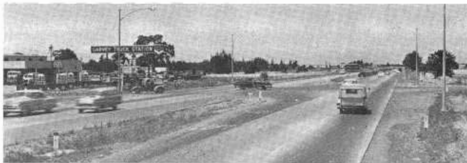
BEFORE: The Cherokee Road intersection looking northward prior to reconstruction of US 99 to full freeway east of Stockton.
