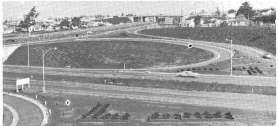
Interstate 80 traffic now speeds safely toward Sacramento over Interstate 680 (foreground) and under Benicia Road (background) near Cordelia.
