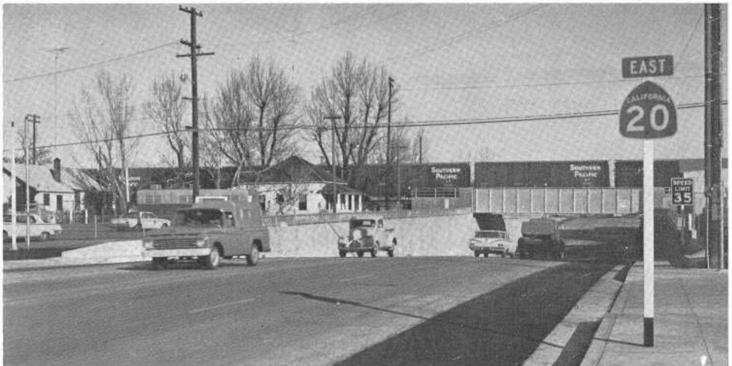
The new East Marysville Underpass on Route 20 carries four lanes of traffic under the Southern Pacific railroad tracks and has a vertical clearance of 15 feet 1 inch.
