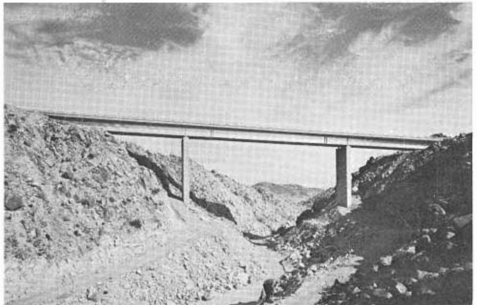
AT RIGHT: Short Span Prize Winner—DEVIL'S CANYON BRIDGE NO. 2 east of San Diego . . . Jurors' Comment: "Done in rather complete, harsh simplicity, fitting in with the country around it. It is a graceful structure using straight cantilever beams. The approaches are nice and look solid. We particularly like the proportionate simplicity of the piers holding the spans of this fine bridge."
