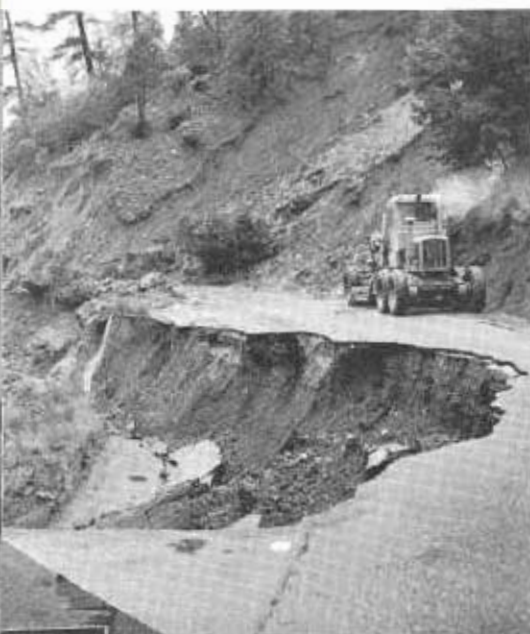
ABOVE: In this photo of roadbed destruction on Northwestern Pacific Railroad debris washed down the slope has filled the culvert and the stream has cut a new bed. (Photo courtesy of Northwestern Pacific Railroad.) BELOW: Destruction here is by slipout, or, in other words, a slide of the supporting slope below the roadbed.
