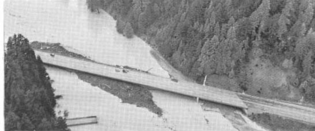
George Leatherwood Memorial Bridge, on US 101 Freeway near Dyerville on South Fork of Eel, withstood flood after blasting of debris by a highway maintenance man. Stubs visible just downstream are approaches to old through-truss bridge on Route 254, Avenue of the Giants. This bridge failed at height of flood, when water was somewhat higher, although it had stood through many previous floods. (Photo courtesy of Eureka Newspapers, Inc.)
