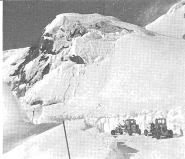
Graders remove snow after the big storm of 1952 on the old Donner Grade about halfway up the east slope near Big Shot.
