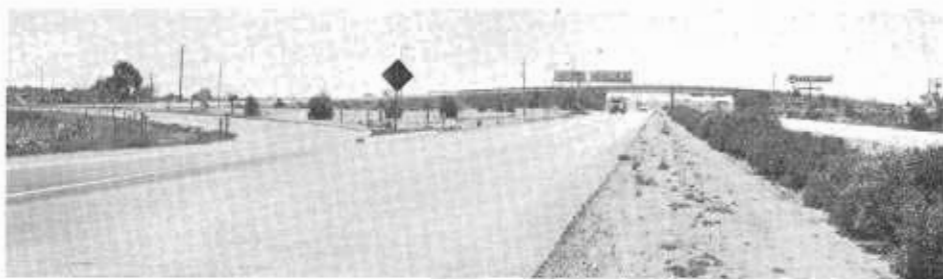
AFTER: Looking south towards the Cherokee Road Overcrossing following the freeway construction.
