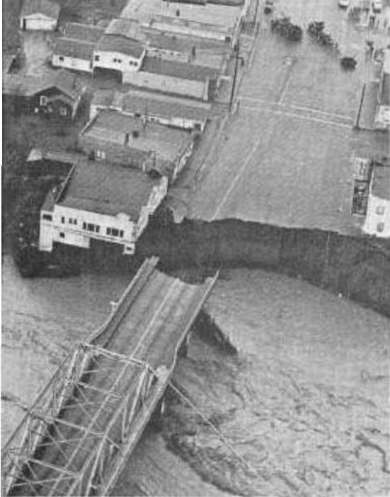
ABOVE: North abutment of North Scotia Bridge at Rio Dell torn out by force of Eel, here shown partly in flood. Building at left of broken bridge end is now gone. (Photo courtesy of Eureka Newspapers, Inc.) BELOW: Looking south along US 101, the Redwood Highway, with the town of Klamath in the foreground, and washed-out bridge in background. (Photo courtesy of Eureka Newspapers, Inc.)
