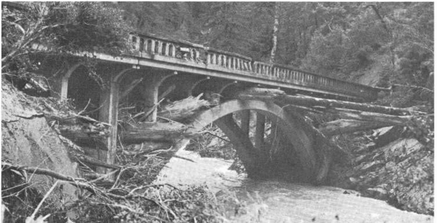
ABOVE: Squaw Creek, cascading down the steep slopes at Cummings on the Redwood Highway, tore this gap in the road. BELOW: This concrete arch bridge on US 199 above Crescent City withstood the flood, despite obvious pounding. Note debris lodged in every opening, and battered conditions of railing.
