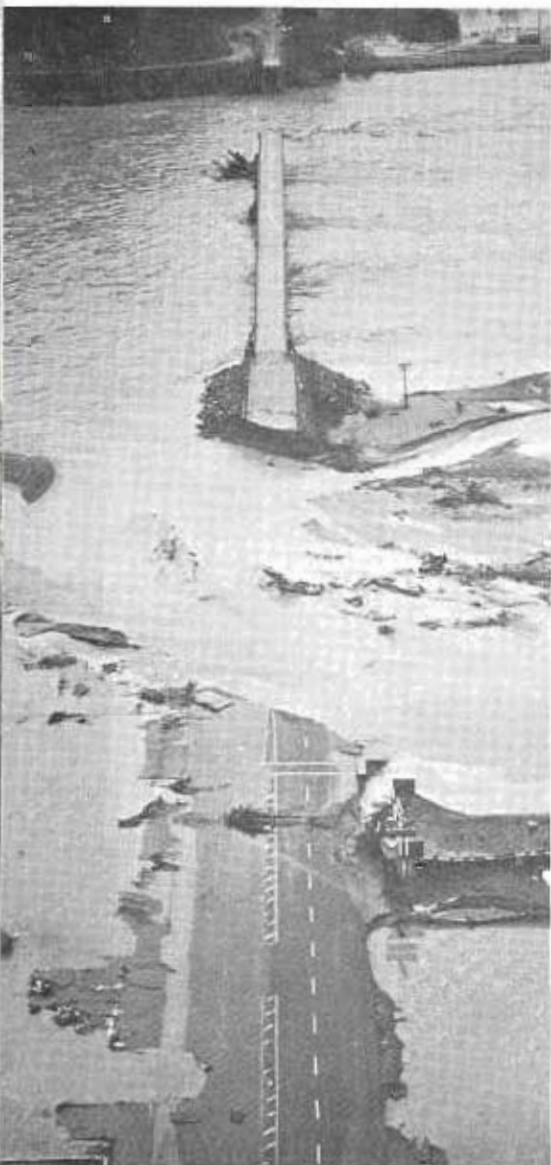
ABOVE: North abutment of North Scotia Bridge at Rio Dell torn out by force of Eel, here shown partly in flood. Building at left of broken bridge end is now gone. (Photo courtesy of Eureka Newspapers, Inc.) BELOW: Looking south along US 101, the Redwood Highway, with the town of Klamath in the foreground, and washed-out bridge in background. (Photo courtesy of Eureka Newspapers, Inc.)
