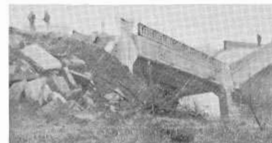
ABOVE: Looking across gap of fallen North Fork of Russian River Bridge at Calpella. Severance of utility lines disrupted telephone service for entire area. (Schroll Studio photo courtesy of Santa Rosa Press Democrat.) BELOW: Stephens Bridge over Cache Creek, Yolo County, 5½ miles west of Woodland.
