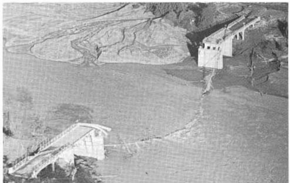
BELOW: Until December, this was the beautiful State suspension bridge at Orleans, which won an award for design in 1940. Flood topped deck before bridge gave way. (Photo courtesy Six Rivers Forest, U.S. Forest Service.)
