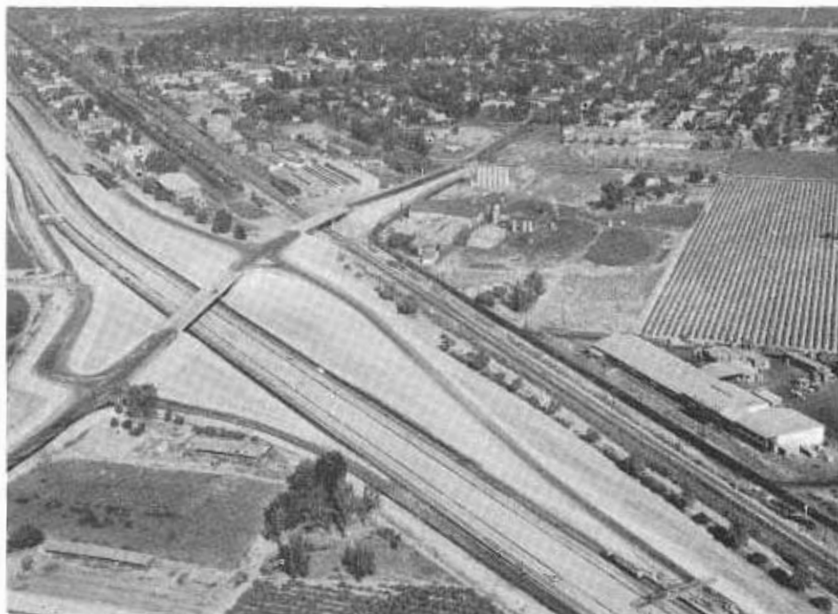
Mendocino Avenue Overcrossing and Overhead south of Kingsburg. The Tulare-Fresno county line is just beyond the structures.
