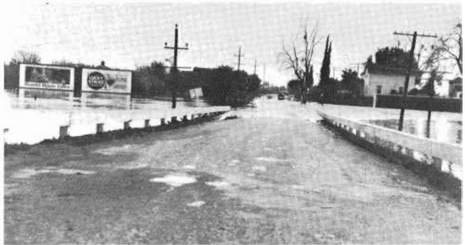
This photo taken in the early 1930's shows US 99 flooded south of the Mokelumne River bridge.
