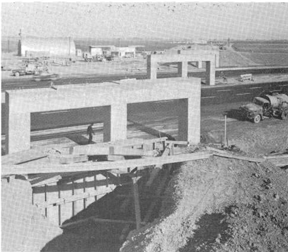
The substructure of the Pedrick Road overcrossing near Dixon on Interstate 80.
