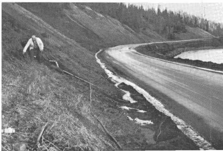
ABOVE: This paving damage was caused by pressure of sliding material on slope at right, forcing its way between road surface and foundation. BELOW: Man in photo has right hand at high-water mark which South Fork of Eel reached here near Phillippsville. This stretch of freeway, recently completed, was constructed five feet above high-water line of 1955 flood.
