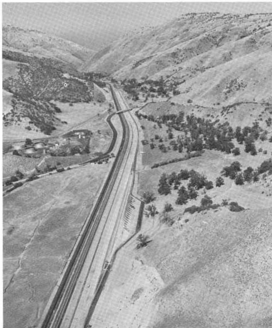
The combination truck brake inspection area and safety rest stop can be seen in the lower center of this aerial photo.
