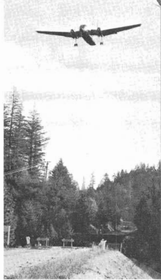
In many places travel by air was the only means of access. A Division of Highways photographer caught here an Army Caribou plane over a destroyed bridge on US 299.
