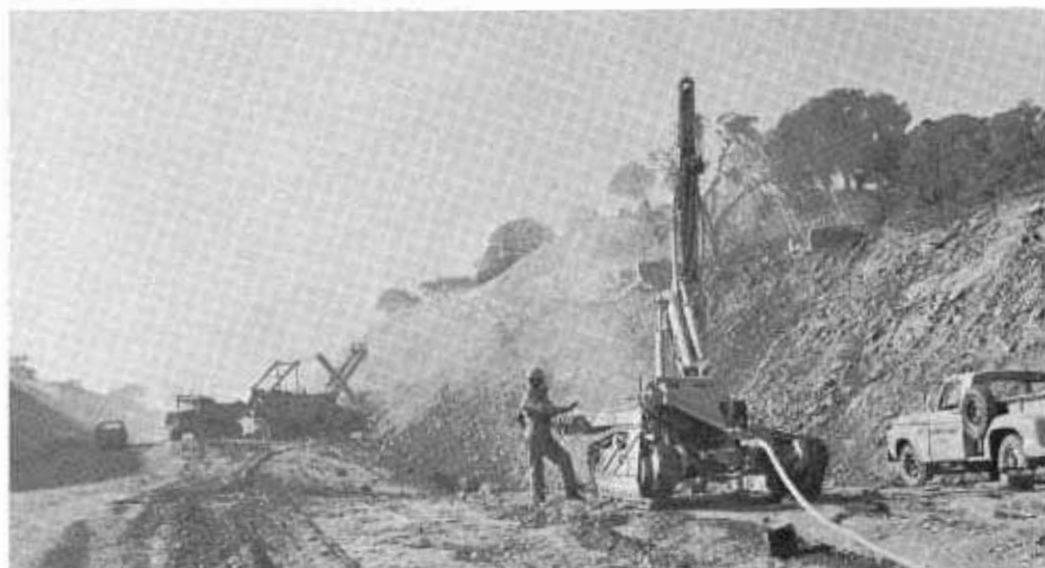
Above—Bin wall is constructed to contain fill slope in a steep canyon. Below—Drilling operations in the foreground coincide with rock loading by a huge power shovel onto dump trucks in background.
