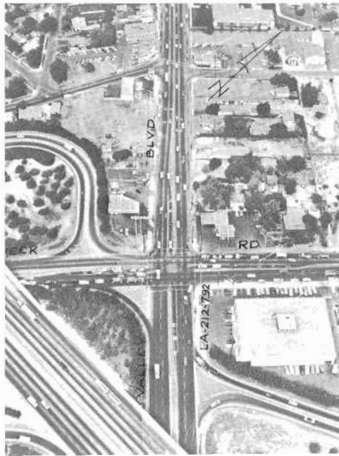
AFTER: Peck Road-Valley Boulevard intersection. With left turn channelization, improved signals, etc., the motorist's right of way is more clearly defined. Accidents have decreased 39 percent (from 64 to 39).
