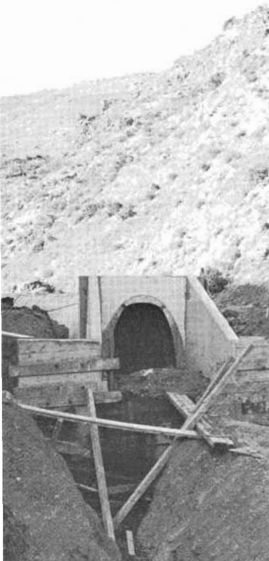
This arch structure now rests under 2,000,000 cubic yards of dirt required for the "Big Fill."
