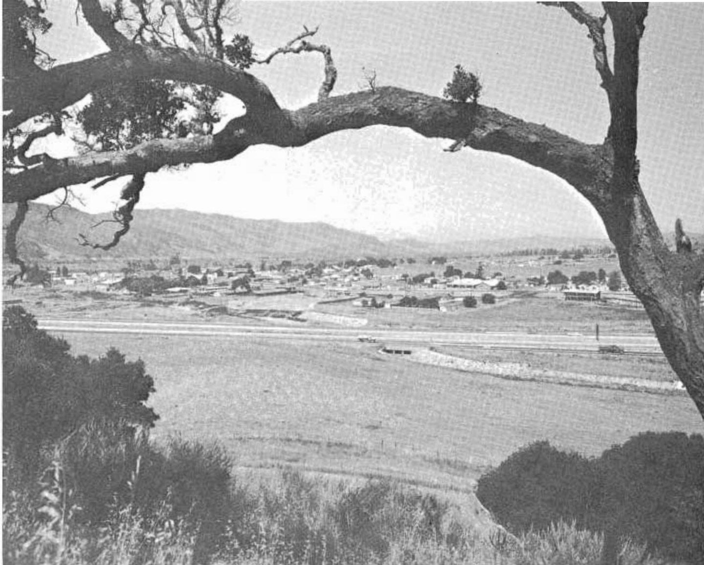
Looking southwesterly across the completed freeway toward the town of Buellton. The Zaca Creek Channel Change is in the middle foreground.
