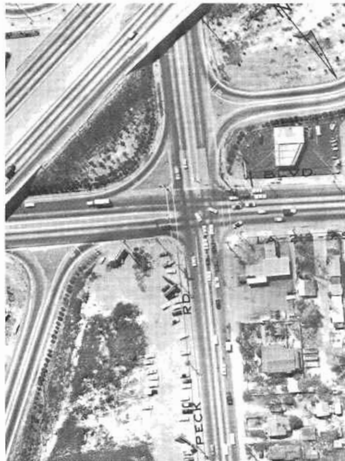
BEFORE: Peck Road-Valley Boulevard intersection in El Monte, California. A high incidence of accidents took place at this intersection before a minor improvement project eliminated uncontrolled left turns from four directions.
