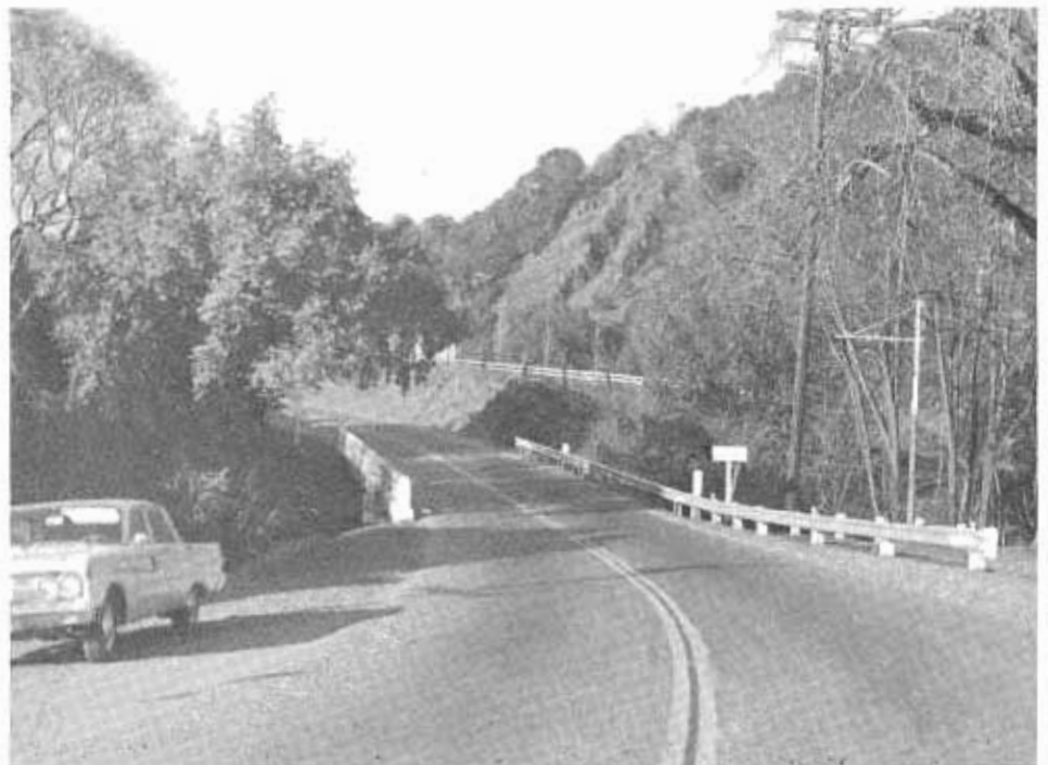
AFTER: Accidents at this location were reduced from seven to two per year by replacing the concrete bridge railing on the offending side with a continuous metal beam strip and correcting the super-elevation (project cost: $4,006).
