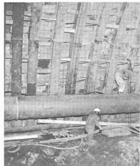
(Below) Steel sets and timber lagging support excavation of upper portion of tunnel. Roadway level is about 14 feet lower.
