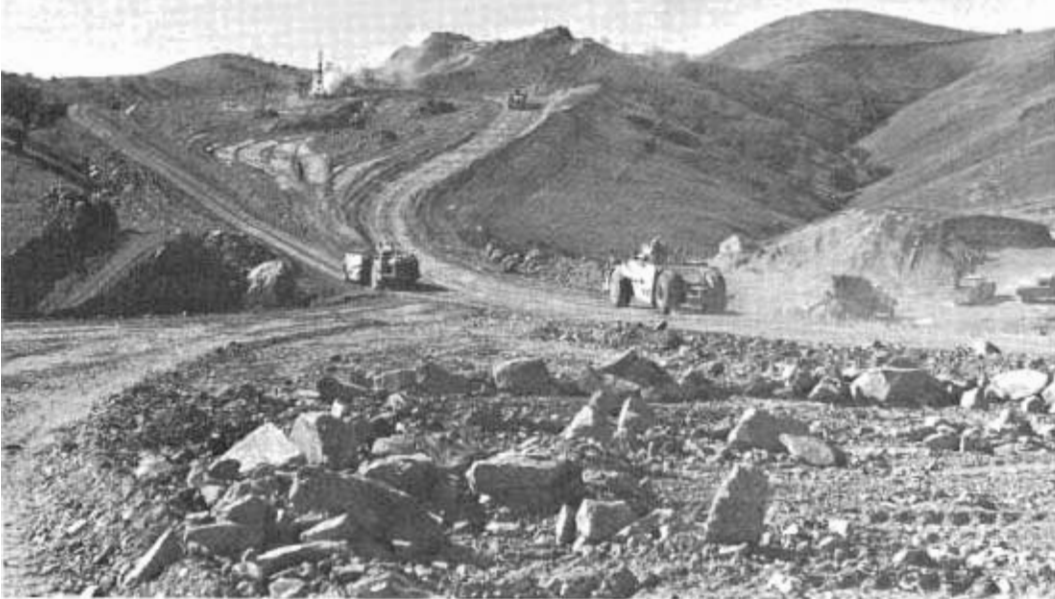
A peak is leveled and a canyon filled. Heavy equipment takes a beating in this rough terrain.
