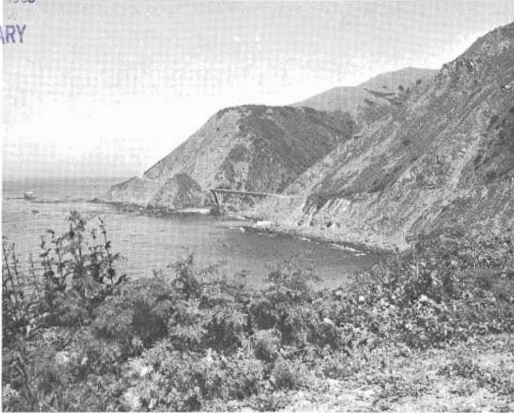
California's first officially designated "Scenic Highway" includes this section near the Big Creek Bridge, south of Big Sur.
