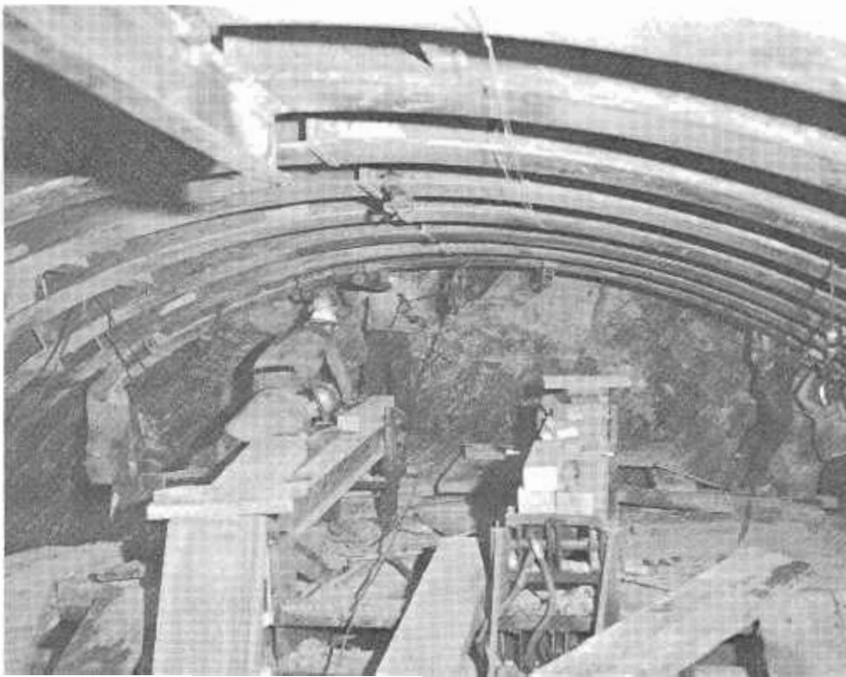
(Below) On the top level of the jumbo, miners demonstrate some of the obstacles of their work. Space is tight and some tasks are awkward to perform.
