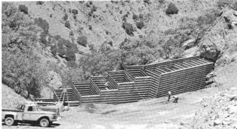
Above—Bin wall is constructed to contain fill slope in a steep canyon. Below—Drilling operations in the foreground coincide with rock loading by a huge power shovel onto dump trucks in background.
