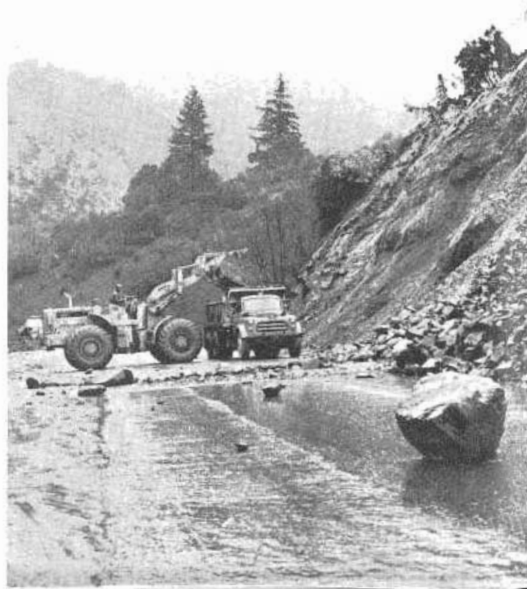
Minor slide on Redwood Highway south of Cummings being cleared by front-end loader and trucks.
