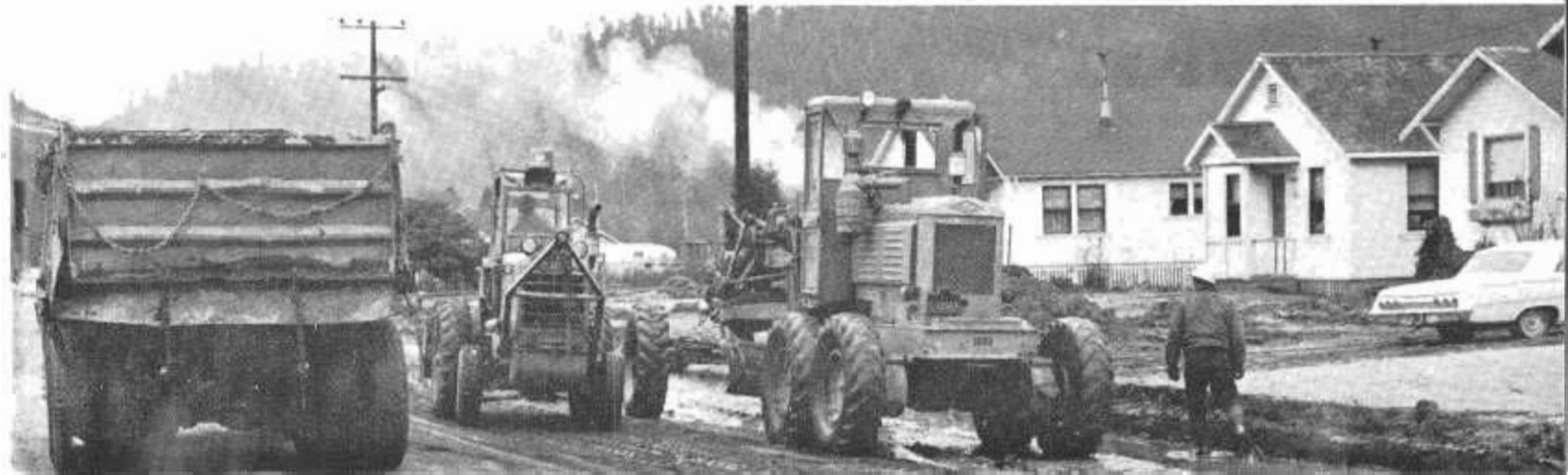
Boom of backhoe is used as crane for lifting sections of culvert into place while repairing washout near Richardson Grove.
