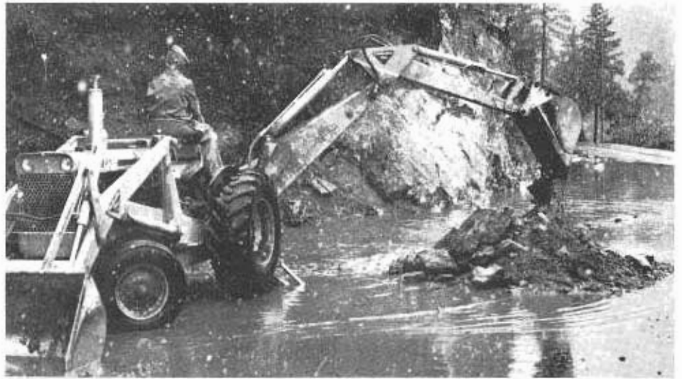
Light backhoe working in snowstorm, clearing drain on Route 299.
