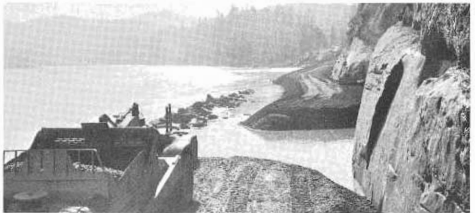
Five photos this page show steps in development of Blue Slide Road detour on Redwood Highway. Upper left is view of road on January 4 after flood; top is traffic moving in one-way convoys above cliffs before lower section repaired; directly above is filling operation on same section as shown in upper left. Directly below, about three weeks later, lumber trucks moving over this section; and bottom, same detour road where it crosses the floodplain, photographed March 17 after asphalt paving laid.
