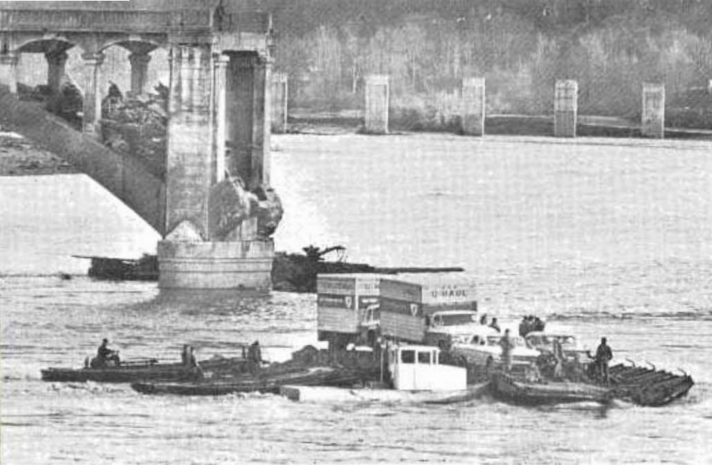
Widely publicized Sixth Army pontoon ferry crossing Klamath River; ruined bridge upper left with log spawner watching upstream. Note debris on bridge. (Eureka Newspapers, Inc., photo.) Piers in background are for new highway bridge under construction.
