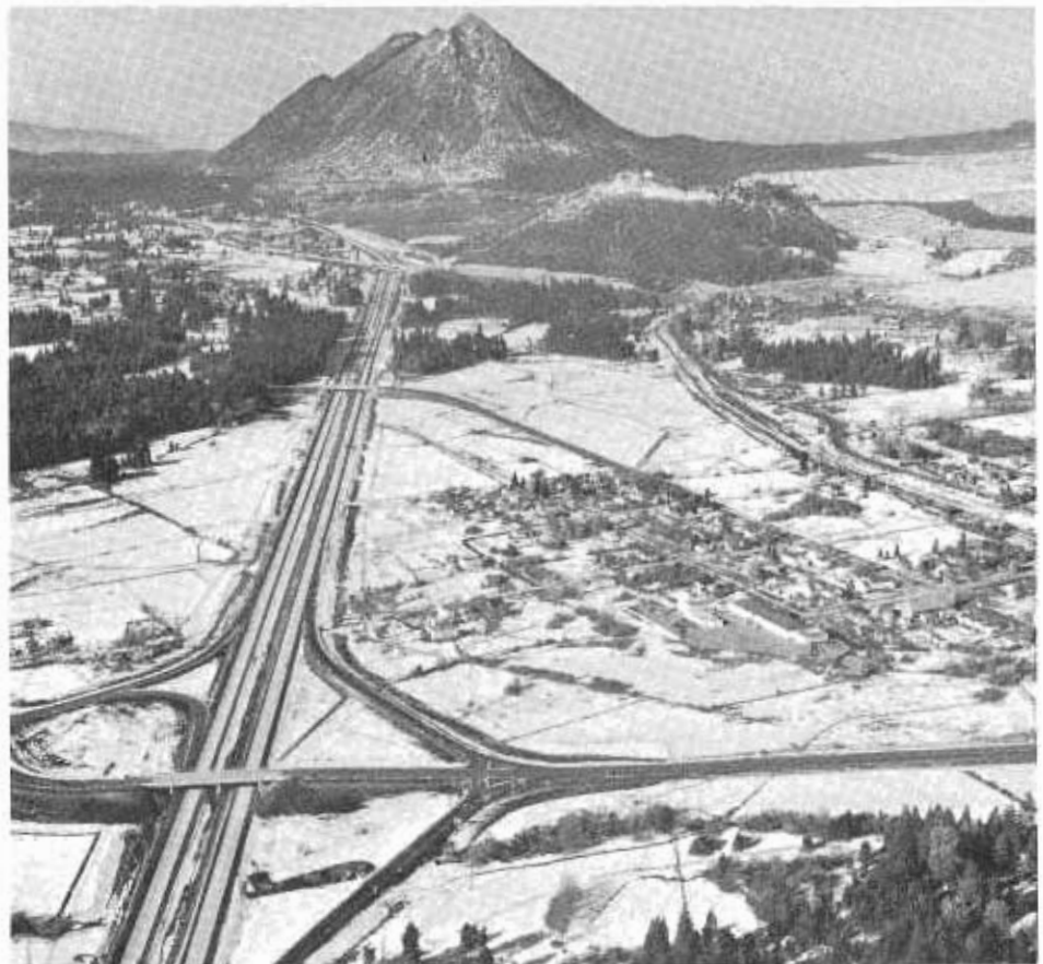
An aerial of the completed freeway looking northwest toward Black Butte Mountain. Structures are Lake Street overcrossing (foreground), Lassen Lane overcrossing (center) and North Mount Shasta railroad underpass in the distance.
