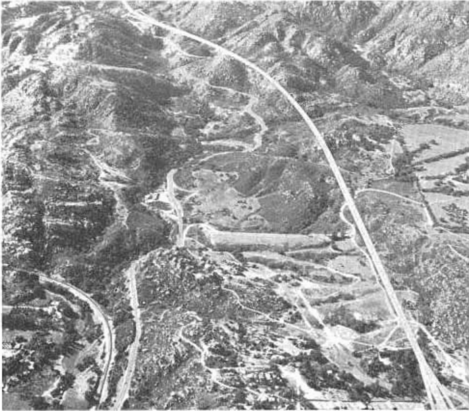
Drawn in at the right is the planned route through Santa Susana Pass. The first project on the Simi Valley Freeway will be advertised for bids this fall.
