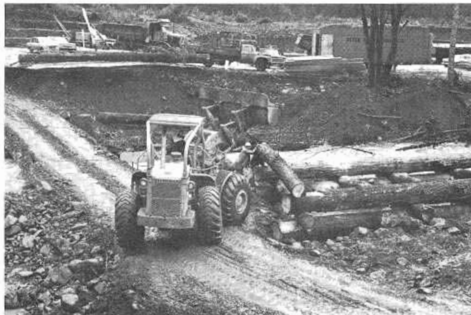
ABOVE: After first building low-level log bridge to move equipment in, contractor here, using front-end loader as crane, puts logs in place for abutment for higher level crossing. BELOW: The finished bridge, crossing Patrick's Creek, US 199.
