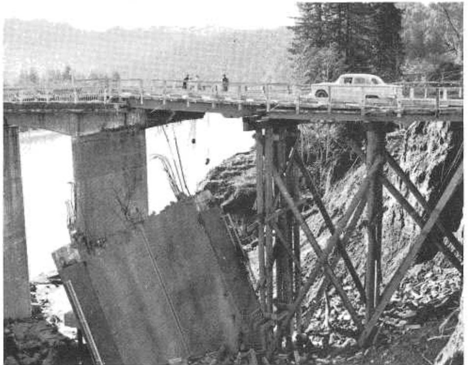
ABOVE: Temporary one-way bridge of wooden piles, beams, and planks built across break at north end of Scotia-Rio Dell Bridge carried legal loads for several months. BELOW LEFT: Footbridge was first span over gap and served many needs for two weeks. Requirements of sign were strictly enforced by civil defense officials. BELOW RIGHT: The footbridge, a simple suspension design, being built by Pacific Lumber Co. and P.G. & E. employees. (Both lower pictures Eureka Newspapers, Inc.)
