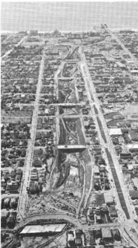
The last contract to be let on the Santa Monica Freeway takes this route seaward. The project in Santa Monica will be completed this fall.
