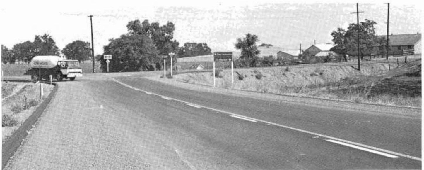
Looking northward along Dillard Road toward the Highway 16 junction.
