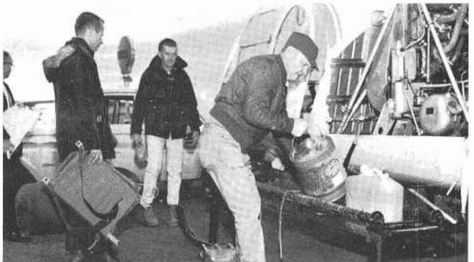
Young highway engineers from Eureka standing by at airport as helicopter pilot loads extra gasoline for flight into Samesbar far up Klamath River. Many small groups such as this were sent by air or on foot to organize emergency road repair contracts in isolated areas.
