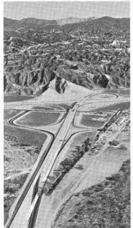
The view looking eastward on Route 126 shows the interchange with Interstate 5 in the Castaic Junction-Saugus area.
