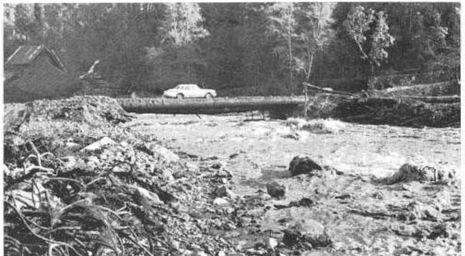
The log emergency bridge at Willow Creek on January 7, 1965. At upper left is collapsed bridge. Photo on opposite page made same day gives aerial view of this area.
