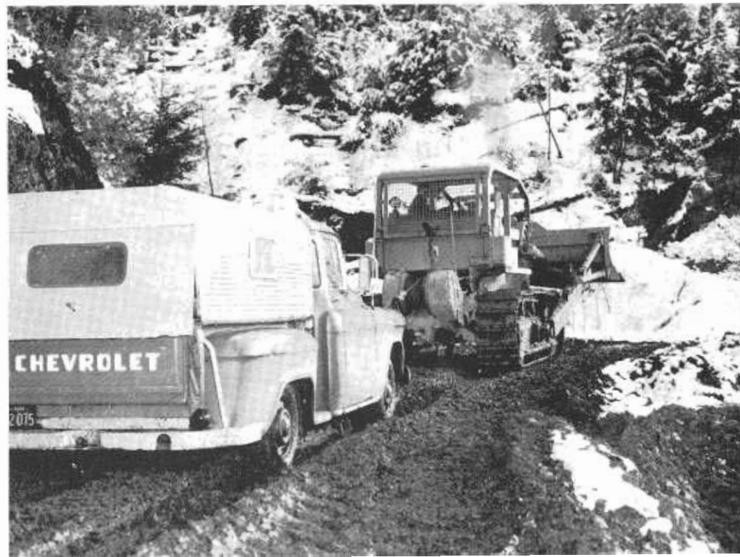
In first days of opening emergency route, assistance from tracked tractors was necessary in places.
