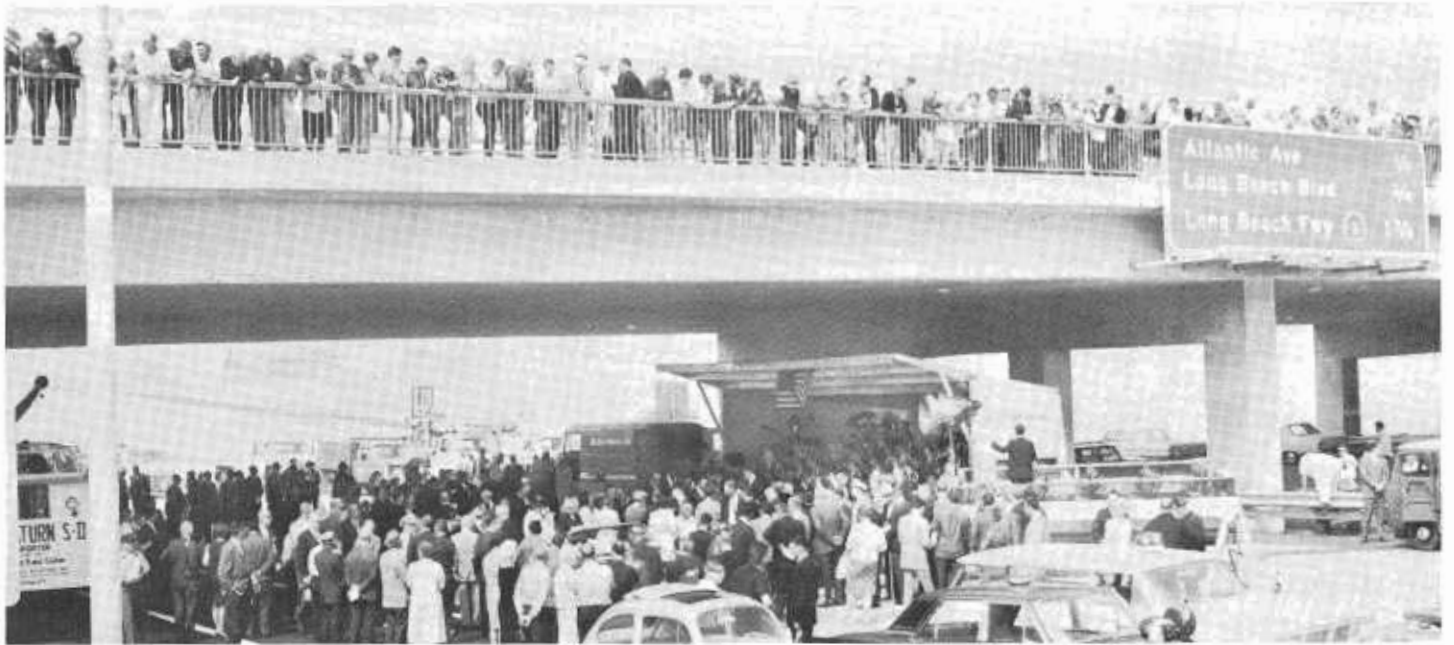
Considerable public interest was evident at the October 1 dedication of this 9.5-mile section of the San Diego Freeway which links Los Angeles and Orange Counties. About 1,000 people were in attendance.
