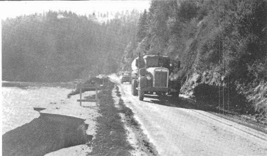
Section of Redwood Highway south of Pepperwood, along main Eel River as it appeared on January 12, 1965. Dirt ridge was used like this wherever paving was destroyed to delineate safe driving area.
