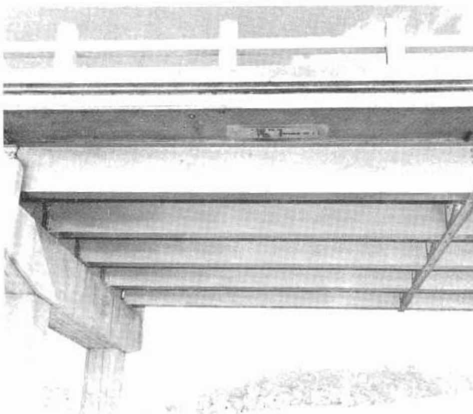
FIGURE 5 Typical condition of paint of system No. 1.
