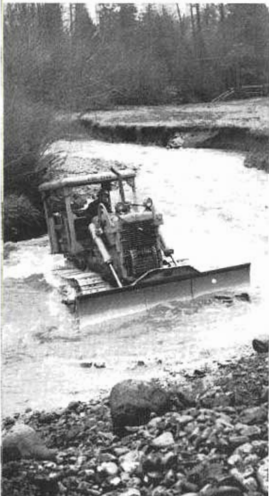
ABOVE: Portable drill rig in operation on Route 299 making holes for charges to blast cliff away to widen road. BELOW: Tractor and blade clearing debris from streambed to increase runoff.
