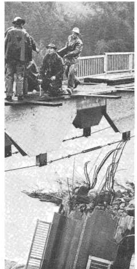
ABOVE: Temporary one-way bridge of wooden piles, beams, and planks built across break at north end of Scotia-Rio Dell Bridge carried legal loads for several months. BELOW LEFT: Footbridge was first span over gap and served many needs for two weeks. Requirements of sign were strictly enforced by civil defense officials. BELOW RIGHT: The footbridge, a simple suspension design, being built by Pacific Lumber Co. and P.G. & E. employees. (Both lower pictures Eureka Newspapers, Inc.)
