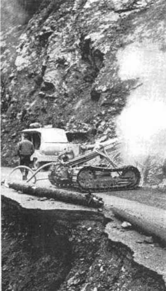
ABOVE: Portable drill rig in operation on Route 299 making holes for charges to blast cliff away to widen road. BELOW: Tractor and blade clearing debris from streambed to increase runoff.
