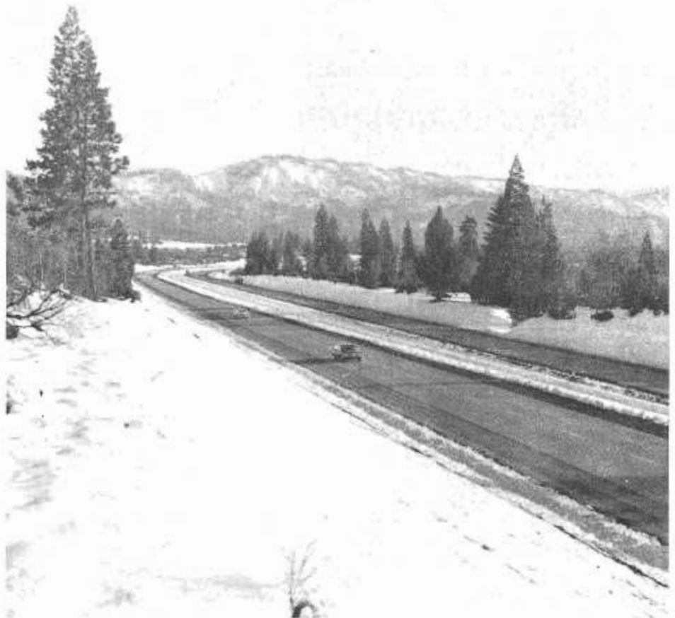
The completed section of I-5 freeway looking south near Mount Shasta City.
