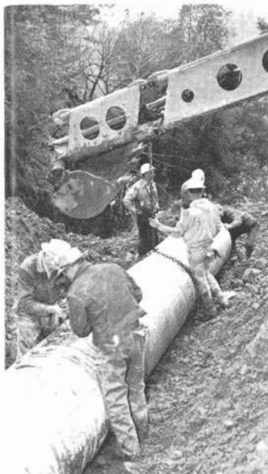
Boom of backhoe is used as crane for lifting sections of culvert into place while repairing washout near Richardson Grove.
