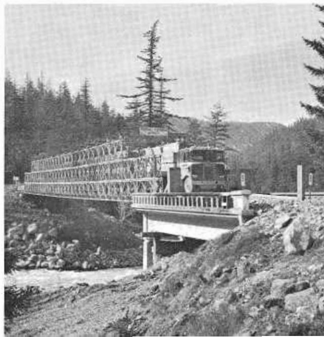
BACK COVER: Photo made exactly two months after disastrous Christmas week floods in northern California shows Bailey bridge in place across washed-out span on Smith River, US Highway 199, between Crescent City and the Oregon line. Torrents tore out several miles of this highway, in addition to three major bridges. Since major traffic load in winter is industrial, reconstruction had to support full legal loads, which road is now carrying. See articles on reconstruction in this issue. Photo by Robert Mulno.
