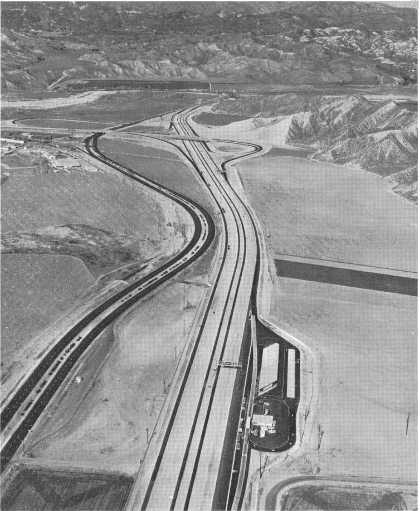
Completion of Interstate 5 in the Castaic Junction area leaves the older US 99 (on left) for frontage access. Truck-weighing facility is in foreground.
