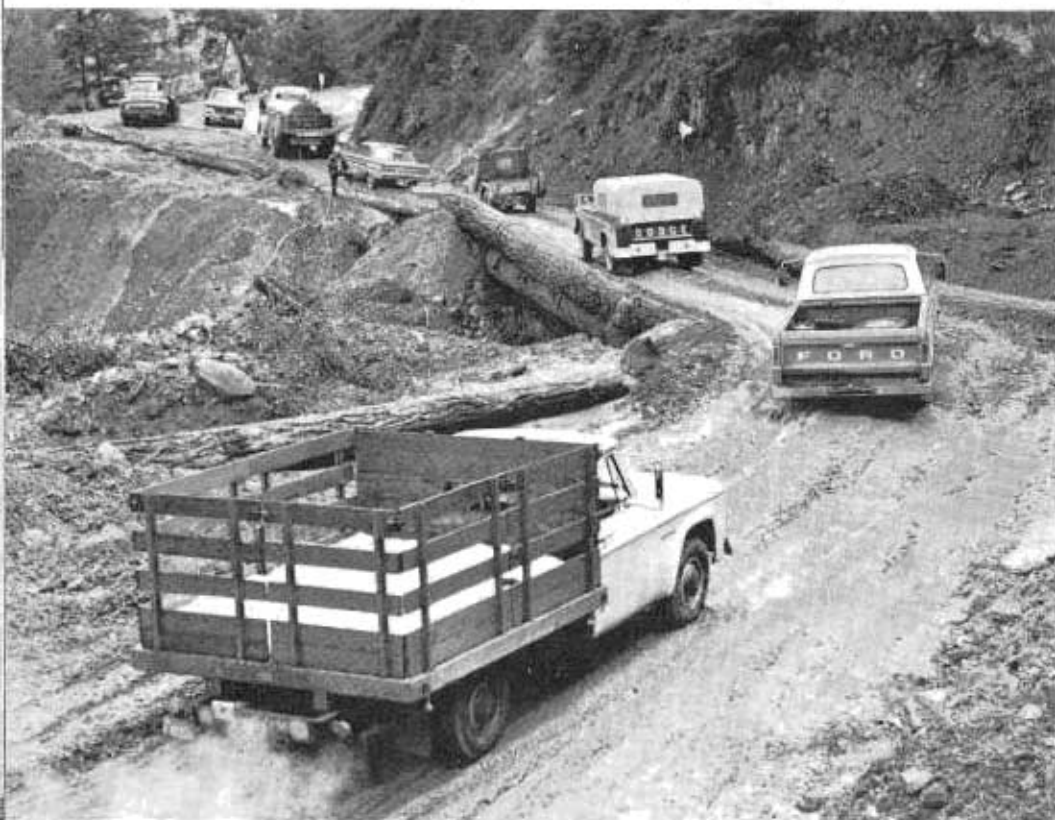
ABOVE: Convoy of evacuees working its way around detour on Route 299 at Junction City on December 28, 1964, over one-way bulldozer road. BELOW: Westbound convoy on Route 299 January 7, 1965, at Pony Creek. Note logs used as guardrails and delineators.
