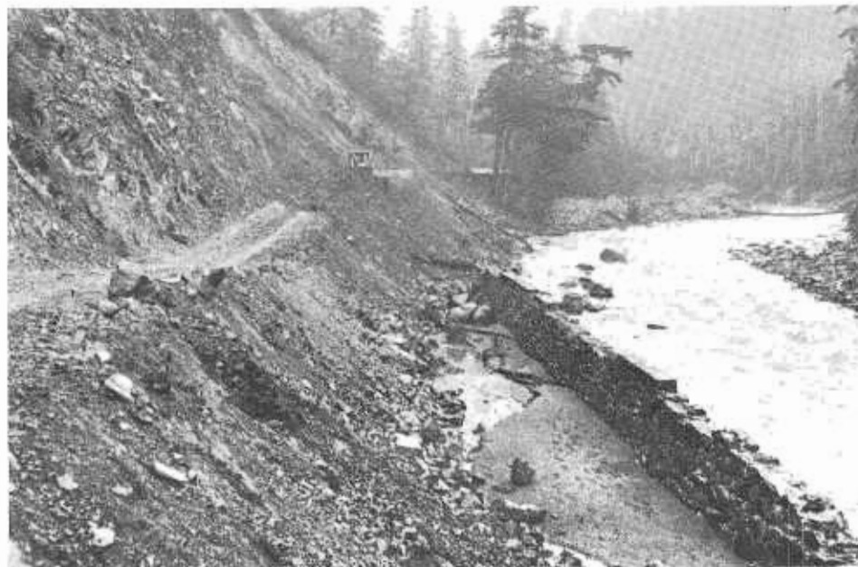
ABOVE: Partly rebuilt section of Route 199 in Smith River Canyon. Rock wall was for protection of fill but river rose much too high. BELOW: First truck convoy south from Eureka area on US 101 at Garberville at 2 a.m. on morning of January 16th waiting order to proceed.
