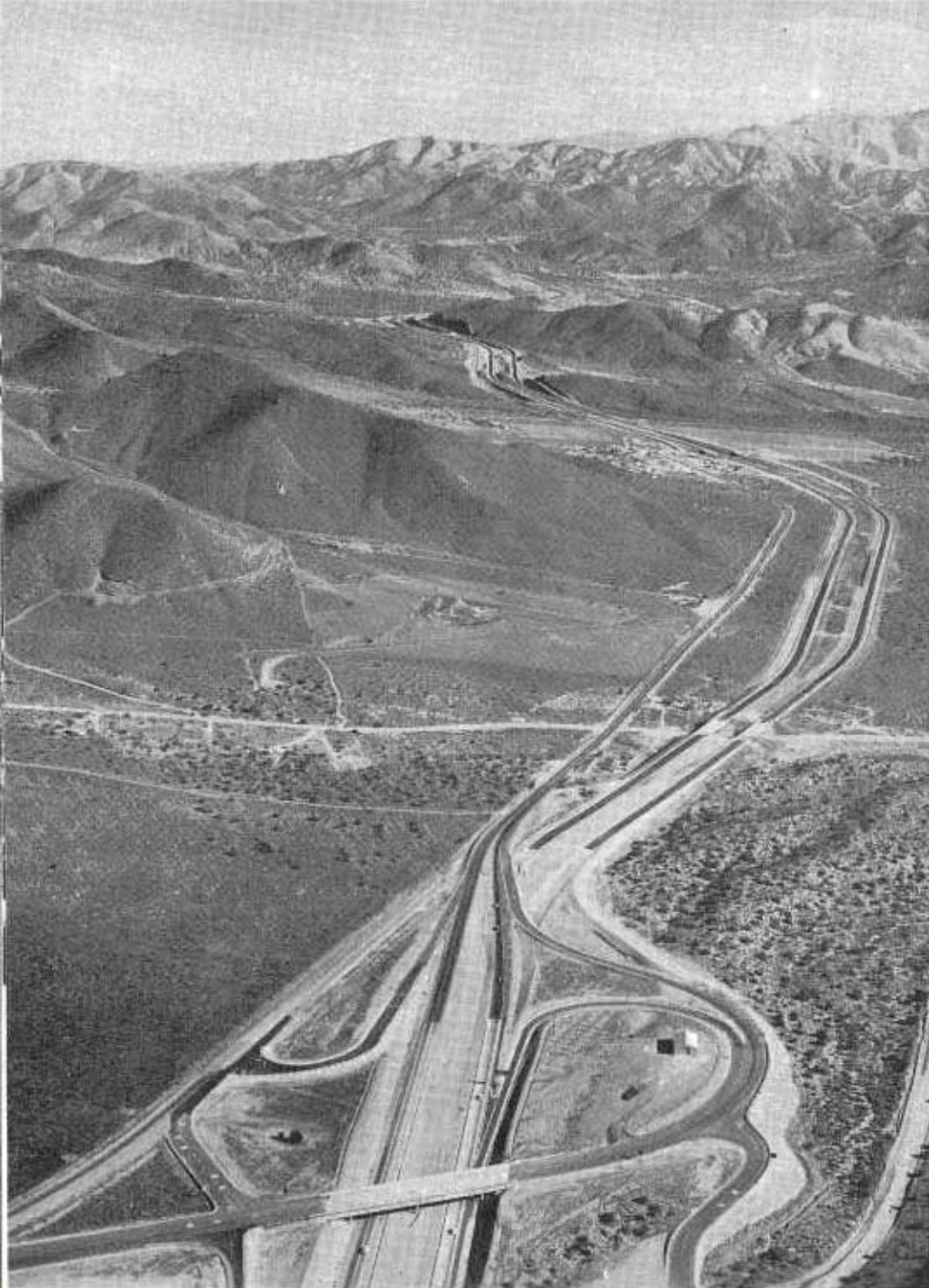
The present eastern terminus of the Antelope Valley Freeway is located at Ward Road Overcrossing in foreground. In photo center, the freeway construction crosses over Red Rover Mine Road.
