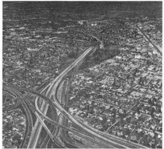
The Hollywood Freeway is also being extended. This view shows construction north of the interchange with the Ventura Freeway.
