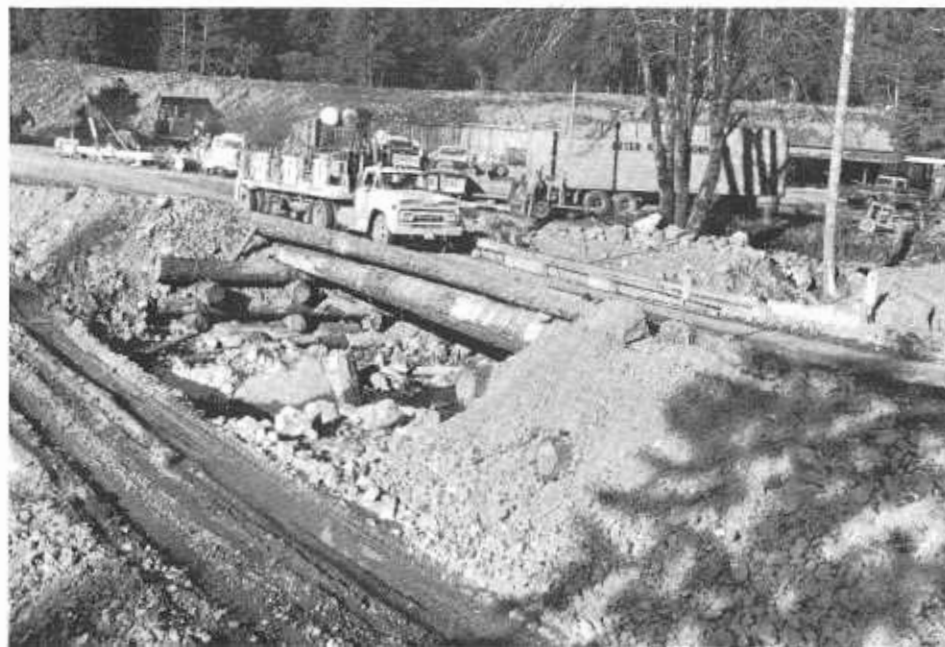
ABOVE: After first building low-level log bridge to move equipment in, contractor here, using front-end loader as crane, puts logs in place for abutment for higher level crossing. BELOW: The finished bridge, crossing Patrick's Creek, US 199.
