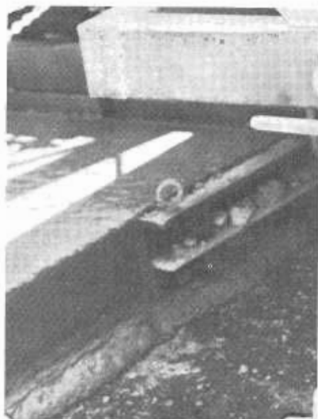
FIGURE 11—A closeup of the pavement edge immediately behind the slide forms.
