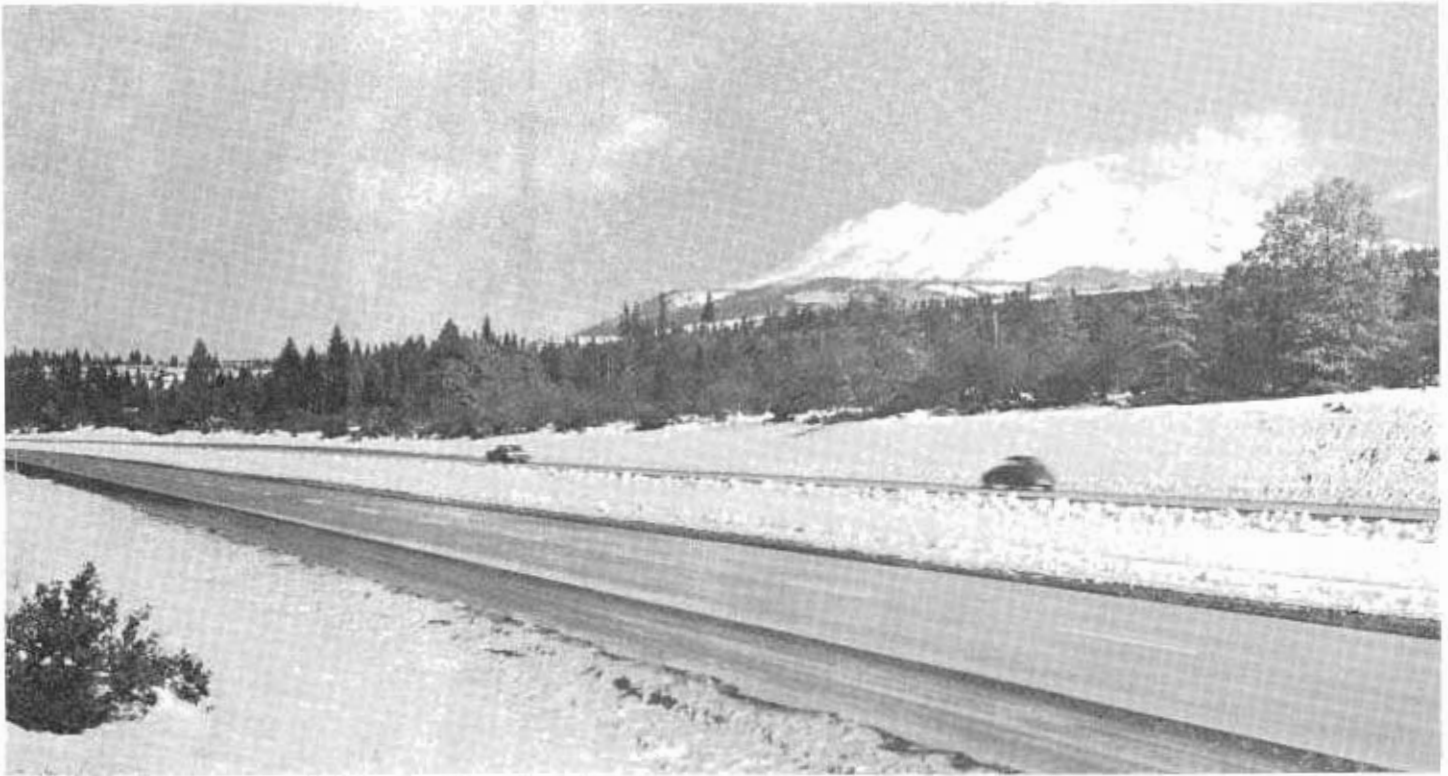
Looking toward Mount Shasta from above the completed freeway south of Mount Shasta City.
