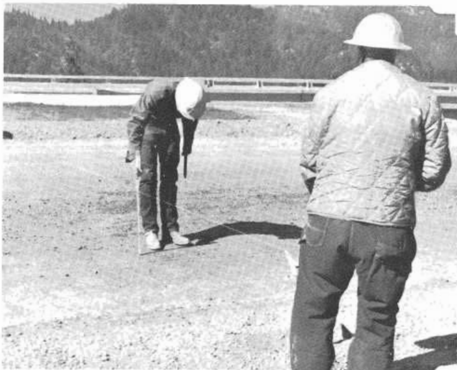
FIGURE 10—A taut stringline is used to measure subgrade.
