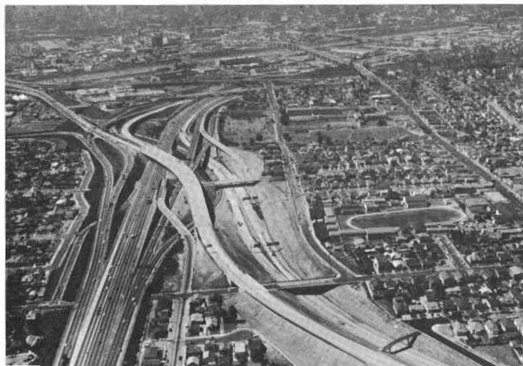
The first unit of the Pomona (Route 60) Freeway from the East Los Angeles Interchange has been completed, connecting to construction in progress easterly to Industry. The older freeway at left is the Santa Ana (Interstate 5).
