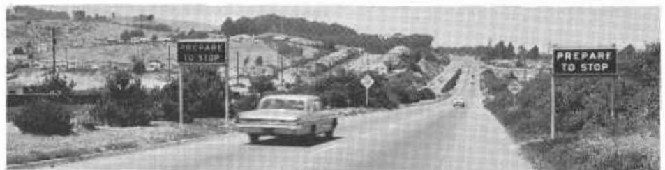
The same location as in the above photo a few minutes later showing the PREPARE TO STOP signs in operation, giving motorists a warning of conditions in advance.
