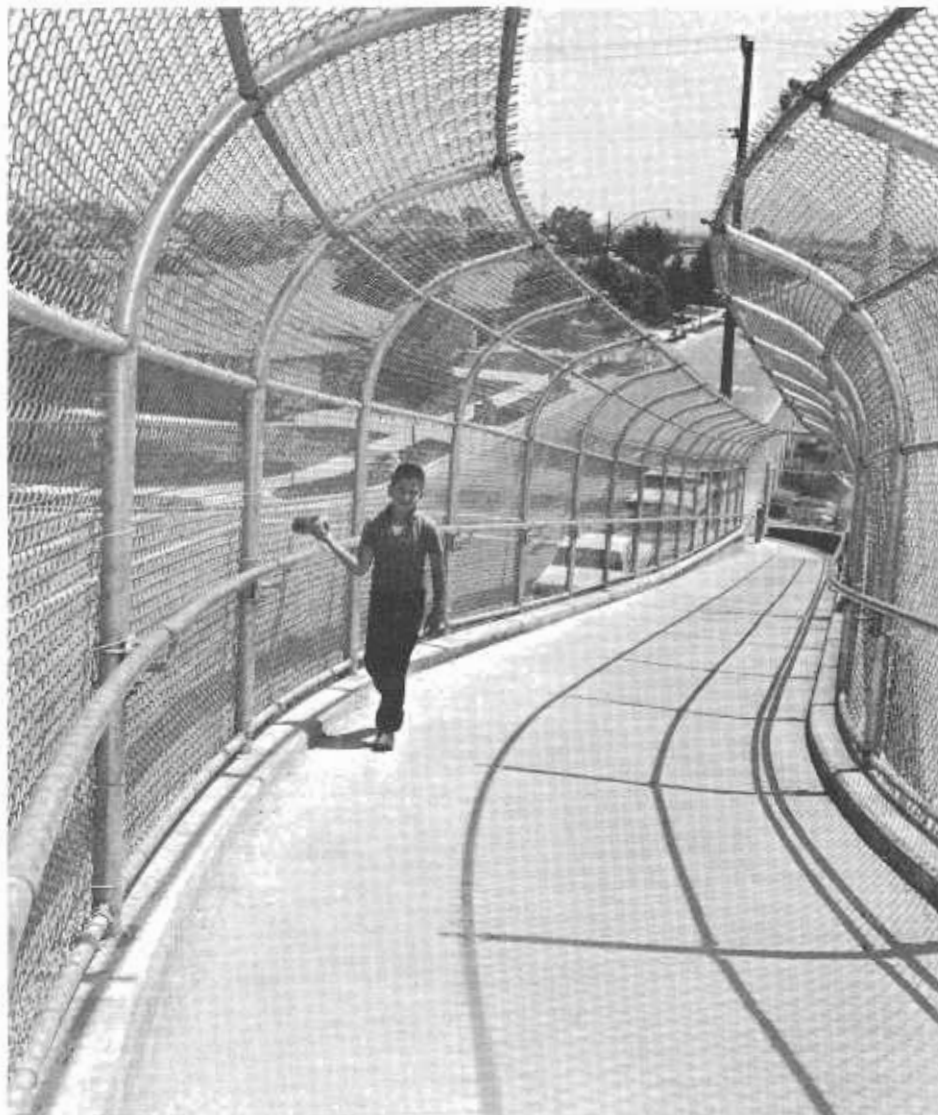
The chain link fences that form protective barriers on freeway overcrossings designed in recent years for pedestrian use have been modified from a square cagelike effect to this less confining structure. This type provides full protection and at the same time avoids any tunnel effect.
