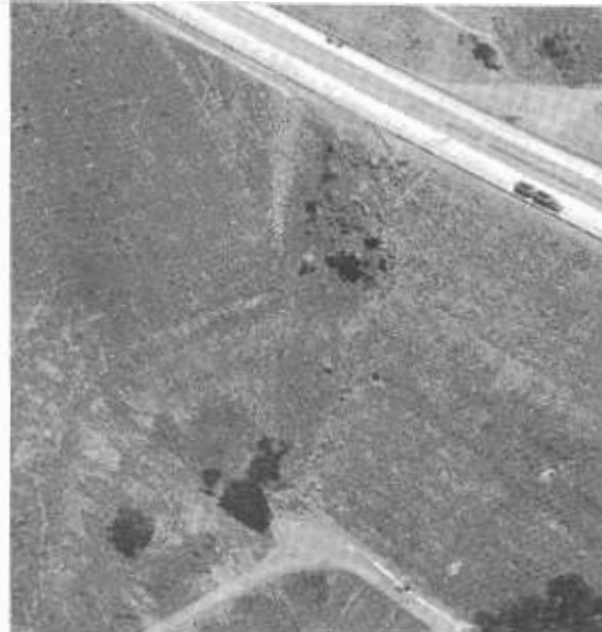
Shown is one of the highest highway fills in this country, required by the completion of the 12.4-mile Route 152 Expressway through Pacheco Pass around the area to be inundated by the San Luis Reservoir.
