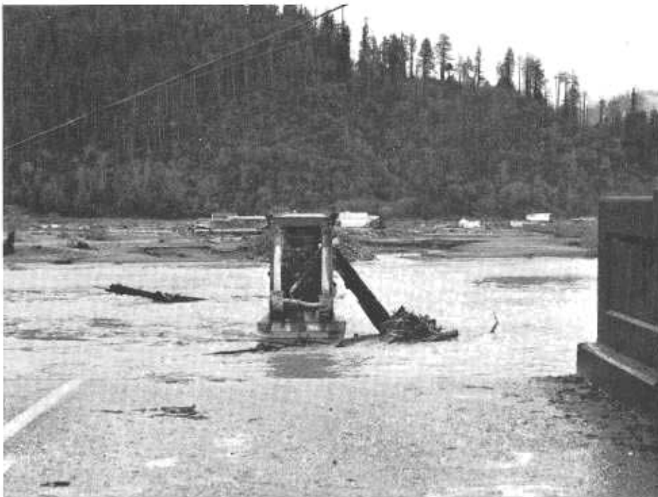
The Klamath River Bridge looking north at the remains of the town of Klamath on December 30, 1964. Note the debris that has collected in the supporting members of the bridge. The large log leaning against the side of the bridge weighed about 30 tons. (See previous photo.)
