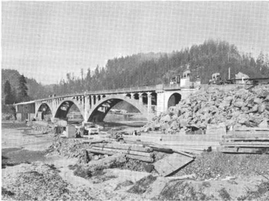
The Klamath River Bridge, looking south, shortly after it was opened to traffic. The steel trestle with timber deck is visible at the far end. The famous bears at each end of the bridge survived the flood.
