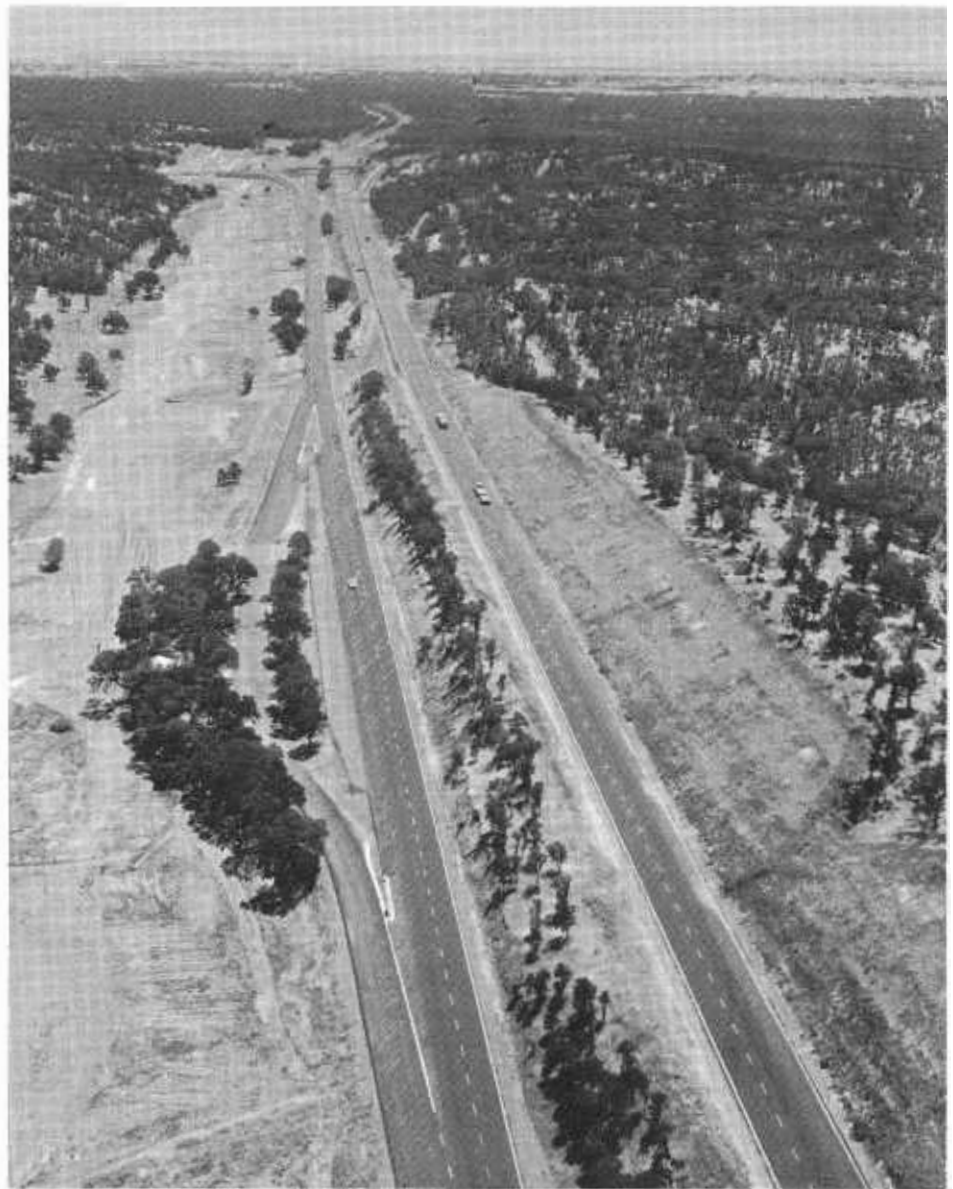
A pleasant group of native oak trees furnish a natural and comfortable roadside rest along this section of Interstate 5 in Tehama County. Facilities include a comfort station, chilled drinking water, and picnic tables and benches.
