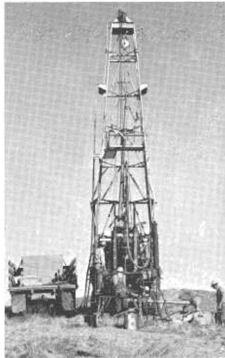
Drilling crews sample subsurface materials for foundation exploration.
