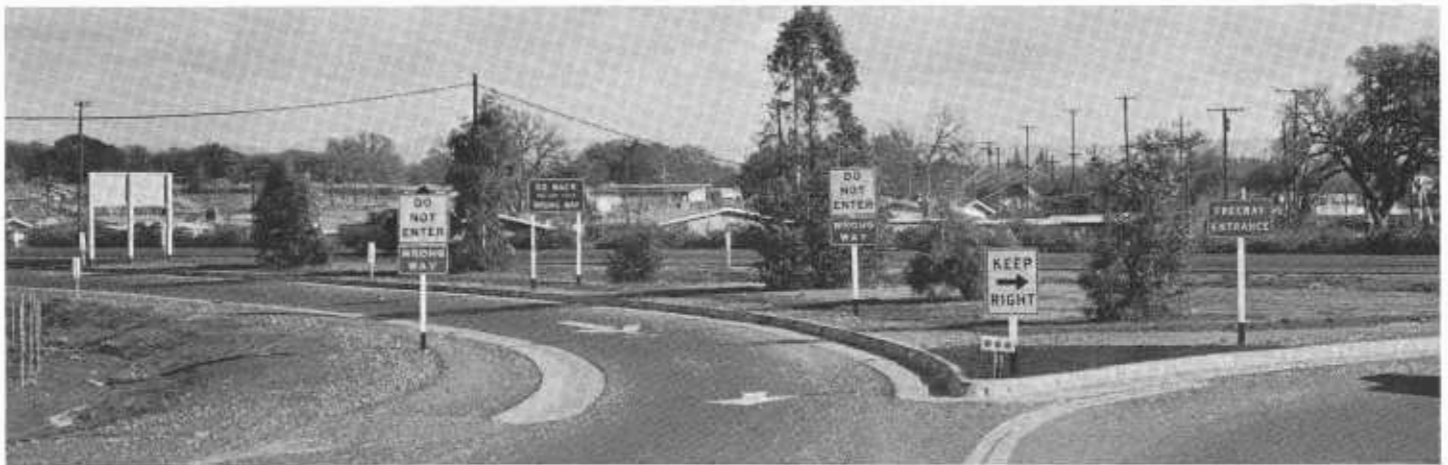
A detailed analysis is being made of the design of off-ramps and the effectiveness of traffic control signs and devices to determine whether certain features discourage wrong-way entry more than others.
