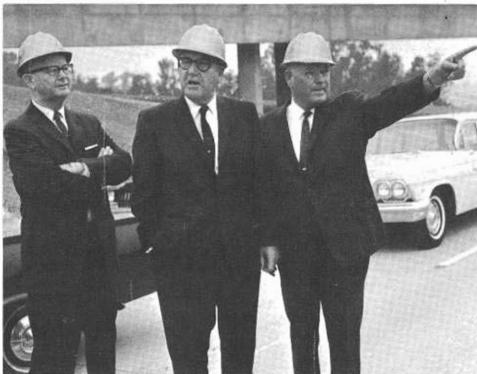
An on-the-spot inspection by Governor Edmund G. Brown of new MacArthur Freeway construction in Oakland took place in October. He was accompanied by (left) Alan Hart, district engineer, and (right) Gordon Ball, the contractor whose firm accomplished the construction. The Governor cited the fact that vehicles that travel the new stretch of approximately four freeway miles in lieu of city streets save eight minutes.
