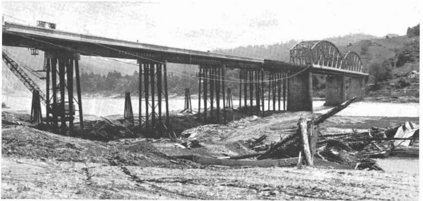
The reconstructed Eel River Bridge at Rio Dell was opened to traffic in May 1965. (See next photo.)
