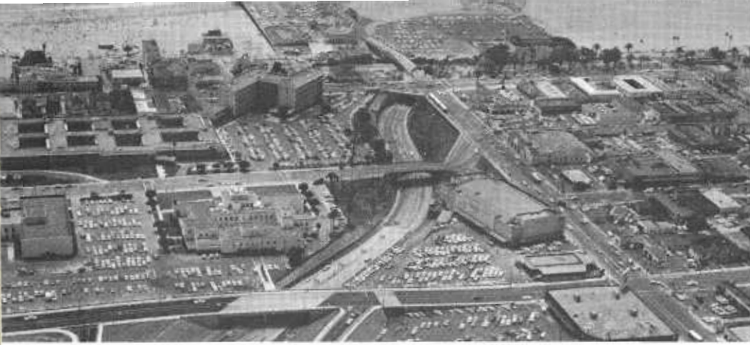
The recent opening of the Santa Monica (I-10) Freeway between Bundy Drive in West Los Angeles and the Pacific Coast Highway (Route 1) at the Santa Monica Tunnel (center) completed this freeway between the East Los Angeles Interchange and the Pacific Ocean.
