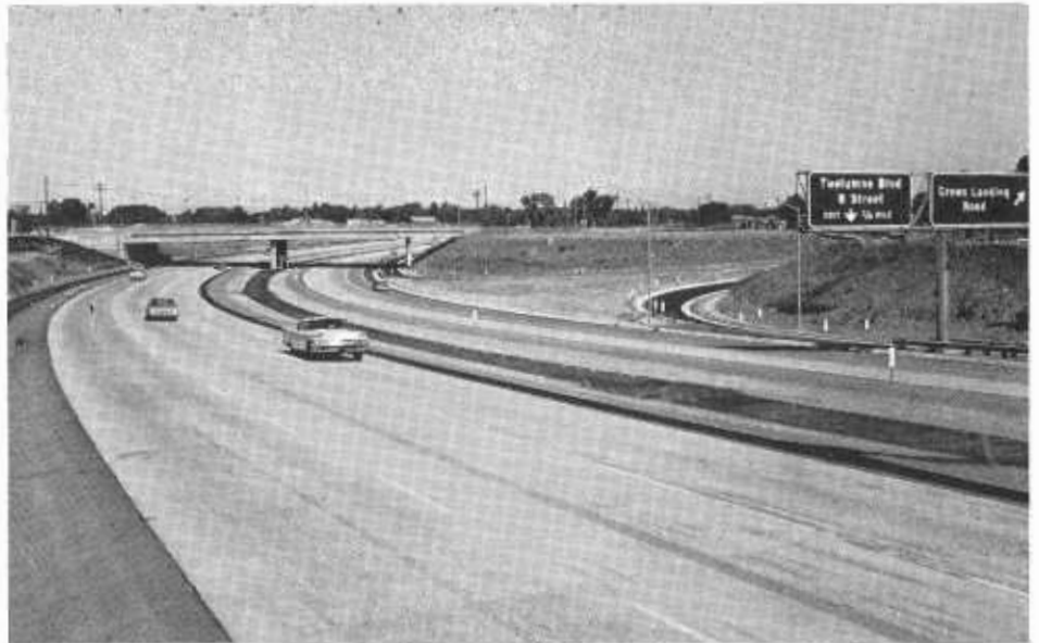
The freeway now carries with ease twice the volume of traffic which formerly bogged down by congestion on Modesto's Ninth Street.
