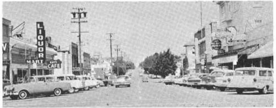
BEFORE: Main Street in Rio Vista prior to widening and reconstruction. The street had two lanes and diagonal parking. (Photo by J. B. Andrew)
