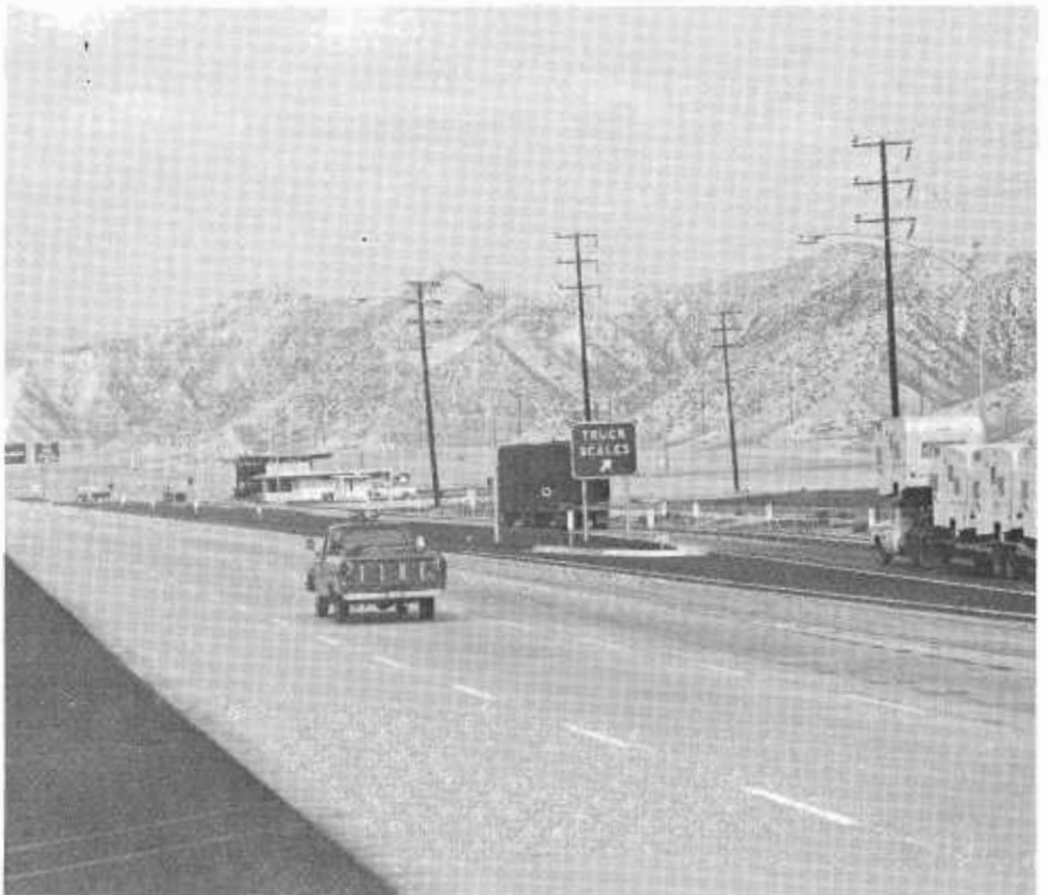
The new California Highway Patrol truck scales went into operation last January near the Interstate 5-Route 126 interchange. (See map previous page)
