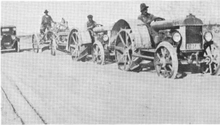
A Division of Highways' maintenance crew used two Fordson tractors to tow a grader in 1924. The Dodge at left is in "step" with those times.
