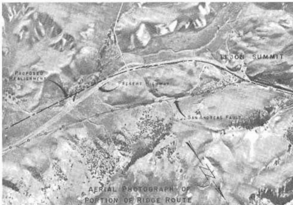
A vertical aerial of the Tejon Summit area shows the present highway and a section of the proposed realignment. Line with circles shows location of the San Andreas Fault through this area.
