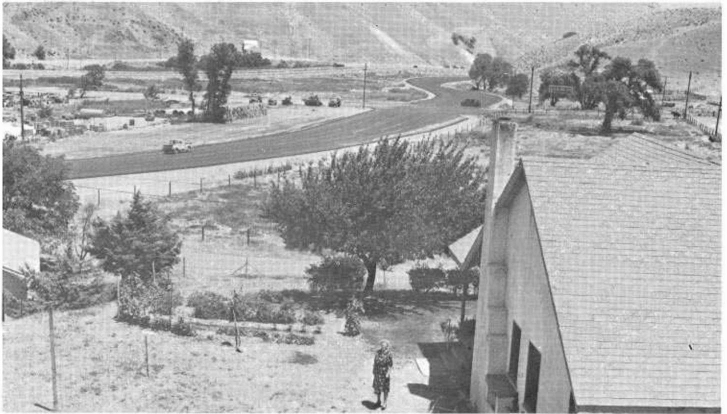
The Ralphs' ranch house today overlooks massive construction activity on the new Interstate 5 Freeway. Mrs. Mary Ralphs stands in the front yard.
