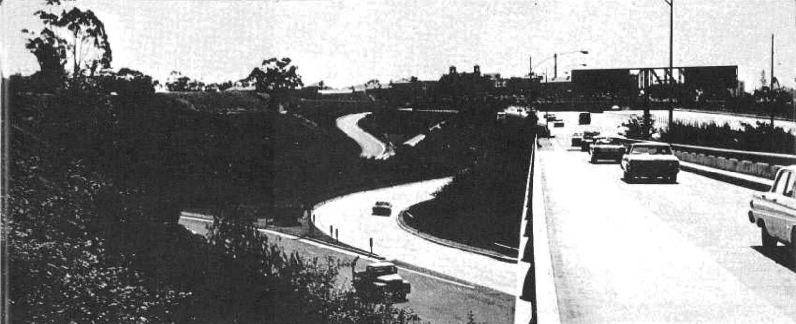
An outstanding feature of I-5 is the fully landscaped four-level interchange with Route 395 in Balboa Park.
