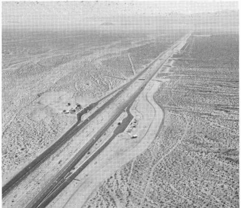
Aerial panorama of the Halloran Springs Roadside Rest areas. View is westerly down Baker Grade toward Soda Dry Lake.
