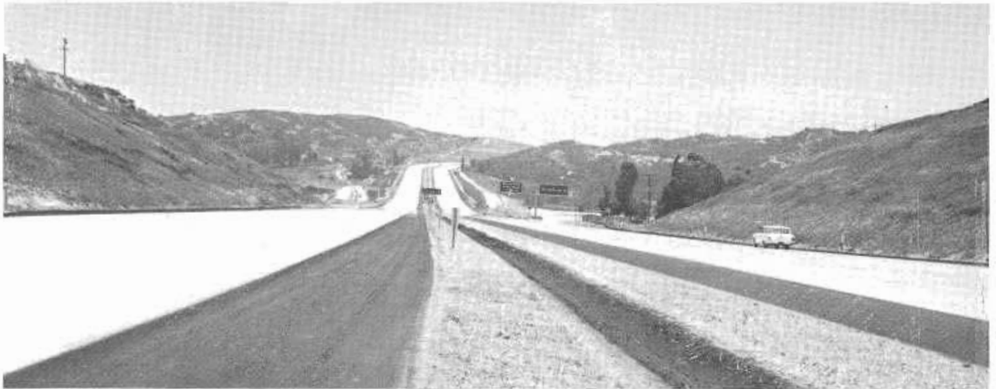
A section of the new freeway just prior to its being opened to traffic.
