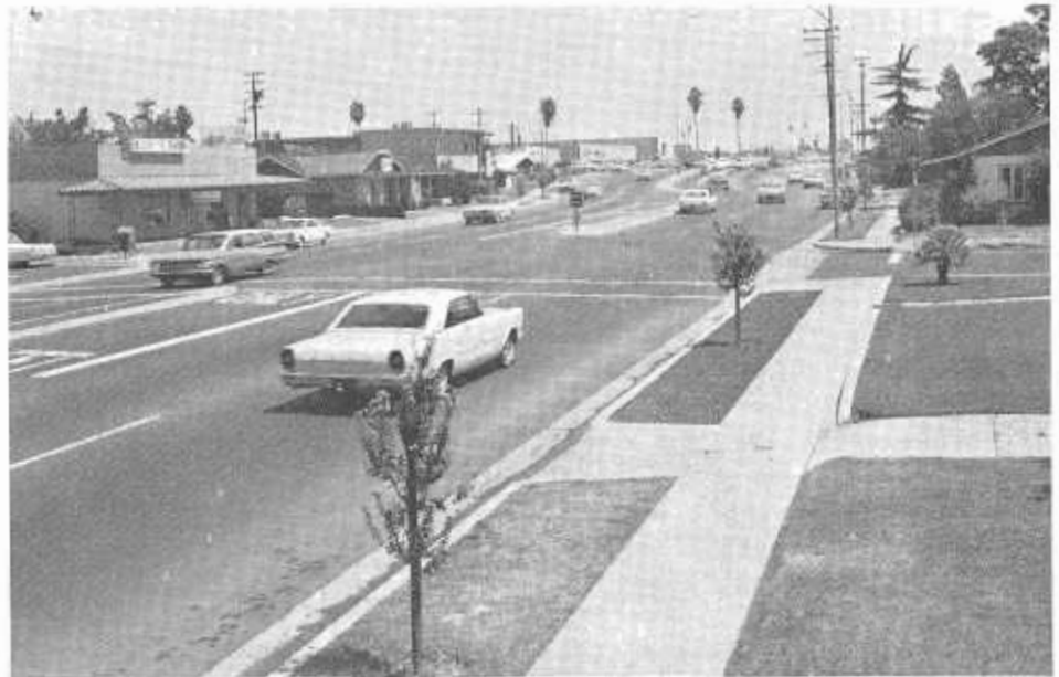
Shields Avenue in the City of Fresno after its widening to a four-lane, divided roadway.
