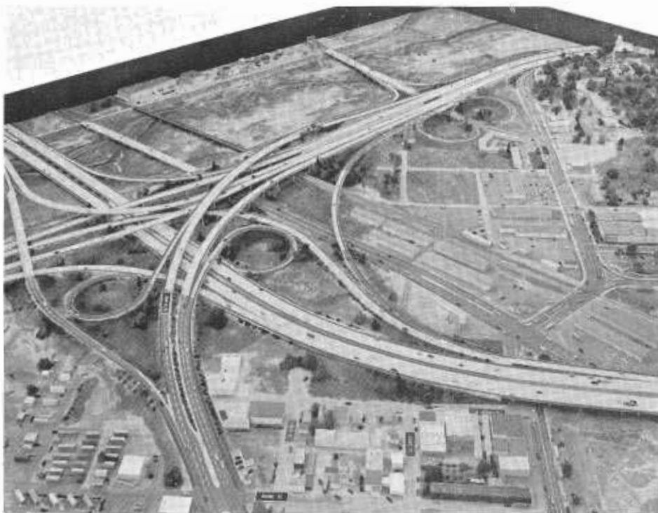
For design study and public information purposes, the Bridge Department constructed the Interstate 5 and 8 interchange in model form.
