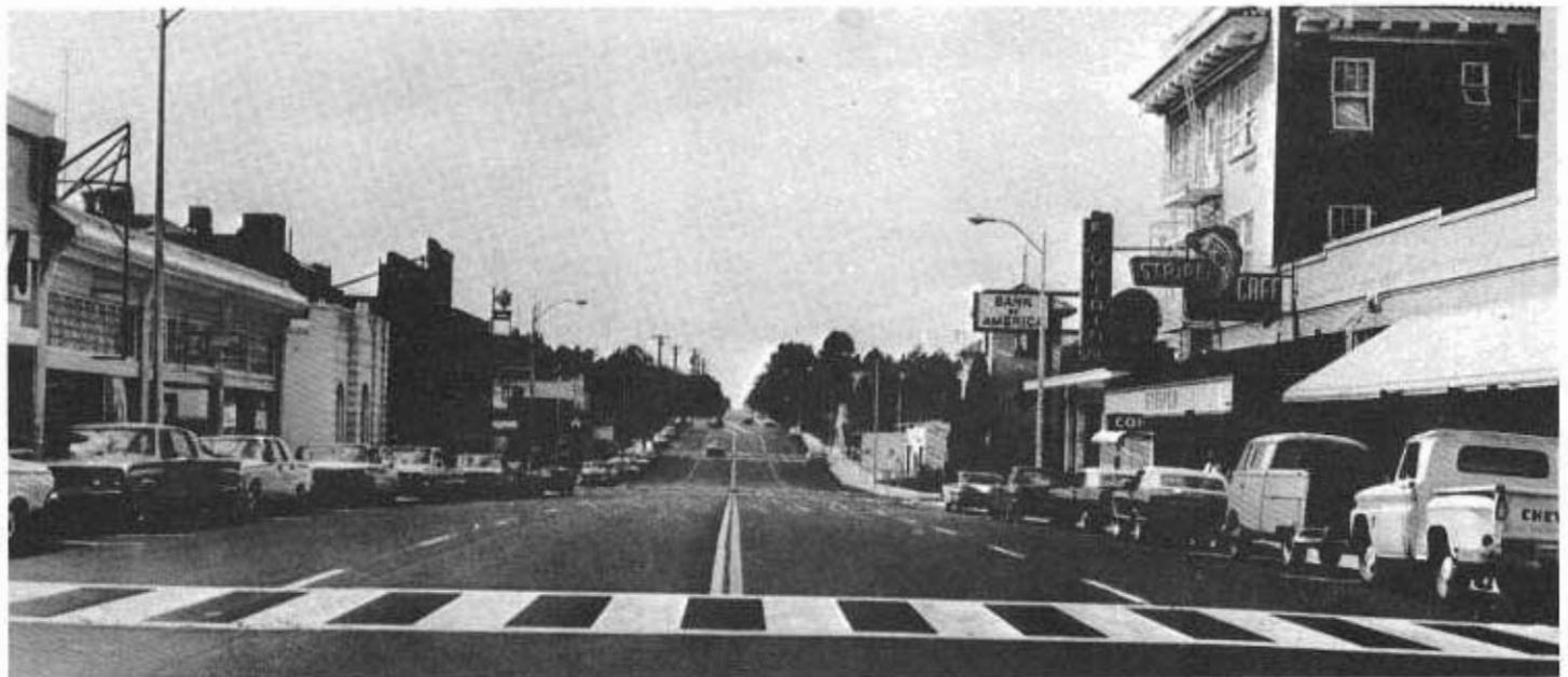
AFTER: Main Street in Rio Vista following reconstruction. A wider roadway and parallel parking have given enough space for four lanes of traffic. (Photo by River News-Herald)
