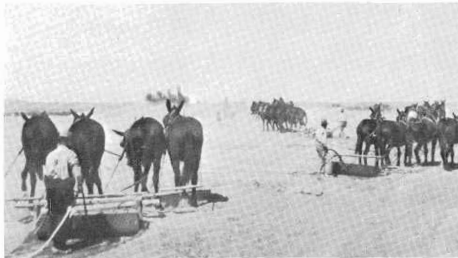
Much of the roadway excavation during early construction was accomplished with mule-drawn fresnos.
