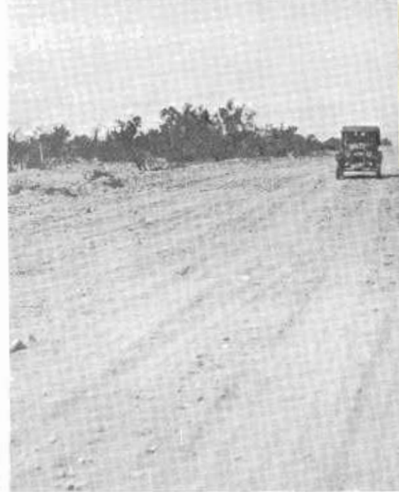
An early view of an improved section of the Arrowhead Trail after the ruts had been dragged smooth and tire-puncturing rocks removed. Speeds of 35 miles per hour could be attained.
