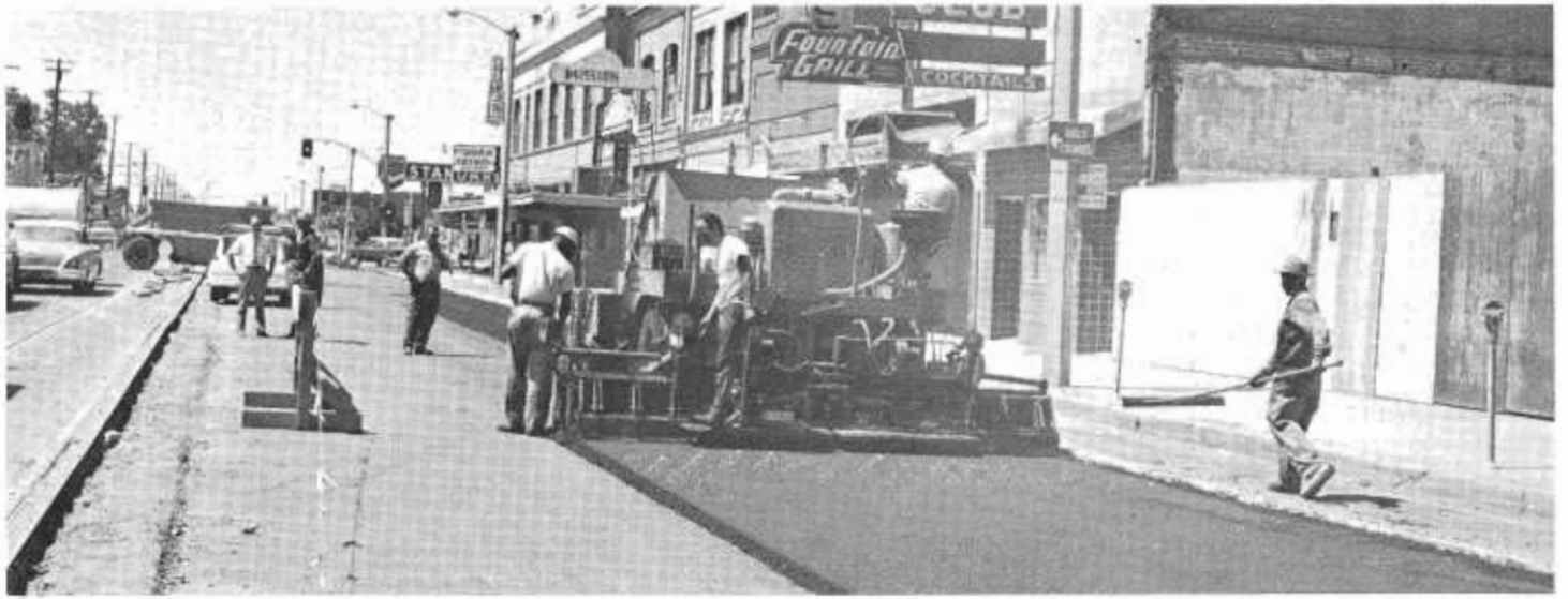
Old Highway 99 (Ninth Street in Modesto) was resurfaced by the state prior to relinquishing a portion to the city to become a part of the downtown commercial core.
