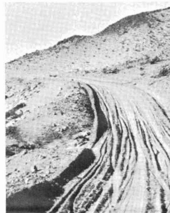
A view of the unsurfaced Arrowhead Trail west of Cronese Dry Lake in 1927. Rocks, removed from the traveled roadway as tire hazards, are visible at left.
