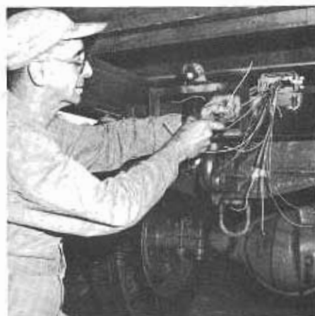
Changing wiring on snow-going machines to synthetic rubber jacketing has prevented freezing and corroding that once made lights inoperable.
