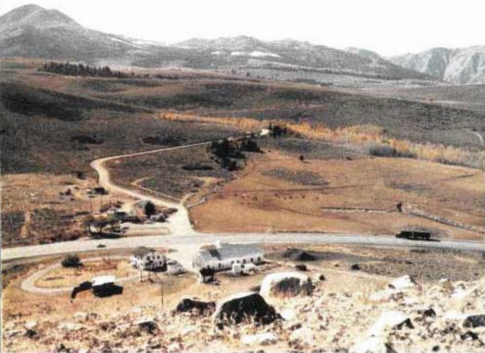
Conway Summit maintenance station, elevation 8,138 feet, lies east of the main Sierra ridge (background) above Mono Lake. North-south traffic on U.S. 395 (foreground) is dependent upon clearing operations of this District 9 station when snows come.
