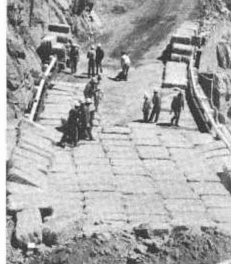
Upper left: When blasting was necessary near contractors' and resident engineers' office complex, contractor placed big dump trucks as shields for office trailers. Above: Photo made in 1964 on middle Tioga Pass job shows baled hay used on old sidehill viaduct to protect it from rocks thrown in blast.
