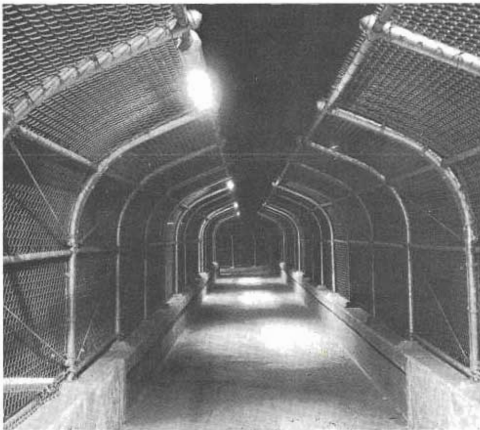
A night view of a pedestrian overcrossing lighted by one of the new fluorescent fixtures.
