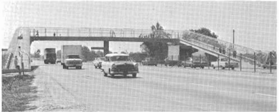
The Tweedy Lane pedestrian overcrossing in Los Angeles with the new-style fluorescent luminaires in the chain link sidewalk railing.
