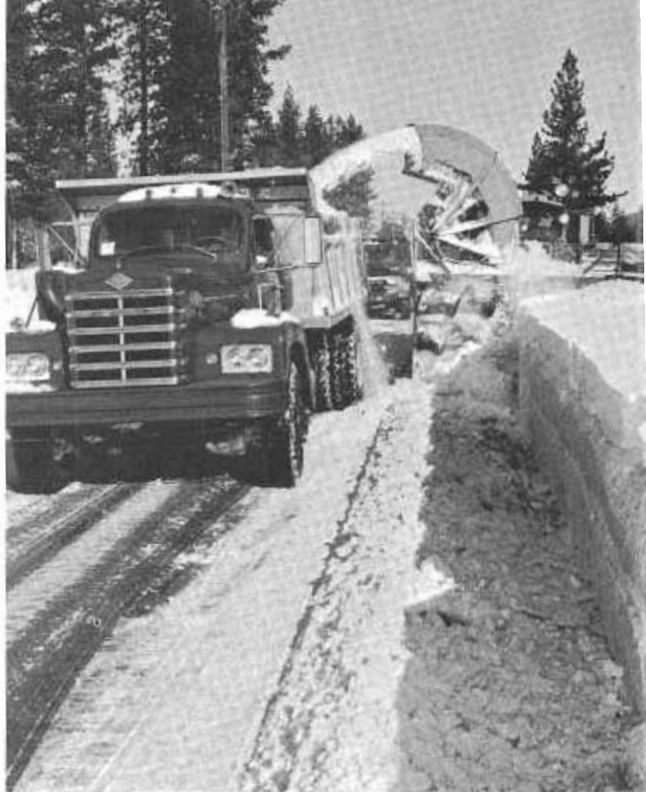
In areas without wide medians for snow storage, rotary plows funnel their intake into waiting snow loaders. The loaders then proceed to other areas where they deposit their winter bounty.
