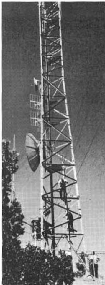
On left is one of six radio repeater stations in the District 3 network. Built on mountain peaks, these units support antenna and reflector dishes sending radio and microwave signals to highway units in 11 counties. Mrs. June DeVore, dispatcher (above), gives complete road/weather information to field workers and highway officials using a three-way combination of telephone, VHF radio and microwave.
