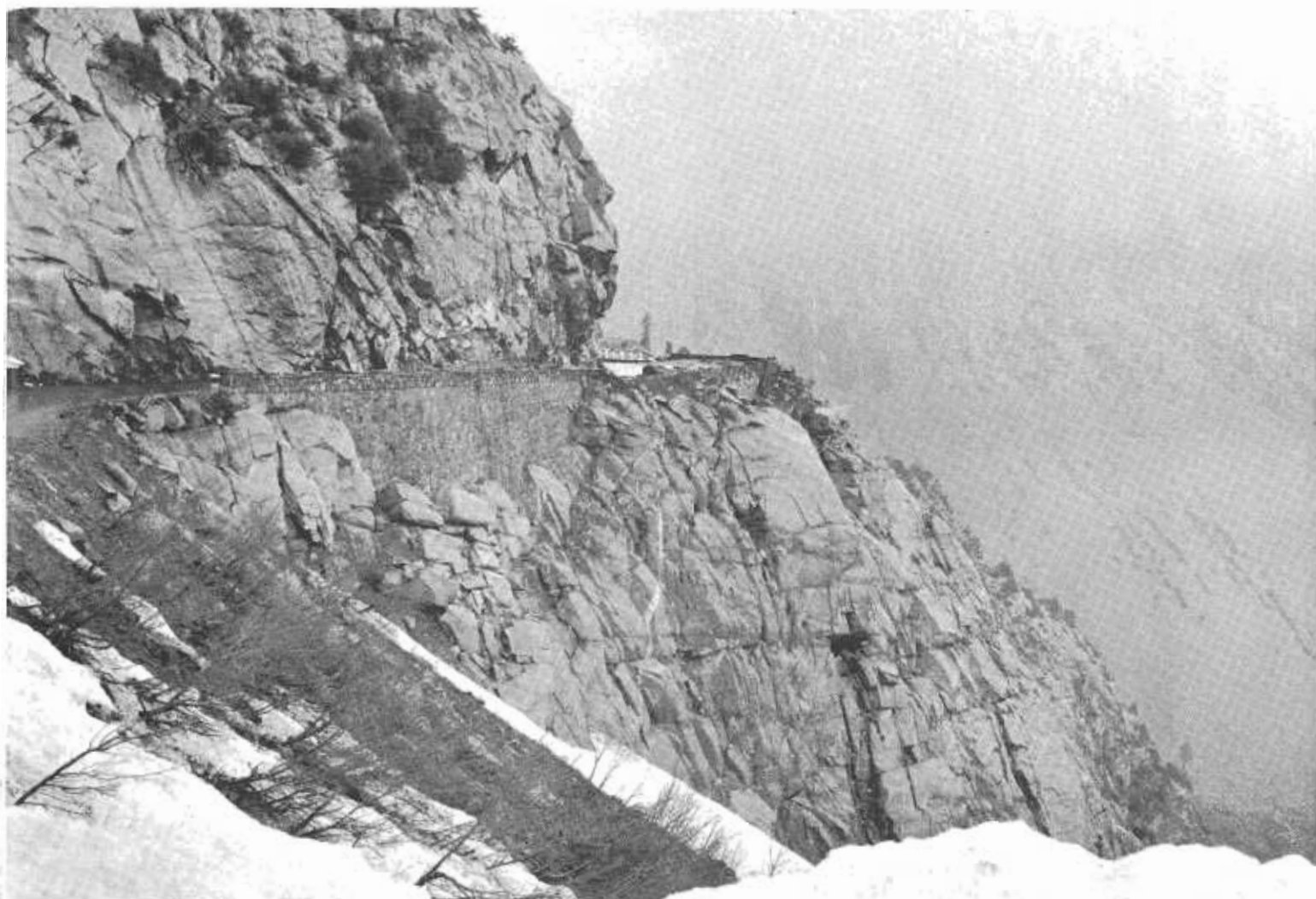
Section of State Route 120, Tioga Pass Road, made in spring 1963, before contractor began work. Curve in center of photo rounds Dodge Point, with sidehill viaduct just beyond. Contract now completed has widened road here, and provided viewpoint.
