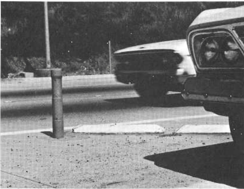
A popup in raised position. Made of flexible plastic, it can be hit by an auto with no damage to the vehicle and little or no damage to itself.
