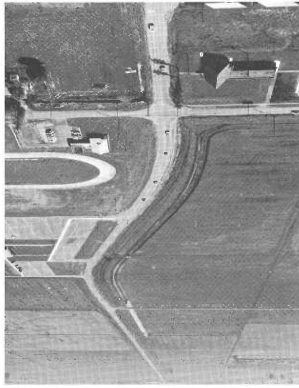
NEW AND OLD. Photo above—the new, four-lane, divided section of Santa Fe Drive from above G Street and looking west. El Capitan High School is to the right. A portion of Merced is visible left background. Photo right—the old, two-lane highway looking from approximately the same spot as the photo above.
