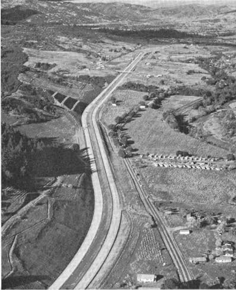
(Left) Looking north over new freeway section toward Calpella and Redwood Valley
