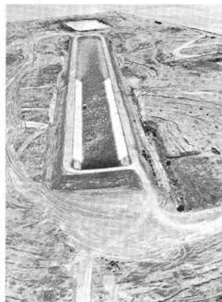
An aerial photo of a prototype test canal built by the Department of Water Resources some 15 miles south of Mendota. Note concrete-lined and earth-lined portions.
