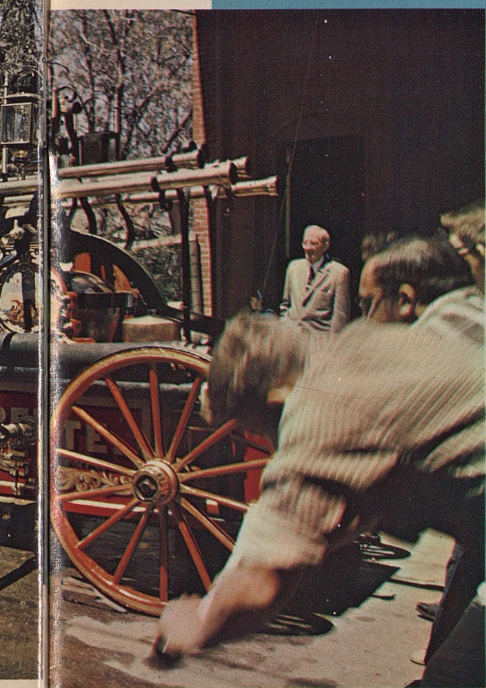
With 20 men on the handles (center photo) Papeete's outlet hose is filled hard as a rock, and stream from her nozzle outcarries that of a modern commercial pumper despite its dials and big engine.
