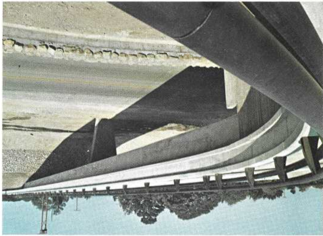
Above: This structure combines a liberal use of rubble masonry in abutment retaining walls, with heavily textured abutment and pier faces, sloping girder sides and an anodized aluminum railing. (Farrington Road Overcrossing in Monterey County.) Below: Sloping sides on the girders, tapered columns and long sweeping lines combine to give grace to this section of elevated freeway. Beneath is a huge area which may be used for a variety of purposes. (Fort Sutter Viaduct in Sacramento.)
