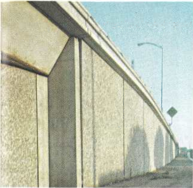
Above left: To add interest to long areas of retaining wall face, exposed aggregate panels were specified. The exposed pebbles are about 50 percent white, with the remainder ranging from light gray to black. (Fort Sutter Viaduct in Sacramento.) Above right: Here an interesting texture relieves what would have been a plain smooth face of concrete on these bridge piers. (The American River Bridge at Sacramento.)
