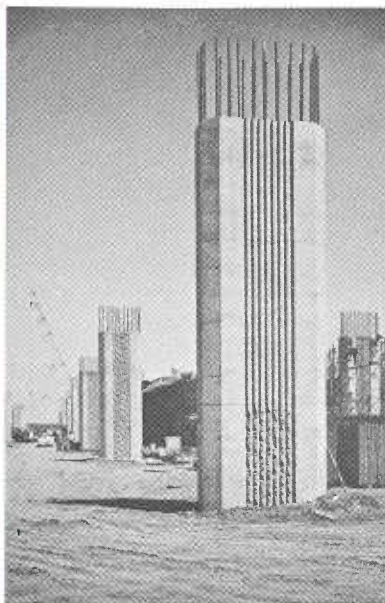
Above left: To add interest to long areas of retaining wall face, exposed aggregate panels were specified. The exposed pebbles are about 50 percent white, with the remainder ranging from light gray to black. (Fort Sutter Viaduct in Sacramento.) Above right: Here an interesting texture relieves what would have been a plain smooth face of concrete on these bridge piers. (The American River Bridge at Sacramento.)
