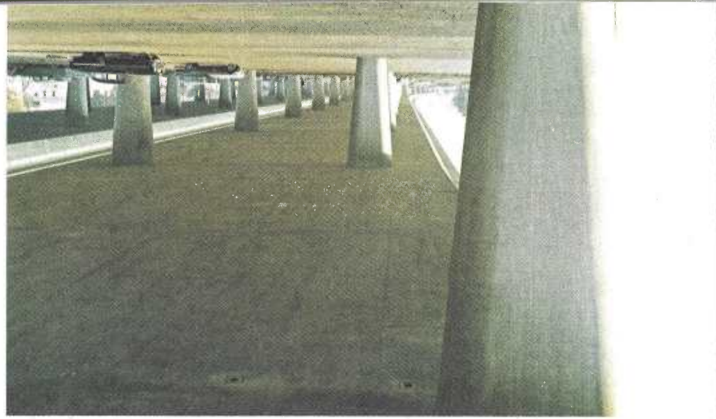
Above: This structure combines a liberal use of rubble masonry in abutment retaining walls, with heavily textured abutment and pier faces, sloping girder sides and an anodized aluminum railing. (Farrington Road Overcrossing in Monterey County.) Below: Sloping sides on the girders, tapered columns and long sweeping lines combine to give grace to this section of elevated freeway. Beneath is a huge area which may be used for a variety of purposes. (Fort Sutter Viaduct in Sacramento.)
