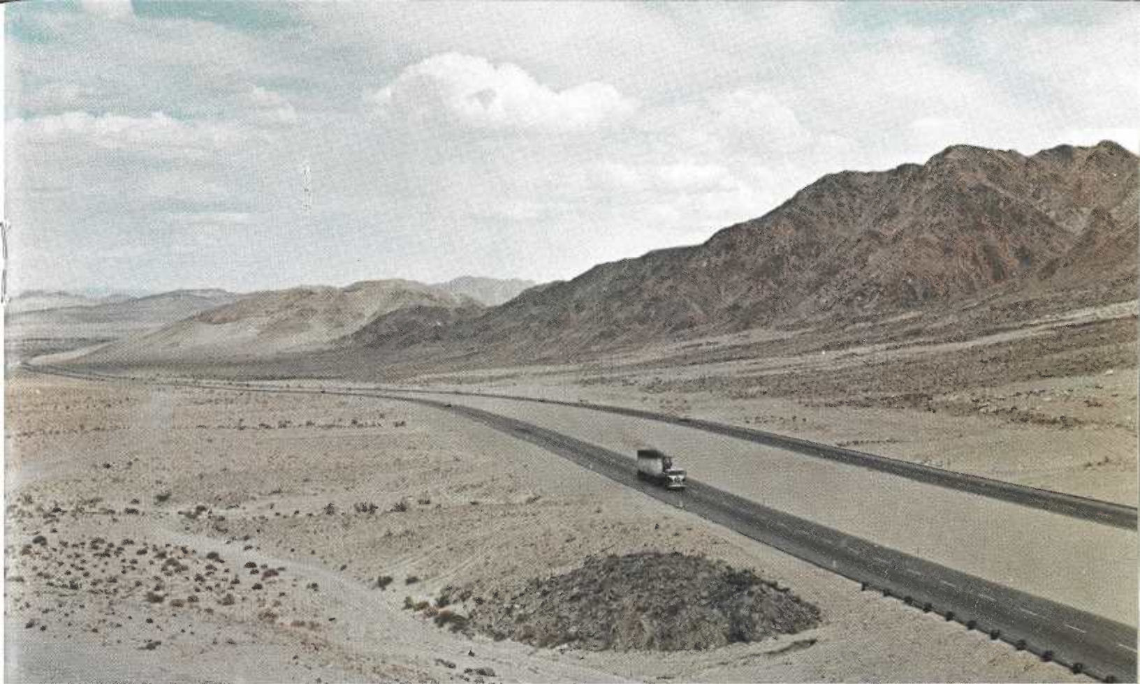
Above: Interstate Route 15 in San Bernardino County. The highway location is well matched to the terrain.
