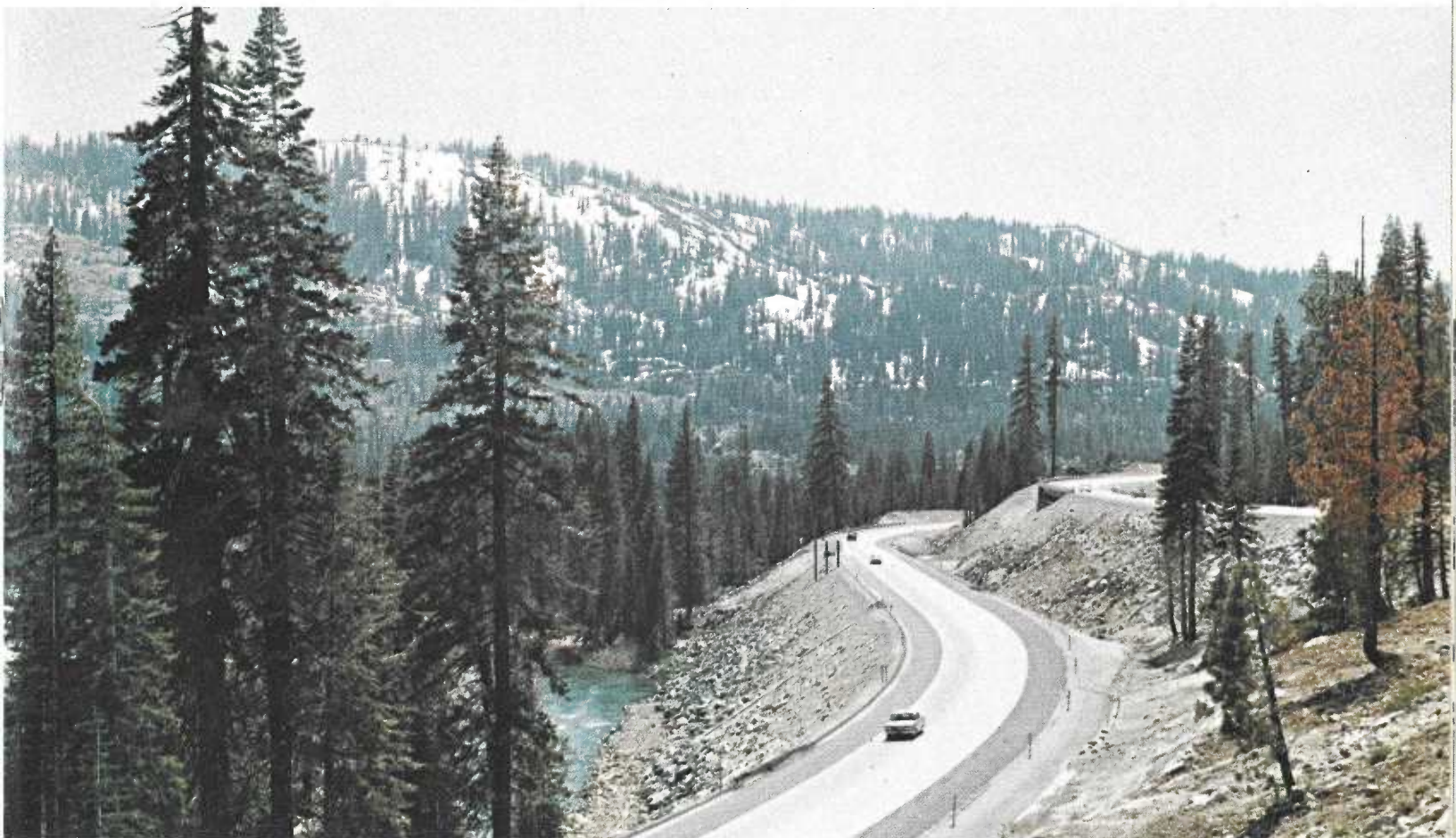
Below: Split level design on Interstate 80 in Nevada County. Native vegetation has been retained in the median. The majesty that is the high Sierra is more easily enjoyed through the use of this free flowing alignment leading the traveler over Donner Summit.
