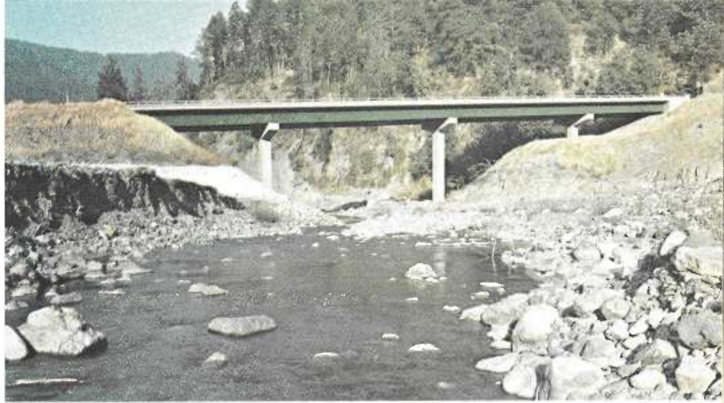
A welded steel girder structure which won a steel contest award in 1966 for its clean, simple lines. (Willow Creek Bridge in Humboldt County.)
