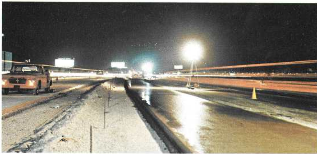
Above: Paving machine operator checks area just ahead of slipform. Below: Slab of freshly poured concrete stretches out behind paver in distance. Completed section at left of excavated median.
