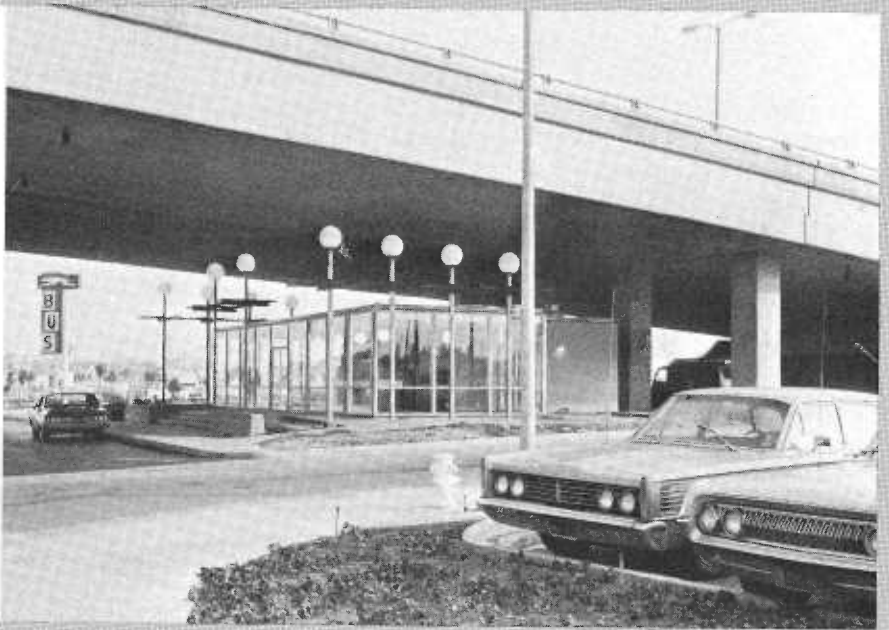
New passenger waiting and freight and luggage storage facilities located beneath Mathilda Avenue overhead.
