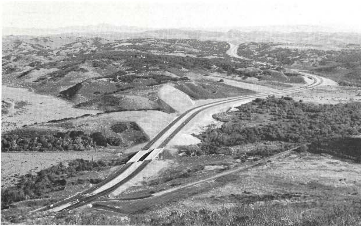
View of new highway, south end looking north.
