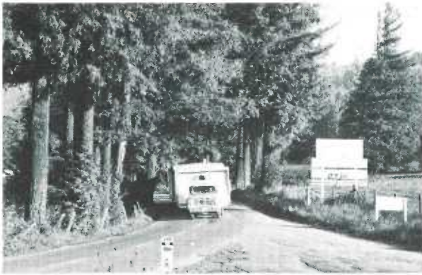
This narrow section and bad alignment on US 290 in the north-western part of the state is typical of the hundreds of such deficiencies which still exist not only on secondary state routes, but on major federal aid routes similar to US 290.
