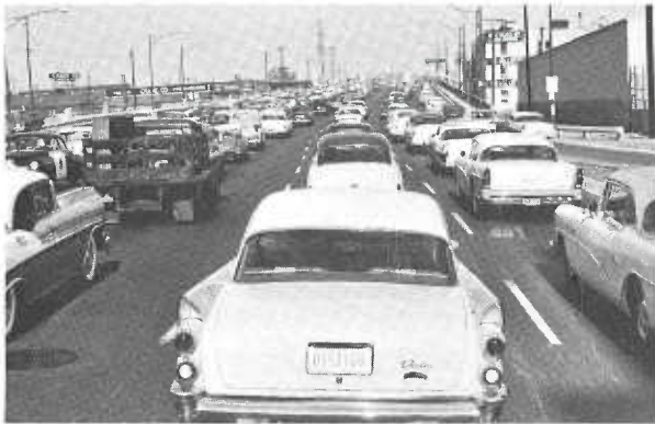
An older freeway section in Los Angeles now carrying more than 150,000 vehicles daily.
