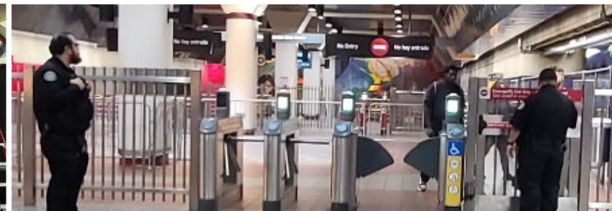
Faregate compliance pilot with updated entrance/exit pathways, upgraded wayfinding and layered staffing has improved customer experience
