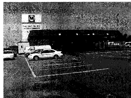
Fuel/Interior Cleaning Building
