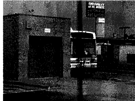
South Fare Recovery Building
