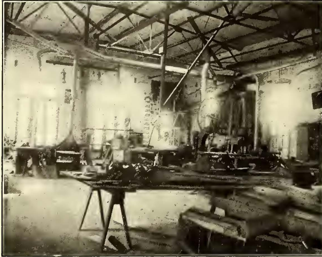
Mobile Repair Shops—Exhausters in the Mill Room
