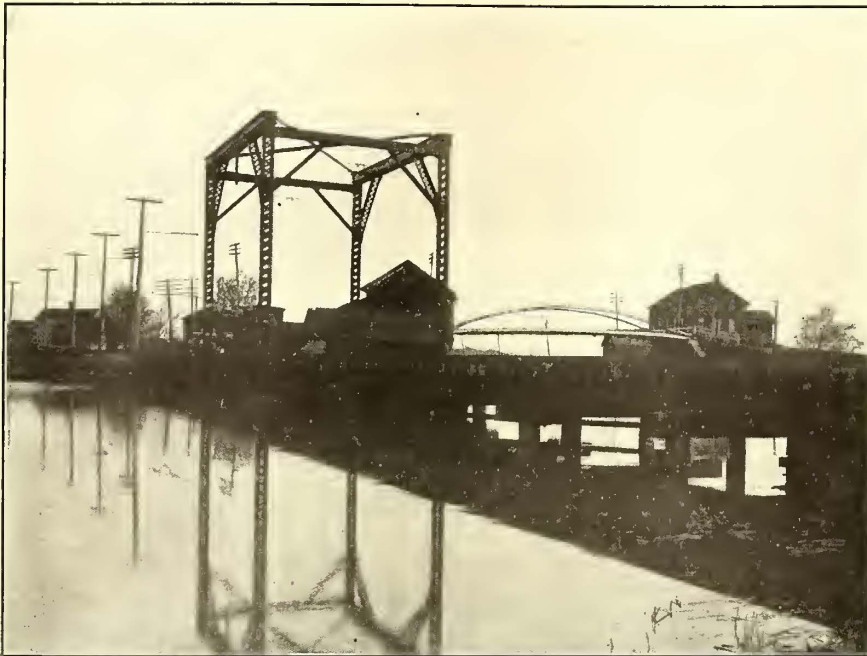
Buffalo, Lockport & Rochester—Lift Bridge at Holley
