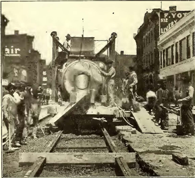
Pouring End of Concrete Mixer
