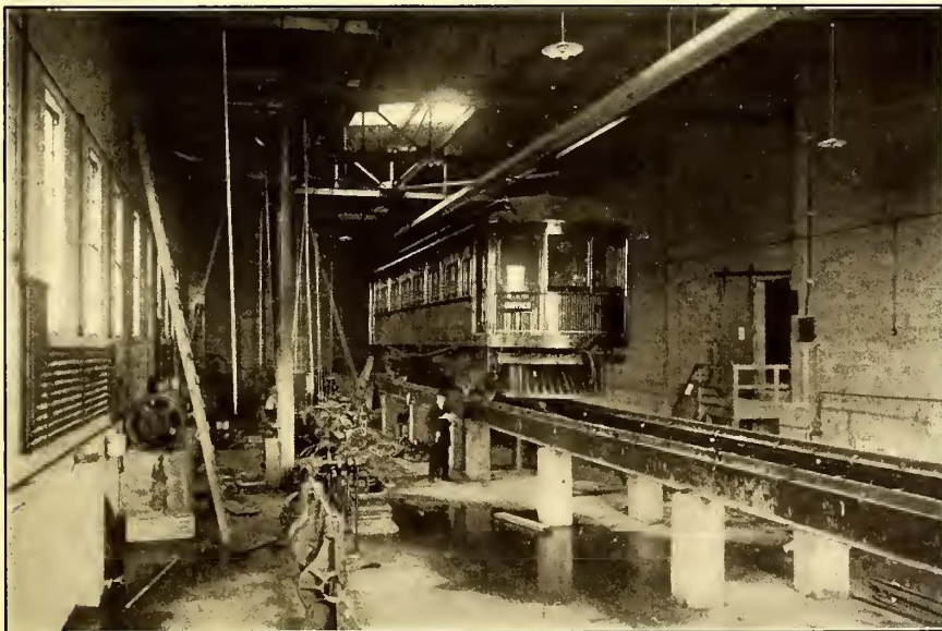
Buffalo, Lockport & Rochester—Depressed Shop Floor, Overhauling Track and Machine Shop Equipment
