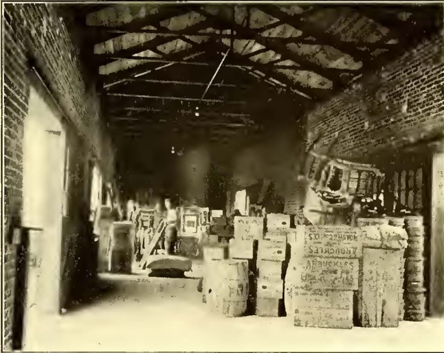
Interior of Freight House at Toledo
