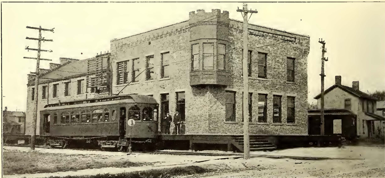
Youngstown & Ohio River Railroad—Substation and Office Building at Leetonia
