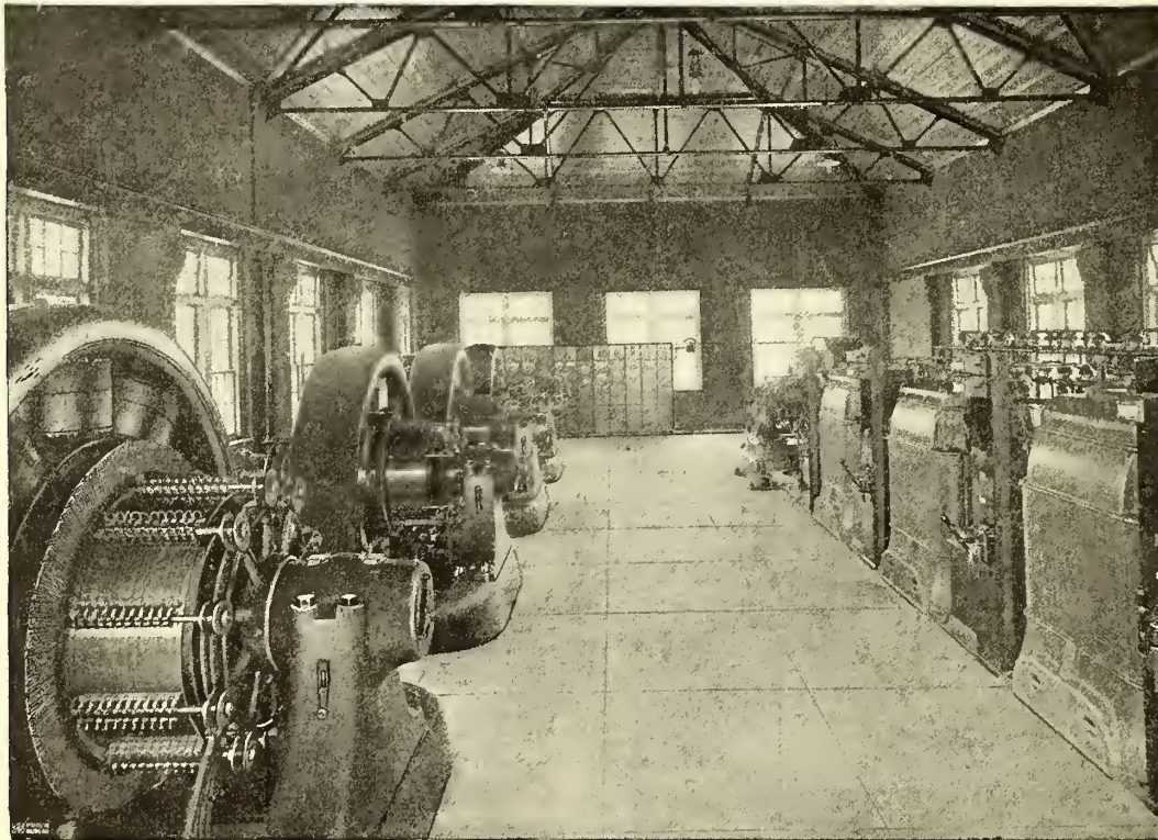
Fig. 4.—Converter Substations—Interior of Taunton Substation of Old Colony Street Railway Company
