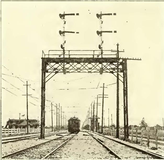
Pacific Electric Railway—Home Signal Bridge over Express Tracks at Slauson Junction
