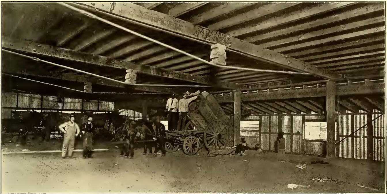
Philadelphia Ash Service—Wagons in Receiving Station Dumping Rubbish Into Cars Below
