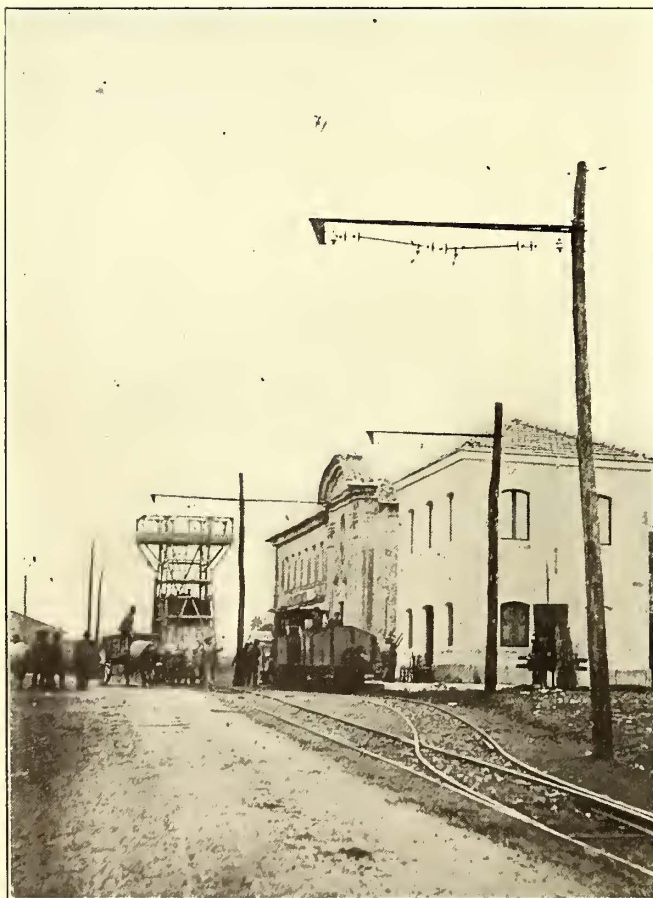
Rome Single-phase Railway—Wiring at Turnout.
