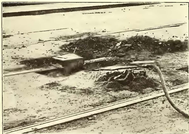
Thermit Rail Welding—Melting Out the Wax with Gasoline from Preheater
