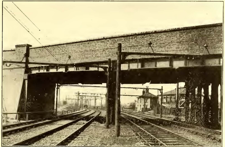
Midland Railway Single-phase Electrification—Four-track Under-crossing at Morecambe, Illustrating the Use of Wooden Guards between the Wires and the Steel Floor of the Bridge
