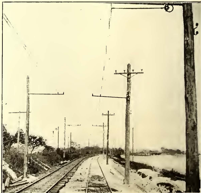
Annapolis Short Line—Double Track Construction
