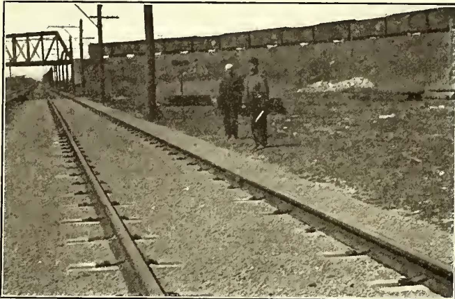
Concrete Tie—Section of Complete Track
