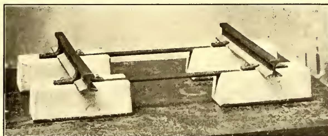
Concrete Tie—Blocks with Cross Tie Rods
