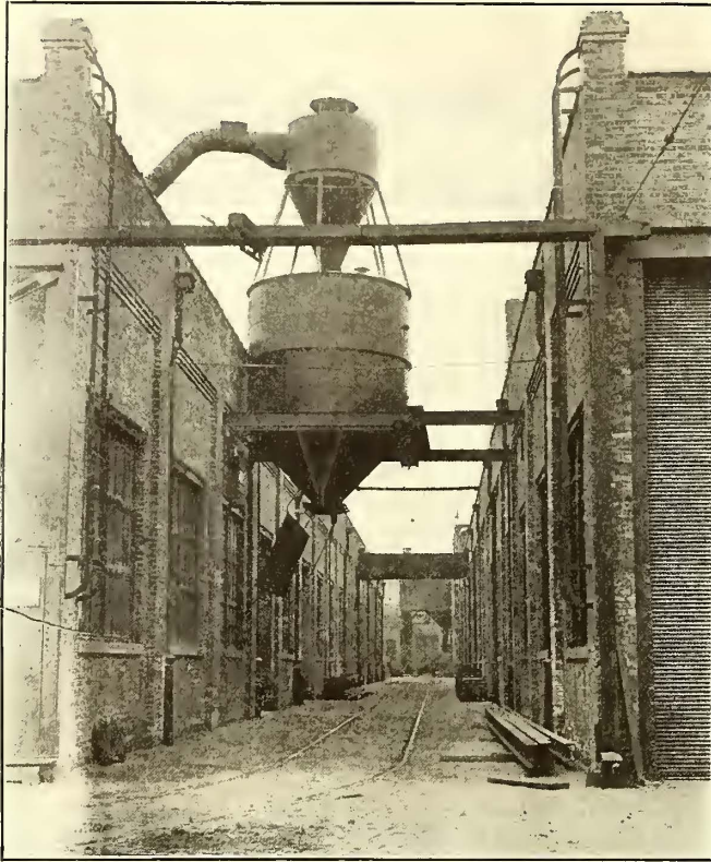
Chicago City Railway Shops—Storage Hopper for Refuse from Woodworking Machines
