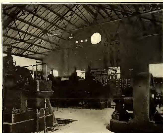
Olean Gas Power Plant—Interior of Station
