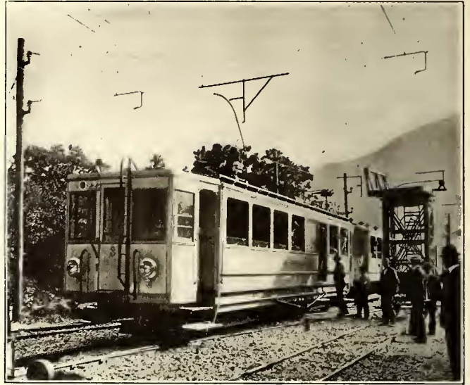
Locarno Single-Phase Line—Overhead Construction at Tunnel and at Turnout
