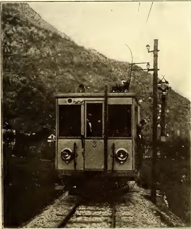
Locarno Single-Phase Line—Section Insulator and Breaker
