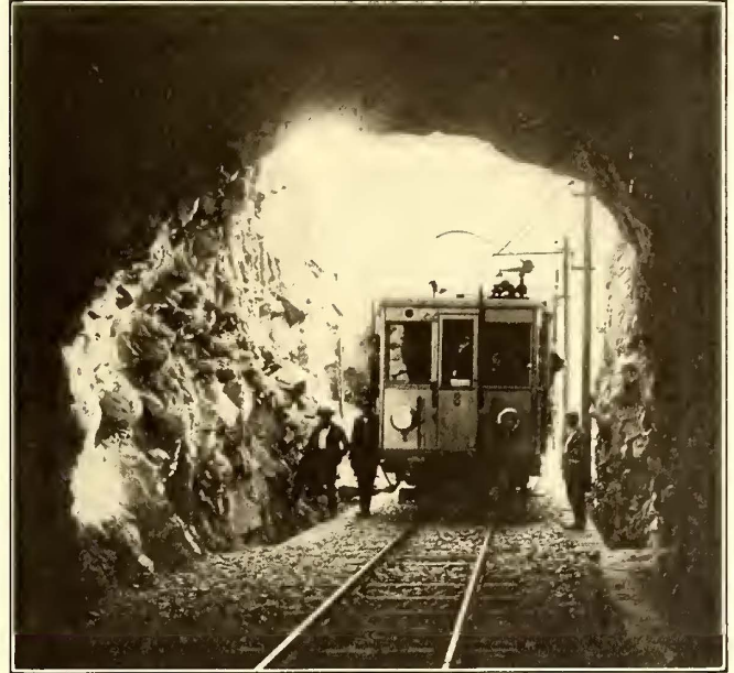
Locarno Single-Phase Line—Tunnel
