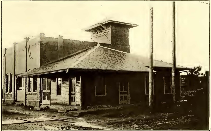
Texas Traction Co.—Substation and Waiting Station at Plano
