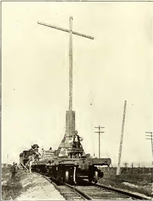
Texas Traction Co.—Steam Construction Train for Erecting Aluminum High Tension Feeders
