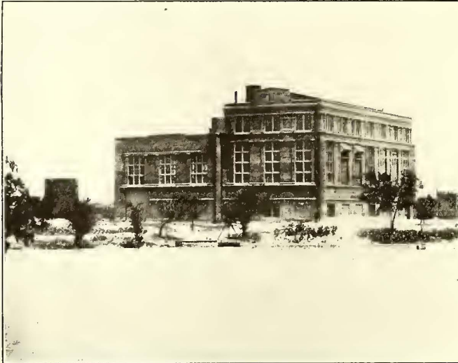
Texas Traction Co.—Power Station
